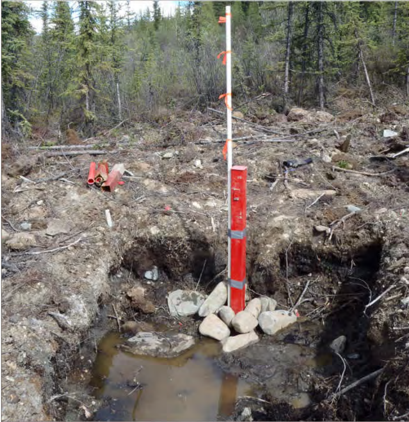
Photo 1: Repaired SI Installation – BH28. May 30, 2012.
