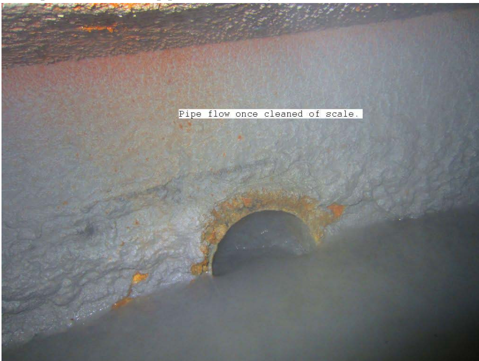
Cleanup Photo 3: Cleaned pipe within Primary mix Tank
