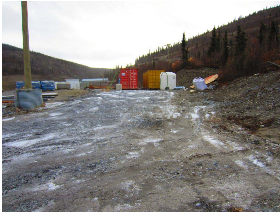
Cleanup Photo 1: 625 Ramp to Roadway
