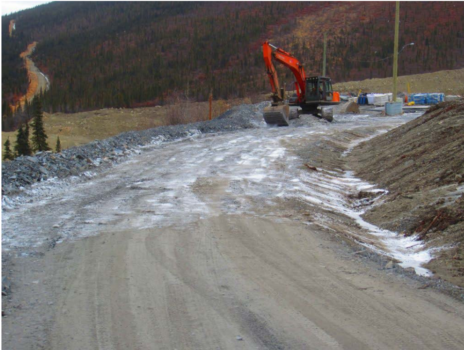
Cleanup Photo 2: Roadway to 625
