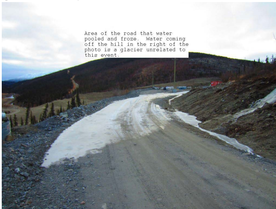
Spill Photo 4: Roadway to 625
