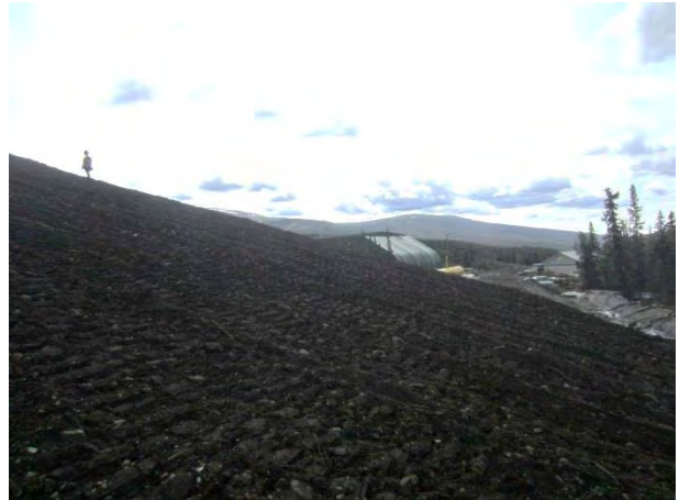
Photo 8: Covered DSTF mid-slope looking south
