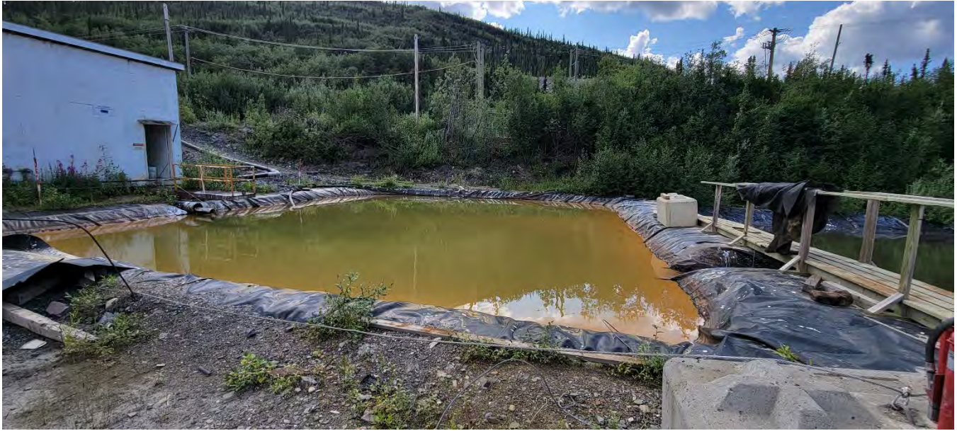
Photo 3: Bellekeno 625 Water Treatment Ponds, facing southwest (I. MacIntyre, July 20, 2023)
