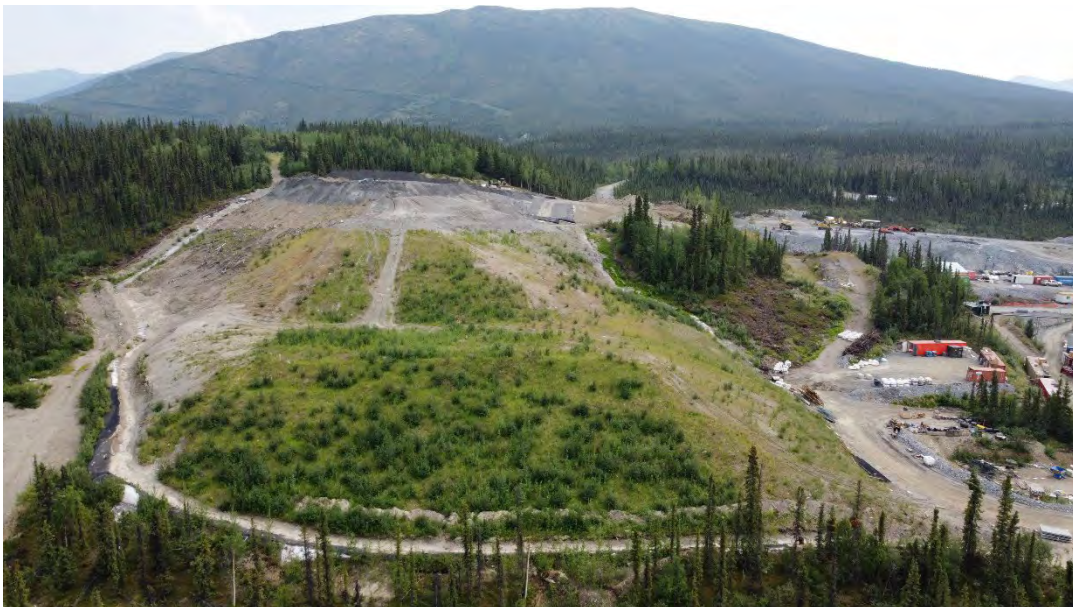
Photo 14: Photo 13: DSTF Phase 1 – aerial view facing east. (I. MacIntyre, July 22, 2023)
