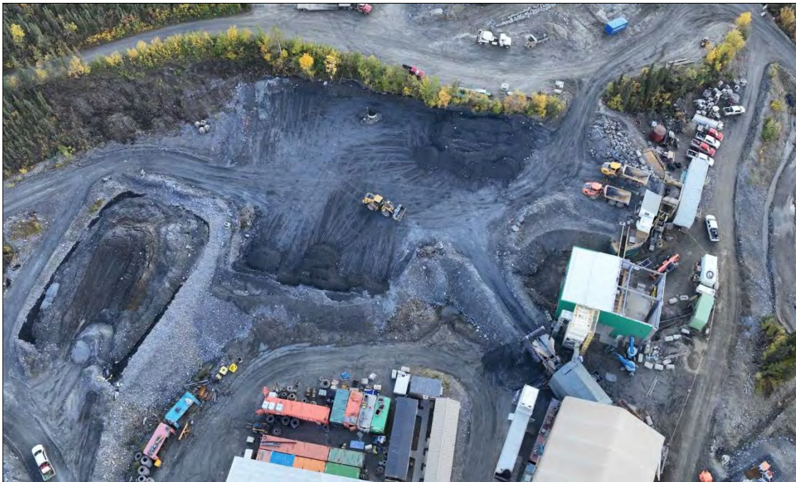
Photo 2-7: ROM and crusher under construction (September 2023)
