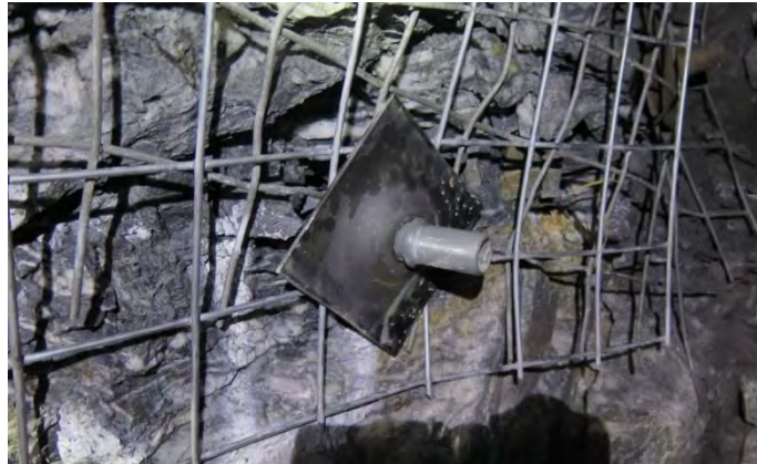
Figure 12. Corrosion-resistant coated Swellex friction set.
