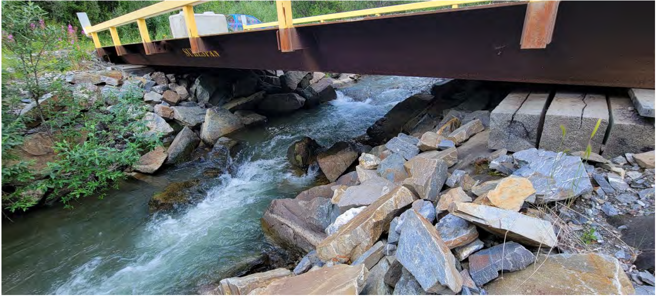
Photo 8: Lightning Creek Bridge – Onek Road (I. MacIntyre, July 20, 2023)
