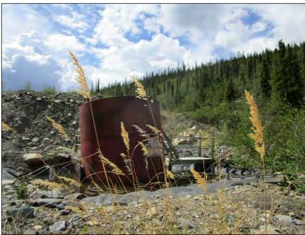
Photo 10-1: Bellekeno Fuel Tank Farm – 2021
