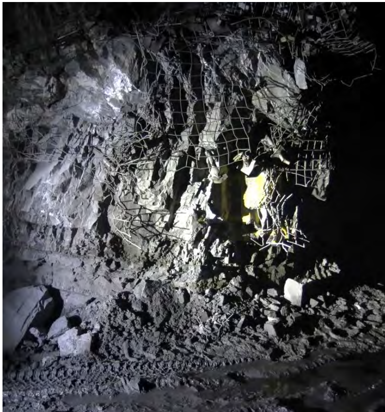
◀ Figure 8. Photograph showing substantial equipment damage on a nose pillar.
