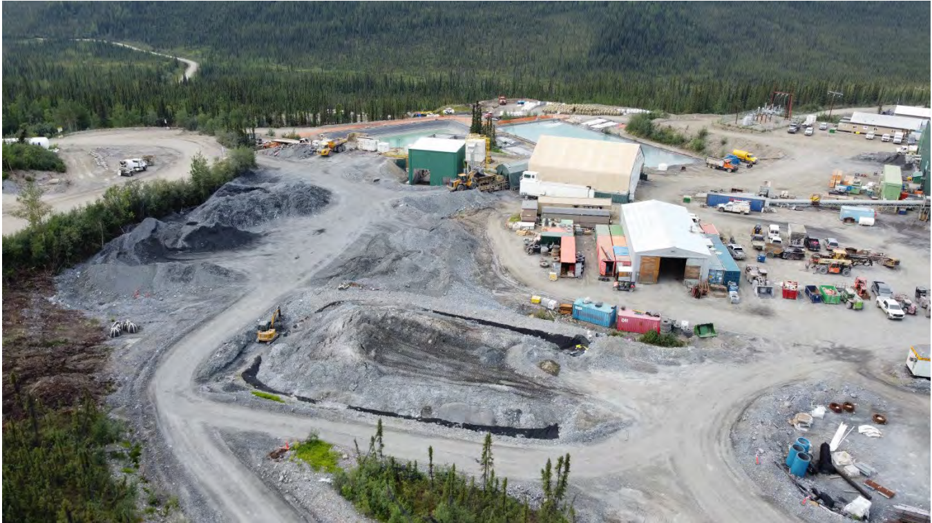
Photo 21: Flame and Moth PAG waste storage facility, aerial view facing west. (I. MacIntyre, July 20, 2023)
