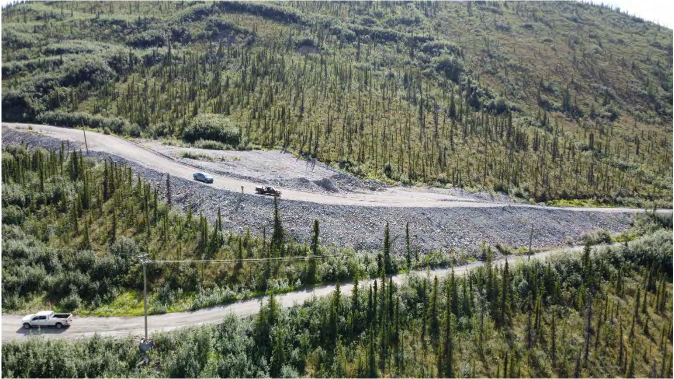
Photo 2: Bellekeno Road Waste Rock Pile, facing southwest (I. MacIntyre, July 20, 2023)
