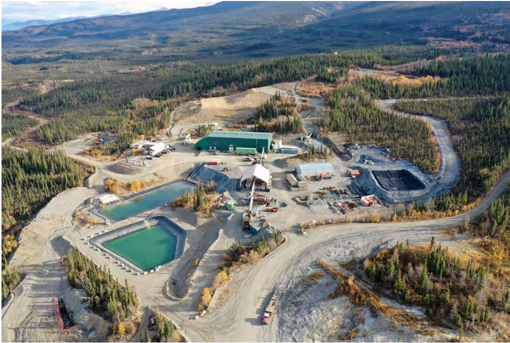
Photo 2-2: Flame & Moth and District Mill Area Overview
