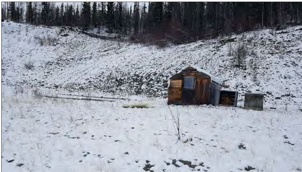
Photo 2-6: Onek 990 portal shed (October 2023)
