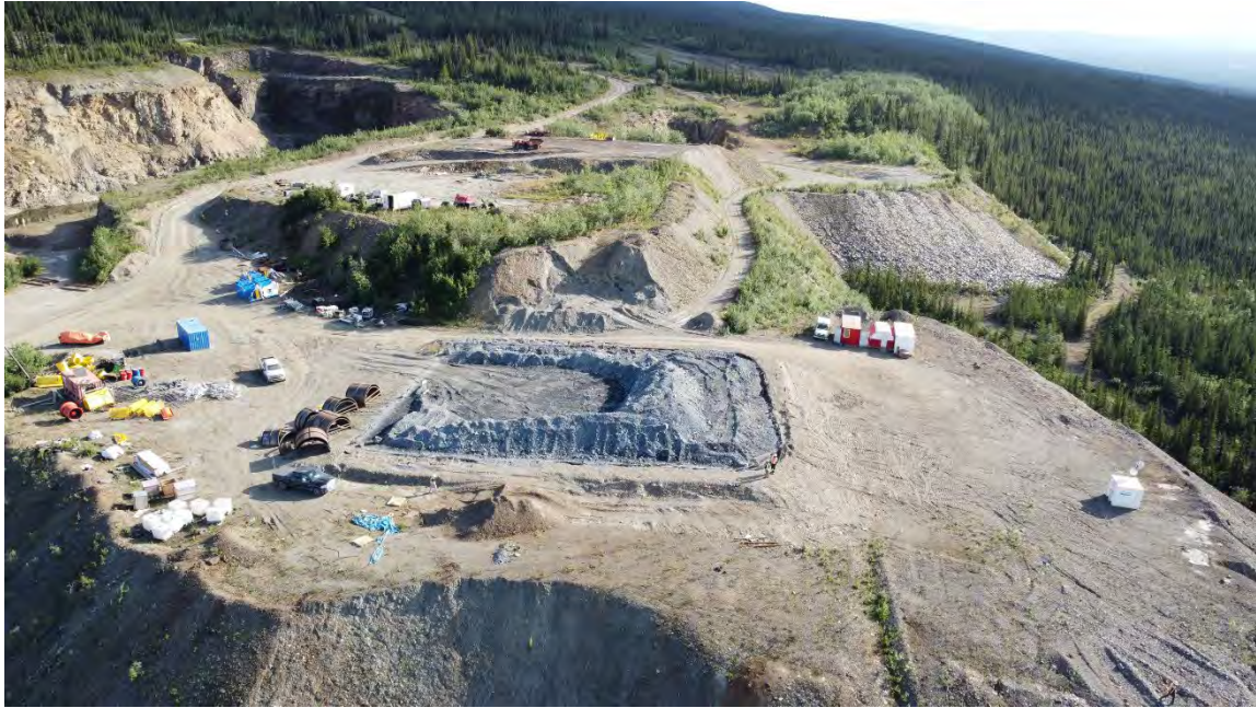
Photo 25: Bermingham PAG waste storage facility, aerial view (P. Johnson, August 30, 2022)
