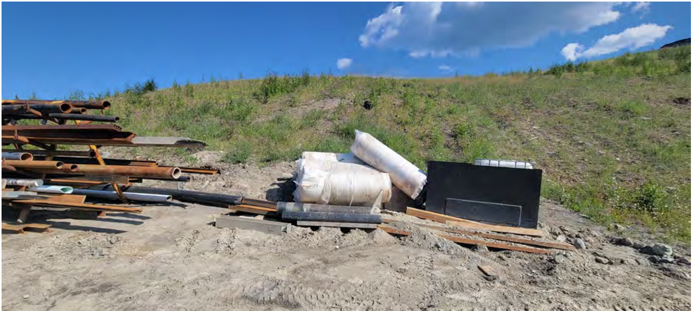
Photo 20: DSTF Phase 1 lower bench south slope. No runoff collection ditching present, possible buildup of debris along toe. Facing North. (I. MacIntyre, July 20, 2023)
