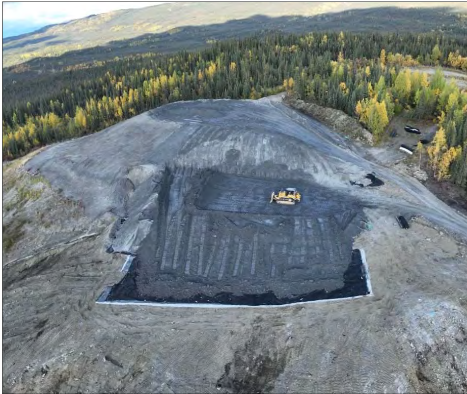
Photo 2-8: Phase 1b DSTF (September 2023)
