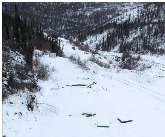
Photo 10-2: Bellekeno Fuel Tank Farm – 2023
