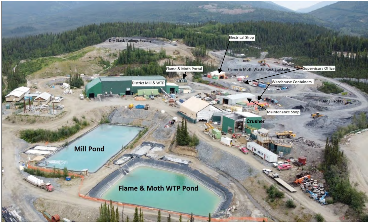
Photo 2-1: Flame & Moth Mine surface infrastructure (July 2023)
