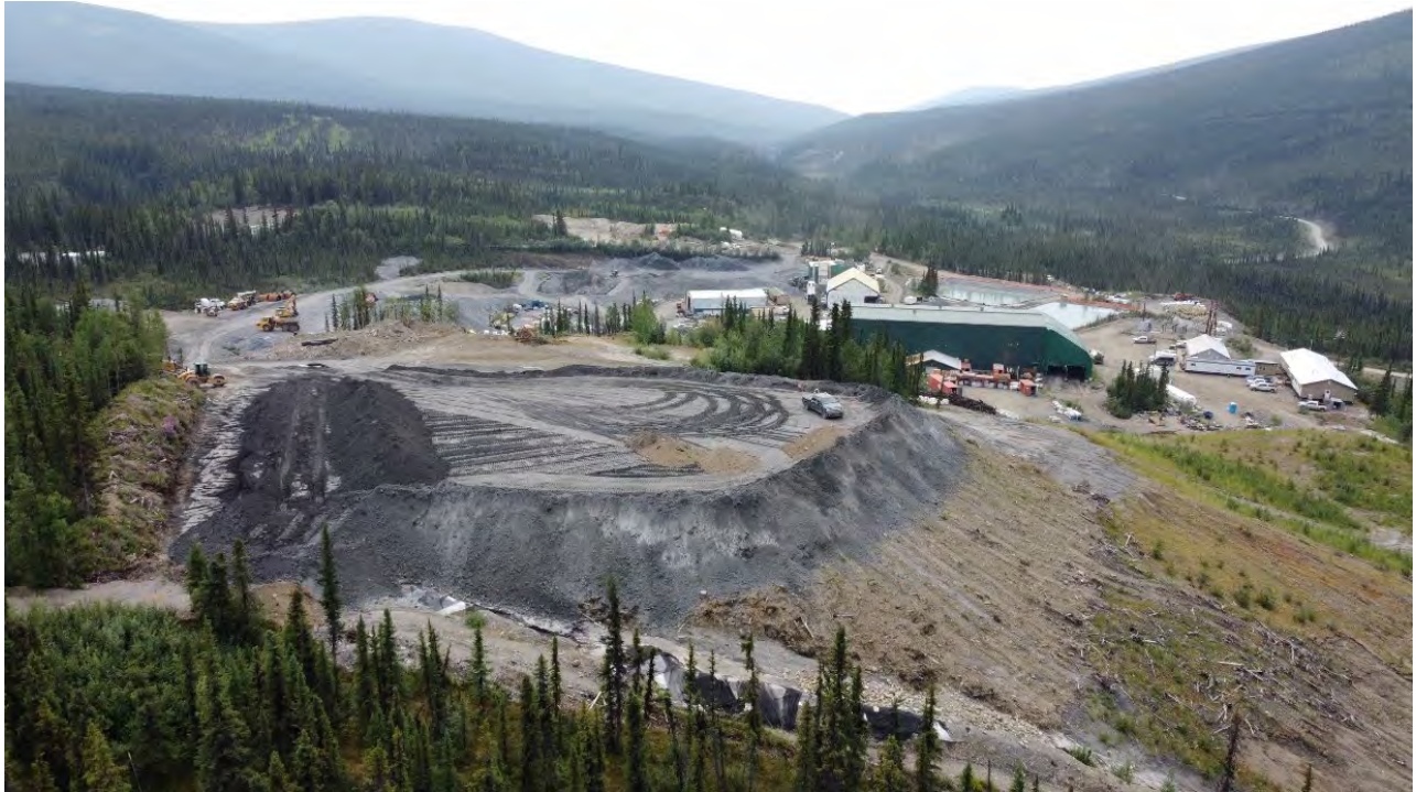
Photo 15: Photo 13: DSTF Phase 1 – aerial view facing southwest. Over steepened areas of recent placement visible in foreground. (I. MacIntyre, July 22, 2023)
