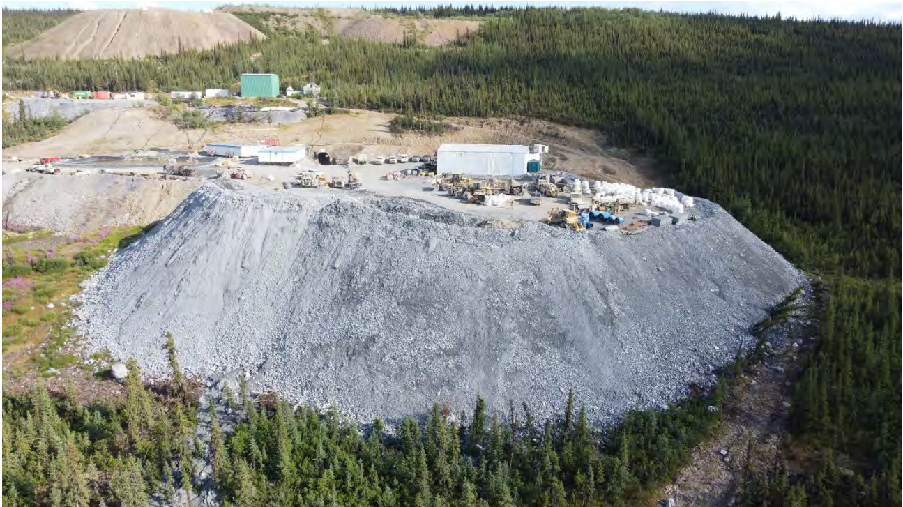
Photo 22: Birmingham NAML waste dump, aerial view facing south. Sloughed material visible in lower left. (I. MacIntyre, July 20, 2023)
