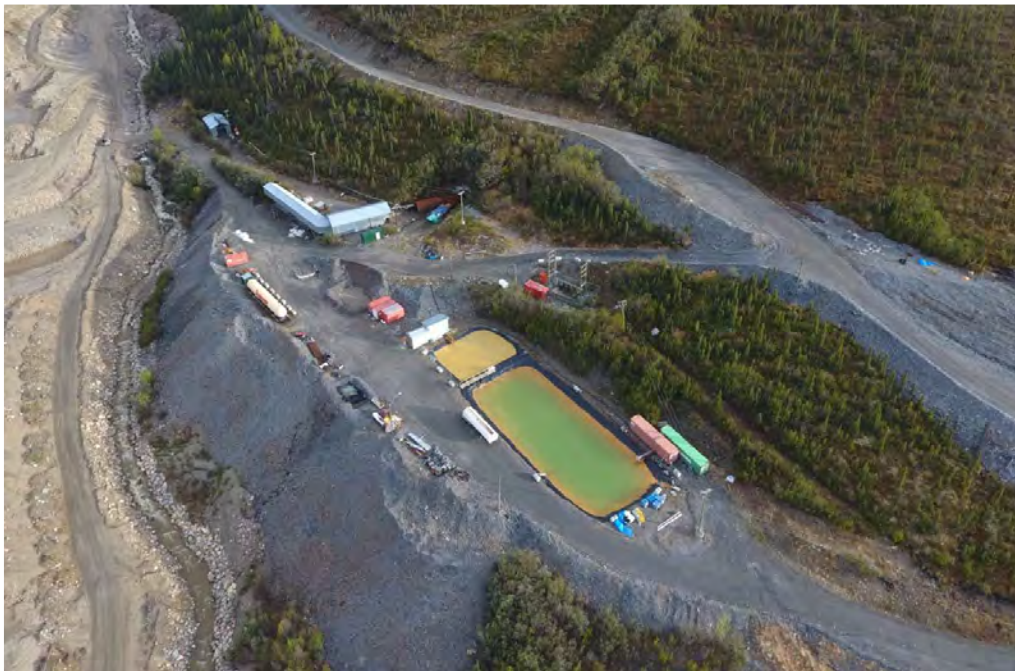
Photo 2-1: Bellekeno 625 WTP Area Overview
