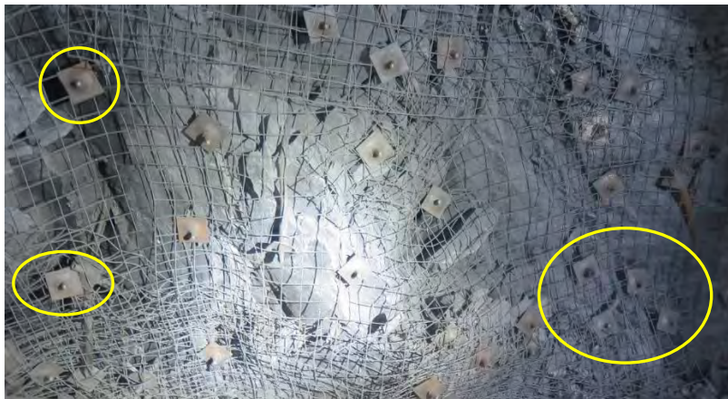
Figure 11. Photograph of the back showing Swellex friction bolts not in contact with the rock surface.
