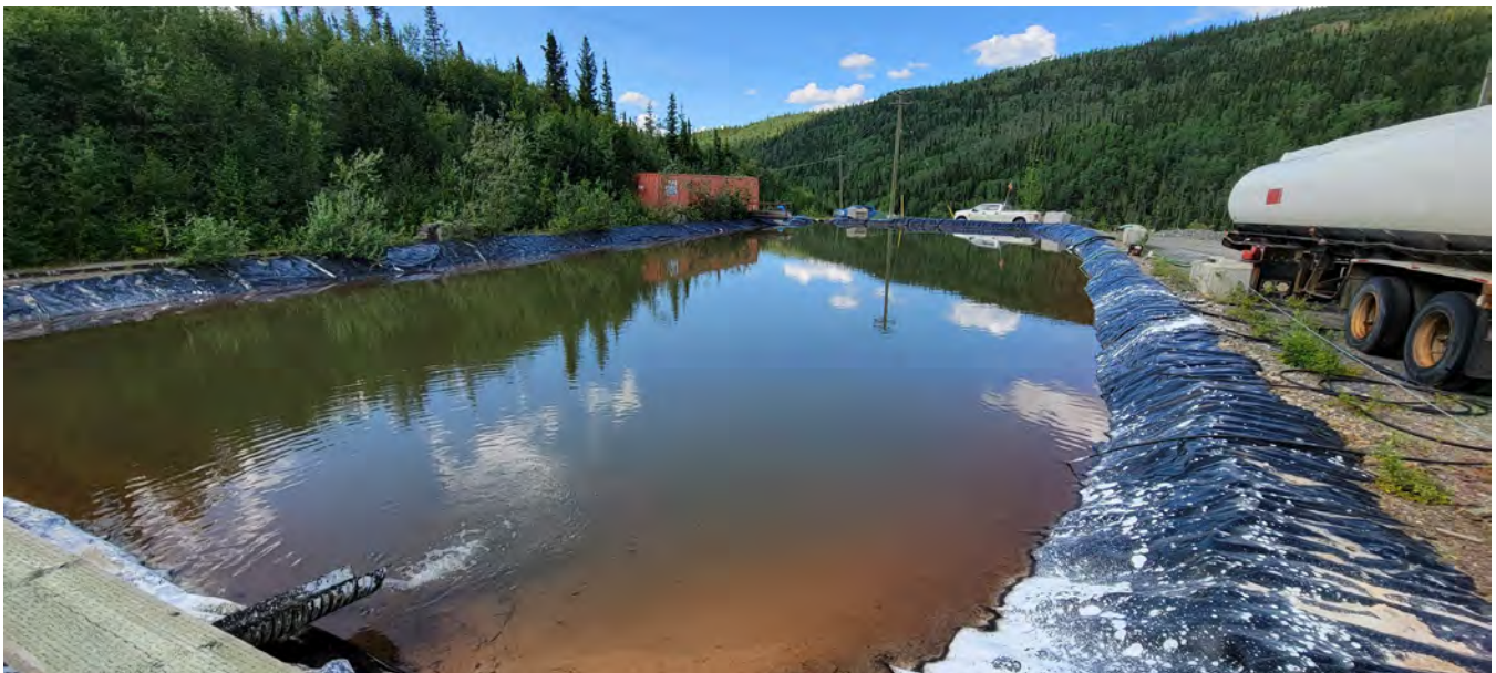
Photo 4: Bellekeno 625 Water Treatment Ponds, facing northwest (I. MacIntyre, July 20, 2023)
