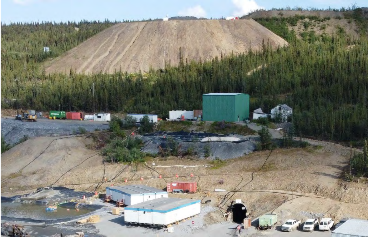
Photo 23: Bermingham Mine Sludge Waste Containment Facility – buried organics and trees visible in foreground. (I. MacIntyre, July 20, 2023)
