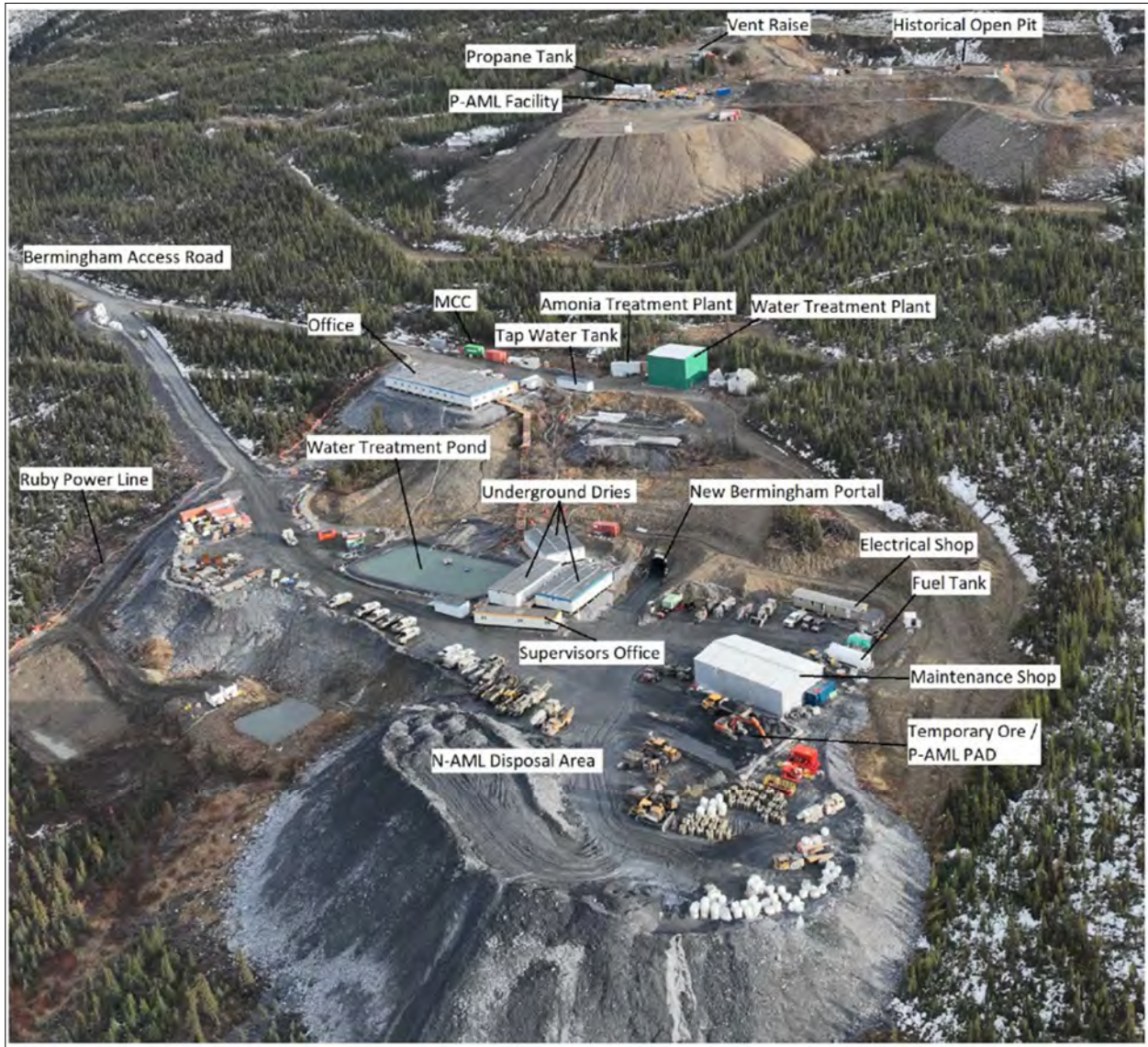
Photo 2-2: New Birmingham Mine surface infrastructure Year-end 2023
