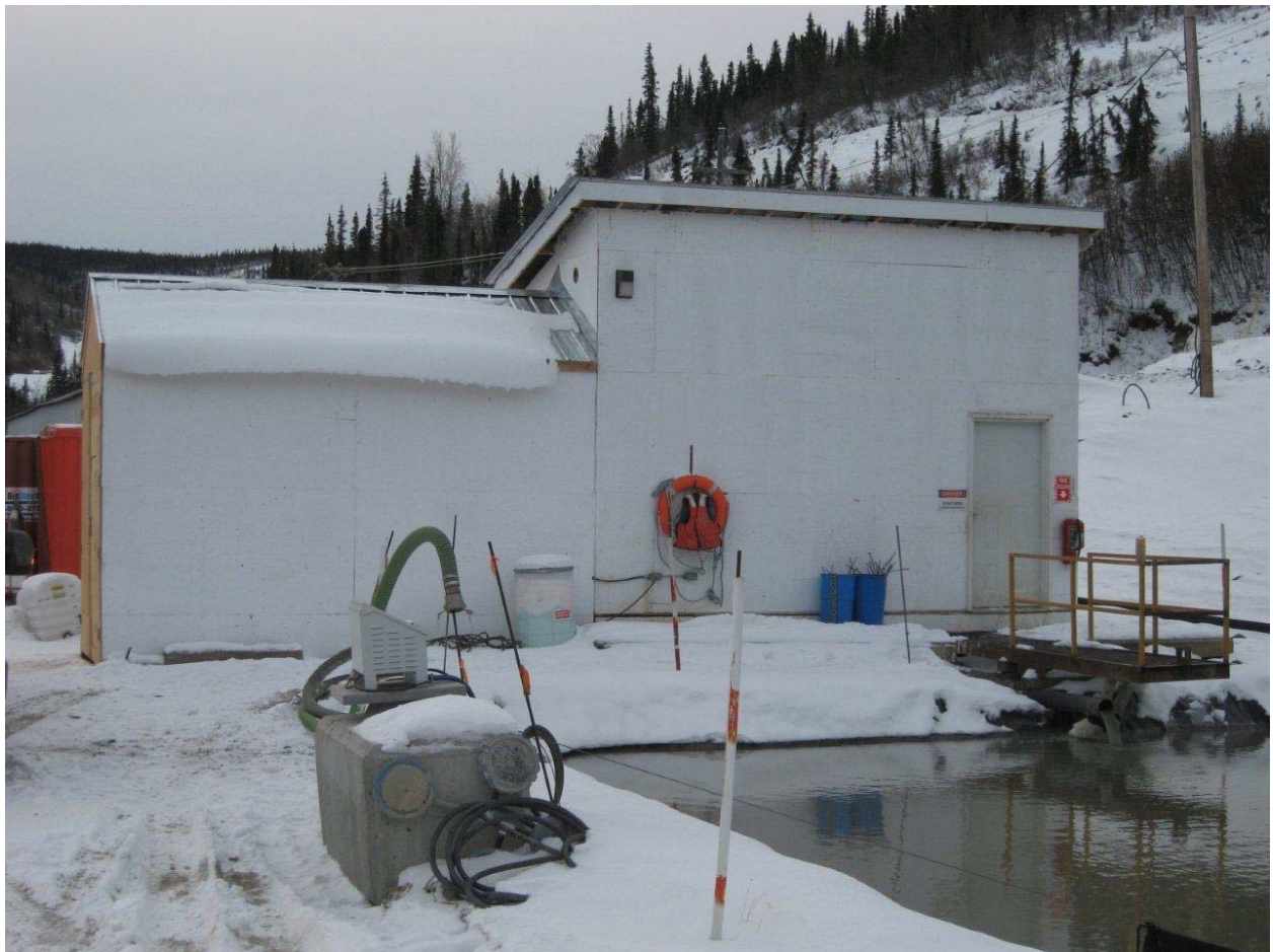
FIGURE 3 – BELLEKENO WATER TREATMENT SHED
