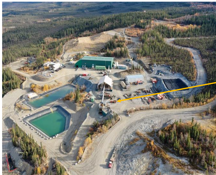
Alexco's Keno Hill District Mill with F&M portal, waste rock storage pad and the Keno City bypass road access
