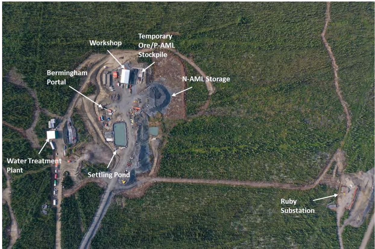
Figure 7-33 Existing Birmingham Surface Infrastructure (September 2021)
