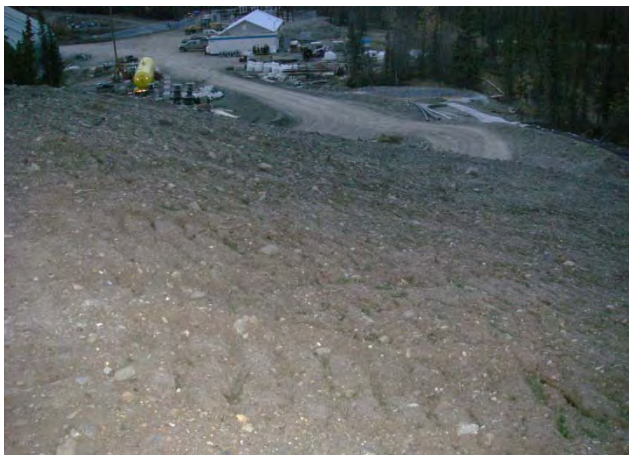
Photo 11: Grass sprouts DSTF looking south from crest
