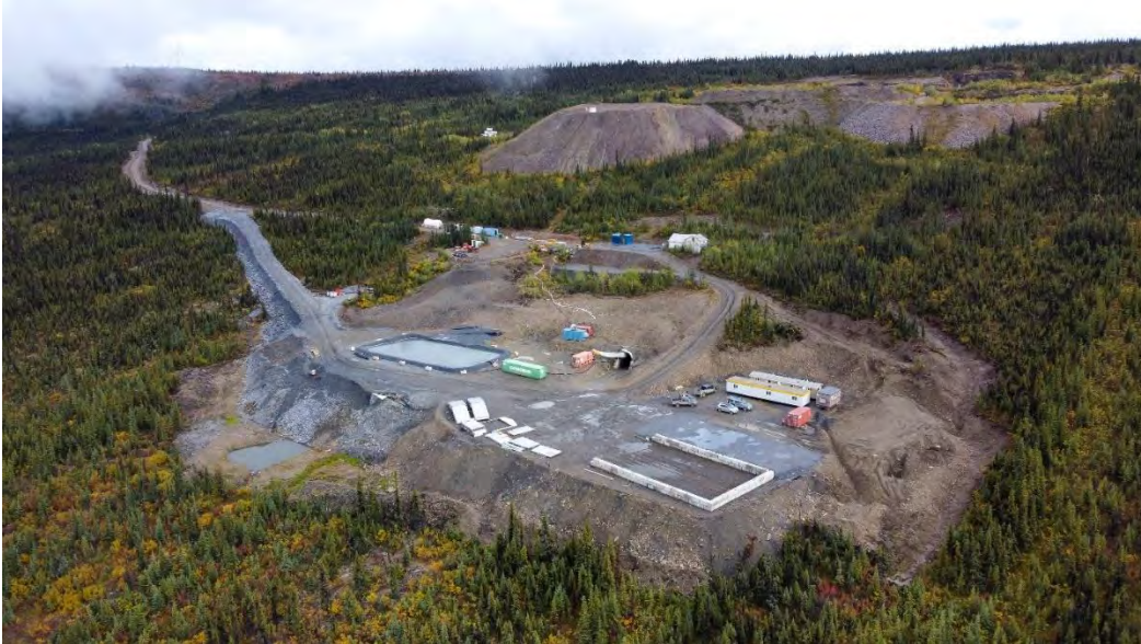
Figure 7-10 Bermingham Portal Area – August 2020
