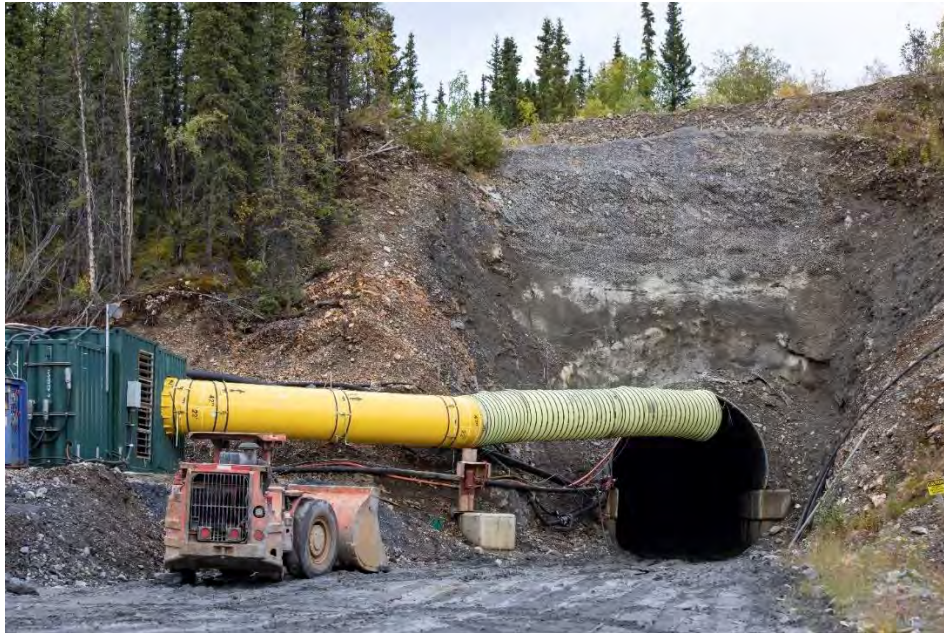
Figure 7-8 Flame & Moth Adit During Developments
