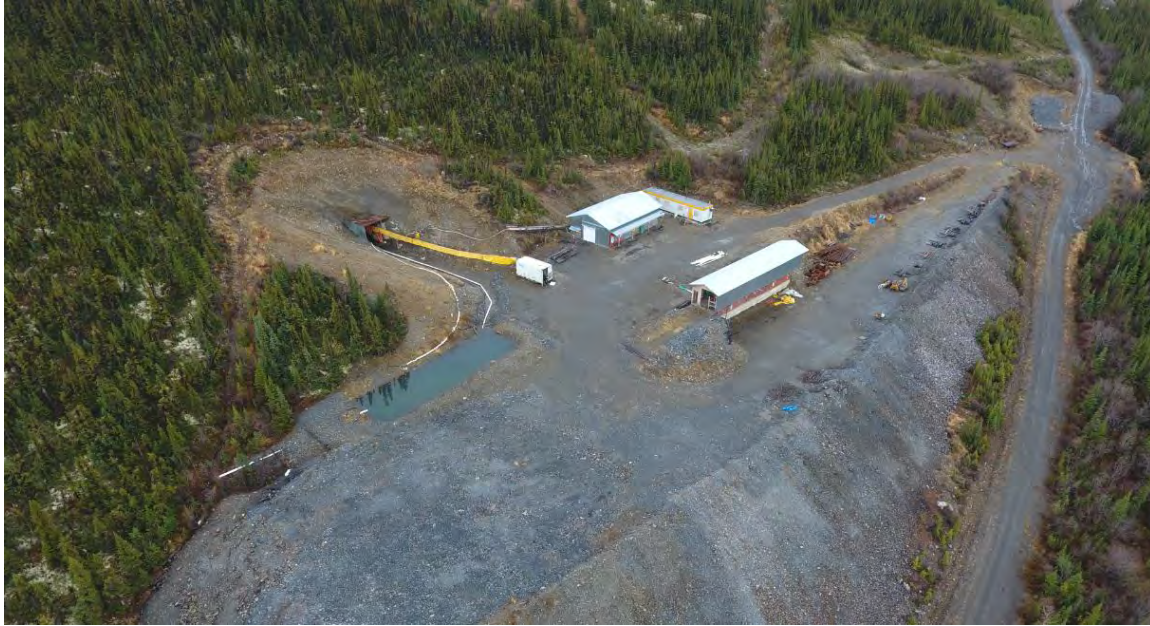
Figure 7-18 Lucky Queen Portal
