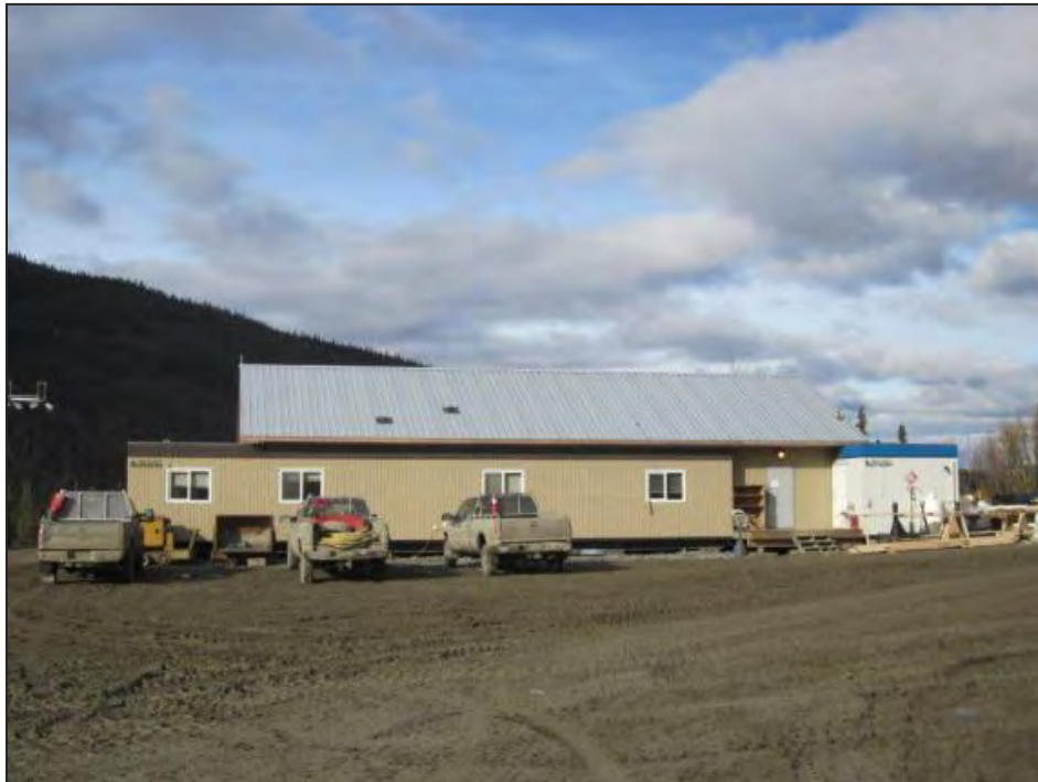
Figure 7-36 Mill Office and Dry
