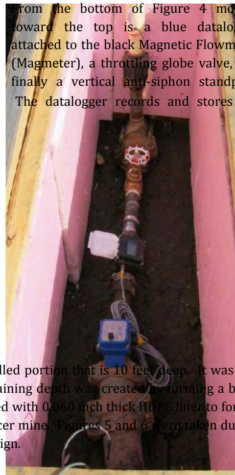
Figure 4 - Bioreactor Inlet
