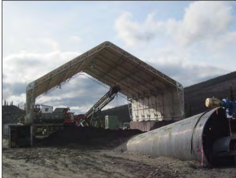
Figure 7-39 Fine Ore Stockpile
