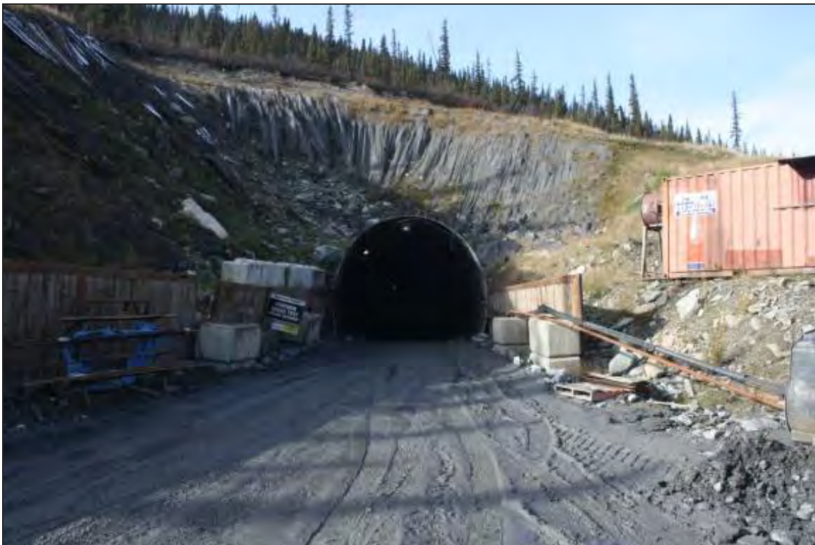
Figure 7-3 Bellekeno East Portal
