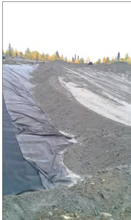
Figure 5-7 Compacted DSTF Lift
