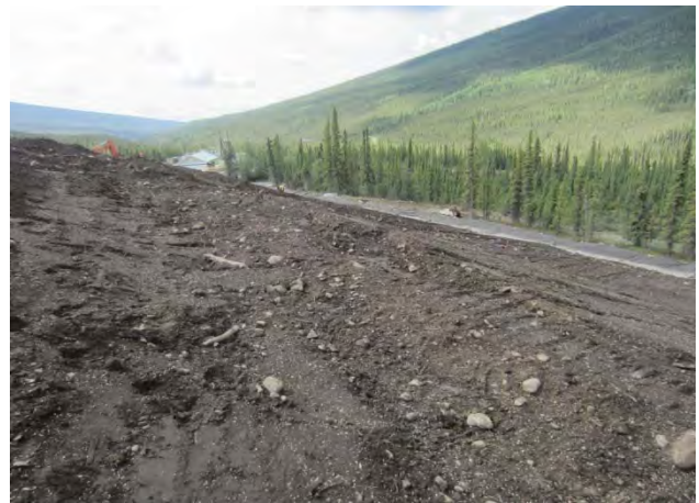
Photo 10: Covered DSTF crest looking south
