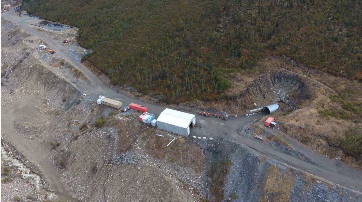
Figure 7-2 Bellekeno East Portal and Site Facilities
