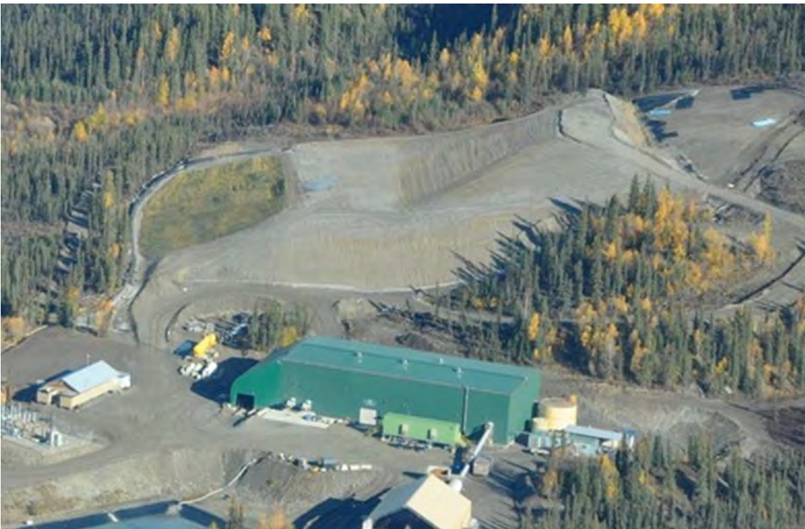
Figure 7-22 DSTF Progressive Reclamation, August 2013
