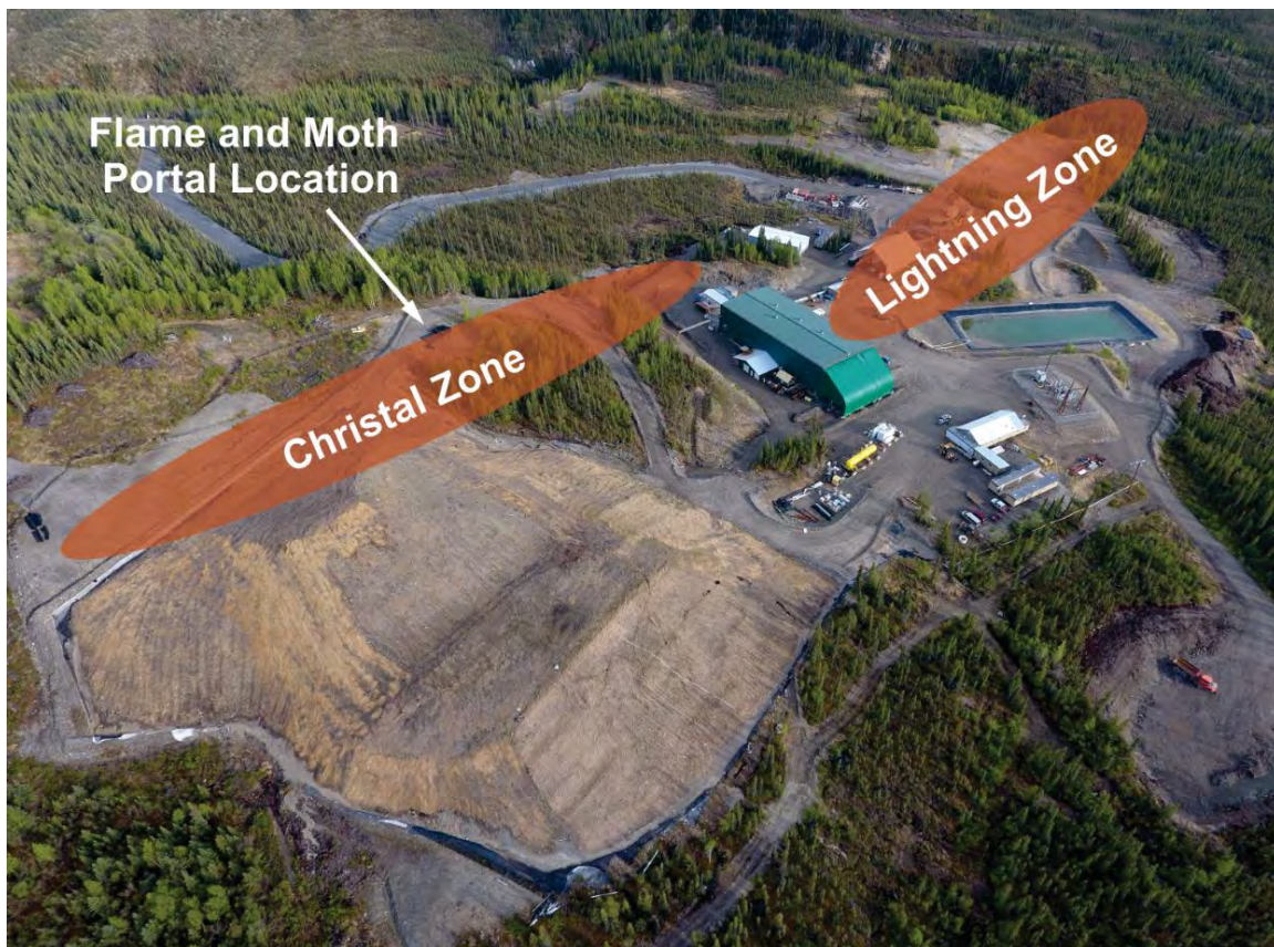
Figure 7-32 Flame and Moth Surface Facilities
