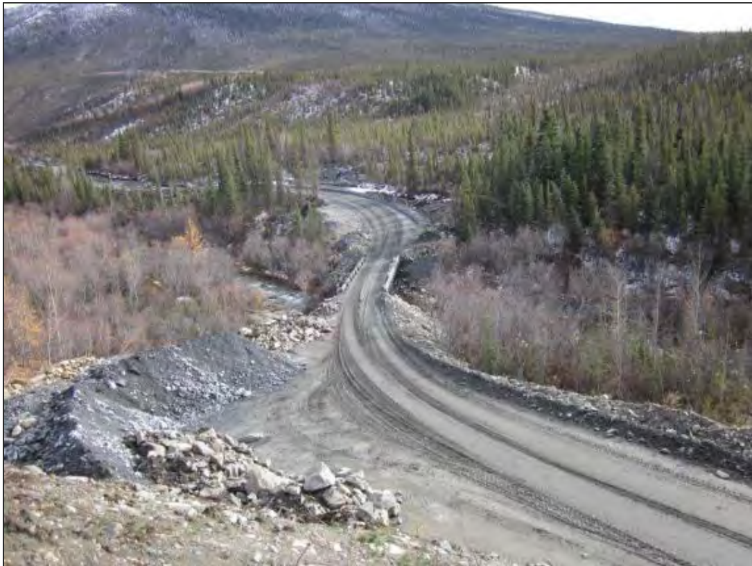
Figure 7-44 Lightning Creek Bridge and Typical Bellekeno Haul Road Section
