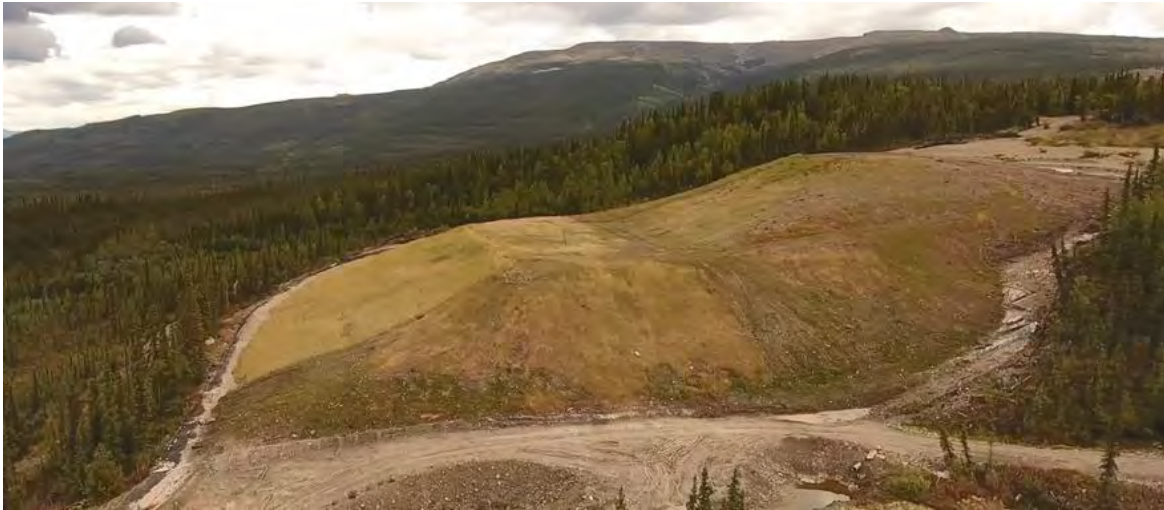
Figure 7-23 DSTF Progressive Reclamation, September 2016
