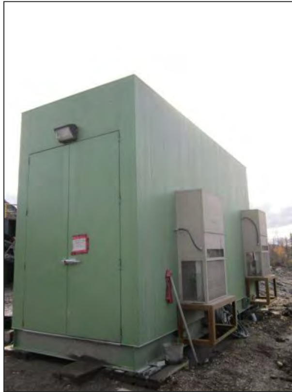
Figure 7-40 Crusher MCC
