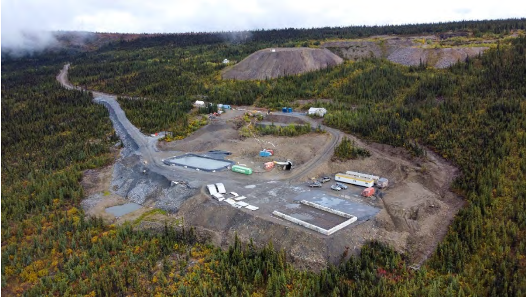
Figure 7-10 Birmingham Portal Area – August 2020
