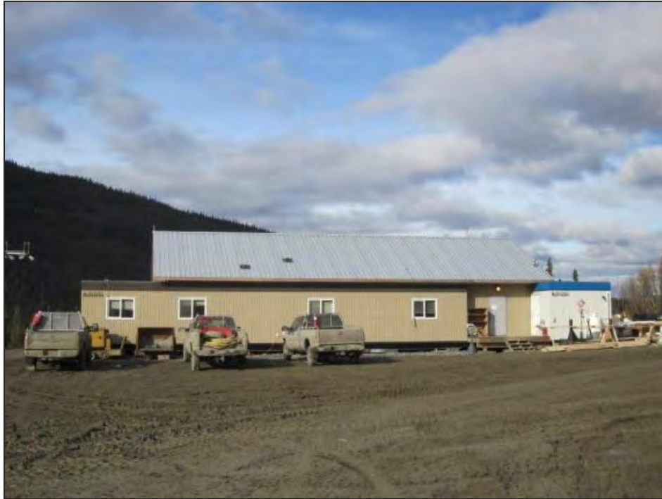
Figure 7-36 Mill Office and Dry
