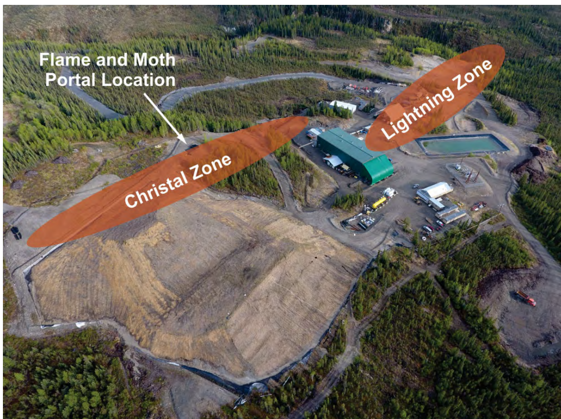
Figure 7-32 Flame and Moth Surface Facilities
