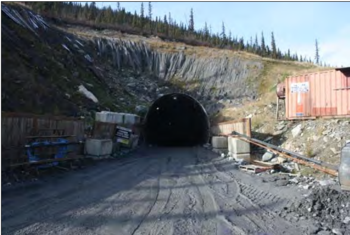
Figure 7-3 Bellekeno East Portal
