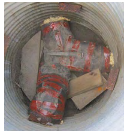
Figure 2 - Inlet Valve
