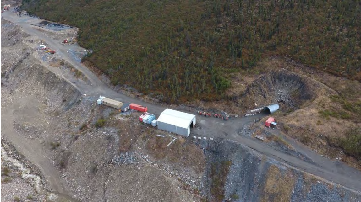
Figure 7-2 Bellekeno East Portal and Site Facilities
