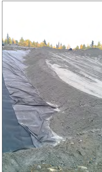
Figure 5-7 Compacted DSTF Lift
