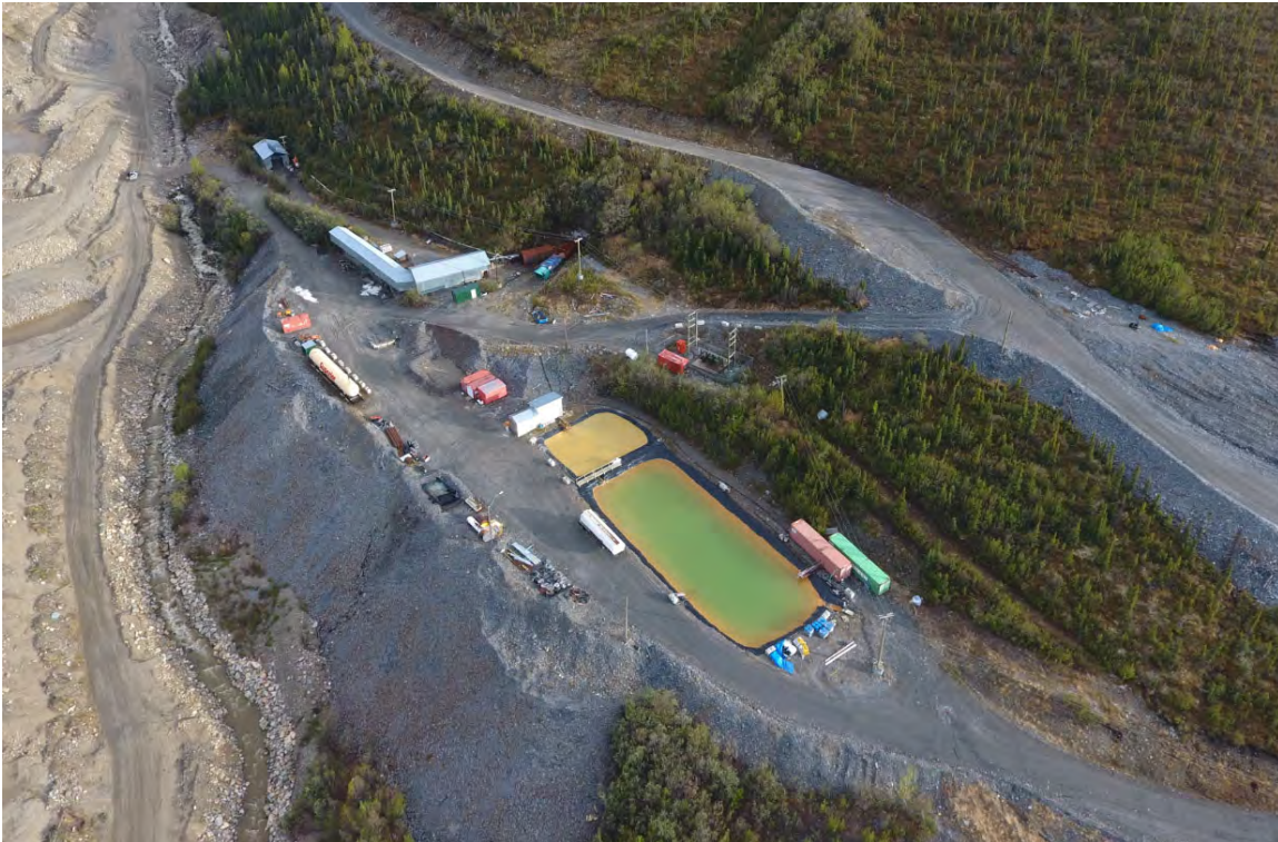
Figure 7-27 Bellekeno 625 WTP Area Overview
