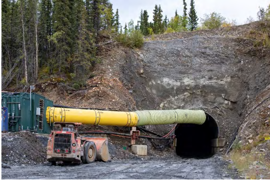
Figure 7-8 Flame & Moth Adit During Developments
