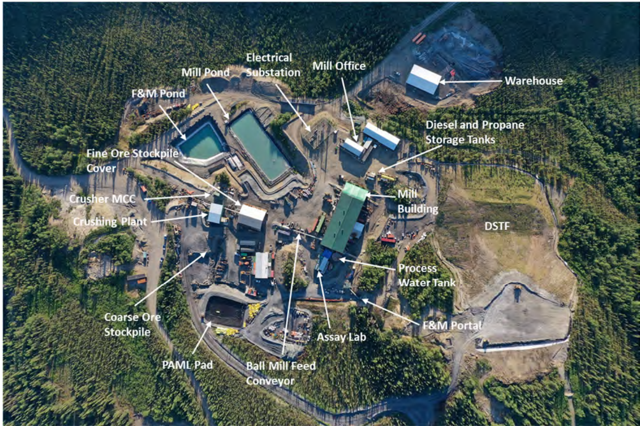
Figure 7-34 Aerial View of Mill Site Infrastructure and Layout
