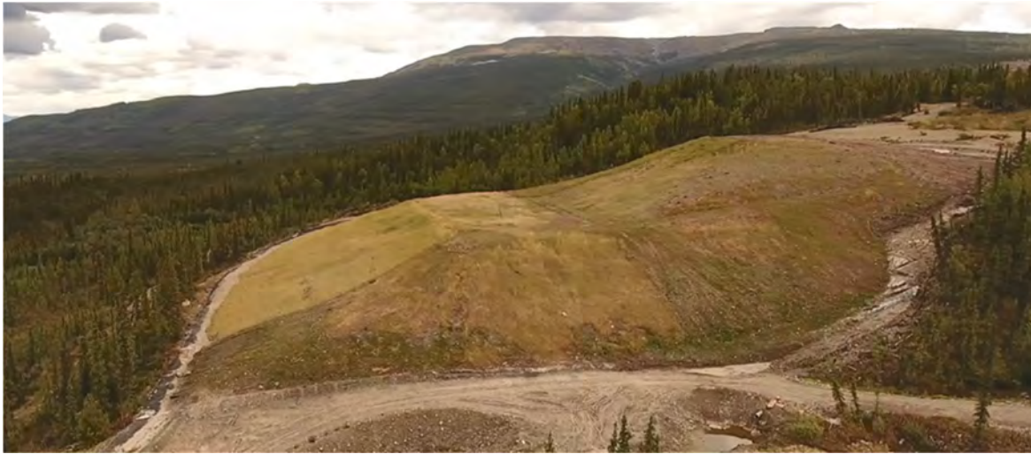
Figure 7-23 DSTF Progressive Reclamation, September 2016
