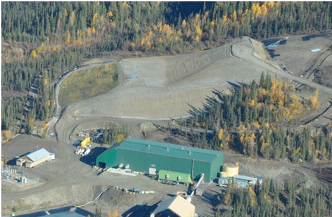
Figure 7-22 DSTF Progressive Reclamation, August 2013
