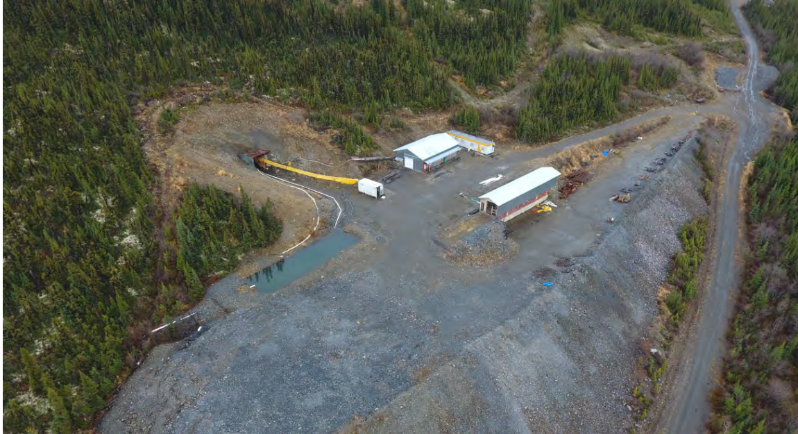
Figure 7-18 Lucky Queen Portal
