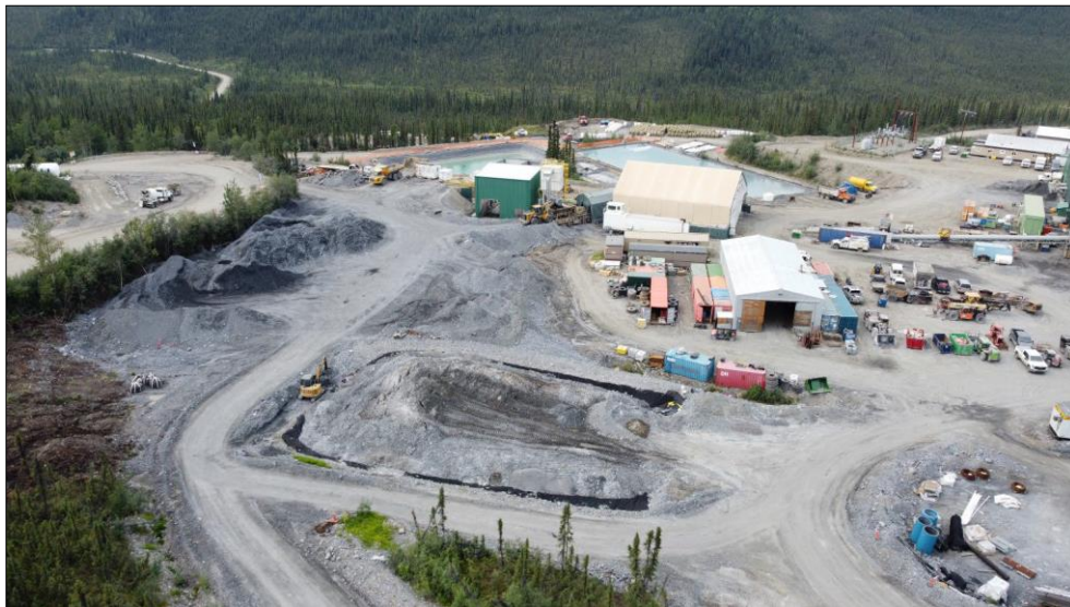
Photo 5-4: Flame & Moth P-AML Pad and Mill Ore Pad
