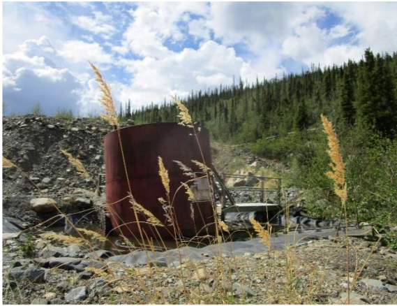
Photo 6-5: Bellekeno Fuel Tank Farm – 2021
