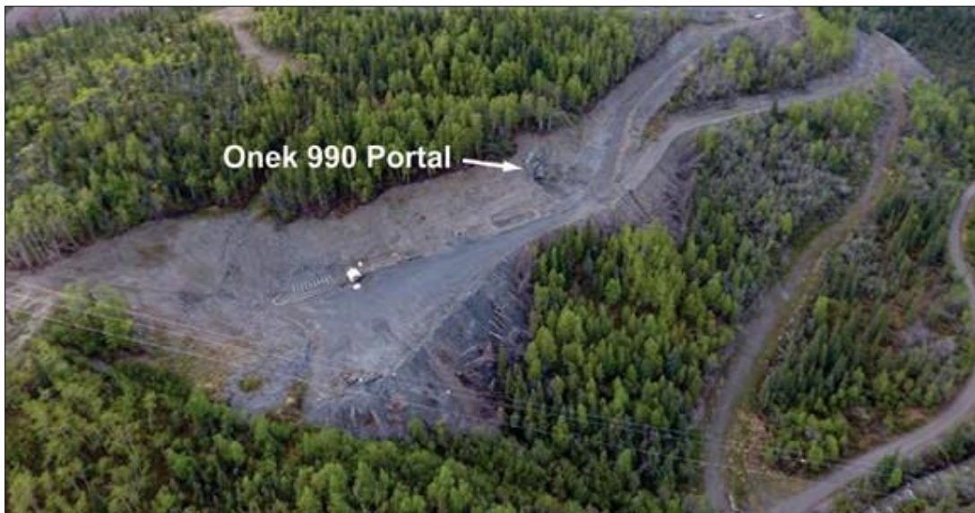
Photo 5-11: Onek Mine Surface Overview
