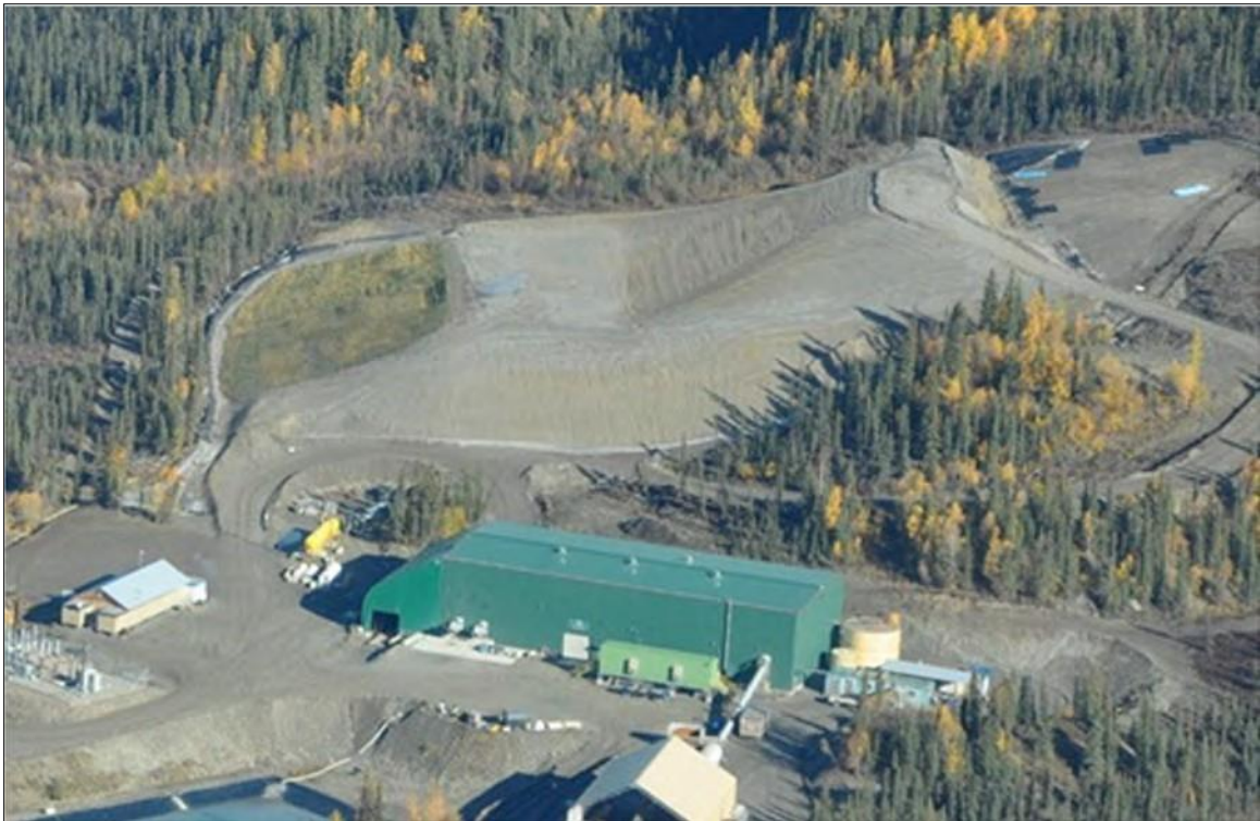
Photo 6-2: DSTF Progressive Reclamation, August 2013
