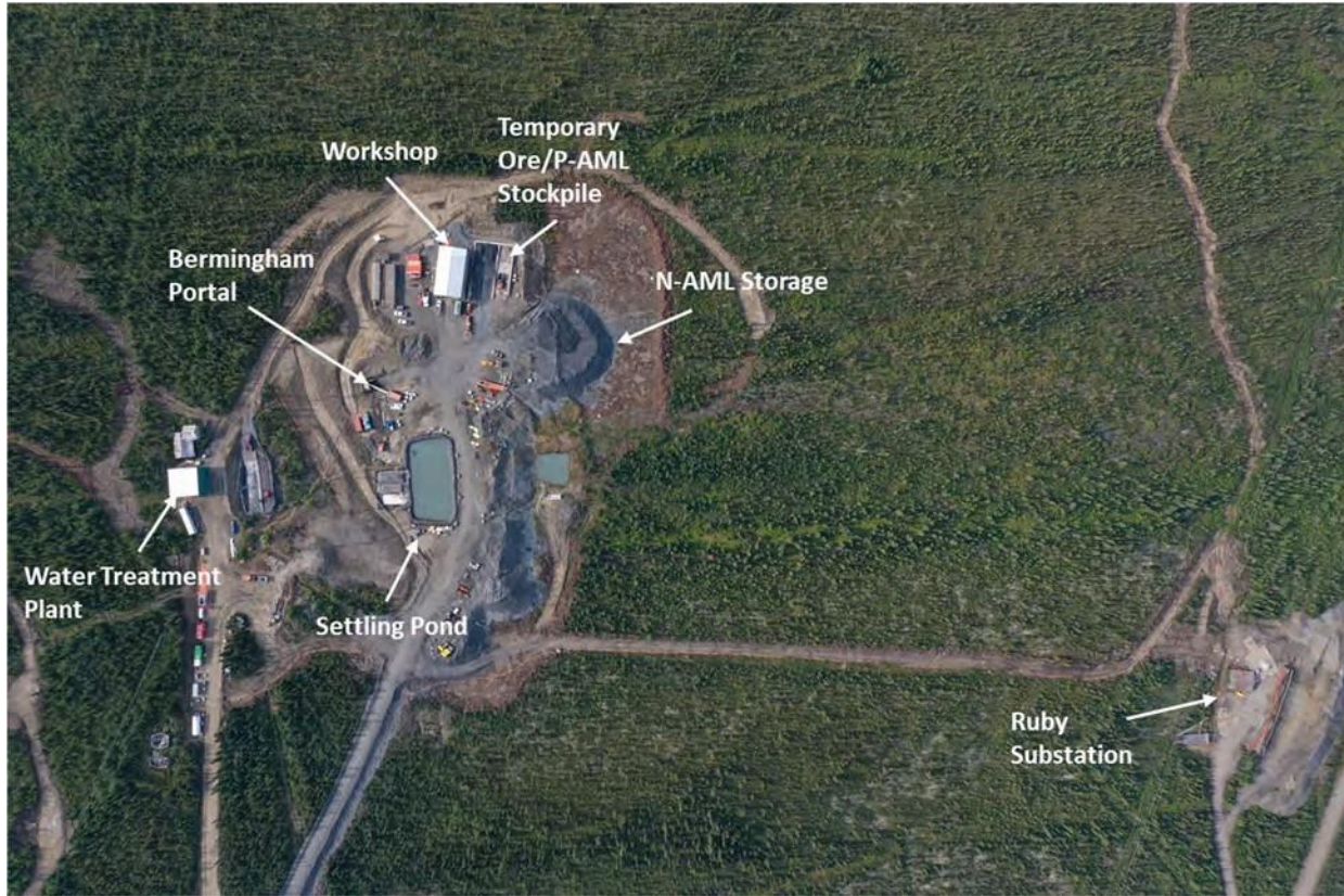
Photo 5-6: New Birmingham Surface Infrastructure (September 2021)
