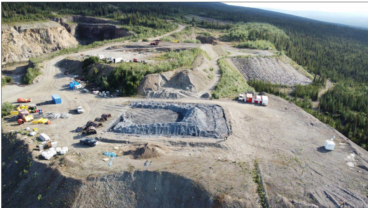
Photo 5-7: New Birmingham P-AML Waste Rock Storage Facility #1
