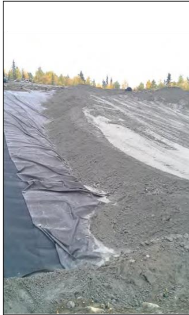
Photo 5-20: Compacted DSTF Lift
