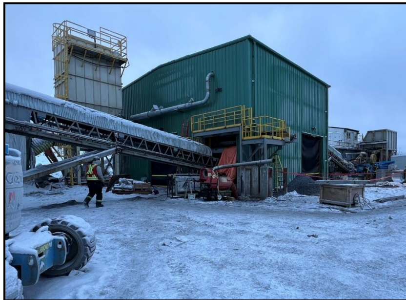
Photo 8-5: Crushing Plant – November 2023
