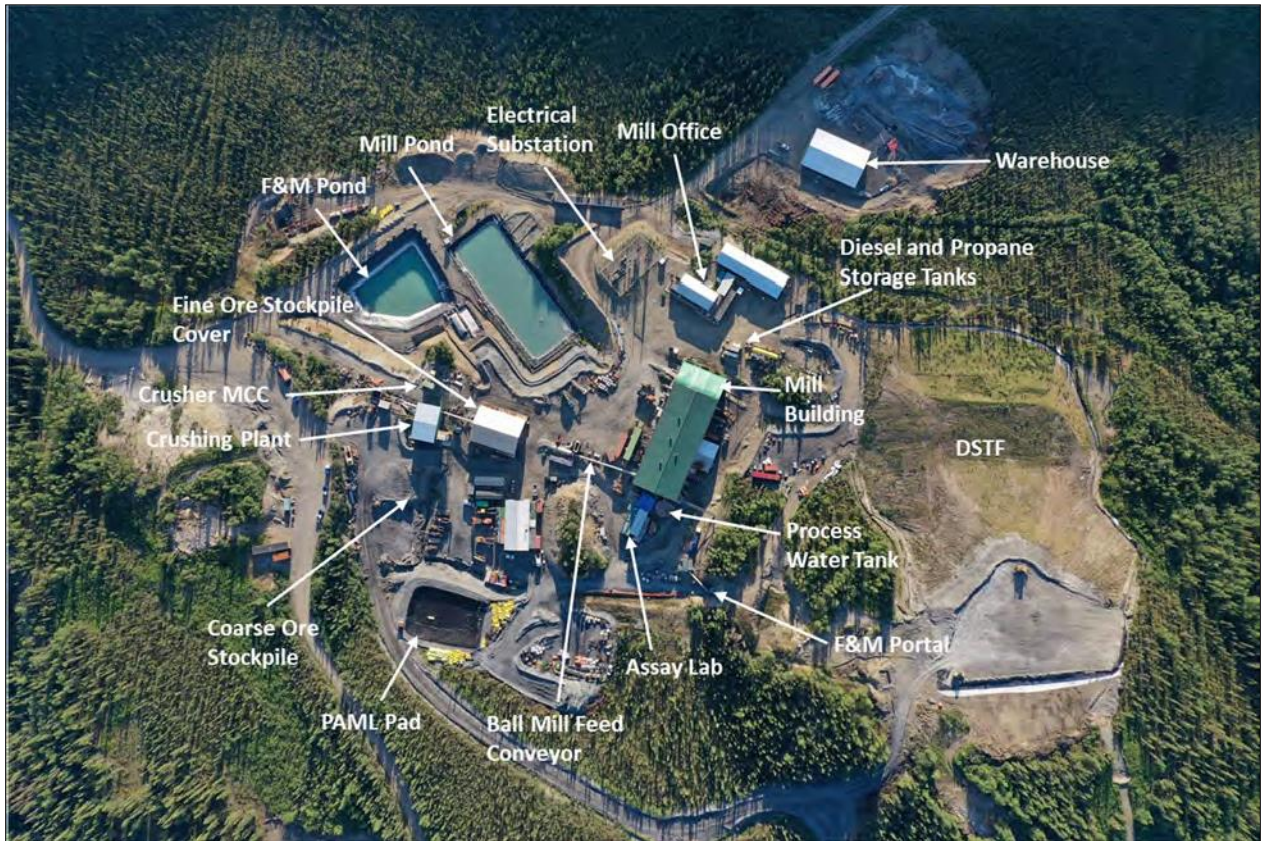
Figure 5-27: Mill Infrastructure Overview
