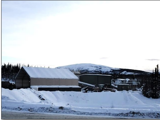
Photo 5-15: Fine Ore Storage, Secondary and Primary Crusher Building
