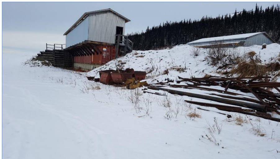
Photo 5-9: Lucky Queen Portal Pad (October 2023)
