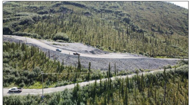
Photo 5-2: Bellekeno N-AML waste rock used for construction of Bellekeno Haul Road
