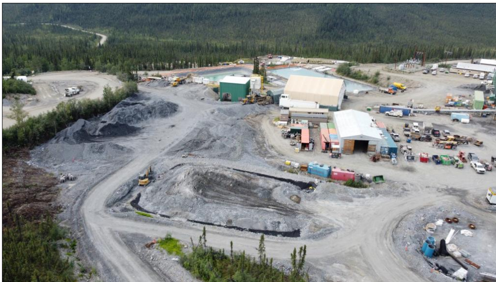
Photo 5-14: Ore Stockpile and Flame & Moth P-AML Pad
