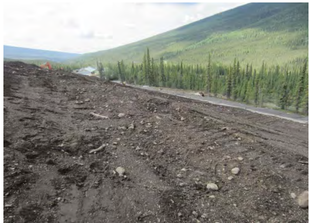
Photo 10: Covered DSTF crest looking south
