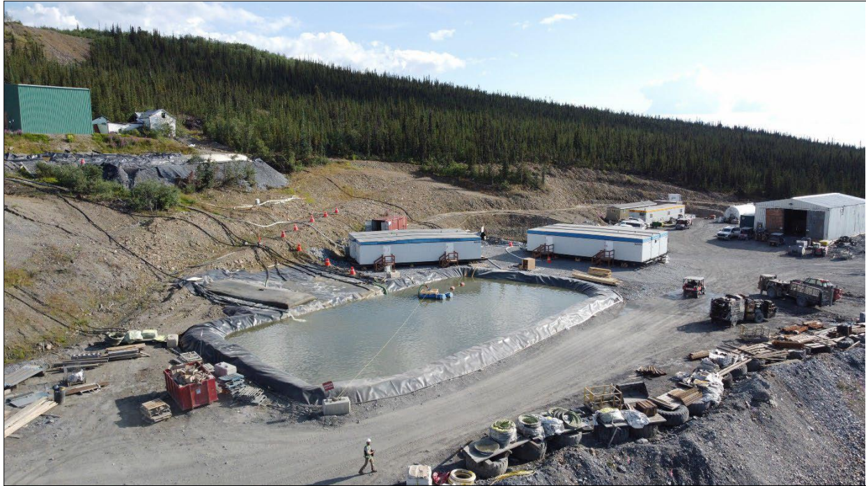
Photo 5-13: New Bermingham Settling Pond
