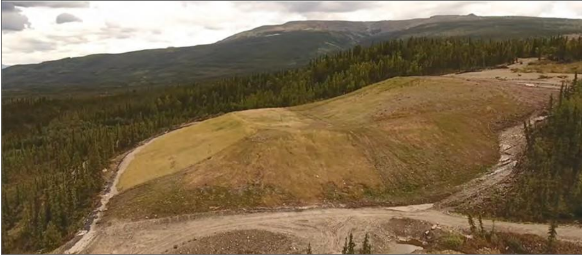
Photo 6-3: DSTF Progressive Reclamation, September 2016
