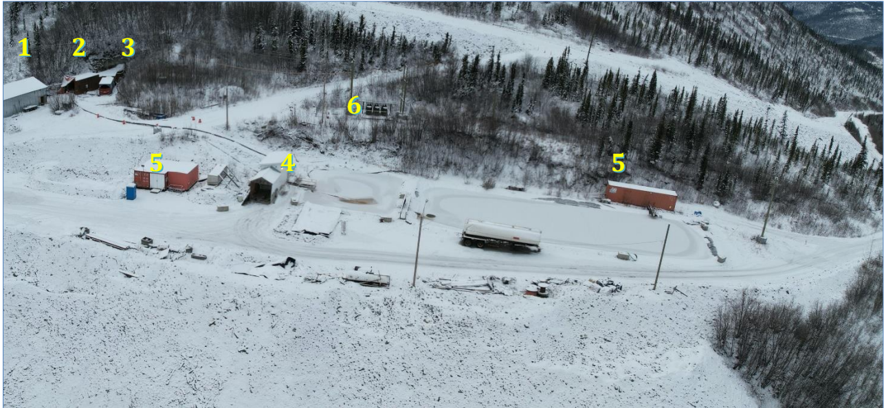
Photo 8-2: Bellekeno 625 Surface Facilities – October 2023
