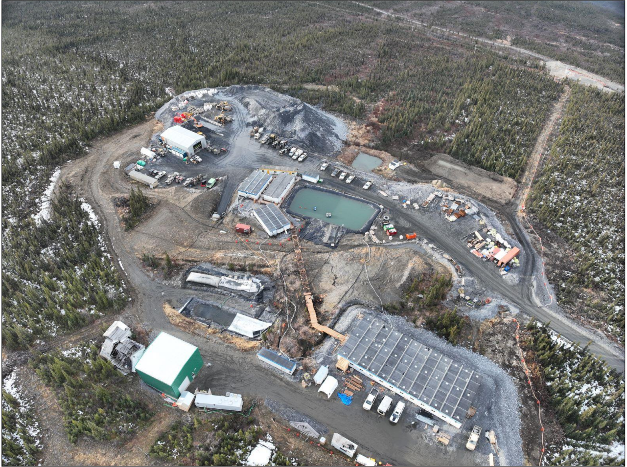
Photo 5-5: New Bermingham Surface Infrastructure (October 2023)
