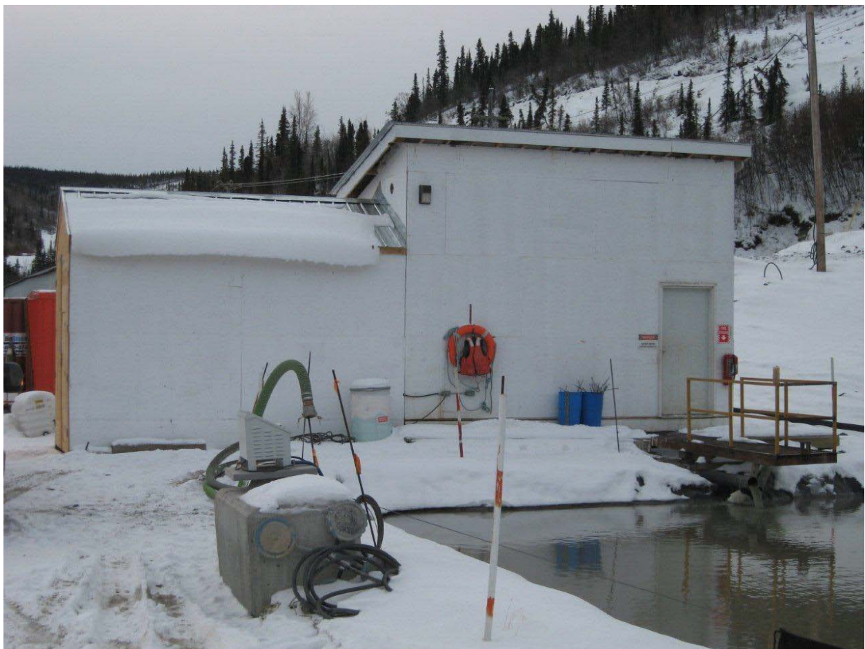
FIGURE 3 - BELLEKENO WATER TREATMENT SHED
