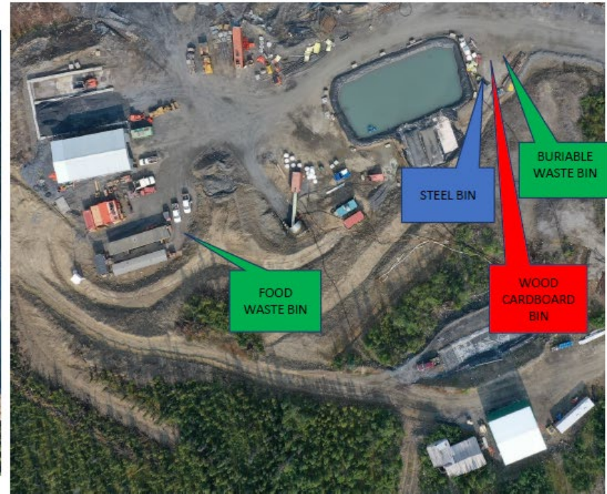
Figure 4-2: New Bermingham Mine waste bins
