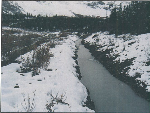
Figure 28 U/S Segment of Interceptor Ditch
