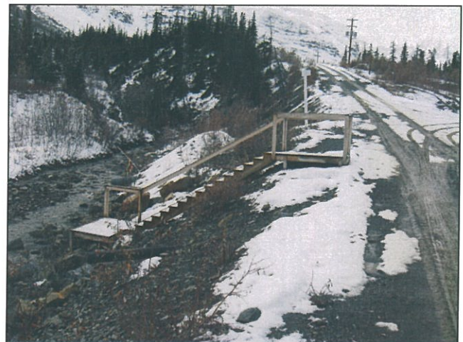
Figure 07 Discharge Line at Cache Cr. Diversion
