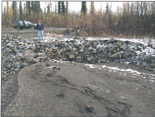
Figure 46 U/S Transition at Location H
