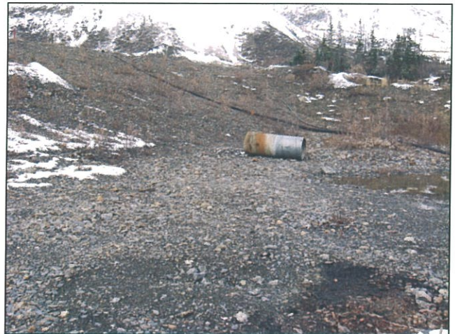
Figure 15 Saplings on D/S Slope of South Dam
