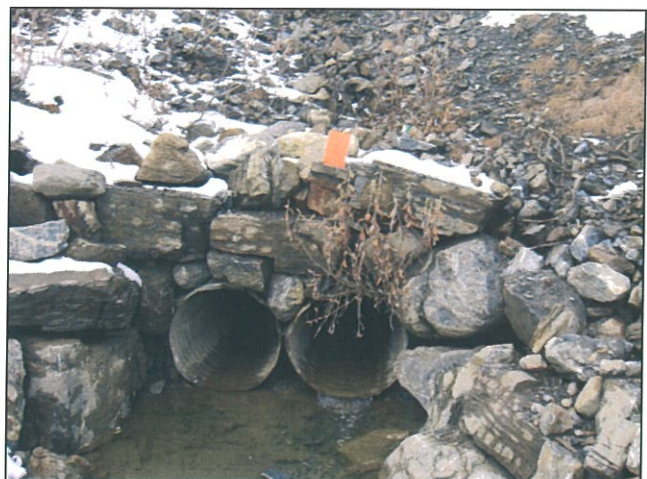
Figure 27 Culverts at Upstream End of Channel
