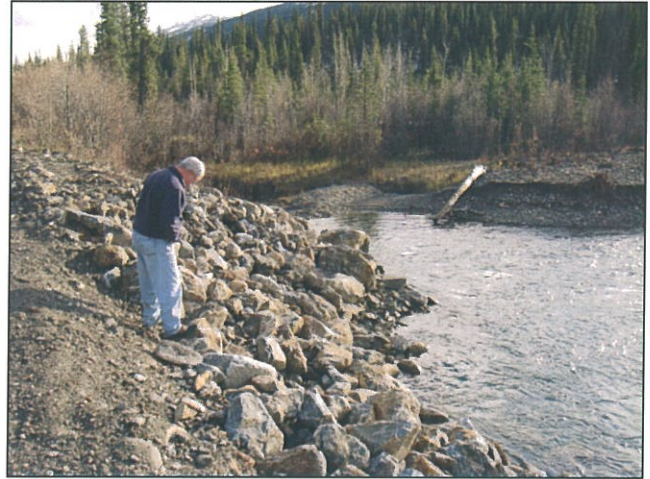
Figure 35 View U/S at Location C
