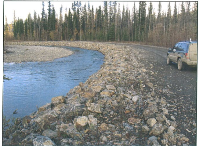
Figure 41 View D/S at Location G
