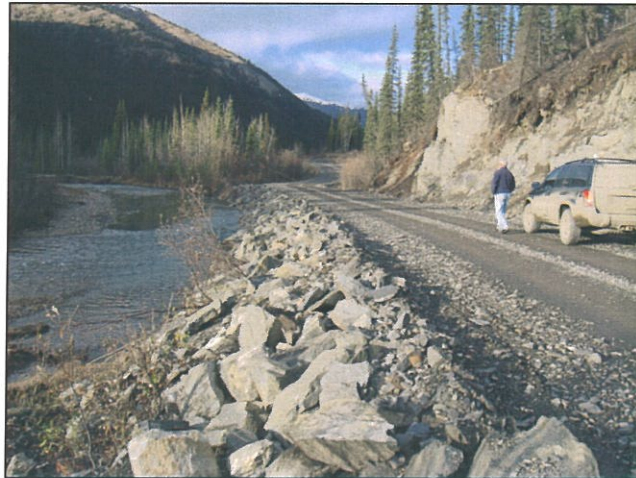
Figure 37 View D/S at Location E
