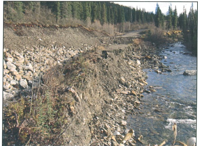
Figure 33 Erosion of Old Roadbed
