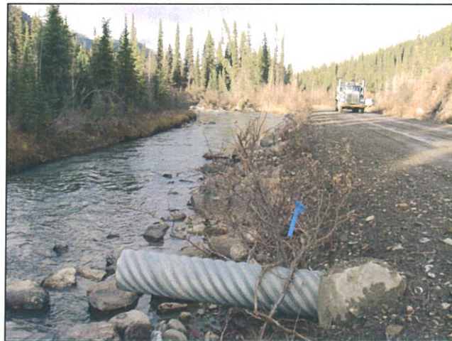
Figure 36 Culvert at Location D
