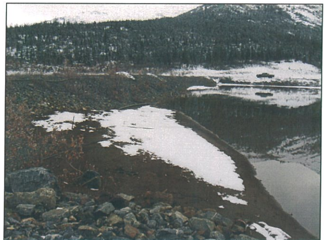
Figure 05 Exposed Tailings Behind South Dam
