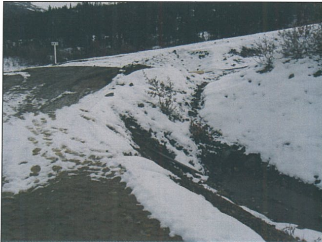
Figure 24 Culvert at End of Diversion Channel
