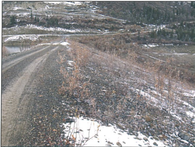
Figure 14 Saplings on North Dam Slopes
