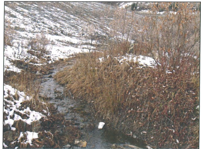
Figure 17 Drainage Channel at Toe of North Dam
