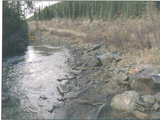
Figure 31 Riprap at Location A
