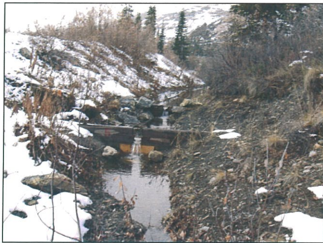
Figure 10 Weirs D/S of South Dam
