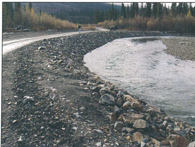
Figure 42 View U/S at Location H
