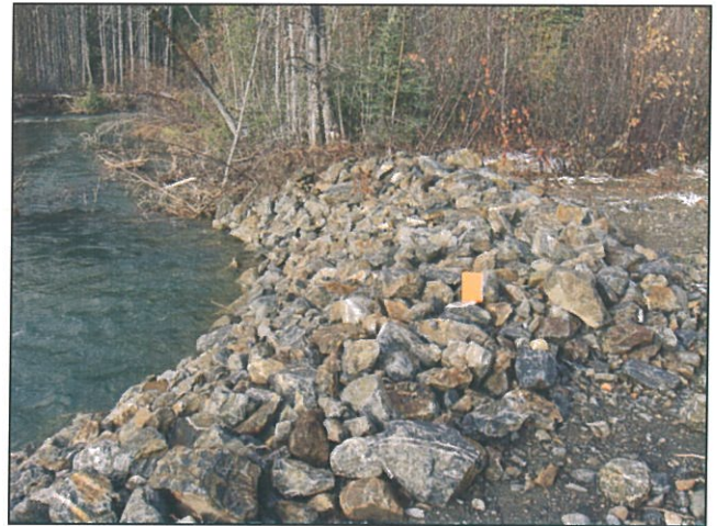
Figure 47 D/S Transition at Location H
