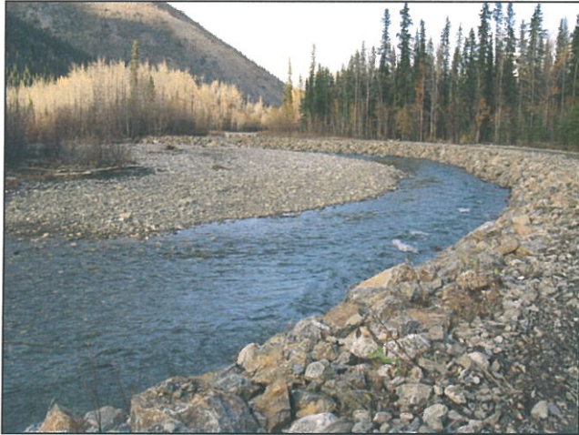
Figure 40 View D/S at Location G
