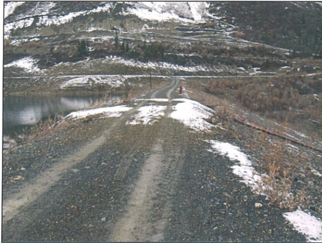
Figure 12 North Dam Crest
