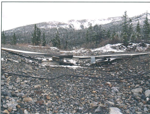
Figure 18 Spillway (view D/S)
