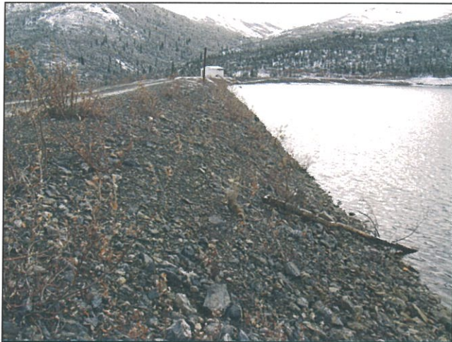
Figure 04 Upstream Side of North Dam
