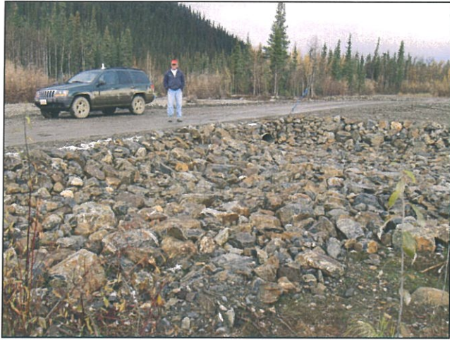
Figure 44 Culvert at Location H
