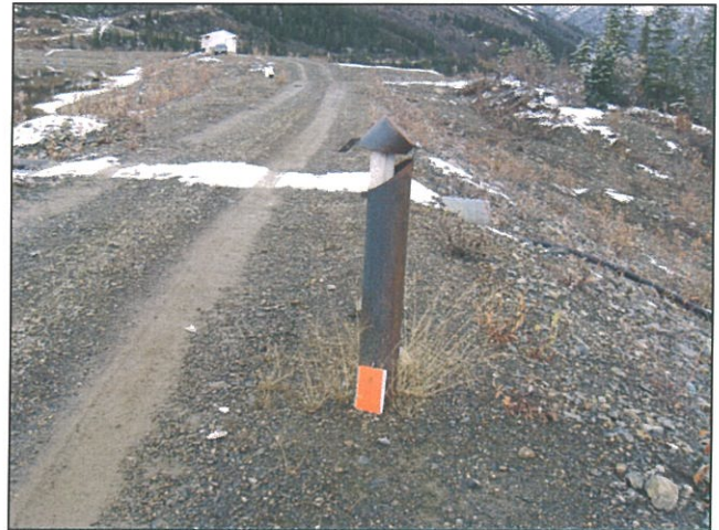
Figure 13 Piezometer P12B&C on South Dam Crest
