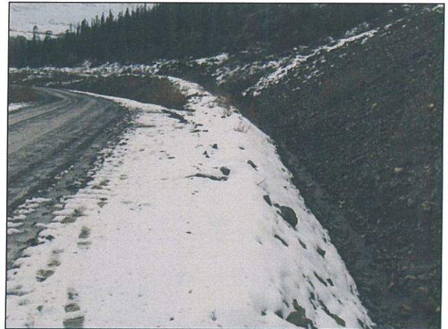
Figure 29 D/S Segment of Interceptor Ditch
