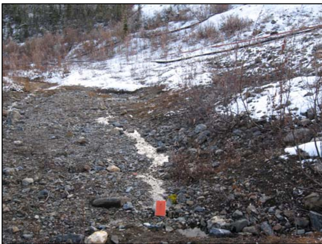
Fig 03 Seepage at Toe of North Dam (2007)
