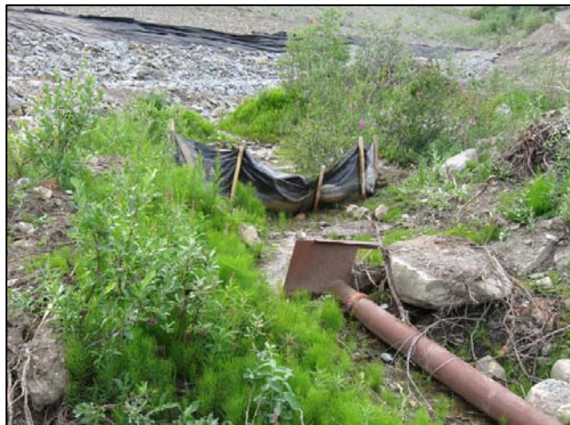
Fig 09 Seepage Channel and Weir Pipe
