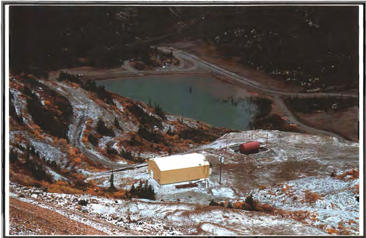
Photo 4: Mine dry and Aboveground Storage Tank (AST) at 1510 portal. Tailings pond and Cache Creek diversion in background.
