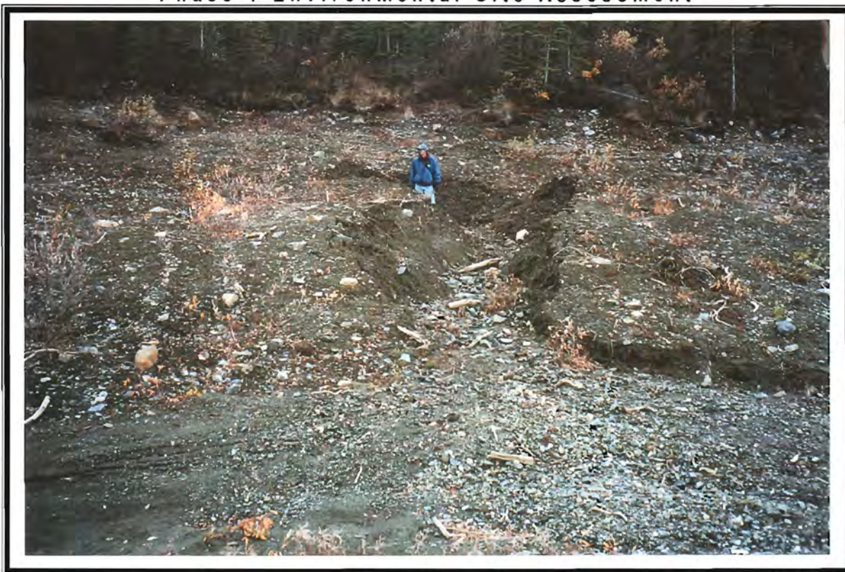
Photo 32: Failure and erosion of northwest diversion ditch.
