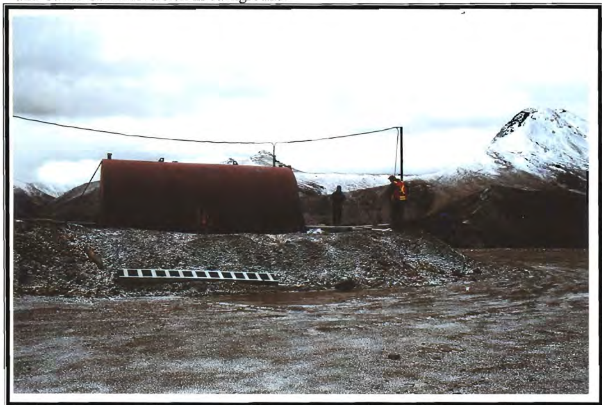
Photo 5: AST at 1510 portal used for fuelling underground equipment.
