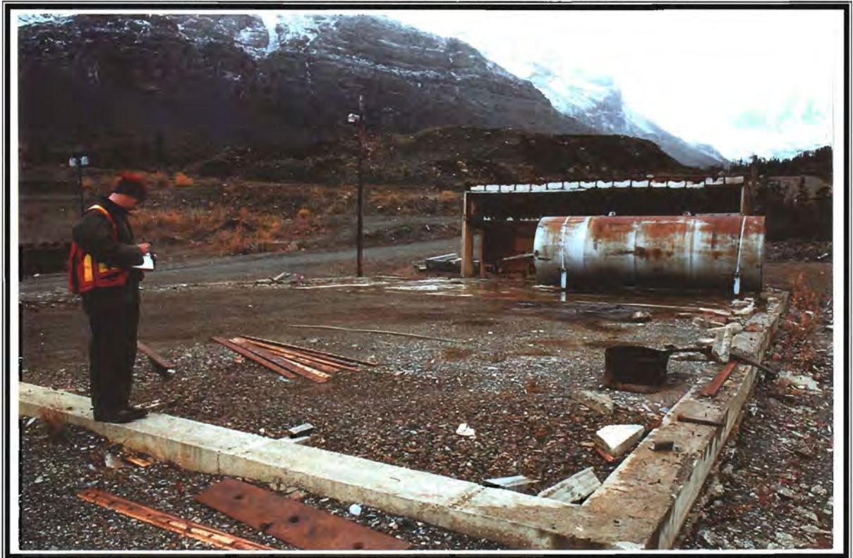
Photo 25: Foundation of road maintenance contractor's Quonset hut. Note heavy hydrocarbon staining of soil in front of gasoline tank. Ore stockpile in background.
