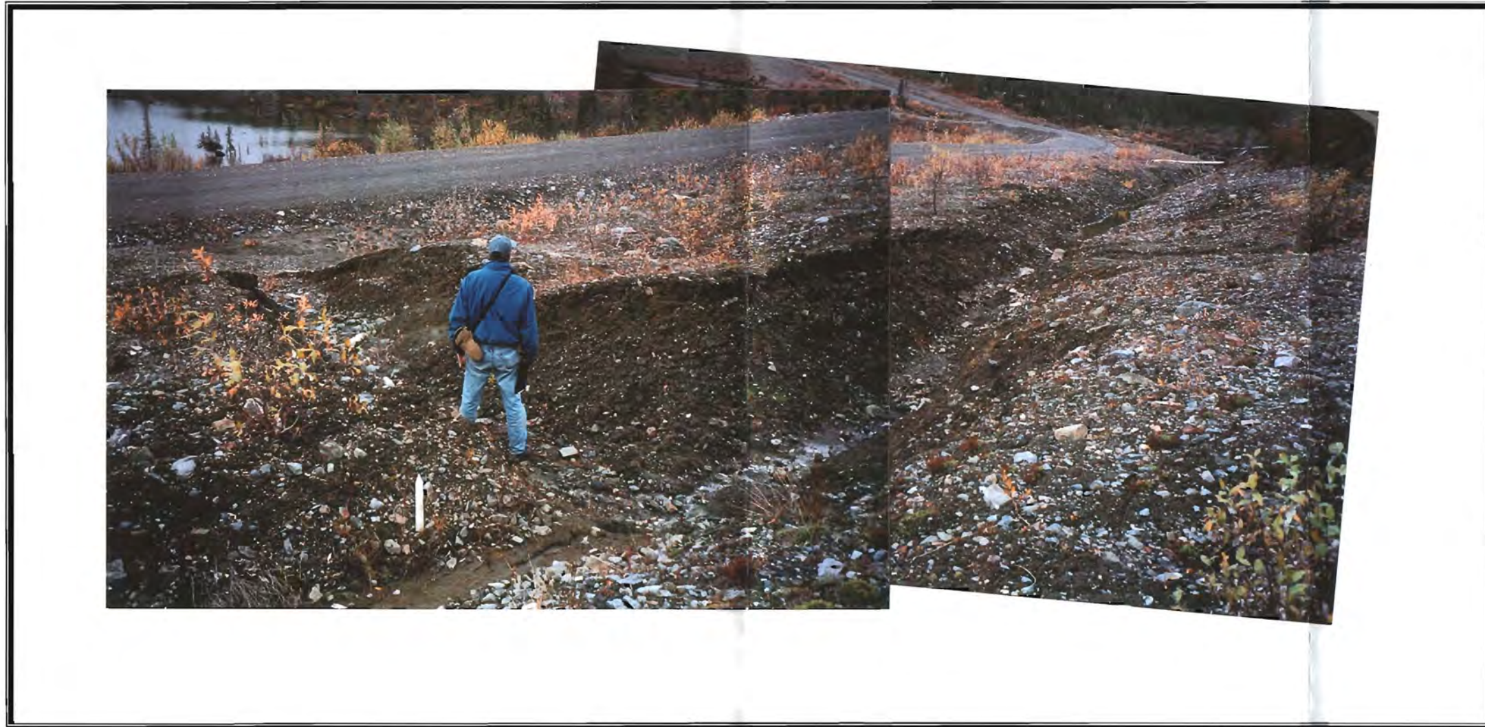
Photo 31: Erosion, failure and pounded water flowing towards failure in northwest diversion ditch.
