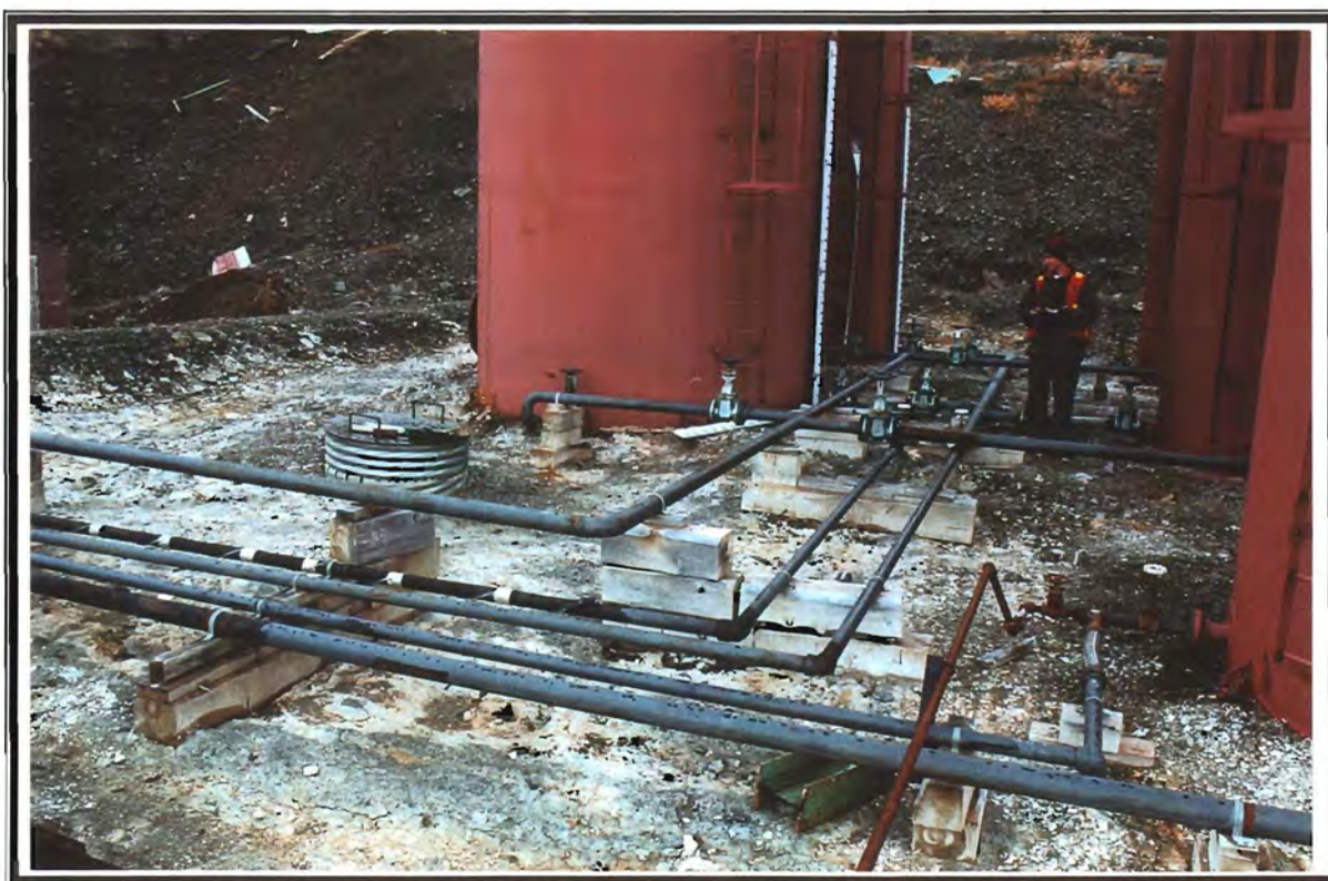
Photo 22: Interior of tank farm. Note limey/concrete liner.
