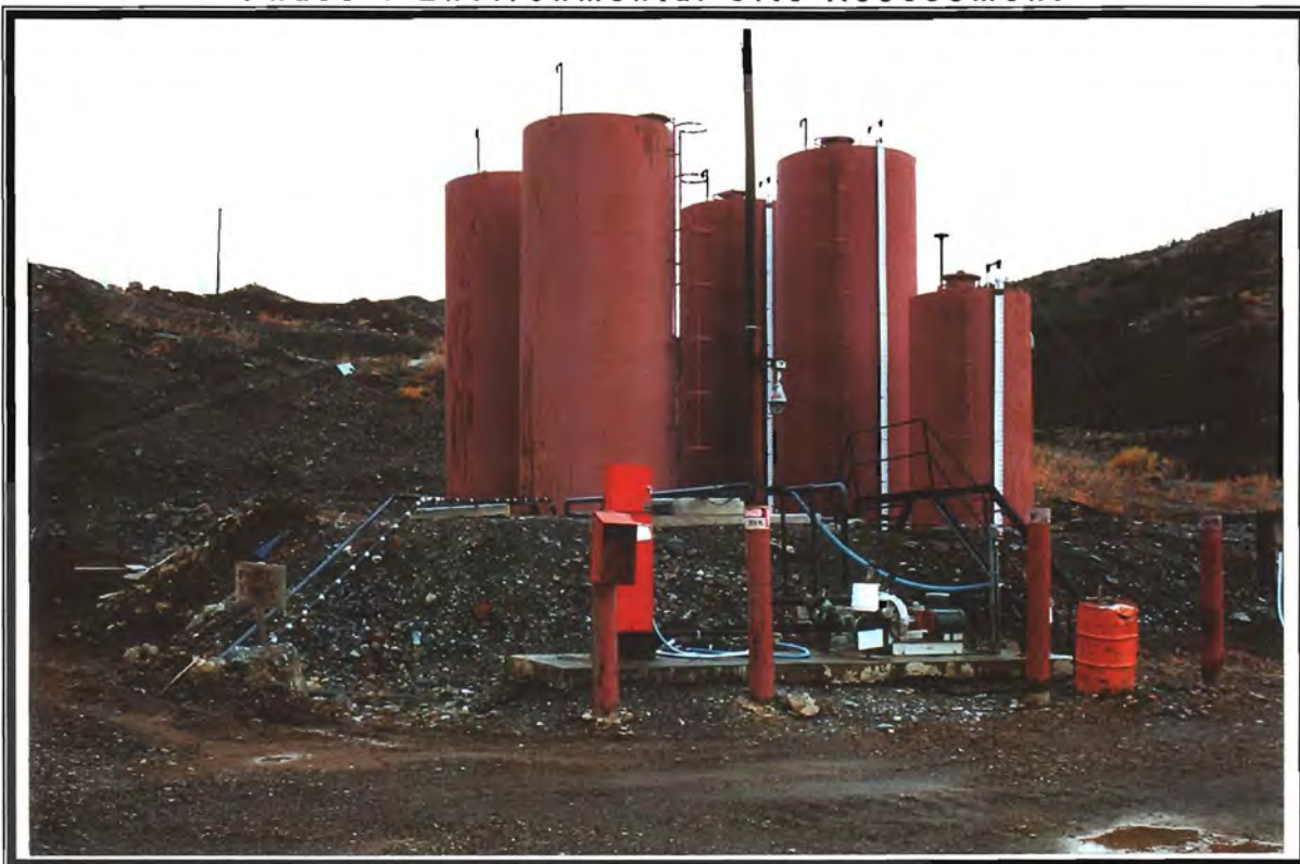
Photo 21: Tank farm and fueling island. Note drum of gasoline.
