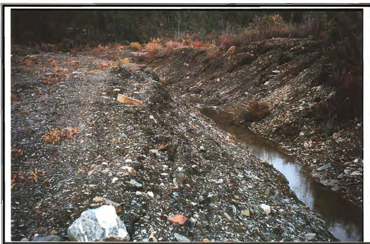
Photo 33: Ditch near confluence/Subsidiary Creek. Note failures and ponding, need for maintenance.
