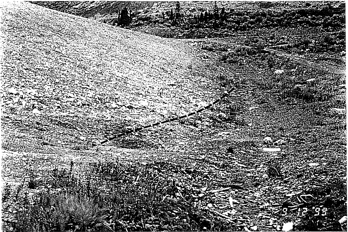
Photo 4: View of the north dam toe. The broken line indicates approximate extent of seeps.
