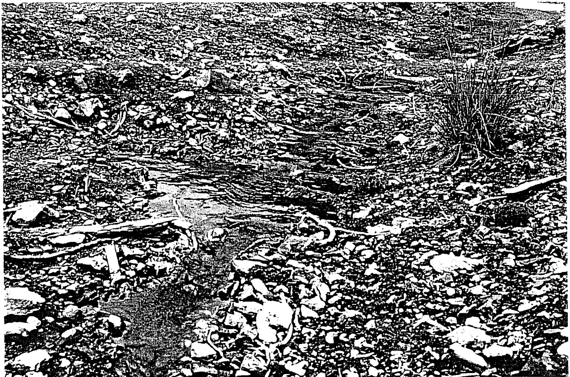
Photo 5: View of the seepage flow below the north dam toe. Note algae growing in the flow channel.
