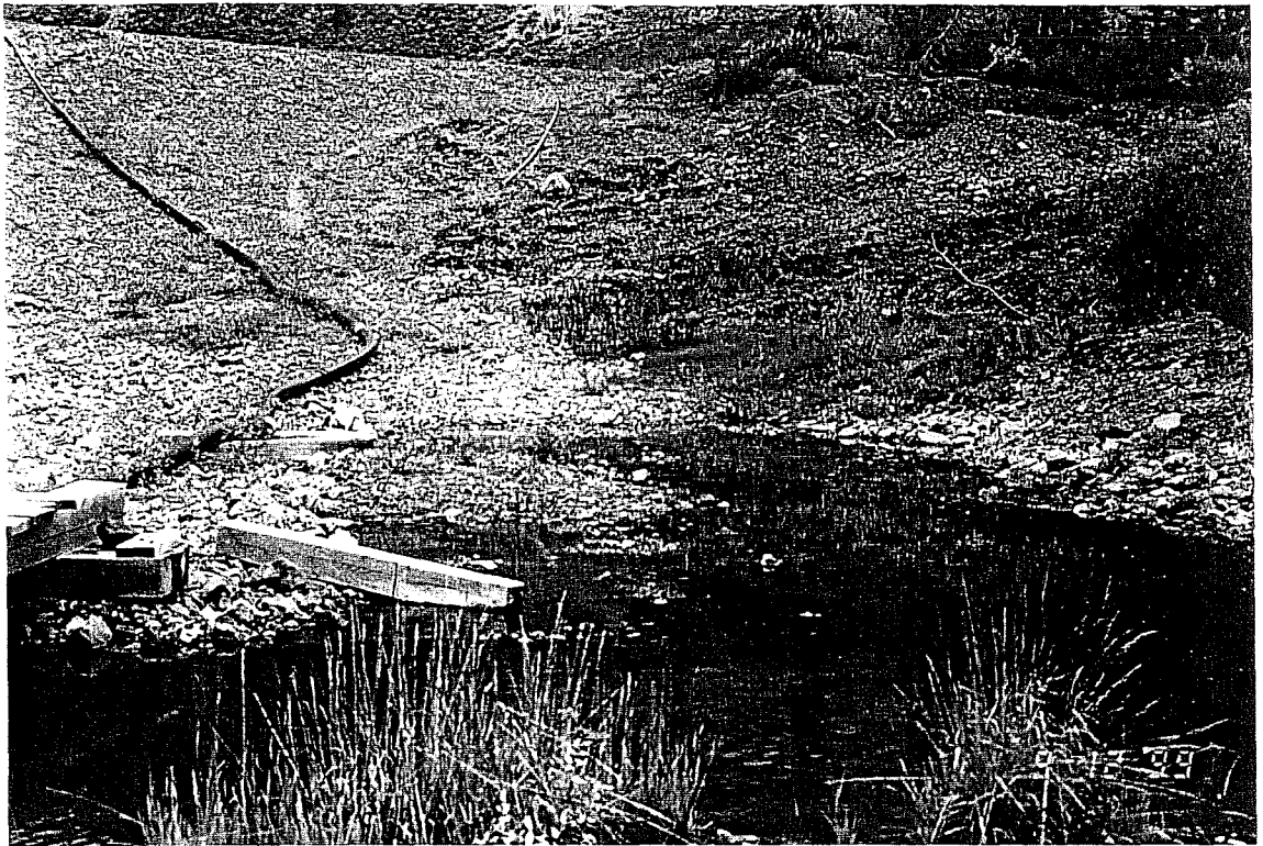
Photo 6: Ponded water below the toe of the south dam.
