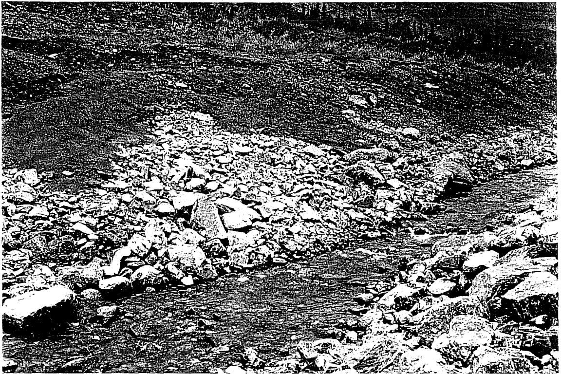
Photo 8: Thawing of permafrost on the south side of the Cache Creek diversion continues, causing extensive sloughing. The centre segment of the slump encroaches into the channel.
