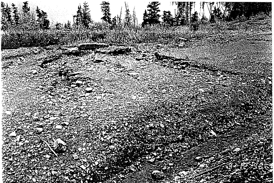
Photo 3: Erosion rills cut into the road indicate overflow from the Subsidiary Creek, likely during the spring break-up time.
