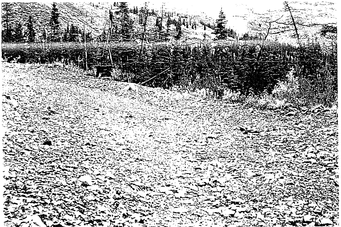
Photo 7: View of the spillway, looking north. Note shallow depth of the channel and small size rip-rap at this location.
