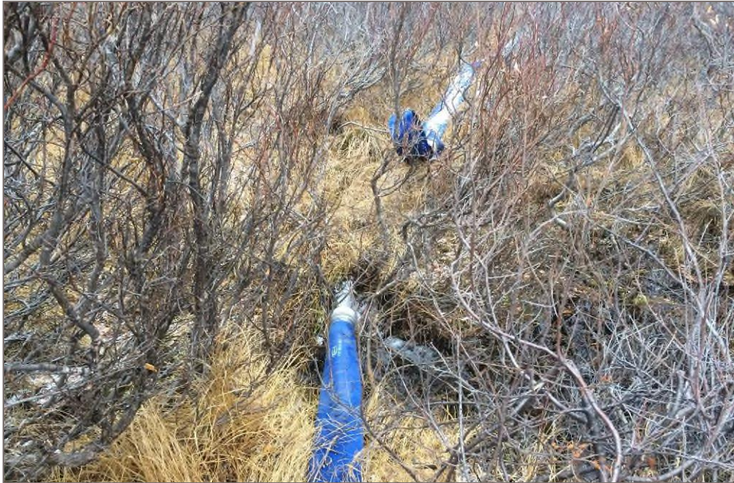
Photo 3: WW15-01 - Discharge to ground
