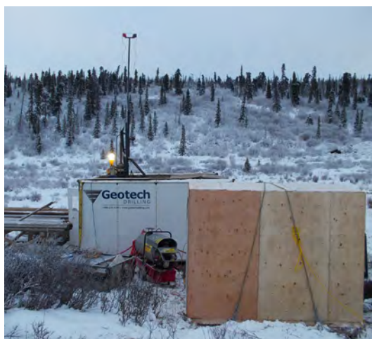
Heli-portable drill rig at geotechnical drillhole KP15-06
