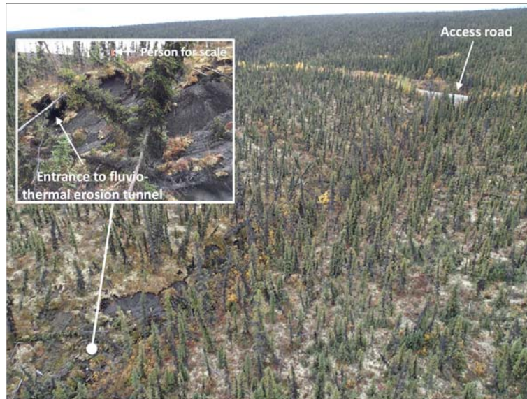
Photo 4-9. Severe thermal erosion and gulying (-Xe) along a stream crossed by the access road at KM 5.8
