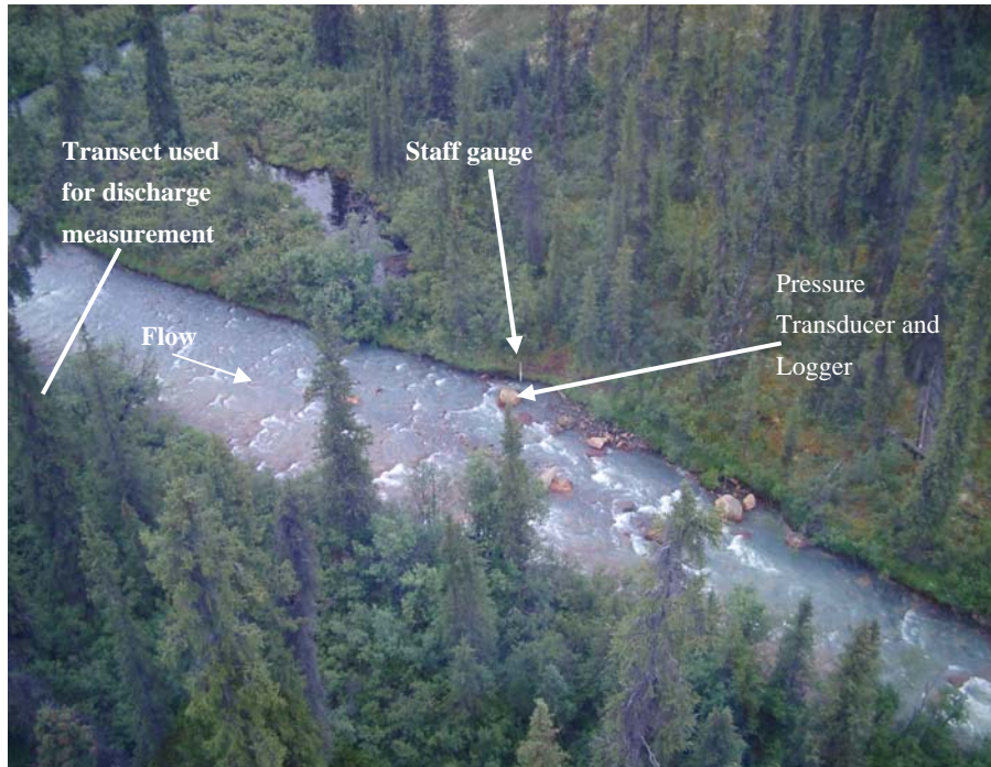
Photo A: Aerial view of the Tributary A hydrometric station.
