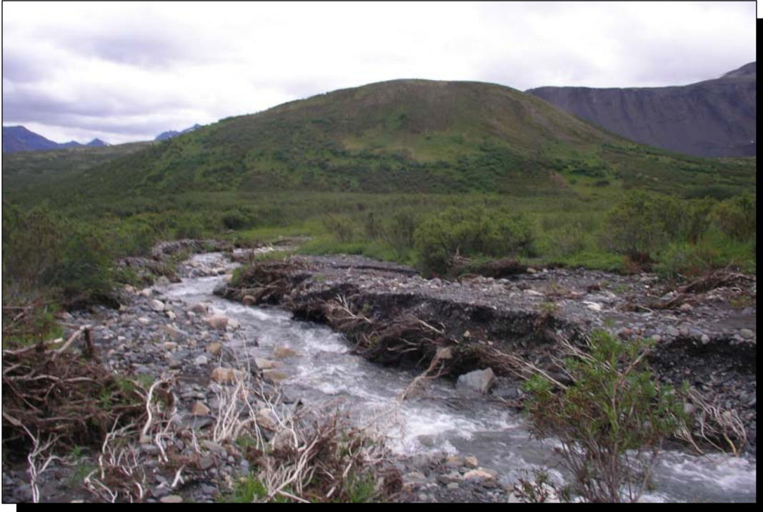
Photo 9 Station FS2 looking downstream
