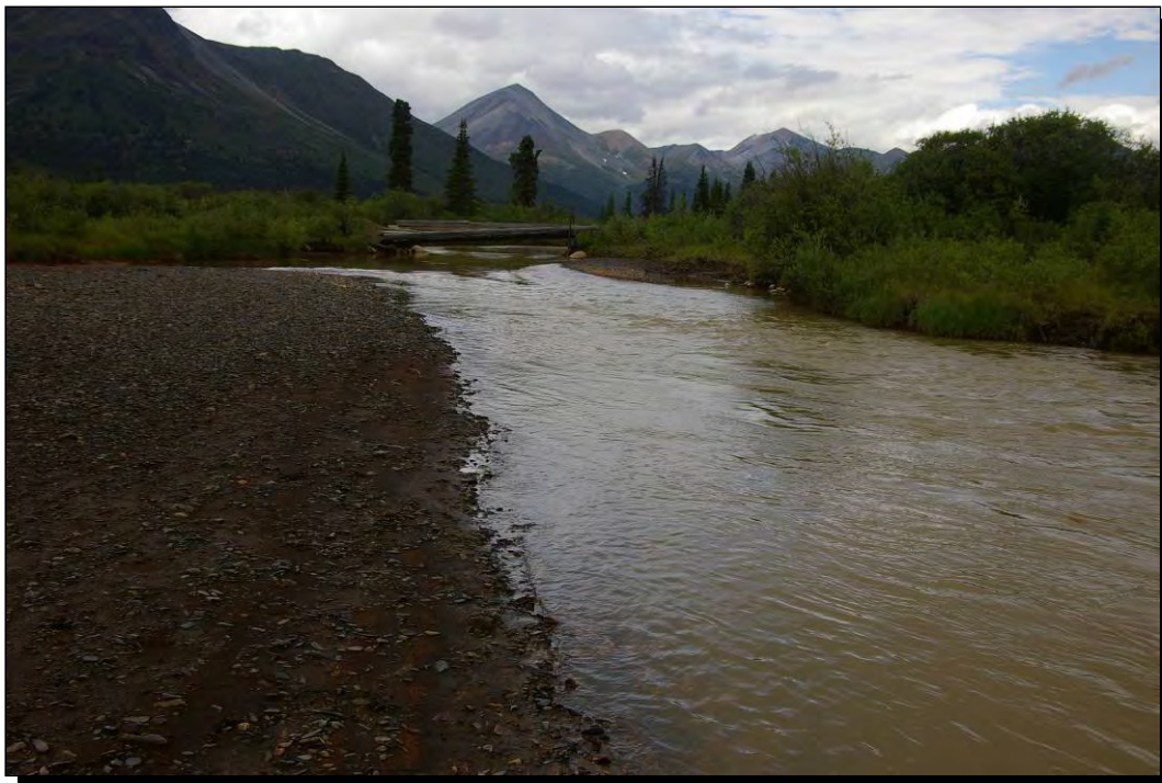
Photo 10 Existing bridge crossing on the South Macmillan River, west of the airstrip, August 2008.
