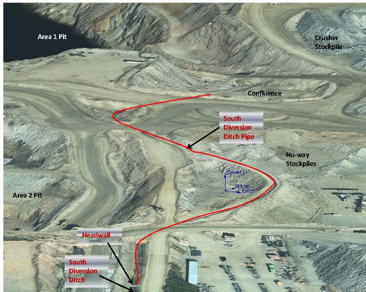
Figure 9-2: South Diversion Ditch (September, 2012).
