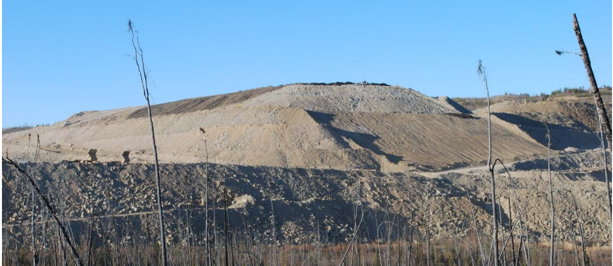
Figure 8-1: Main Waste Dump near the end of construction season 2011 (September).
