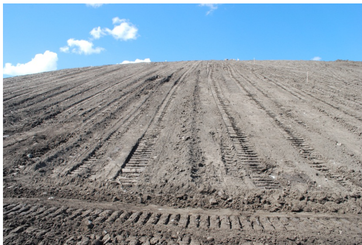
Figure 8-5: Plot surface after grading with the D6 Cat dozer.
