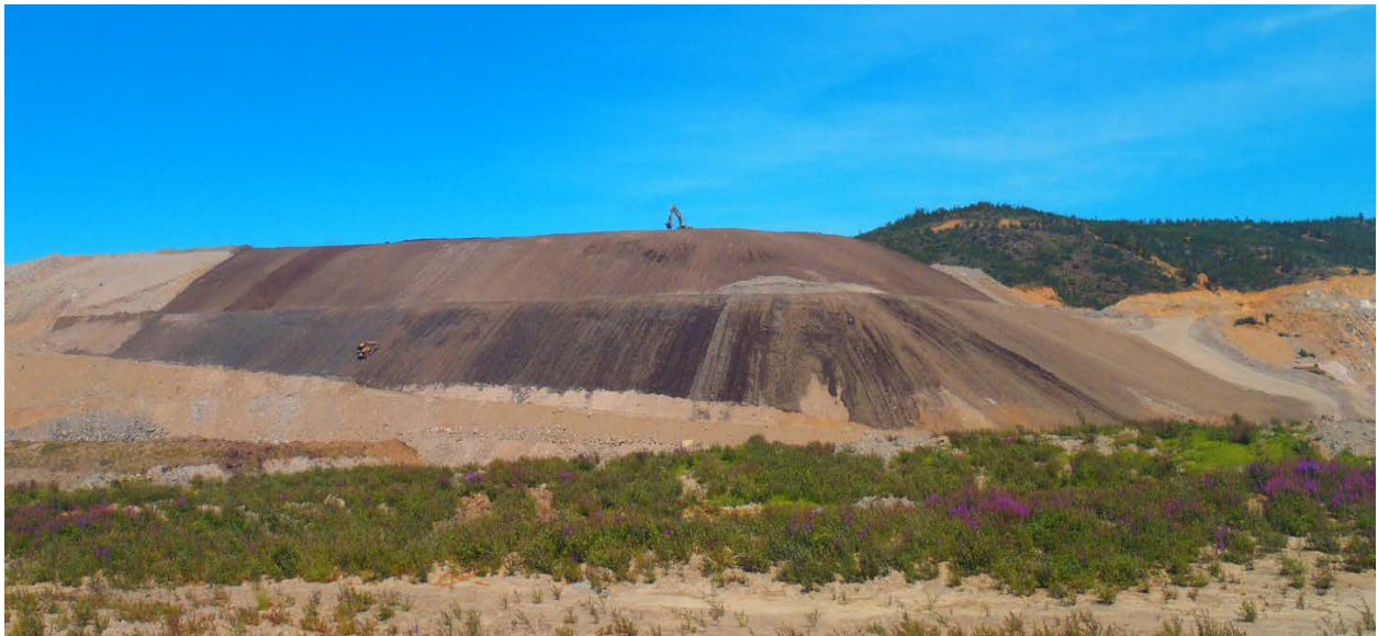
Figure 8-2: Main Waste Dump as it appeared in July 2012 with final placement of overburden into distinct plots.
