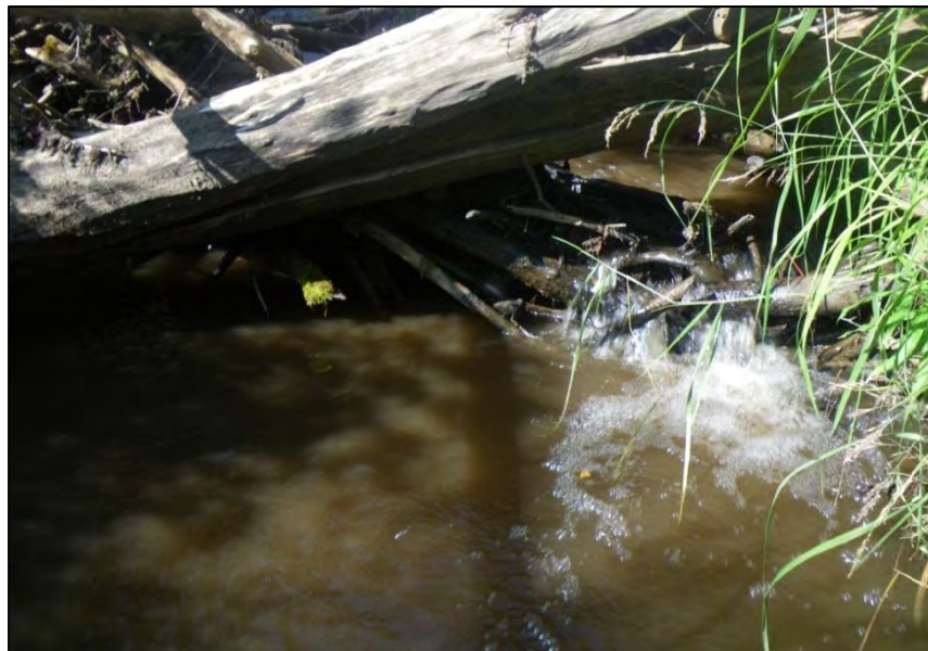
Figure 5-4 Fish Barrier on August 13, 2012.
