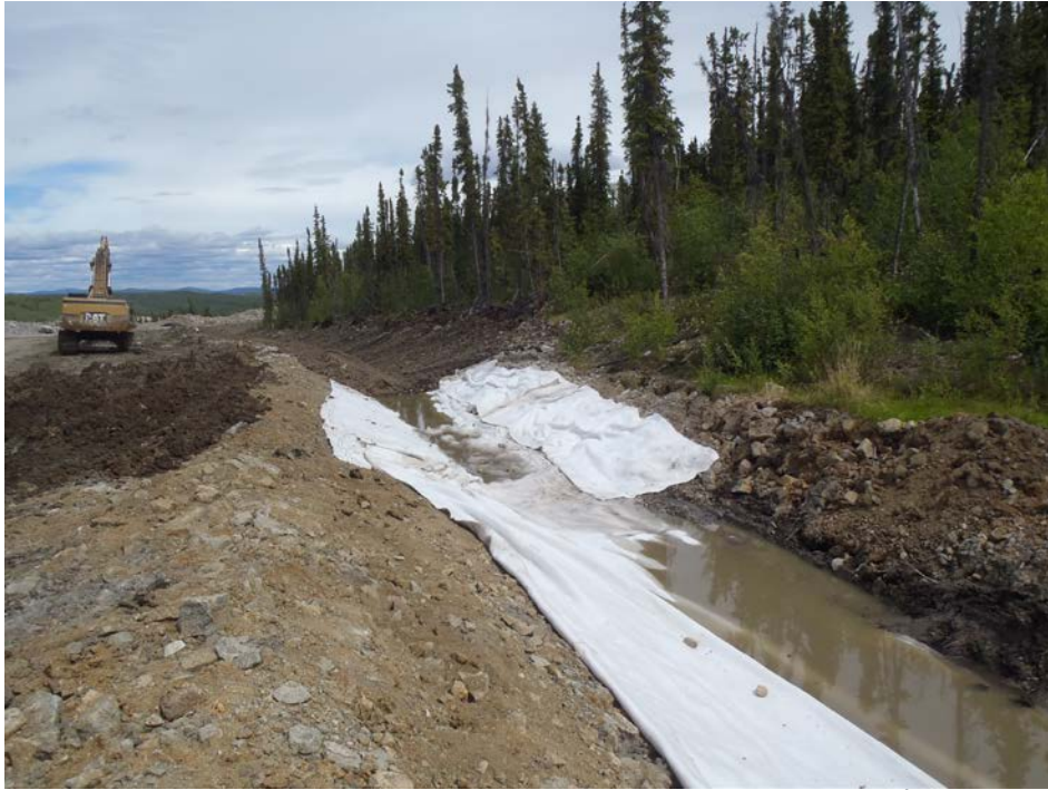
Figure 7: Between Section C and D Looking East, June 23 rd , 2014
