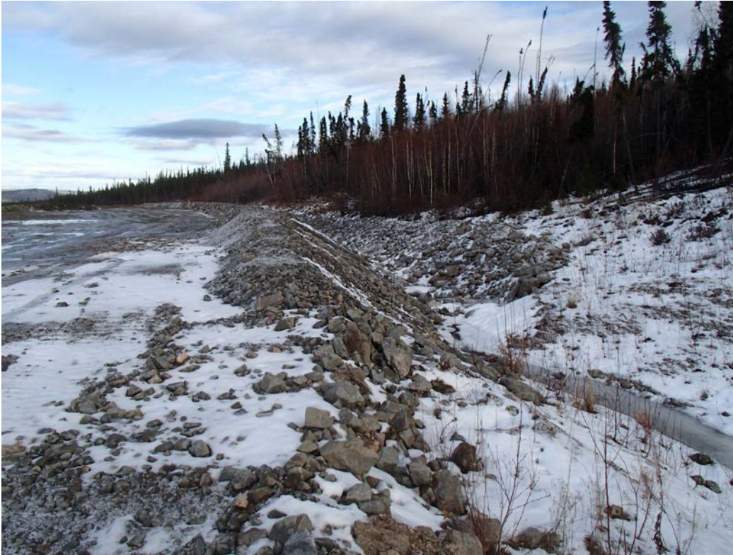
Figure 15: Section A Looking West, Oct 6 th , 2014
