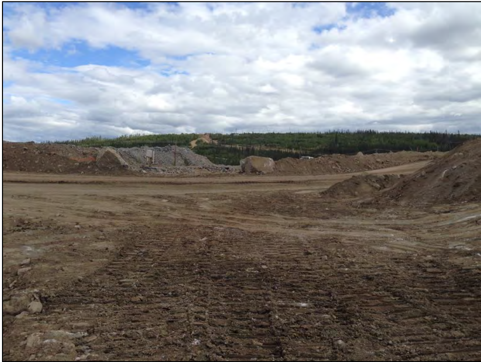
Figure 5 – Spillway across haul road – northeast facing
