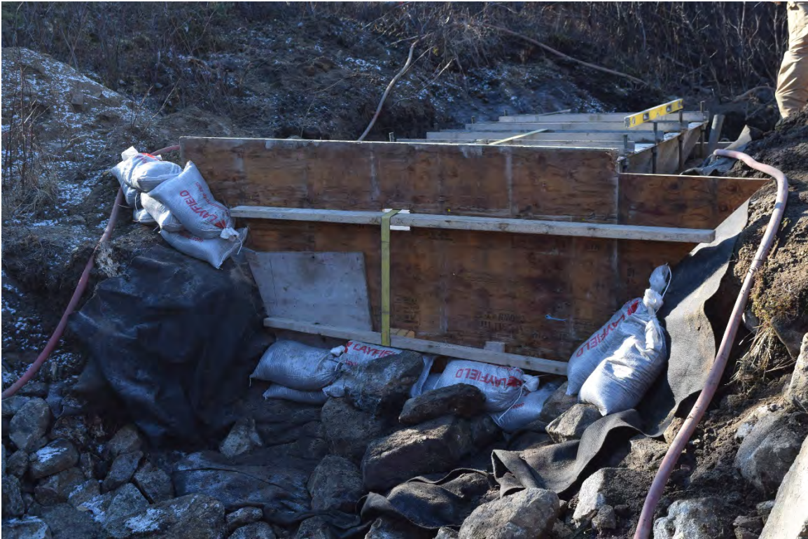
Photo 4: Downstream concrete forms for backfill pour.
