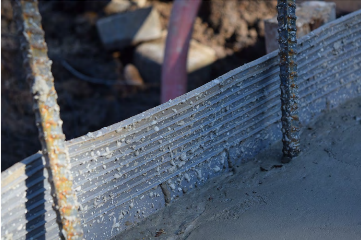
Photo 6: Flexible membrane that seals between the base and wing walls.
