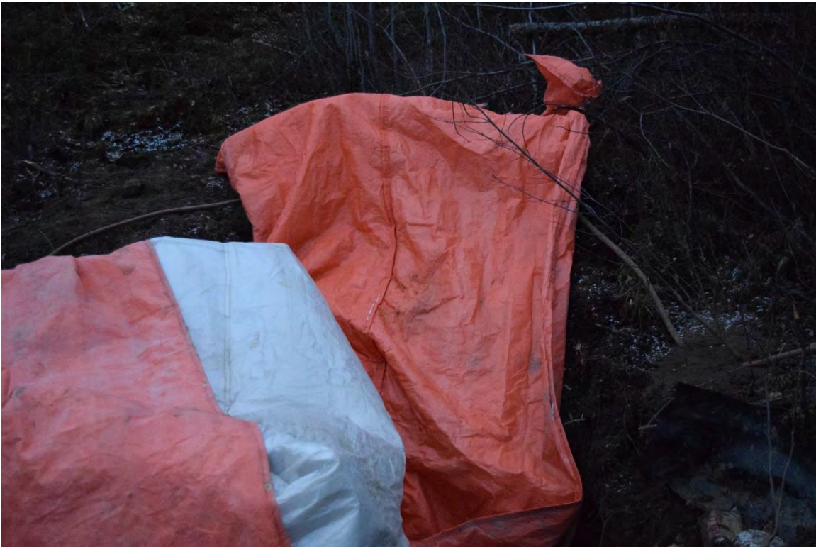
Photo 22: Insulated tarp covering exposed permafrost bank from heated concrete intake structure.
