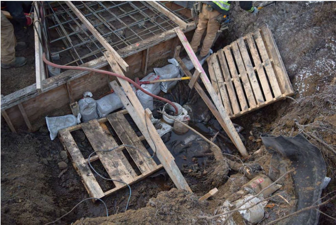
Photo 16: Sump pump dewatering the upstream formwork and excavation area.
