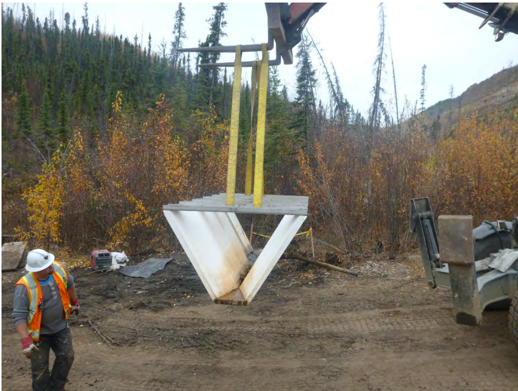
Photo 2: Flume removal
