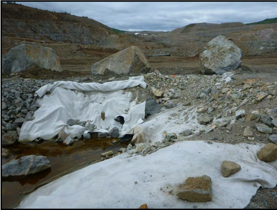
Figure 2 – Installation of geotextile at SDD inlet ditch.
