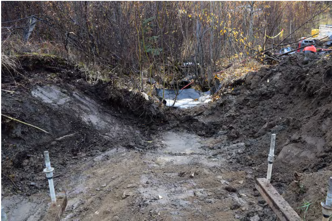
Photo 9: Intermediate backfill compaction and erosion barrier construction (Looking Upstream)
