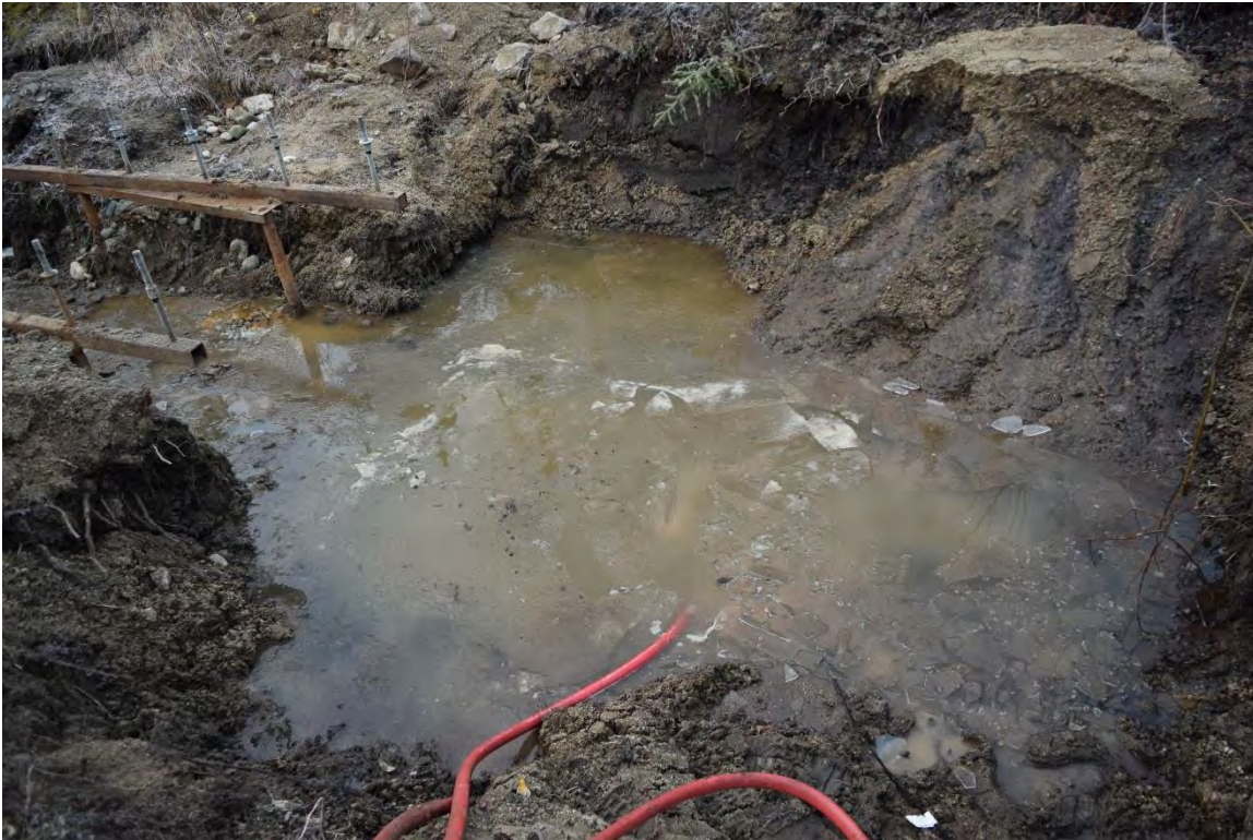
Photo 12: Upstream excavation prior to base backfill compaction
