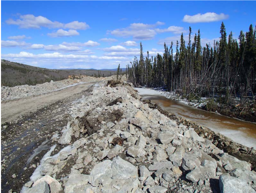
Figure 1: Between Section C and D Looking East, April 19 th , 2014
