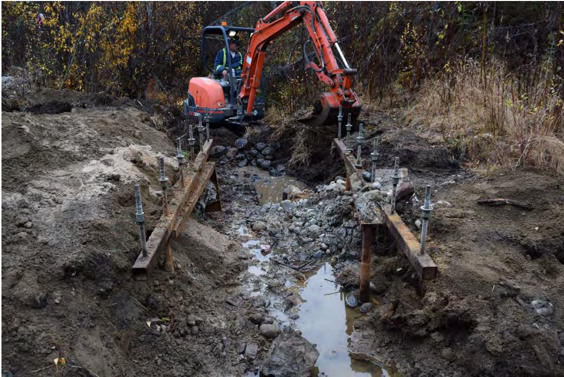
Photo 8: Flume support structure after excavation
