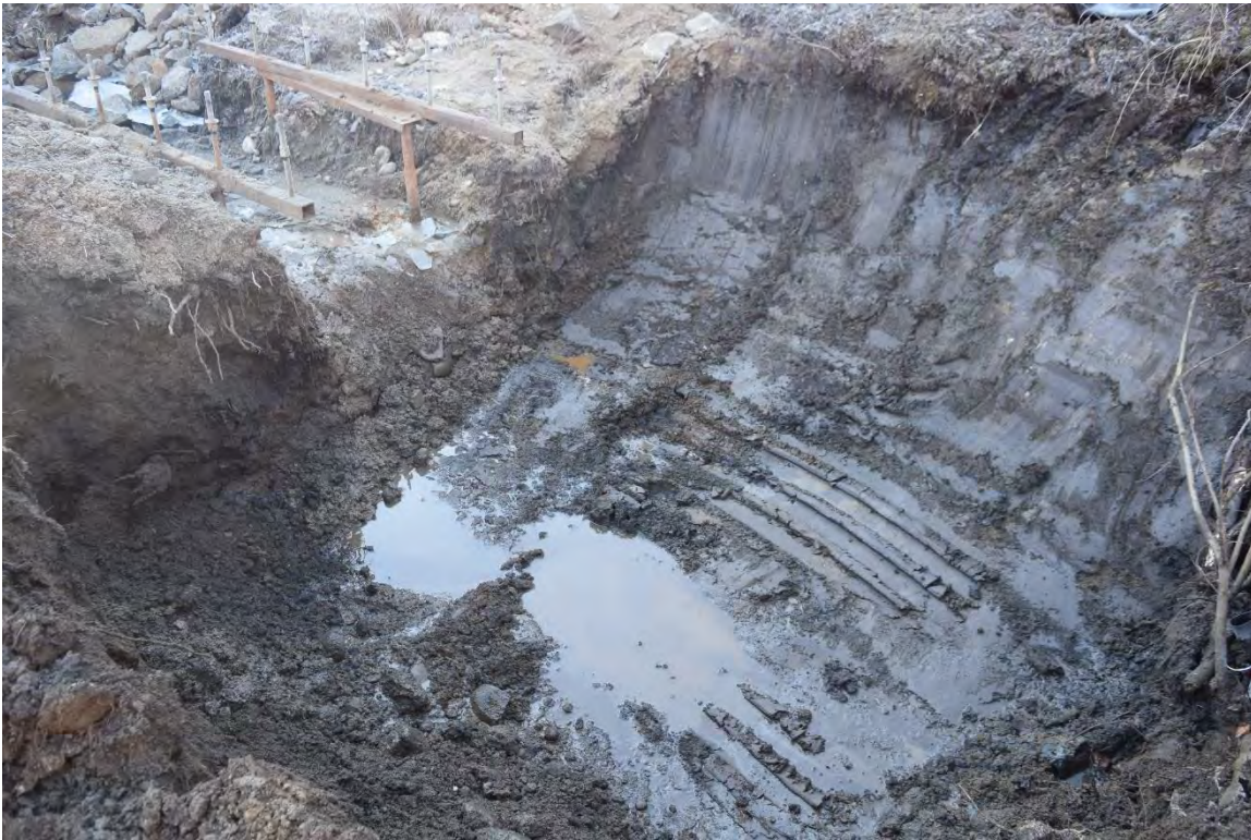
Photo 12: Upstream excavation prior to base backfill compaction
