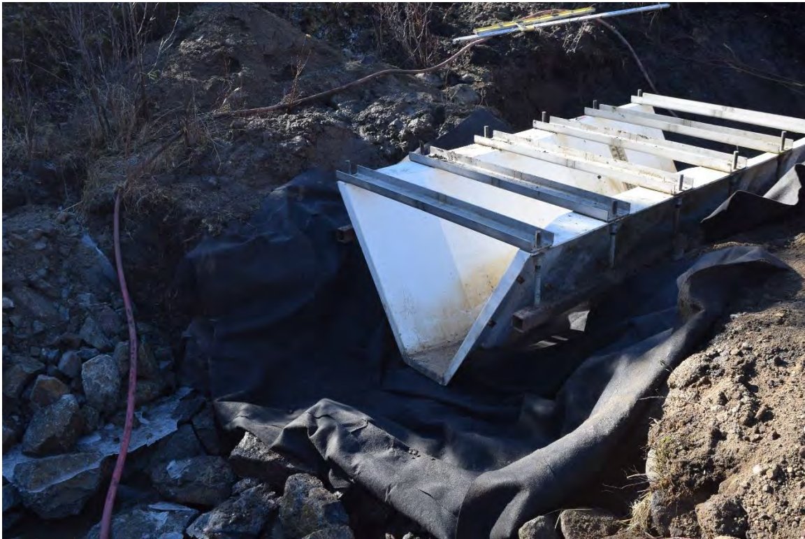
Photo 14: Geotextile installation beneath flume.
