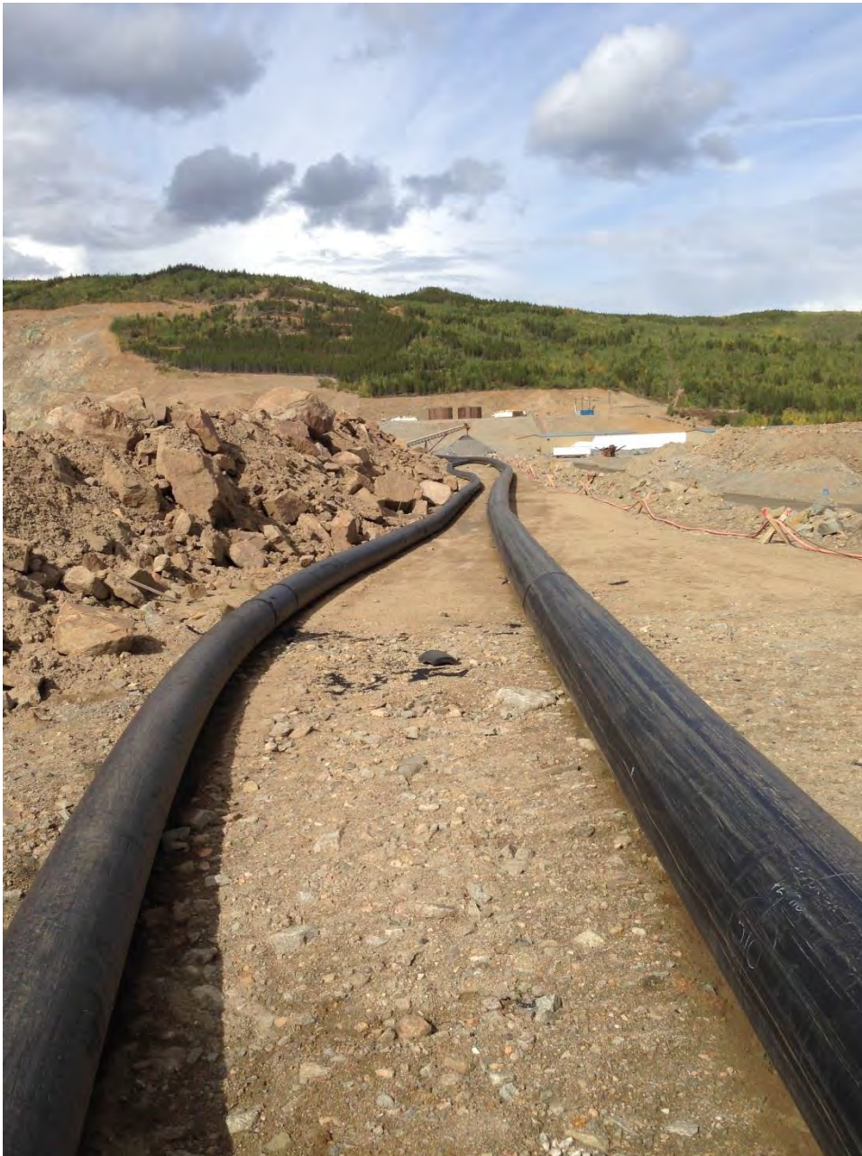
Figure 6 – 24" and 16" piping navigating around the Area 2 pit to the Confluence
