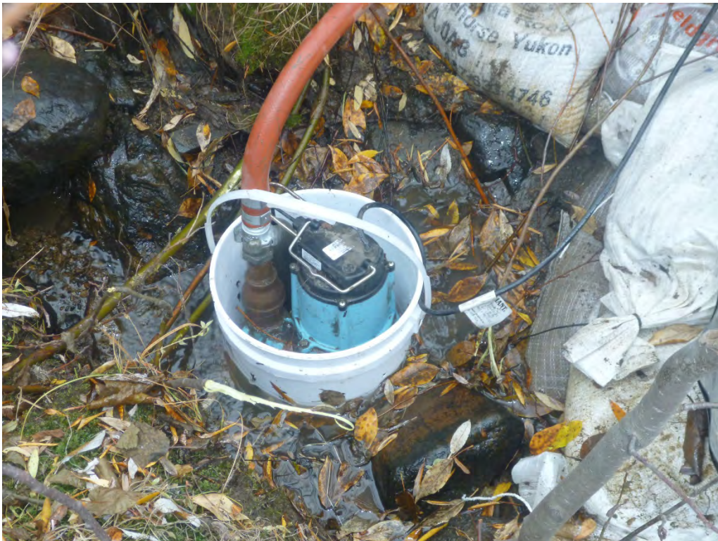
Photo 4: Sump pump discharging into creek bypass
