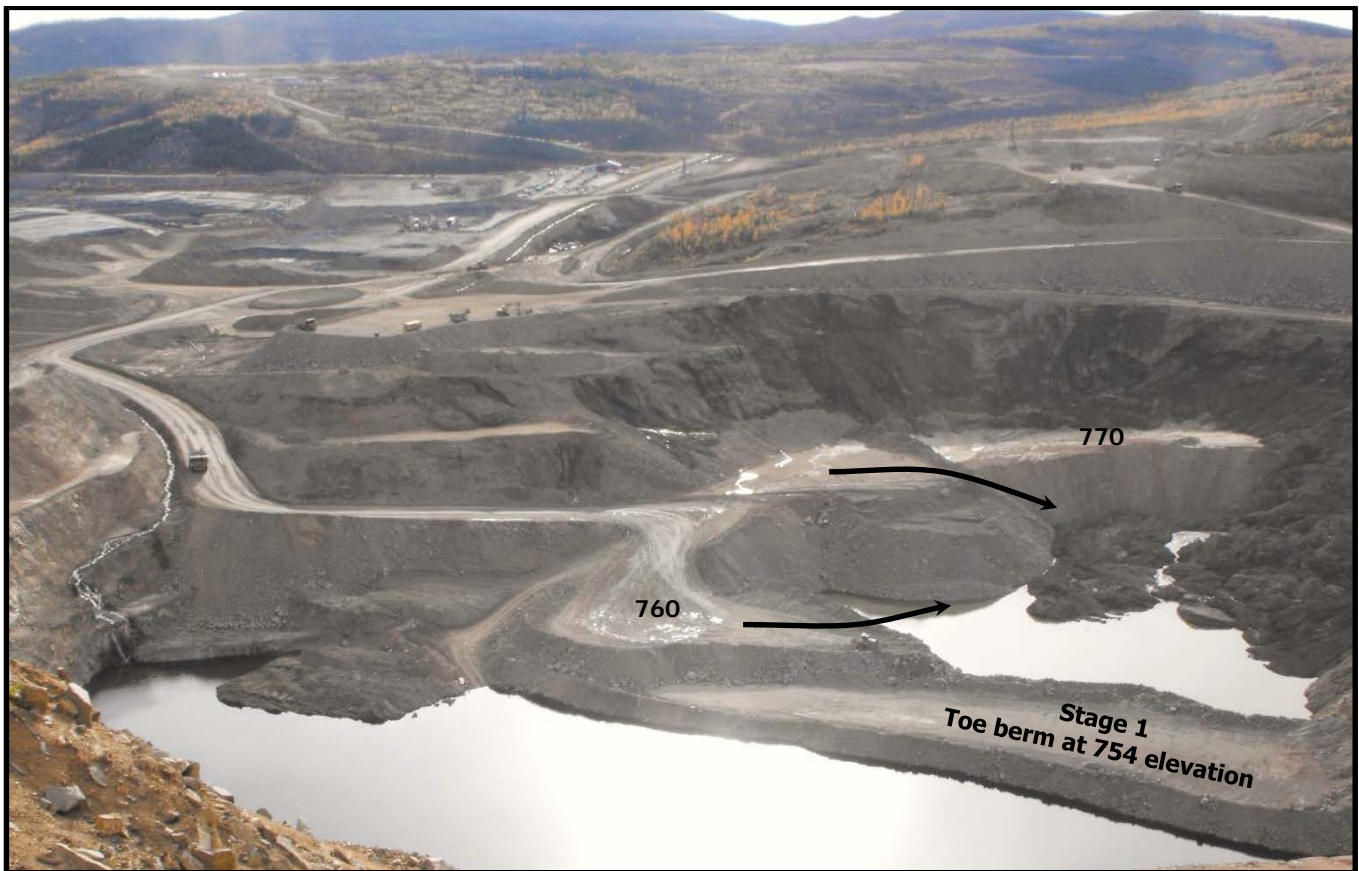
Figure 3-5: Photo showing Stages 1 and 2 of buttress development. September 17, 2011, looking S-SE.
