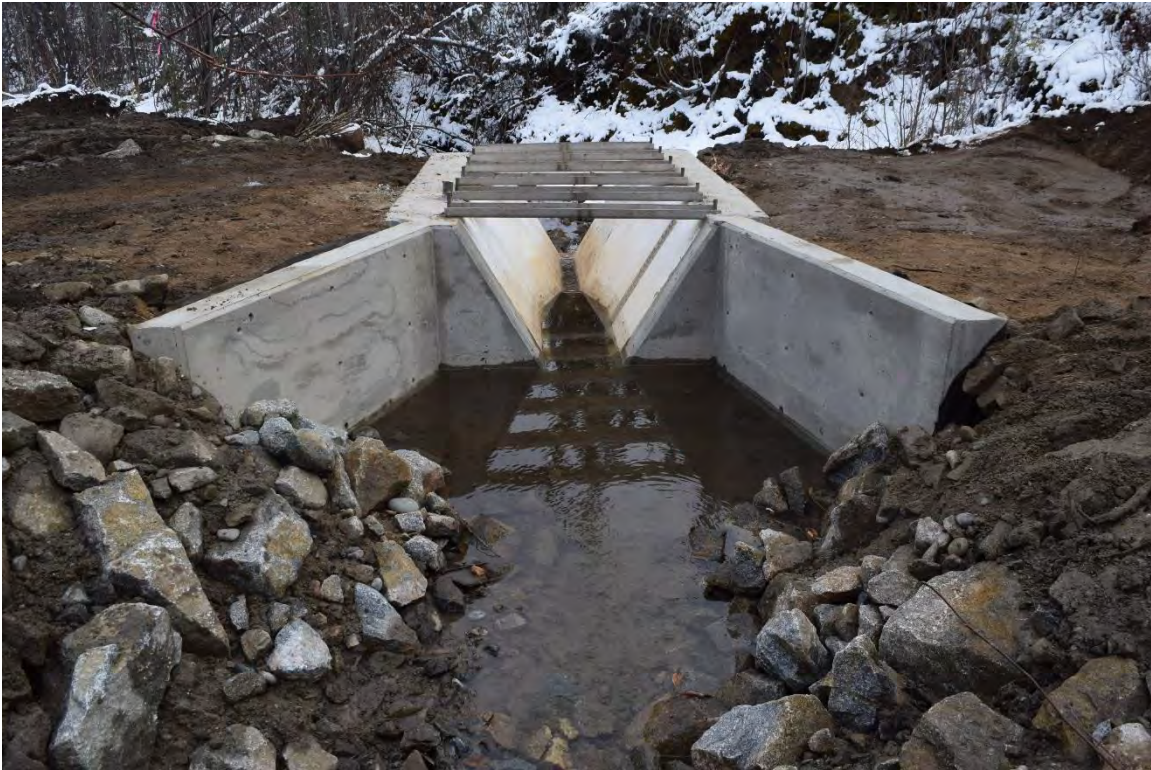
Photo 24: Wing wall entrance section incorporated with riprap.
