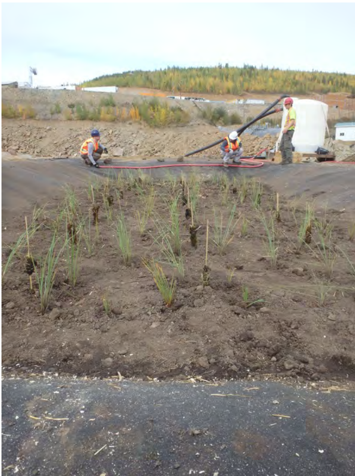
Figure 12. C. aquatilis planted within grid of moss stakes in demonstration-scale CWTS cell 2A, and influent perforated pipe being laid in place.
