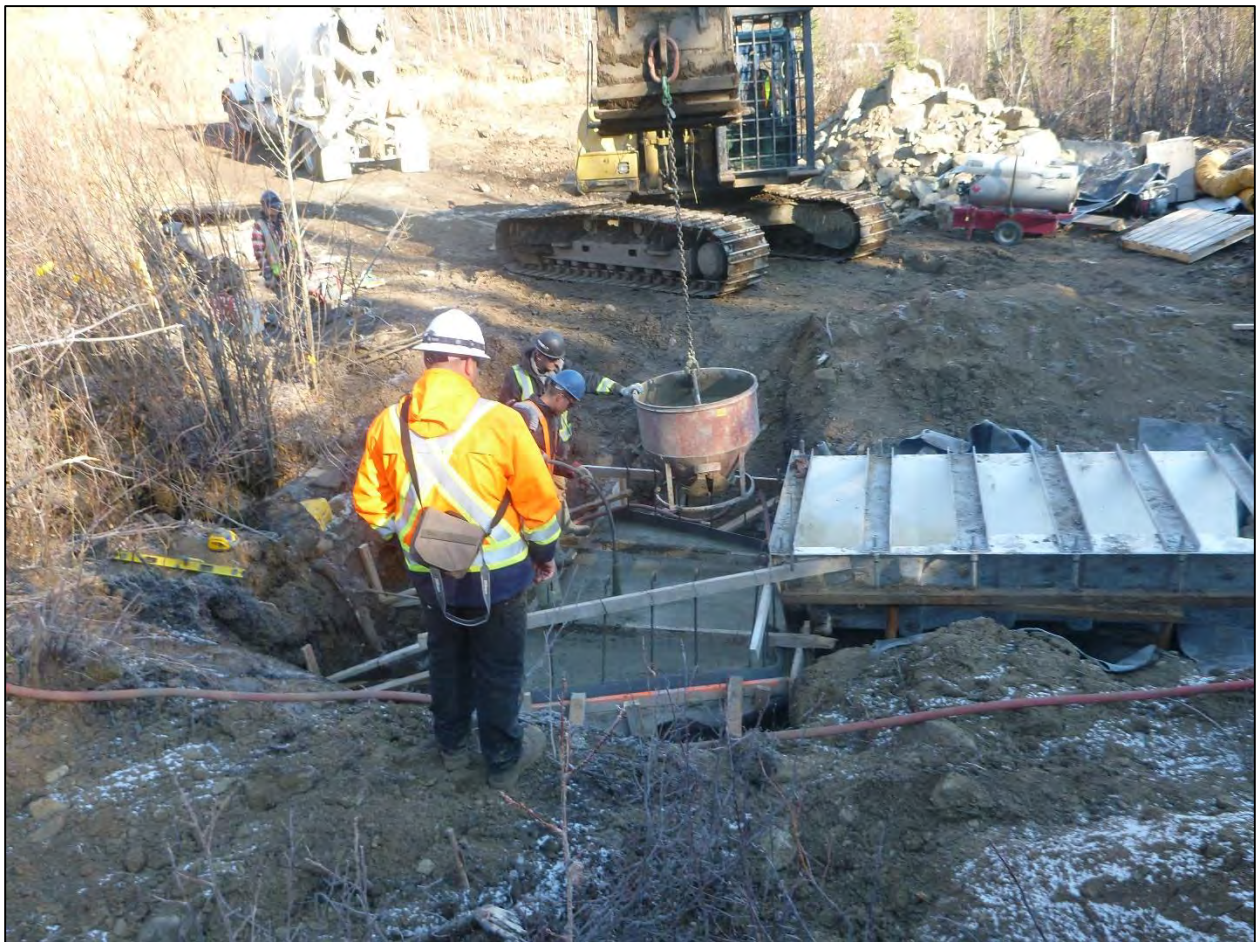
Photograph 7-1: Wing Wall and Footing Construction for W3 Flume Rebuild
