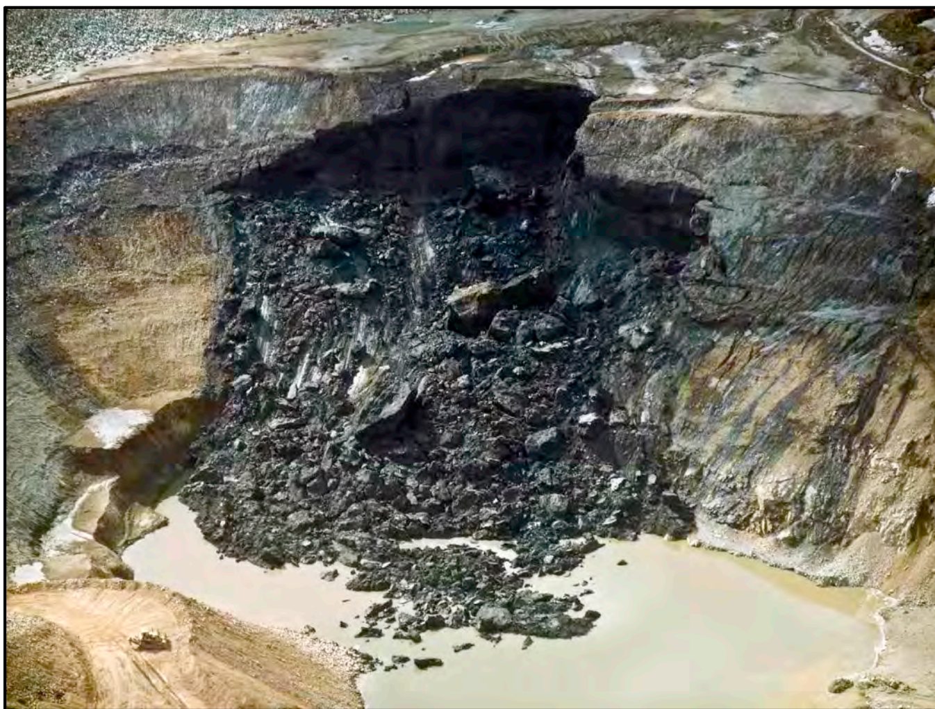
Figure 1-5: South wall failure, Main pit, April 2011. Aerial photo, looking southwest. Start of buttress construction visible at bottom left corner of the photo.
