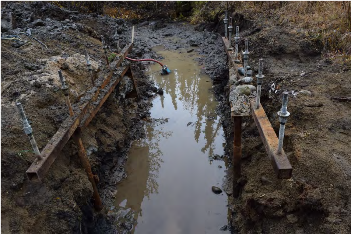
Photo 6: Dewatering seepage in the excavation. (Looking Downstream)
