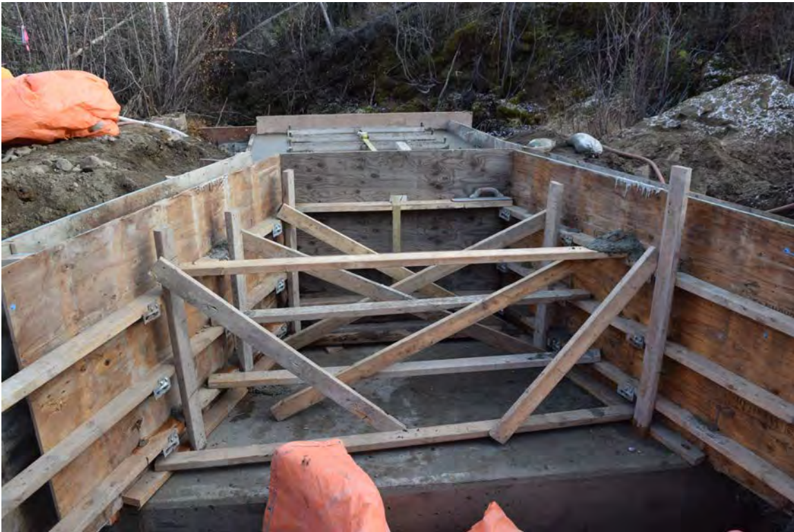
Photo 12: Wing wall cross-bracing
