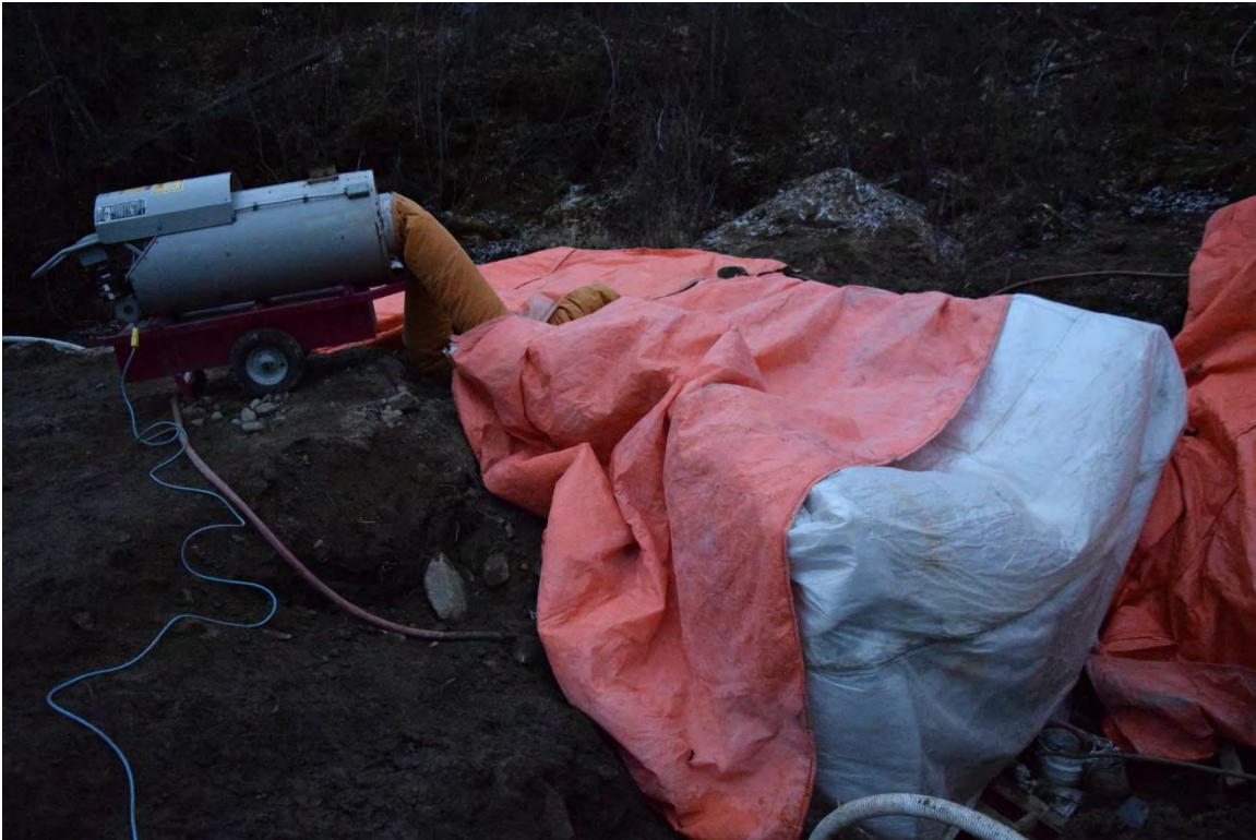
Photo 22: Insulated tarp covering exposed permafrost bank from heated concrete intake structure.
