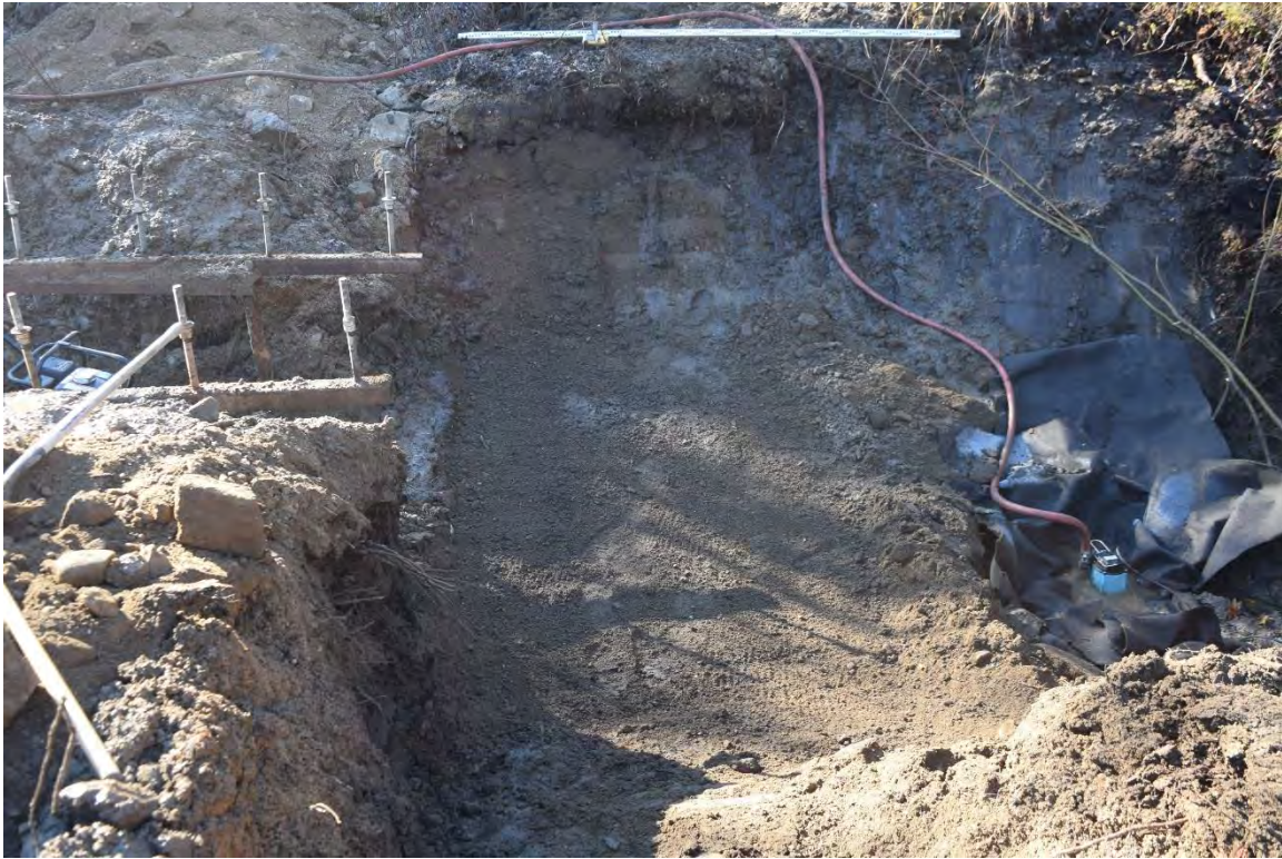
Photo 14: Geotextile installation beneath flume.
