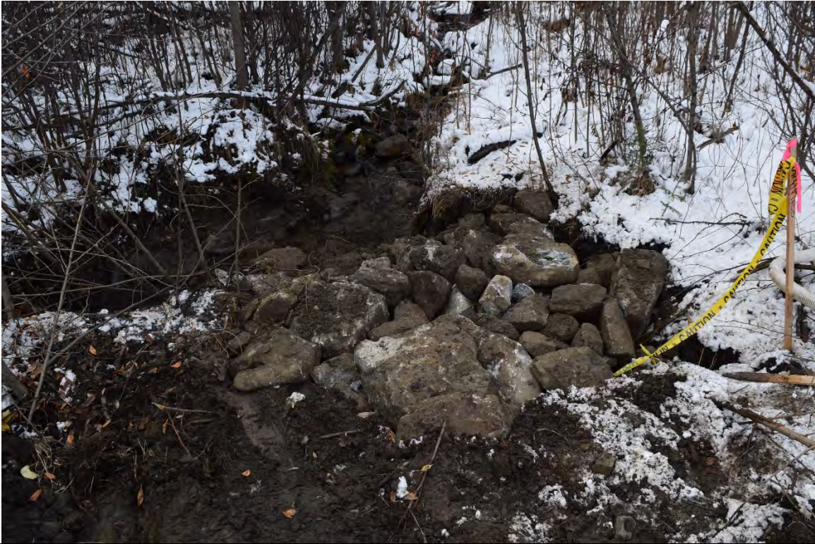
Photo 10: Riprap protection at former diversion pipe discharge
