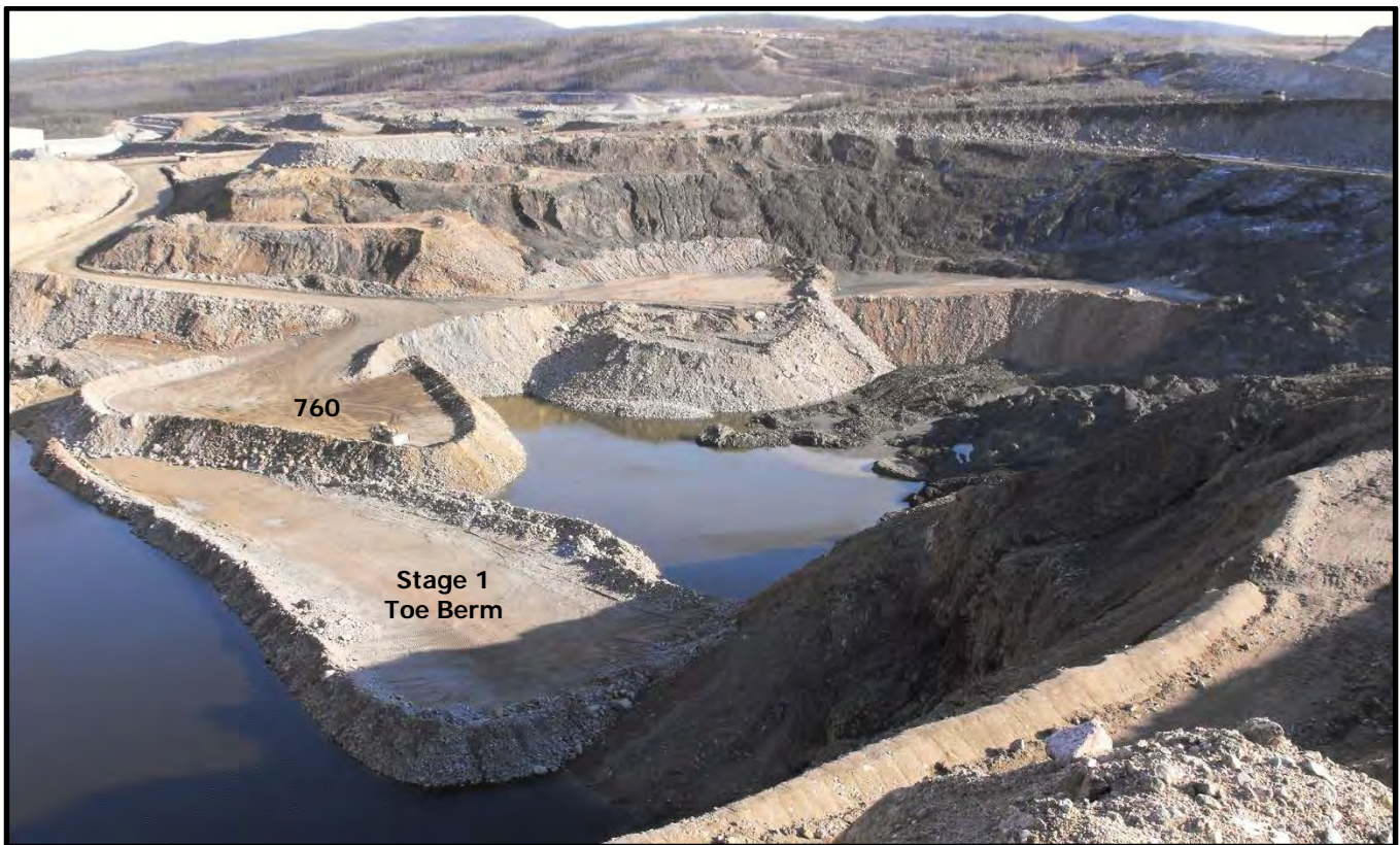
Figure 3-6: Buttress development, October 2, 2011, looking E-SE.
