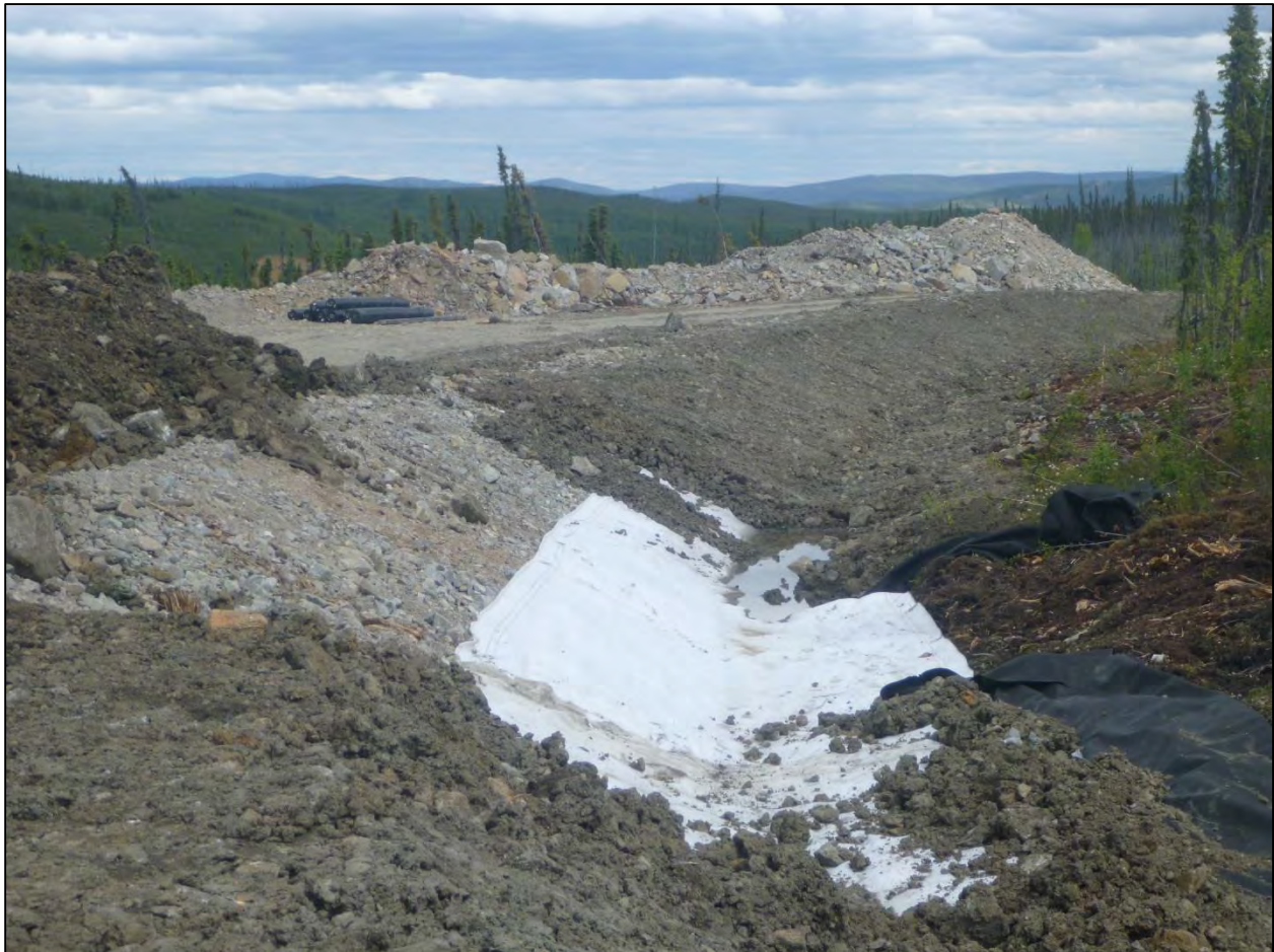
Photograph 7-2: TDD Shaped and Graded Ditch Segment Showing GCL and Geotextile Cloth
