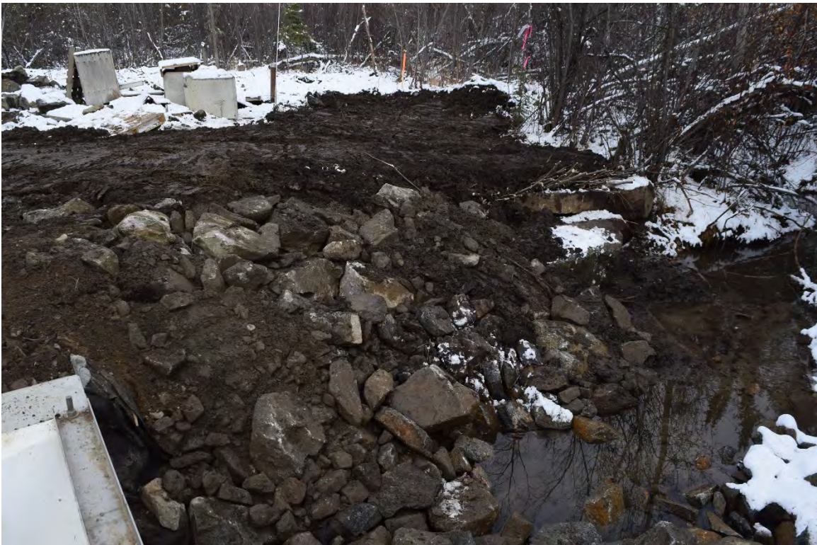
Photo 10: Riprap protection at former diversion pipe discharge
