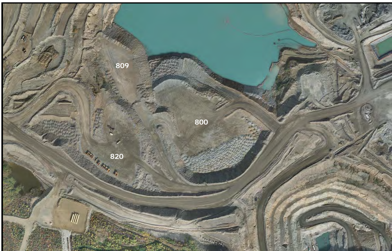
Figure 3-9: Aerial ortho-photo of South Wall Buttress, September 9, 2014.
