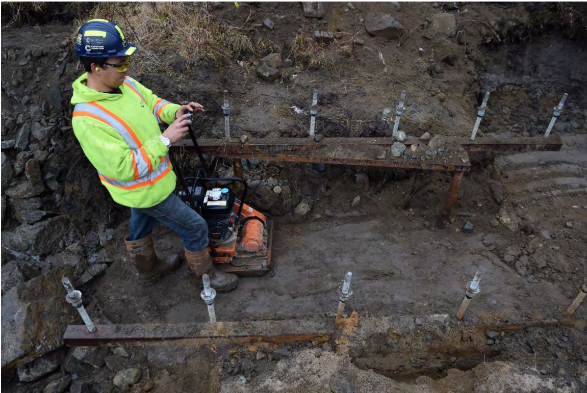
Photo 10: Compacting backfill between steel support structures.
