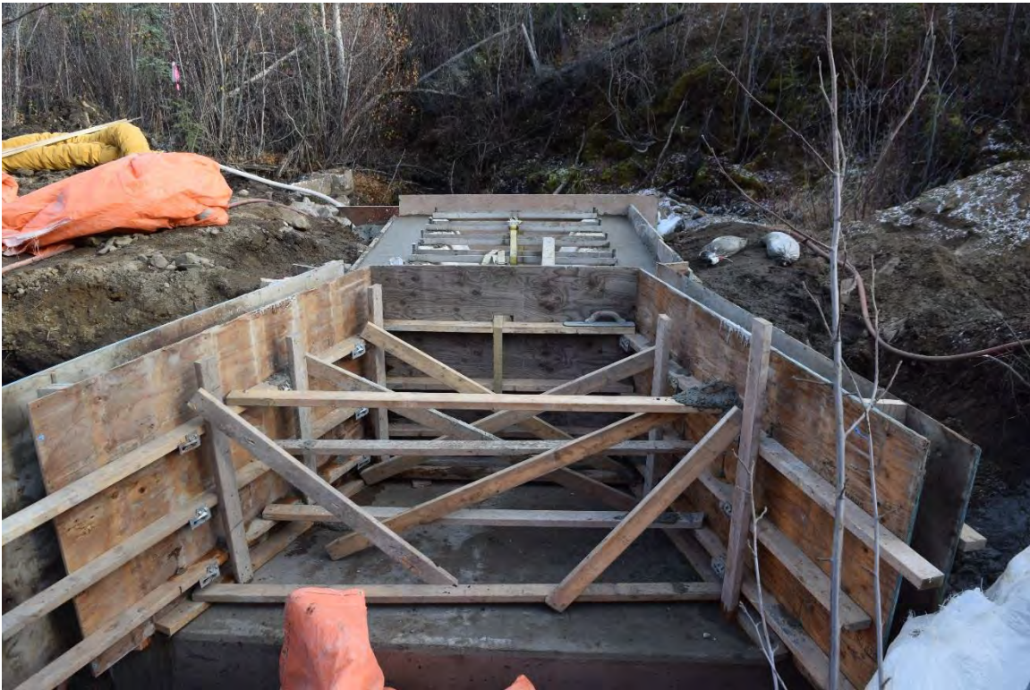
Photo 20: Formwork cross bracing.
