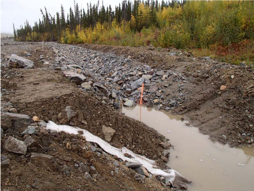
Figure 11: Transition Zone GCL to 12oz Geotextile, Sept 4 th , 2014
