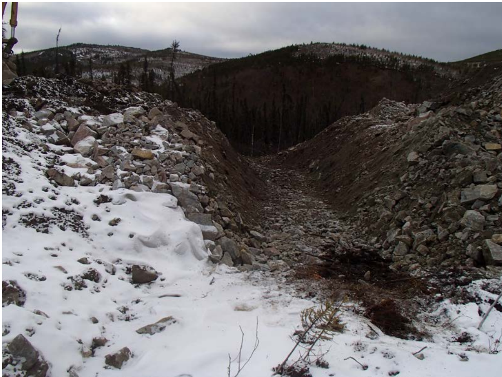
Figure 18: Temporary End Ditch Discharge, Future Works Proposed In Phase 5,6 Mine Plan
