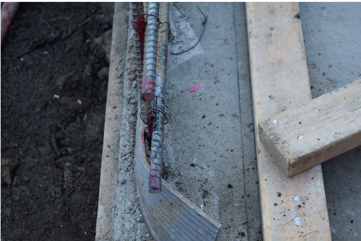
Photo 8: Wing wall form sill plates.
