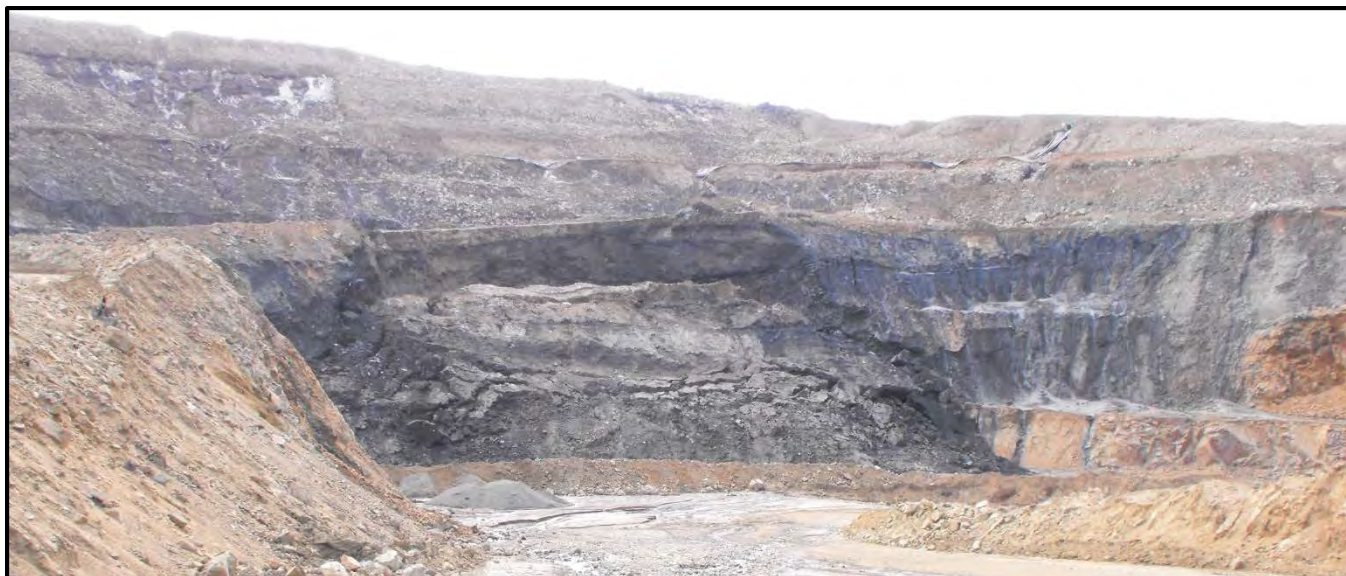
Figure 1-4: Main pit, Stage 3, May 2009 south wall failure. Looking south-southwest, camera positioned at bottom of pit.
