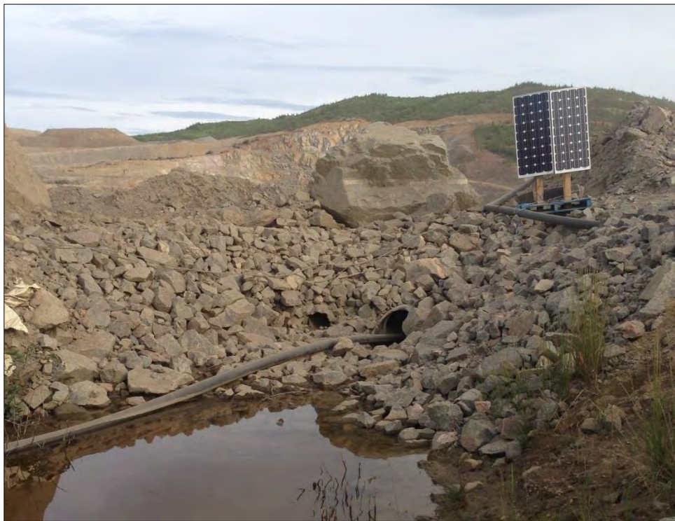
Figure 3 – Completed SDD inlet ditch.
