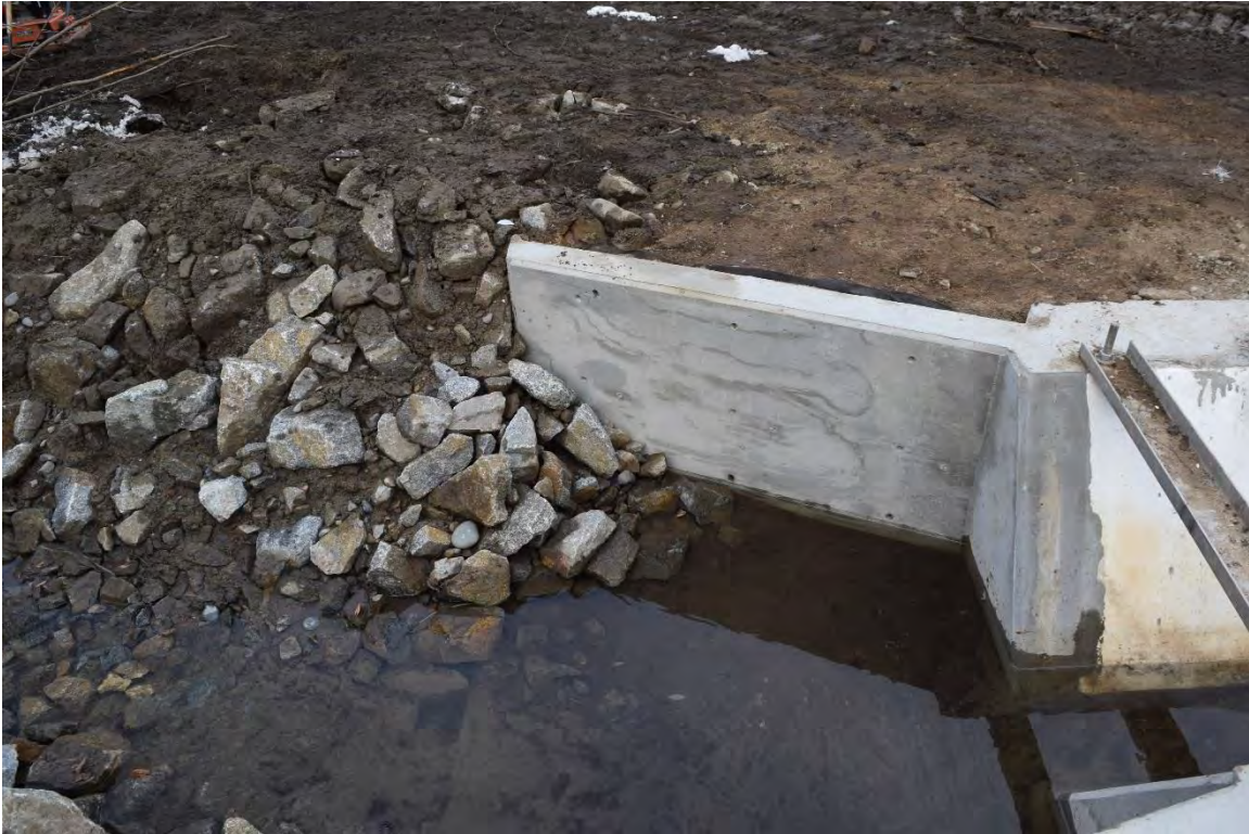
Photo 24: Wing wall entrance section incorporated with riprap.
