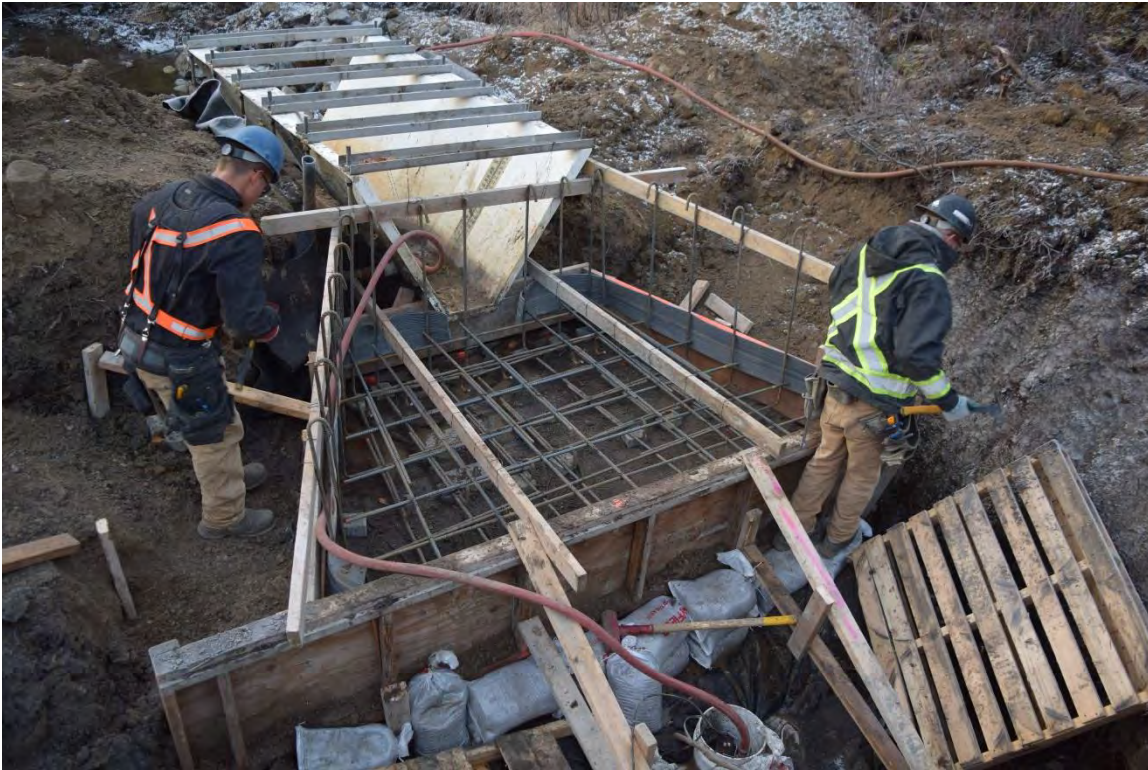
Photo 16: Sump pump dewatering the upstream formwork and excavation area.
