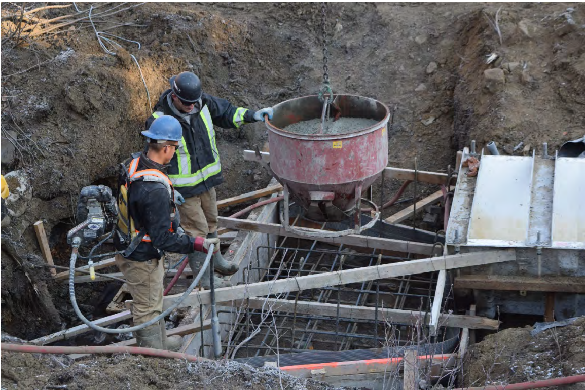
Photo 2: Intake structure base concrete pour.
