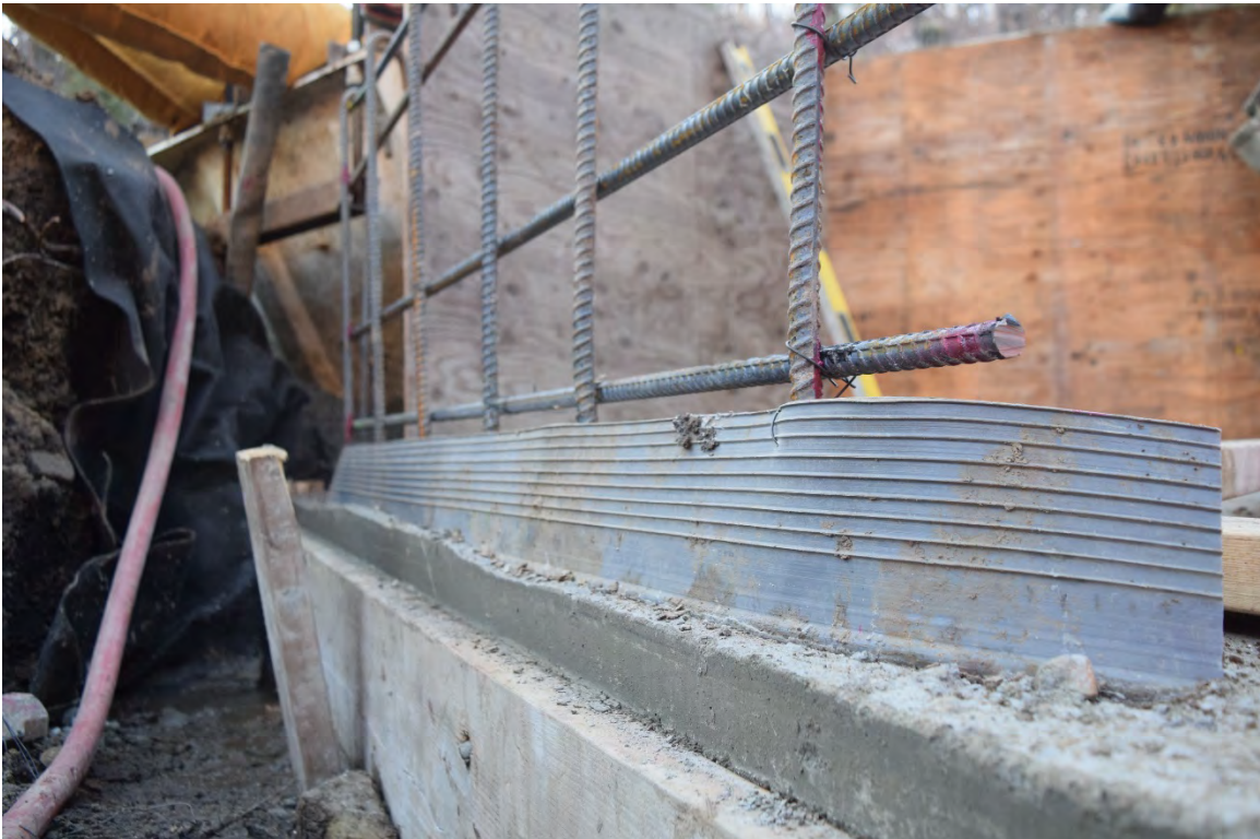
Photo 6: Flexible membrane that seals between the base and wing walls.
