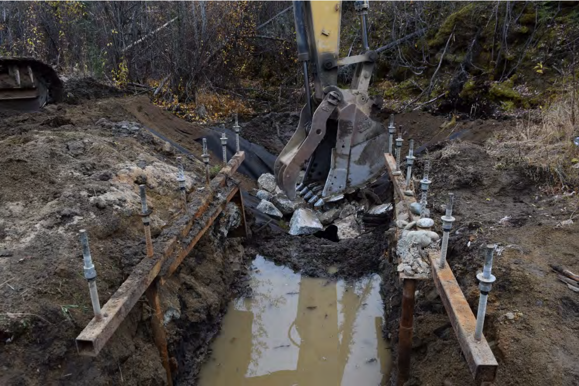
Photo 8: Compaction of backfill to 30mm below final grade.
