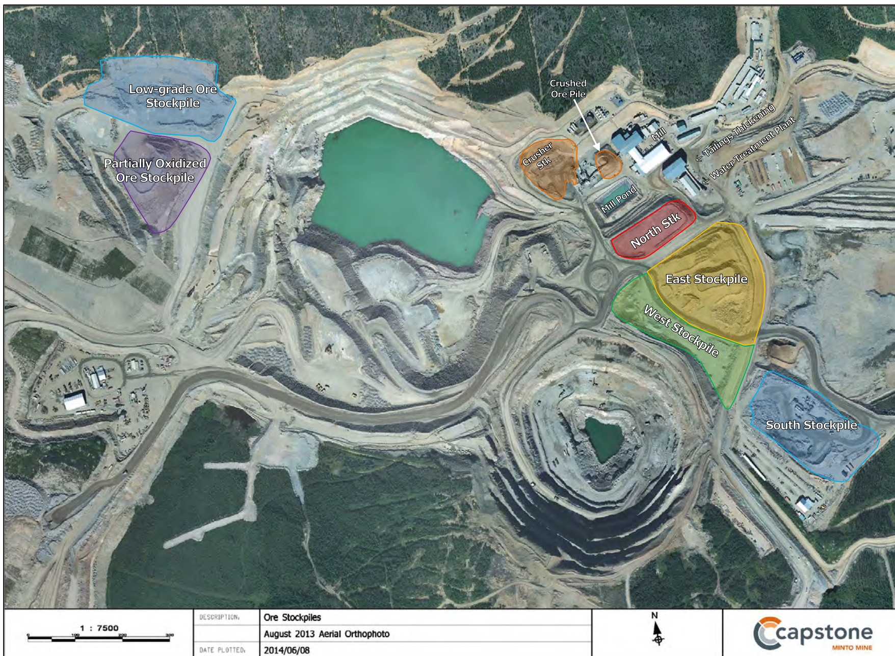
Figure 2-2: Minto Ore Stockpiles (2014)
