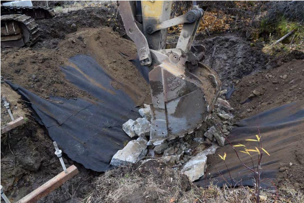
Photo 10: Compacting backfill between steel support structures.
