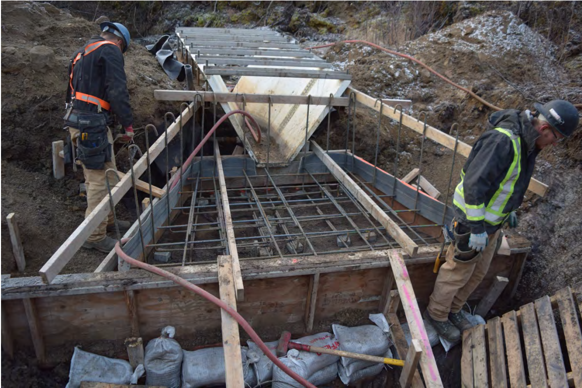
Photo 2: Intake structure base concrete pour.
