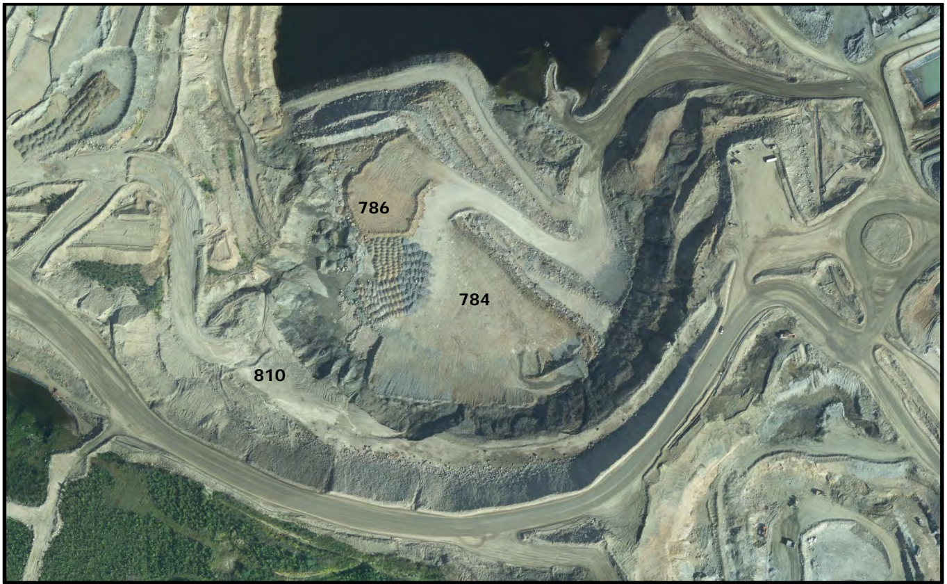
Figure 3-7: Aerial ortho-photo of South Wall Buttress, August 14, 2012.
