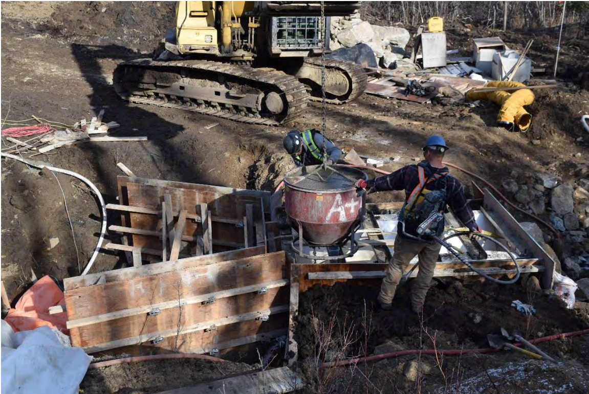
Photo 20: Formwork cross bracing.
