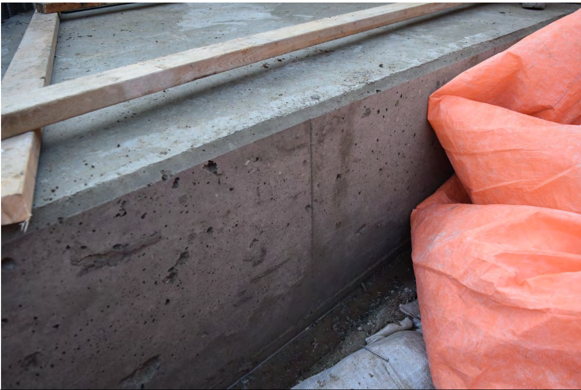
Photo 8: Wing wall form sill plates.
