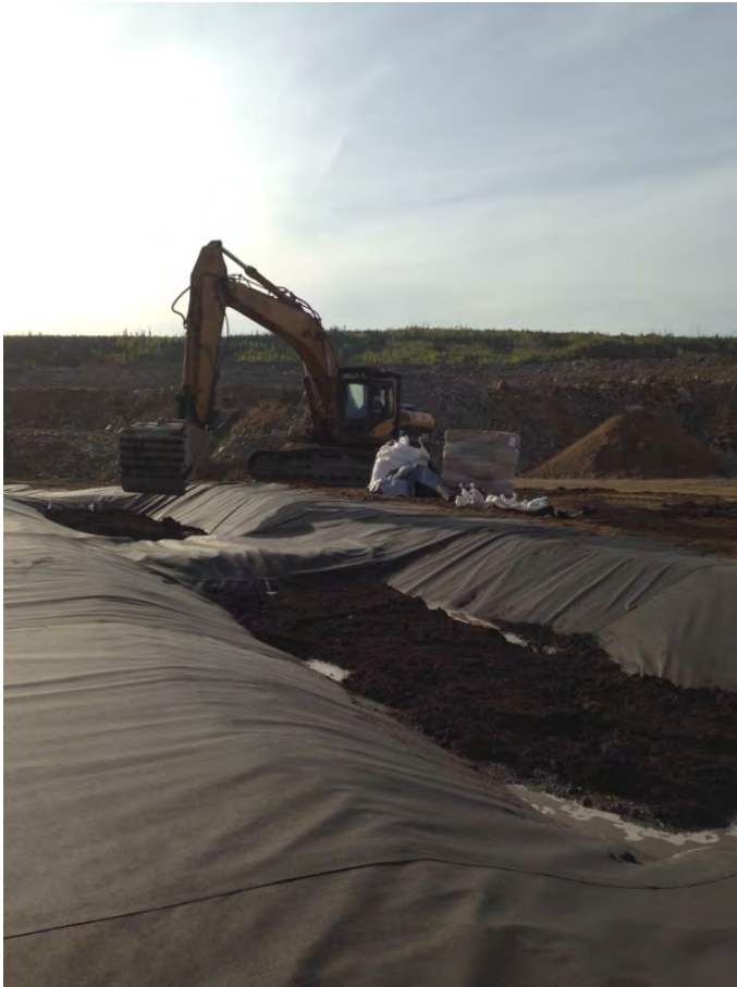
Figure 5. Soil being added to demonstration-scale CWTS cells.
