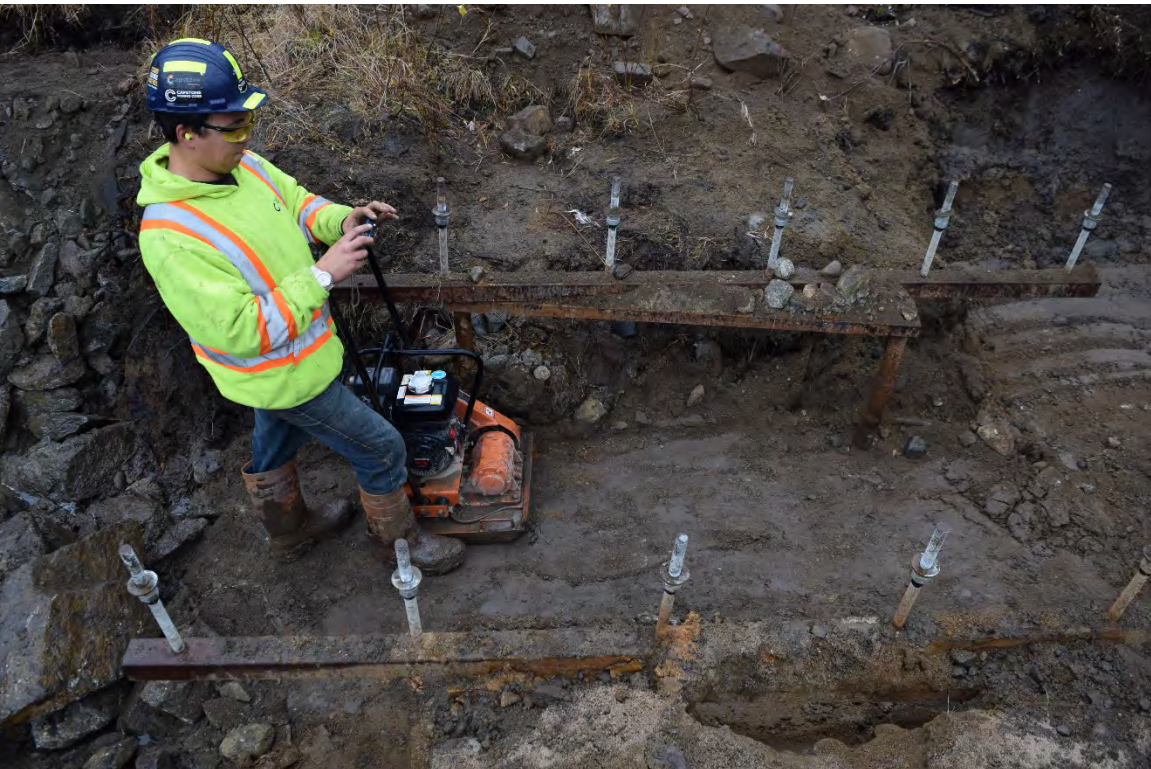
Photo 8: Compaction of backfill to 30mm below final grade.
