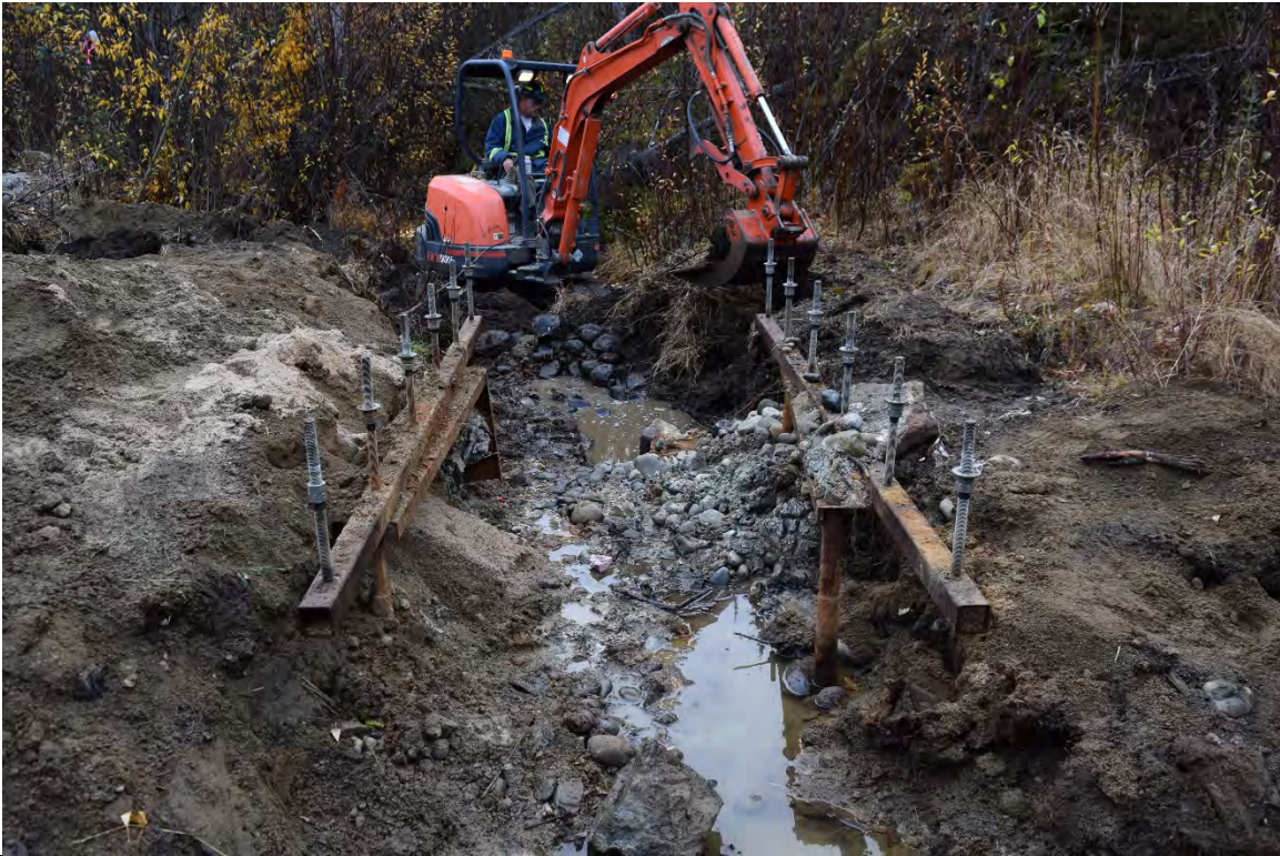
Photo 6: Dewatering seepage in the excavation. (Looking Downstream)
