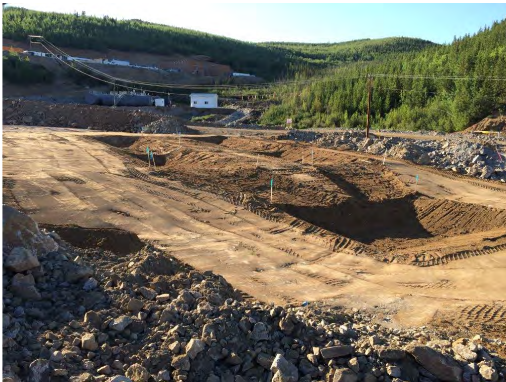
Figure 3. Demonstration-scale CWTS prior to liner installation.
