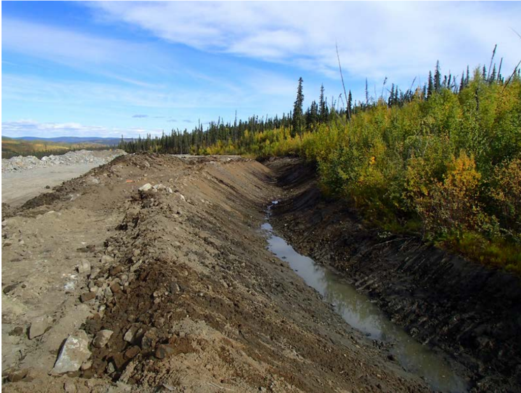
Figure 9: Near Section A Looking East, Sept 4 th , 2014
