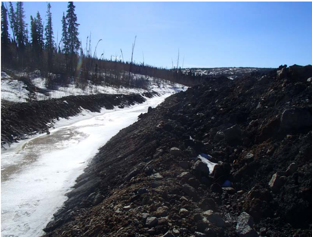
Figure 2: Between Section C and D Looking West, April 19 th , 2014
