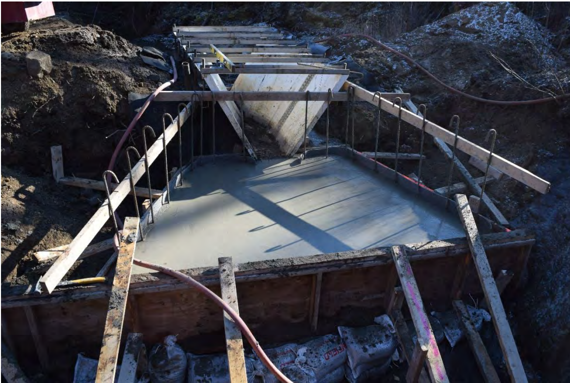
Photo 18: Finished troweled surface on base section.
