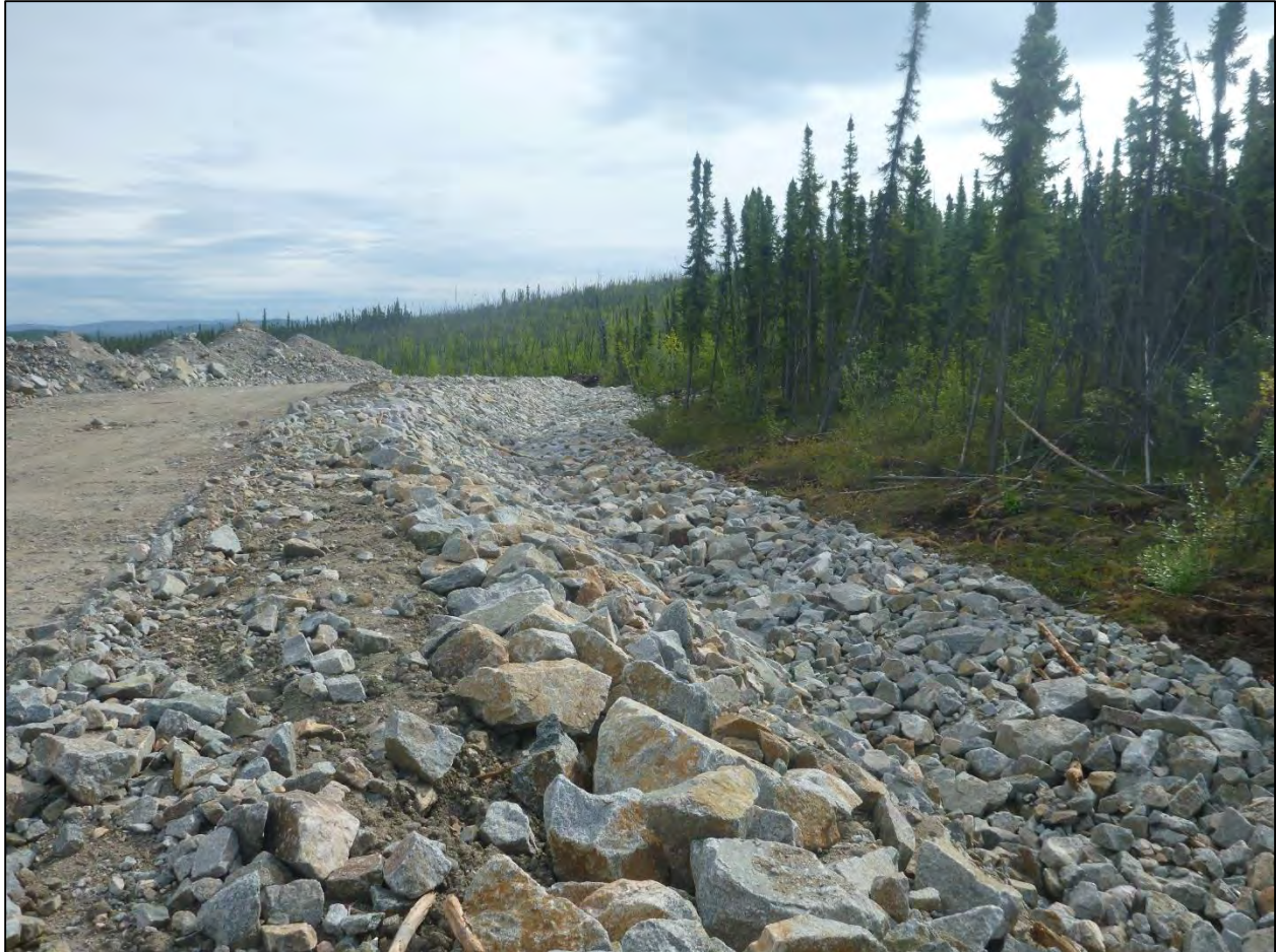
Photograph 7-3: TDD - Completed Section of Ditch Showing Rip Rap Coverage and Grade
