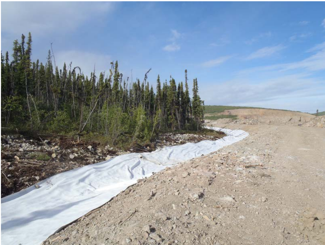
Figure 4: Section E Looking West, June 20 th , 2014
