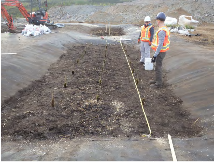
Figure 11. Moss stakes placed in demonstration-scale CWTS cell 2A, looking towards cell 2B.
