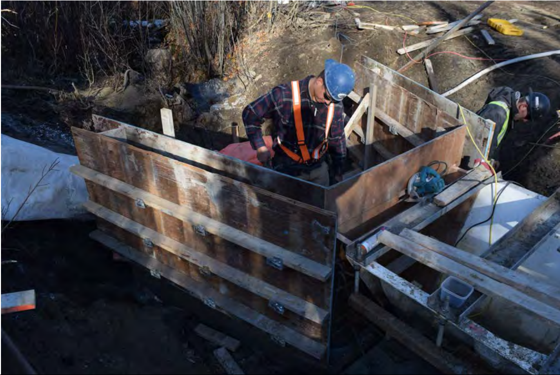
Photo 12: Wing wall cross-bracing
