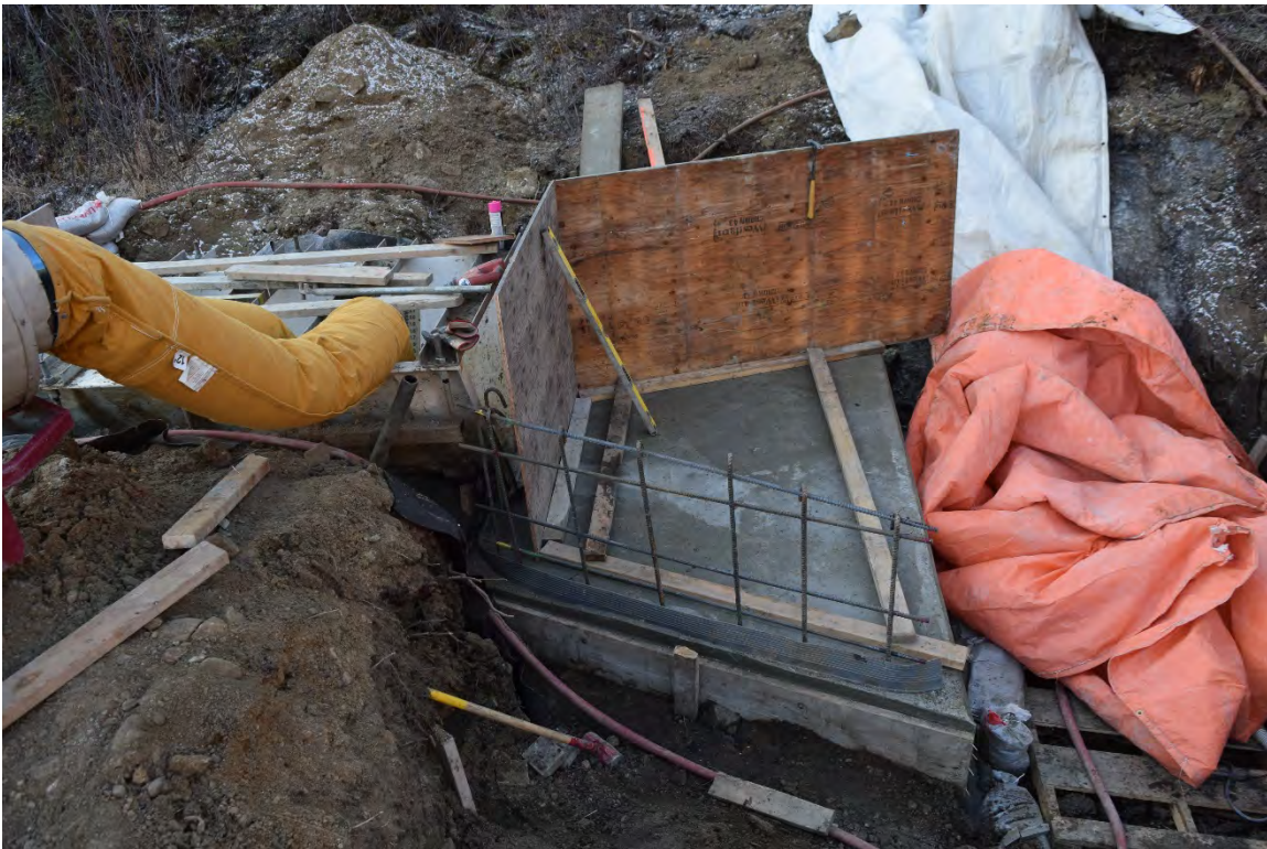
Photo 10: Intermediate wing wall forms before crossing bracing.
