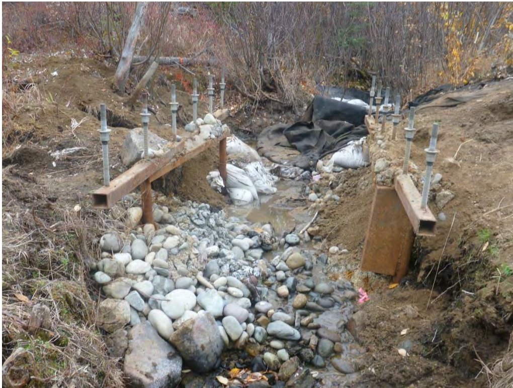
Photo 6: Condition of foundation backfill between steel support structure
