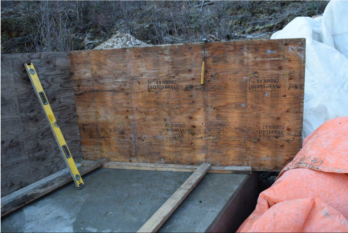
Photo 10: Intermediate wing wall forms before crossing bracing.
