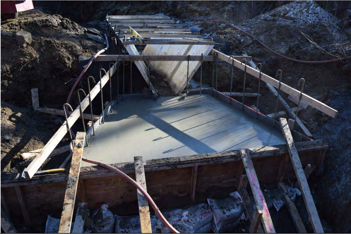
Photo 4: Downstream concrete forms for backfill pour.
