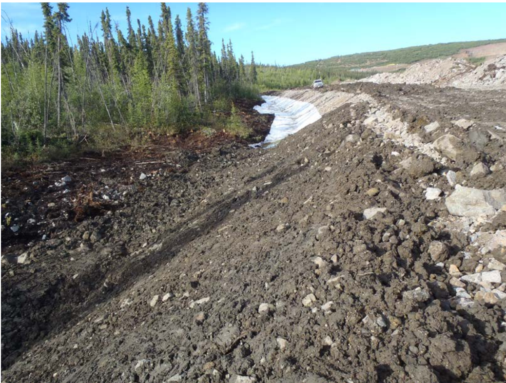
Figure 6: Section D Looking West, June 21 st , 2014
