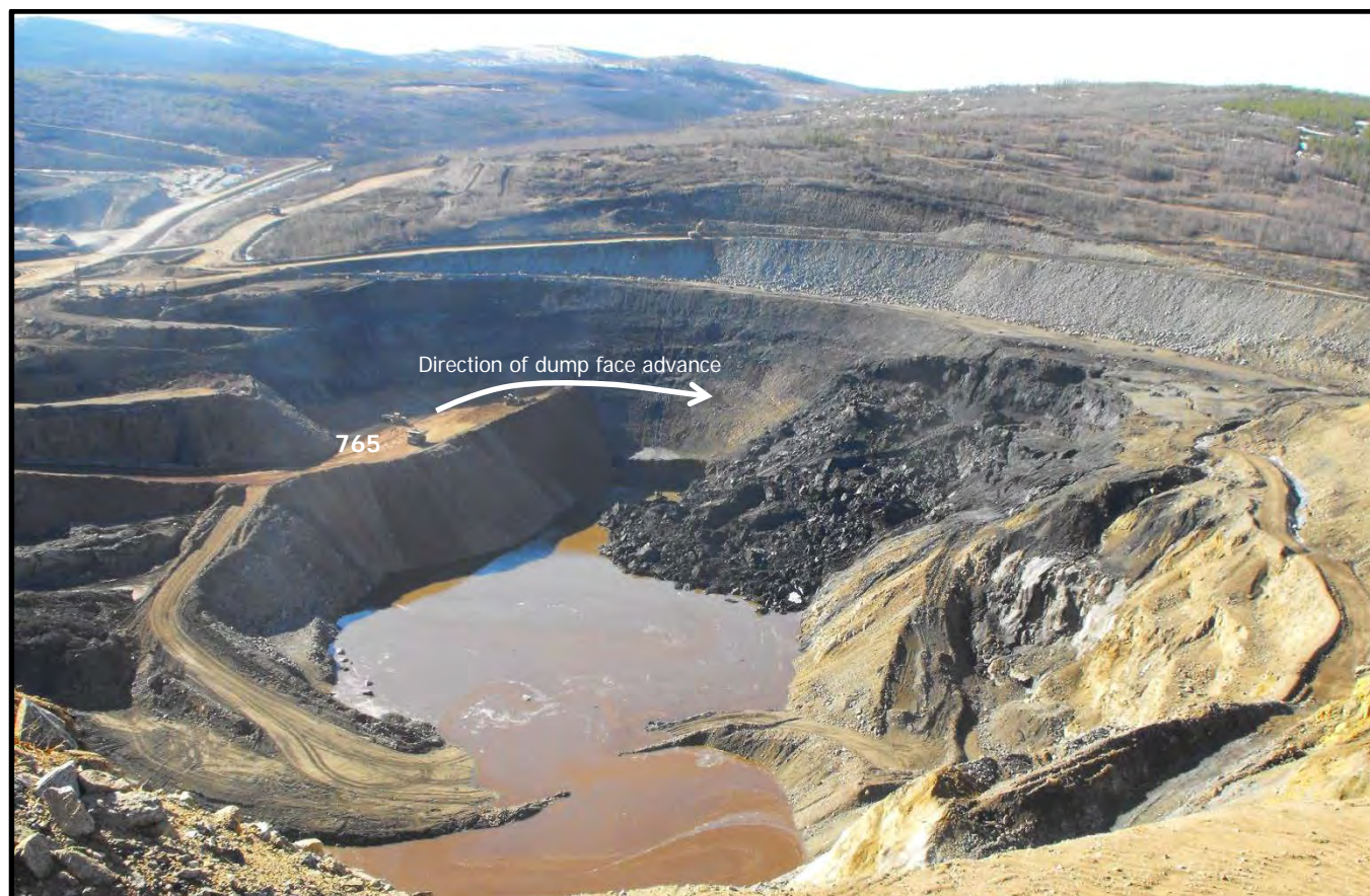
Figure 3-1: Main Pit, looking southeast, June 15. Dumping based on the original wraparound buttress design is shown.
