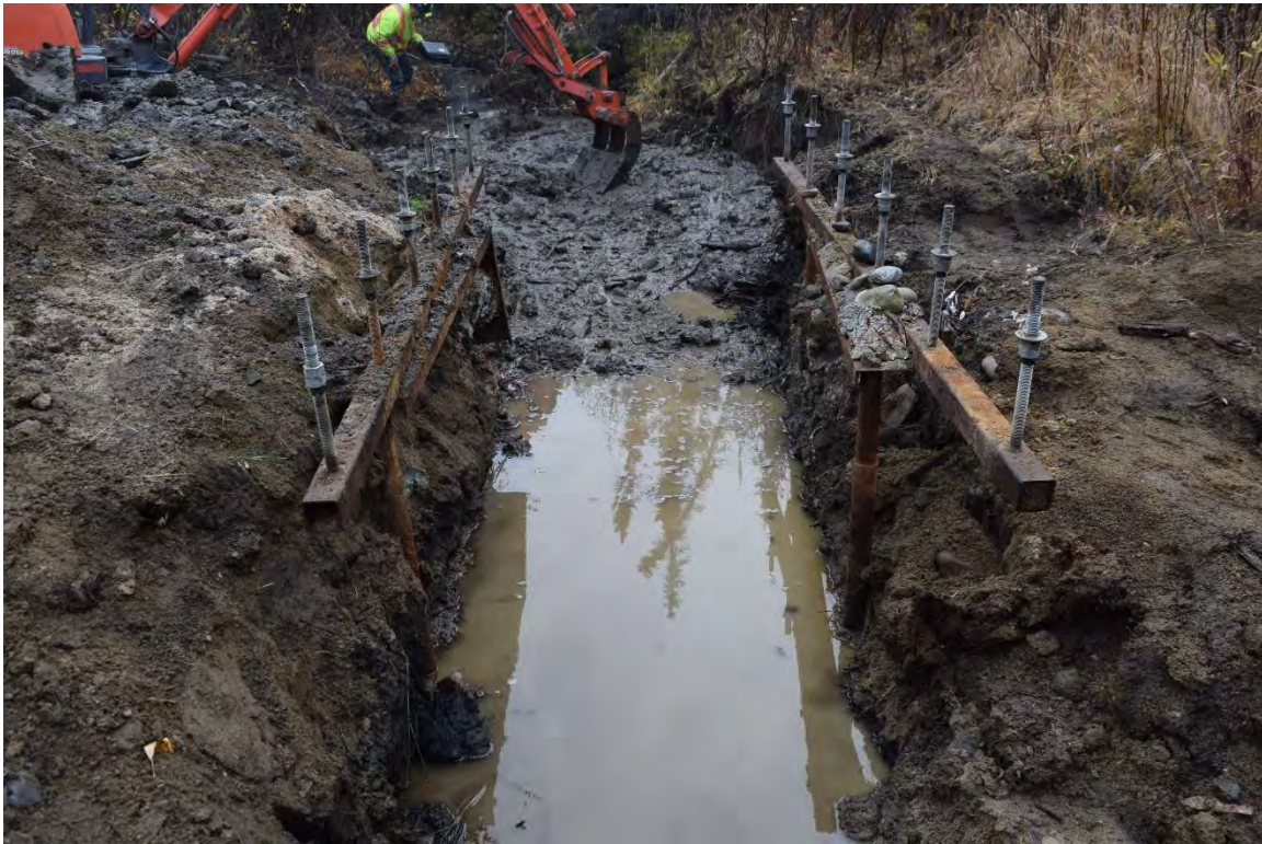
Photo 8: Flume support structure after excavation
