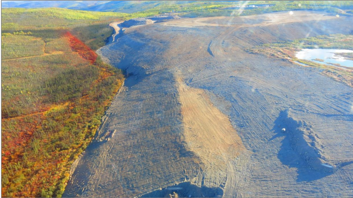
Photograph 6-1: Sloping of the Medium Grade Waste Area
