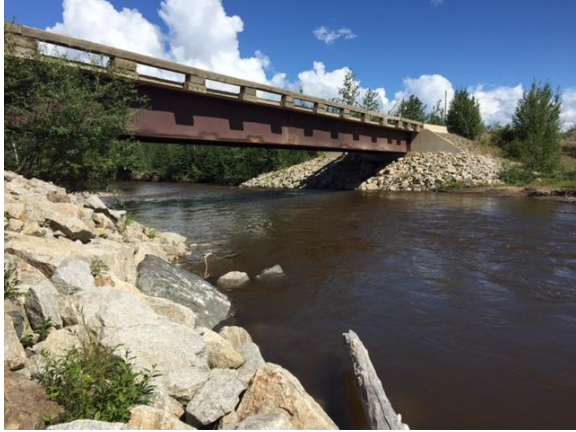
Photo 5: Big Creek Bridge (July)
