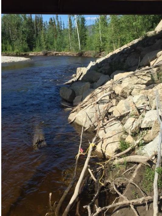
Photo 1: Big Creek looking downstream (June)
