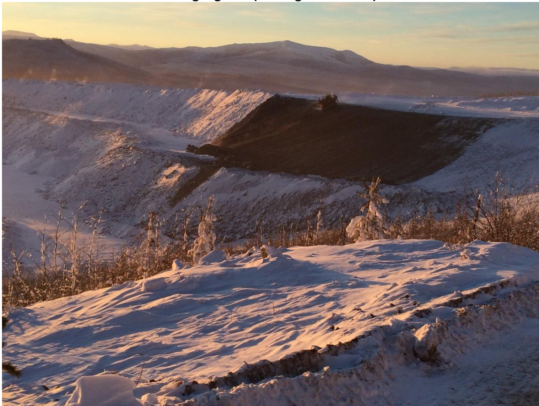
Figure 16-4: Main Waste Dump Expansion (looking west) top bench being recontoured in 2016.
