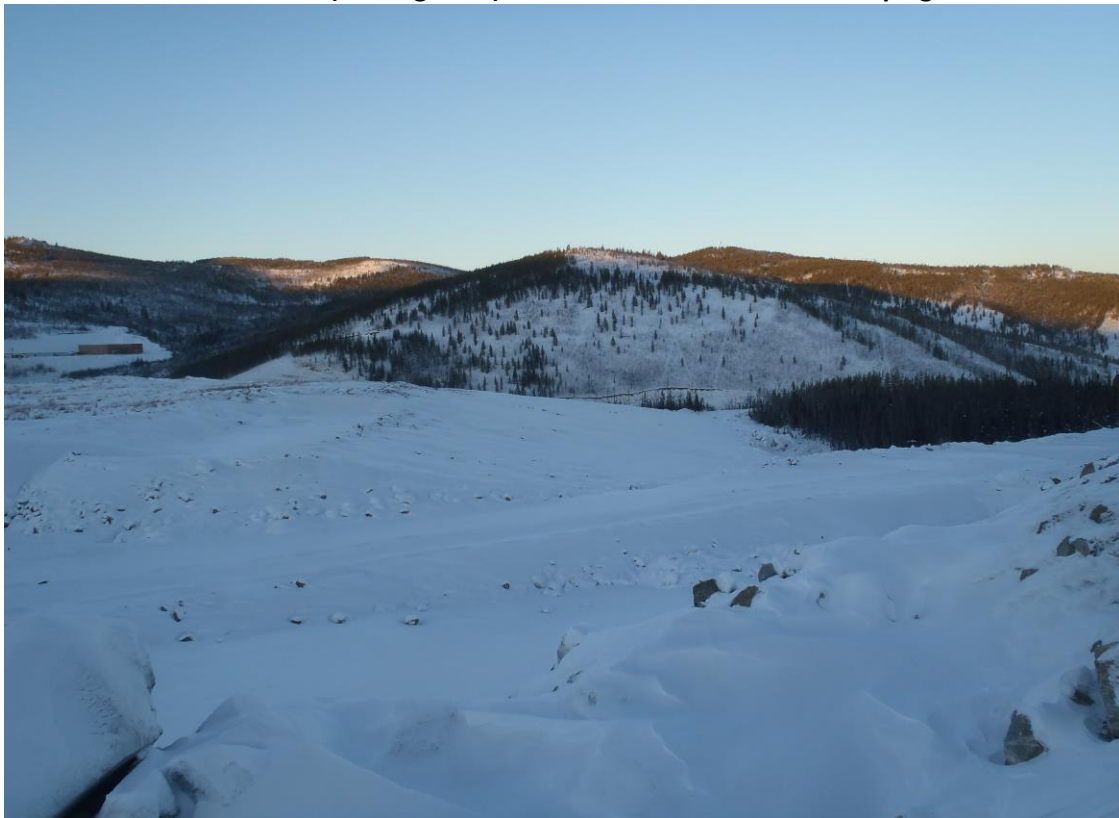
Figure 16-2: DSTSF east slope (looking north) recontoured at a maximum slope grade of 4:1.
