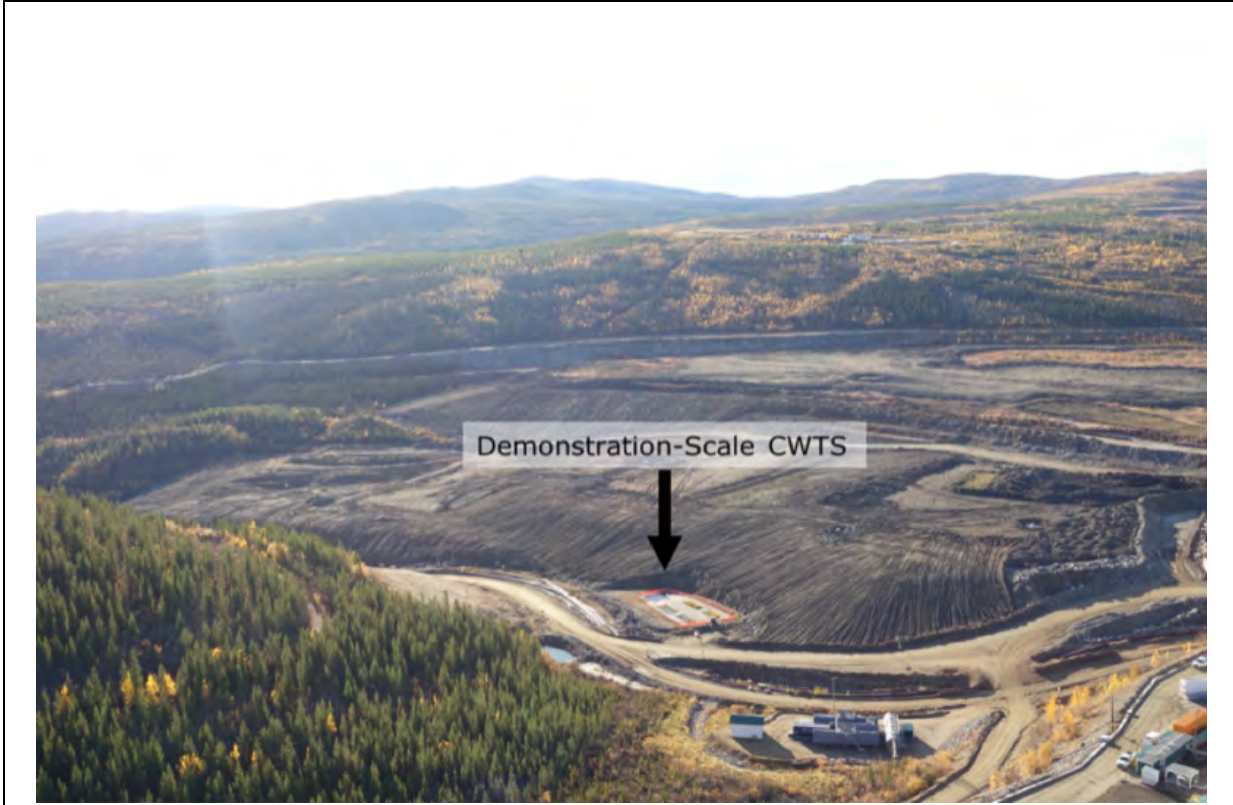
Figure 1 – Picture of demonstration-scale CWTS at Minto Mine. Demonstration-scale CWTS location in relation to its surroundings. To the far right is the mine camp while below is the tree line. This photo was taken on September 24, 2017.
