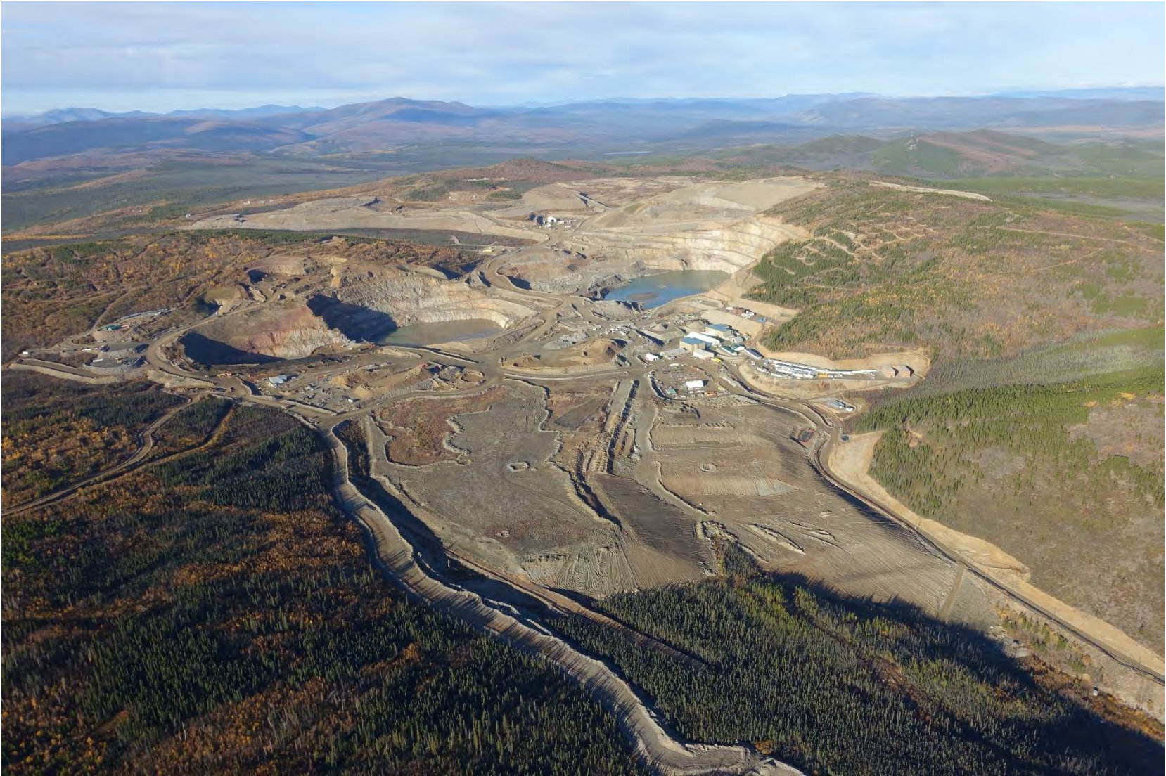
Figure 16-6: Minto Mine – Site overview, all facilities.
