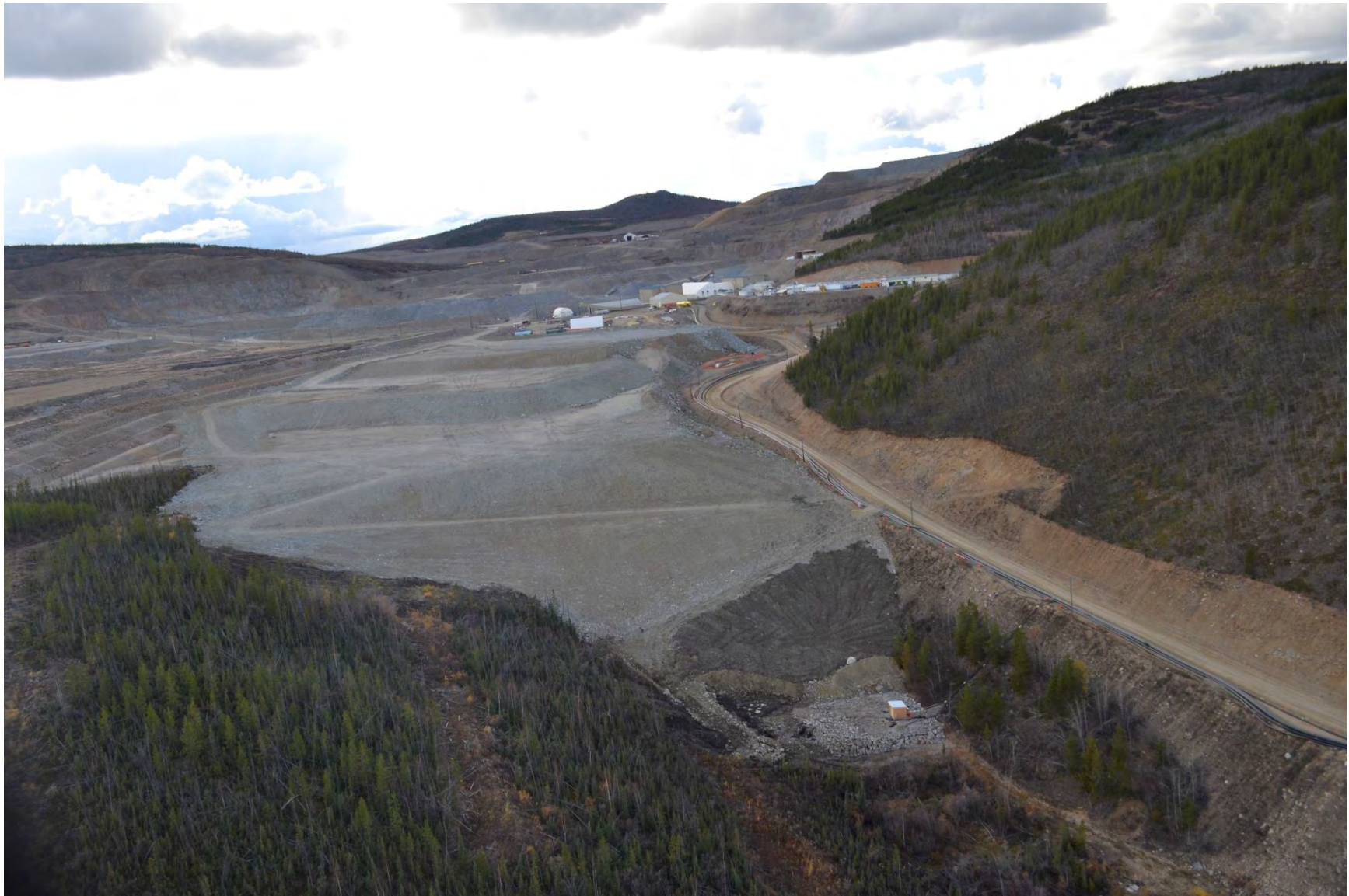
Figure 16-1: Minto Mine – Mill Valley Fill Extension Stage 2 completed in 2016.
