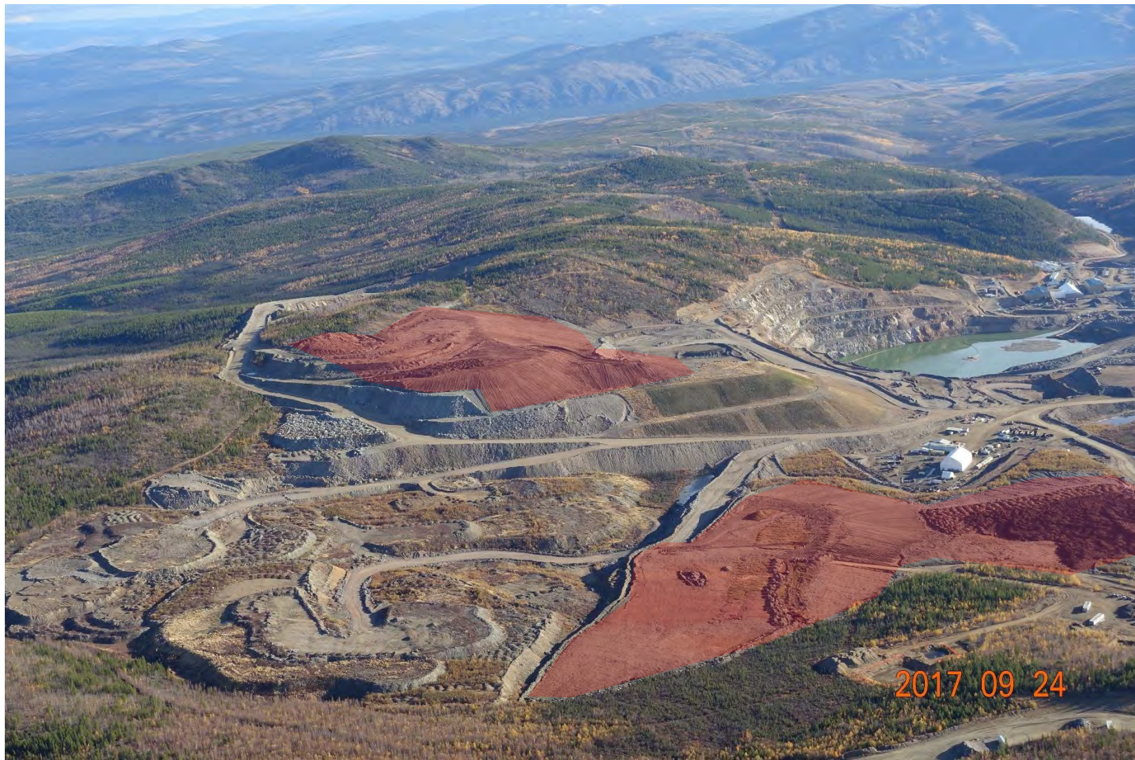
Figure 16-5: Minto Mine – MWDE and Low Grade Waste progressive reclamation, overburden cover placement (highlighted in red).
