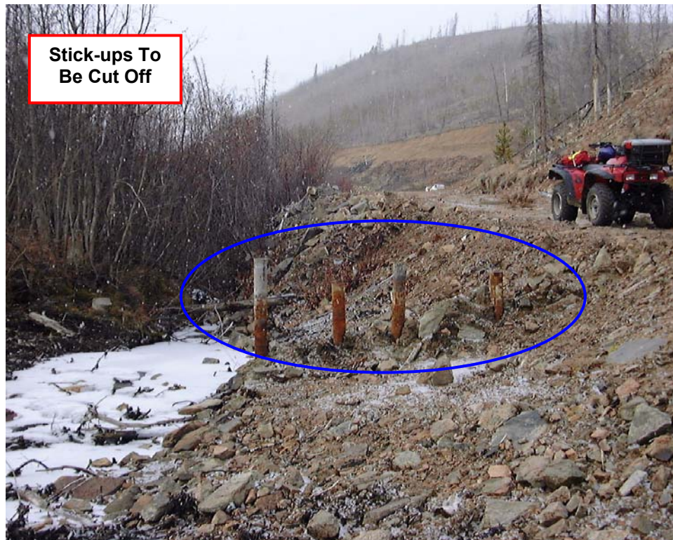
Plate 5 Grout Curtain Injection Pipes (Looking West - Upstream)
