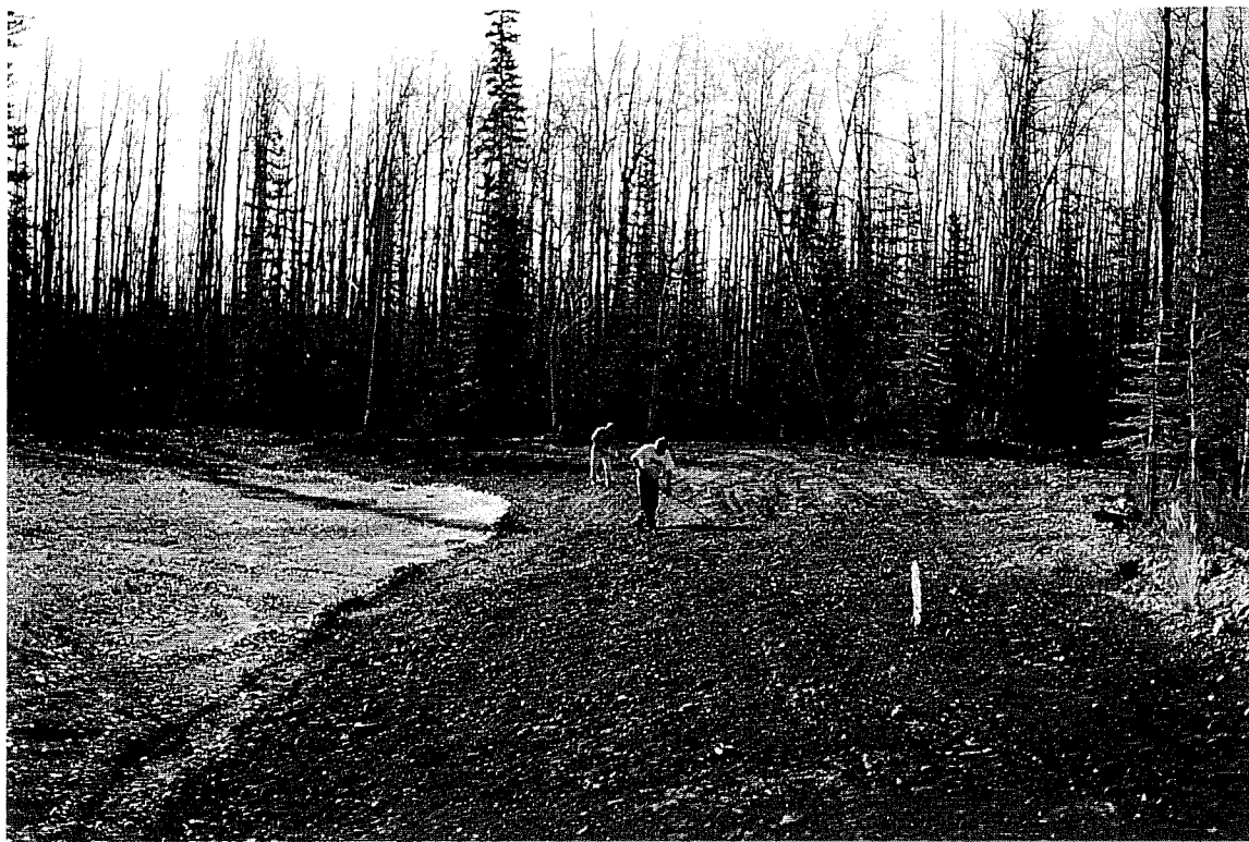
Photograph #4 - Selkirk First Nation workers raking planted ditch slopes - 09/May/2000
