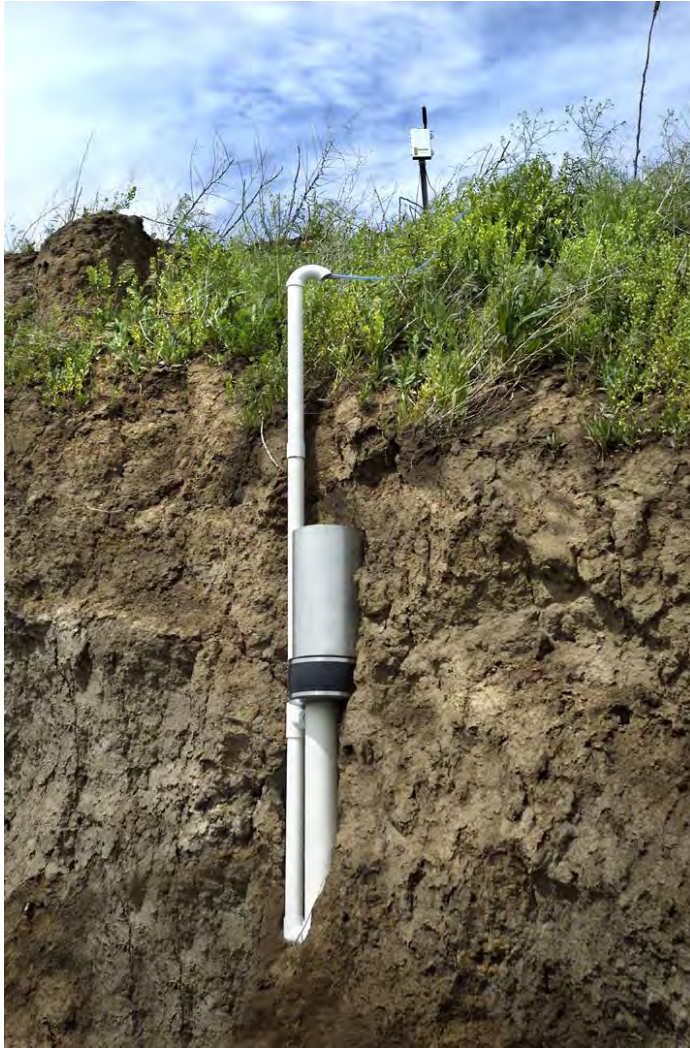
Figure 6: Typical Installation of Passive Lysimeter
