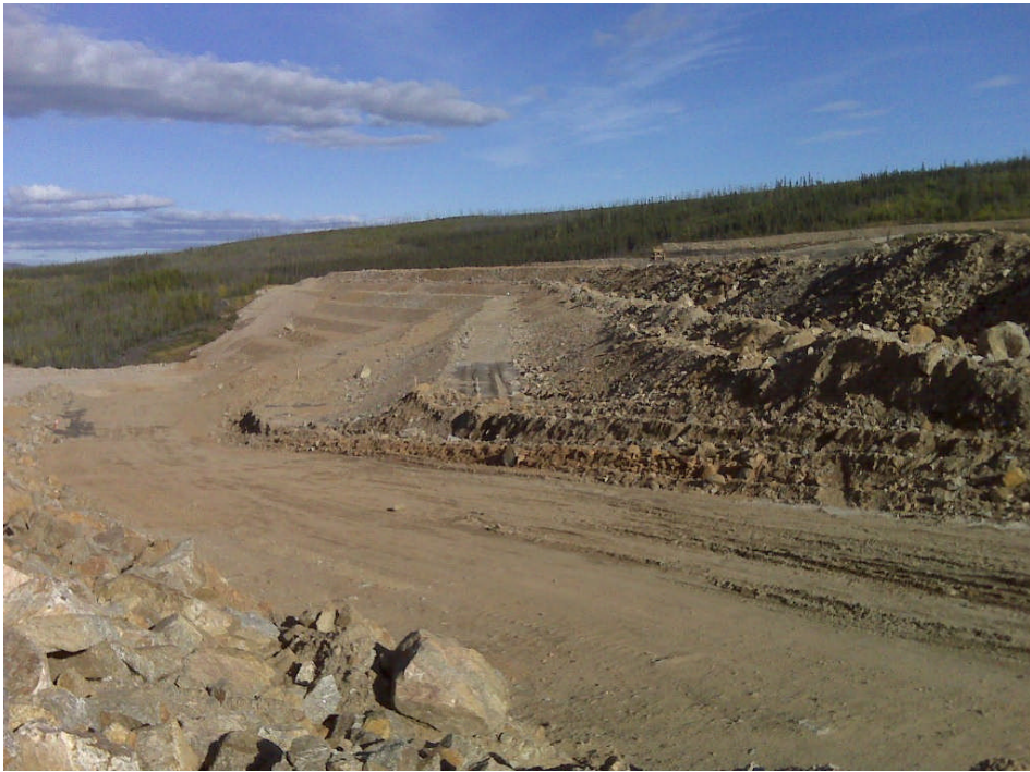
Photo 3 DSTS Front Face, Aspect: East (August 25, 2011)
