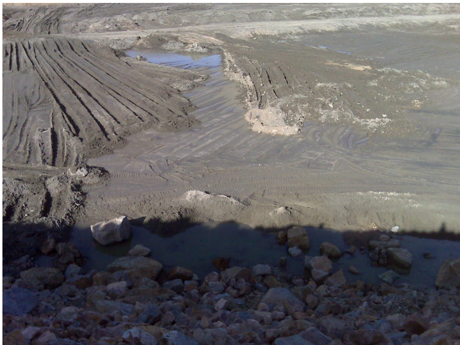
Photo 4 Typical placement and compaction activities (August 25, 2011)
