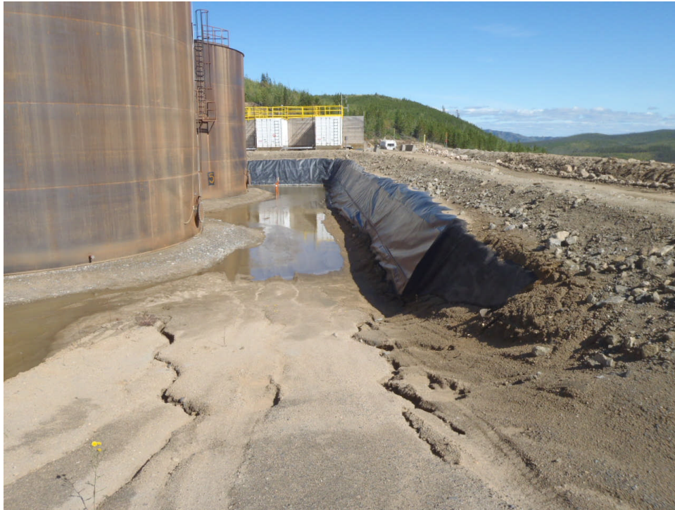
Photo 1 South portion of FCF. (August 25, 2011)
