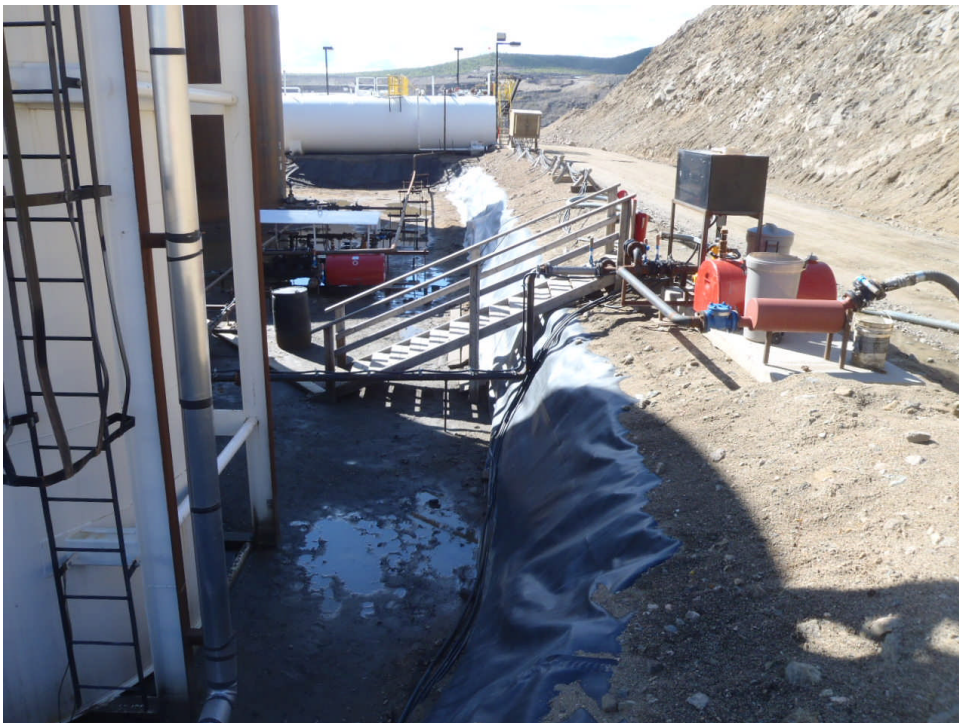
Photo 2 North portion of FCF. (August 25, 2011)
