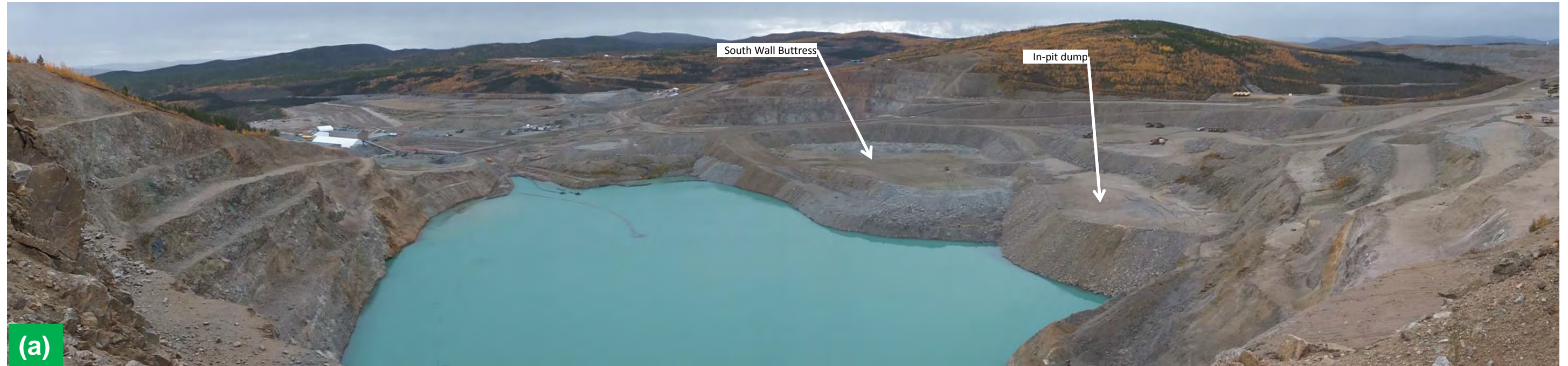
Photo a: View of the Main Pit, South Wall Buttress and In-Pit Dump taken from the north west corner of the pit. Photos b and c: View of the tension cracks on the In-Pit Dump located west of the South Wall Buttress. This area has been blocked off and is inaccessible to equipment. Cracks on the In-Pit Dump are up to 50 cm wide with a 40 cm elevation difference across the crack. The movement is believed to be due to the large dump height, with the material end dumped directly into the pit water.
