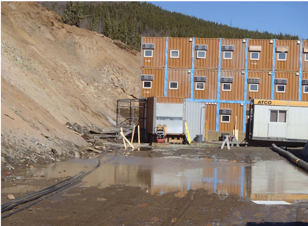
Figure 4: Mine Camp - The low spot behind the new camp should be graded using gravel to continue the drainage channel behind the back of the new camp, as opposed to the ponding which currently occurs.
