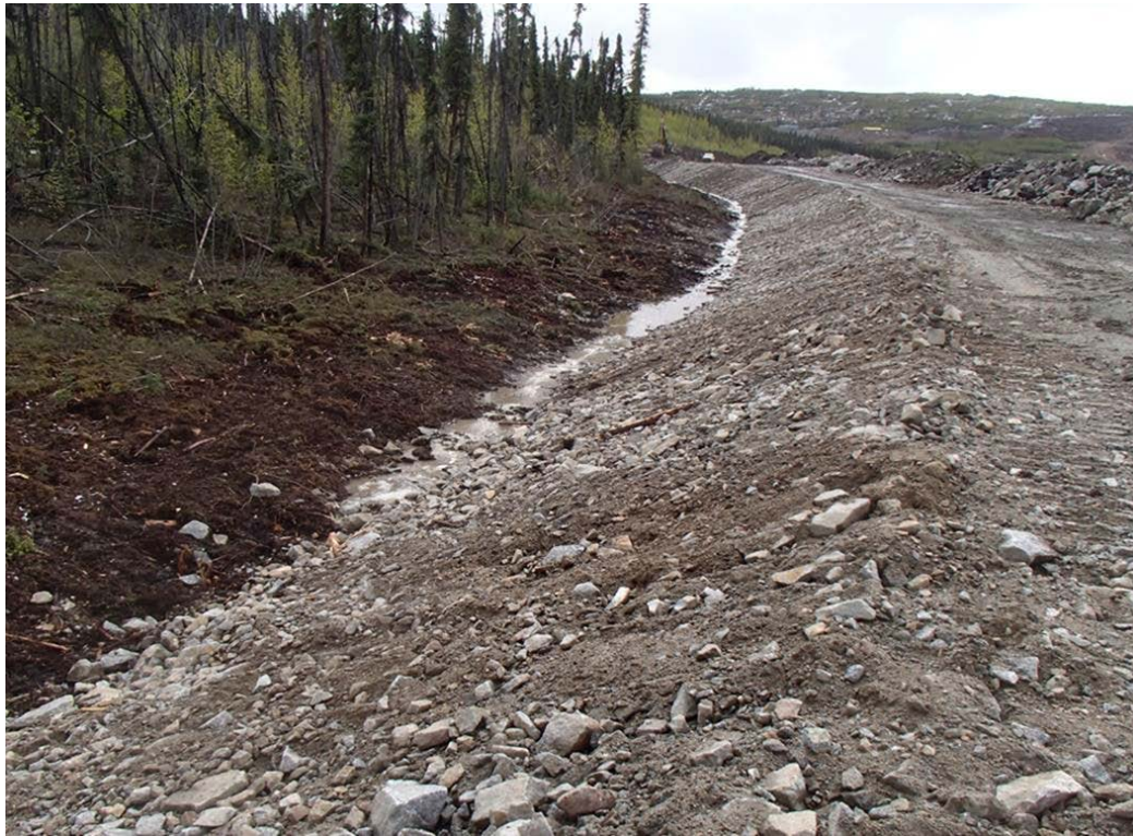
Figure 1: Tailings Diversion Ditch – Construction was observed at the Tailings Diversion Ditch
