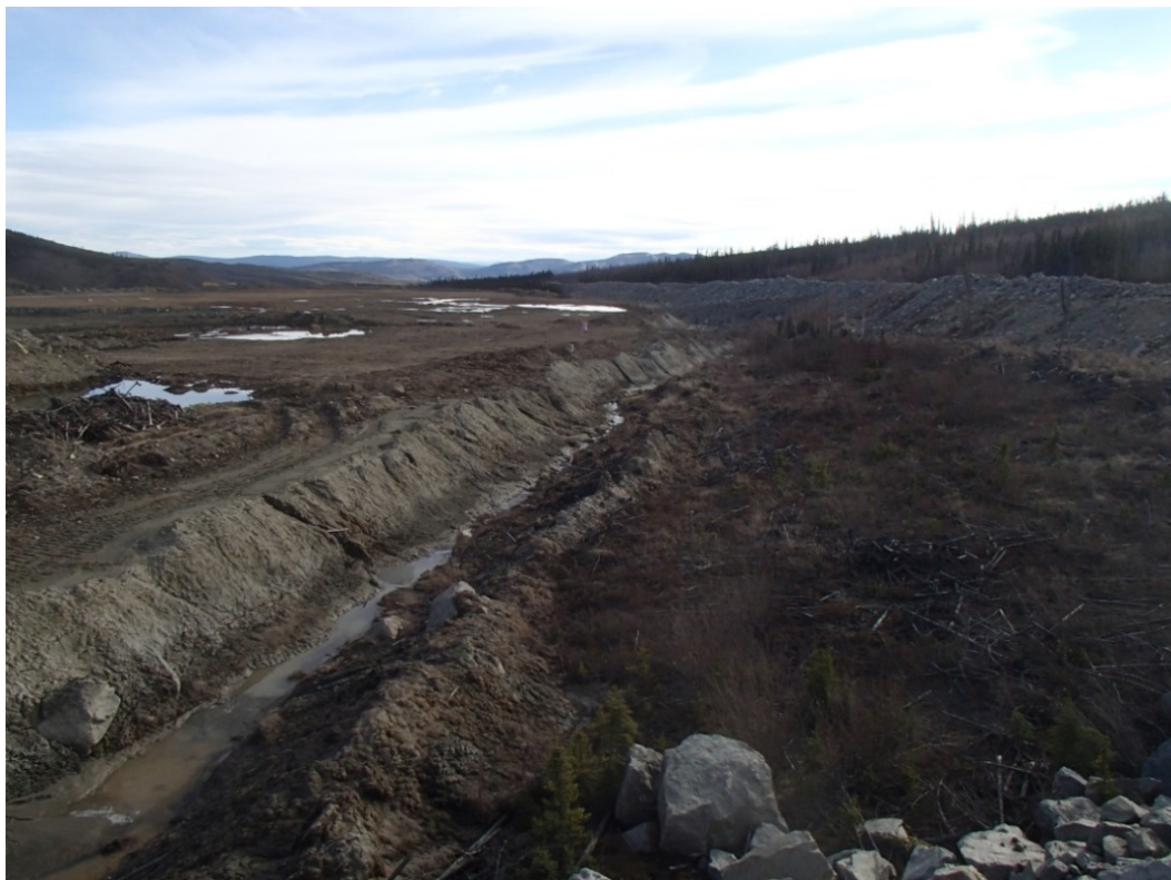
Figure 2: Dry Stack Tailings Storage Facility - South side of DSTSF.
