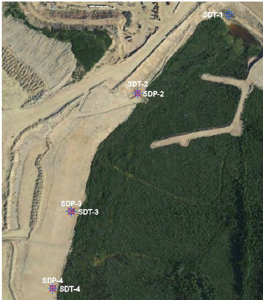
Southwest Dump Piezometers and Ground Temperature Cables
