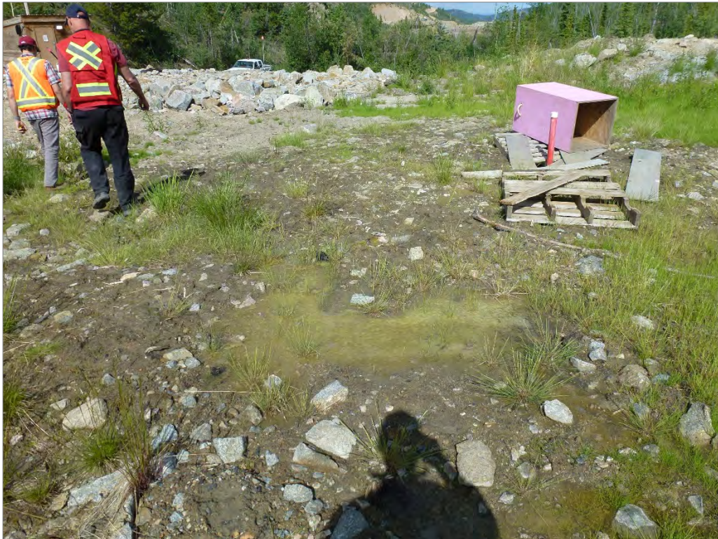
Photo 22: Potential seepage at the toe of the MVFE (but still upstream of seepage collection system)
