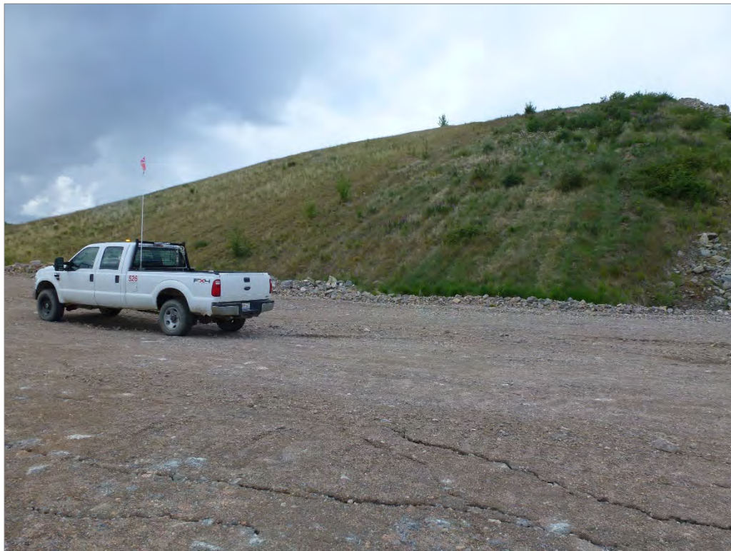
Photo 33: Cracking on the crest of MWD Wrap and vegetated slope of MWD (looking north)
