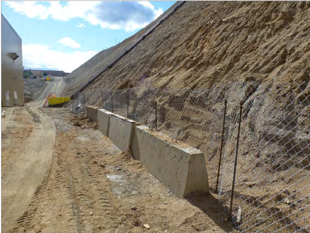
Photo 49: Newly installed concrete jersey barriers. Note over-excavated highwall toe.
