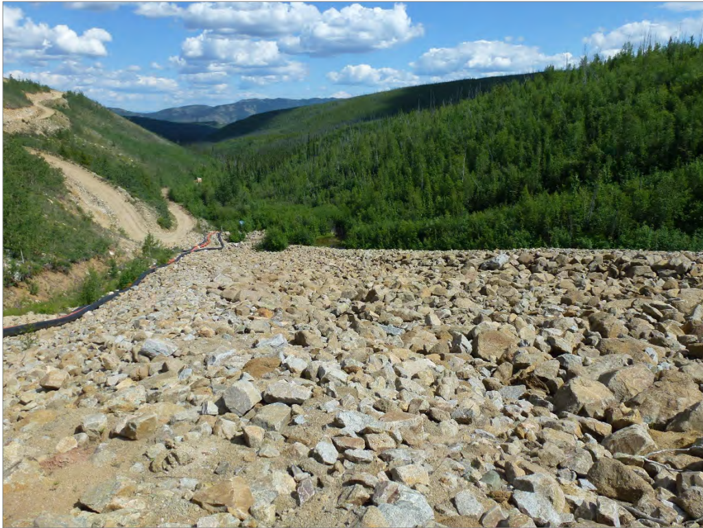
Photo 71: WSP Dam downstream slope (looking east)
