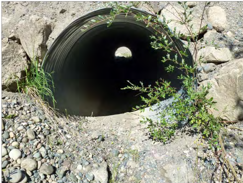
Photo 81: Single road culvert
