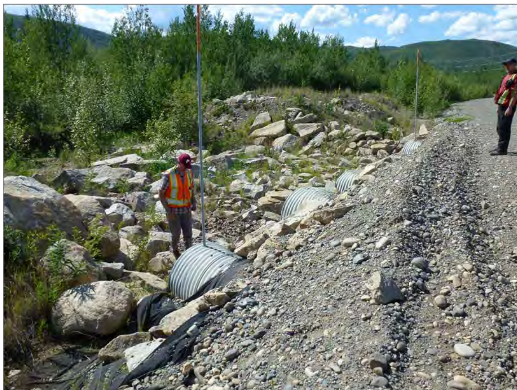
Photo 82: Four road culverts
