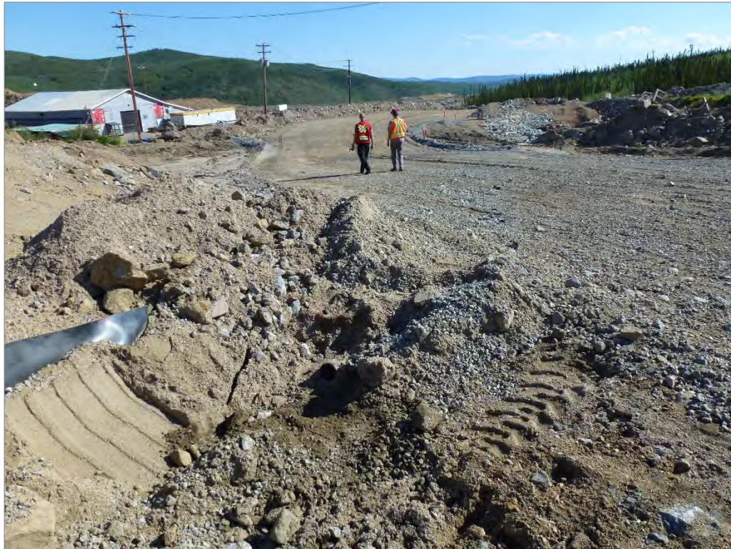
Photo 107: Looking downstream towards Underground Maintenance Shop. Note culvert underneath haul road.
