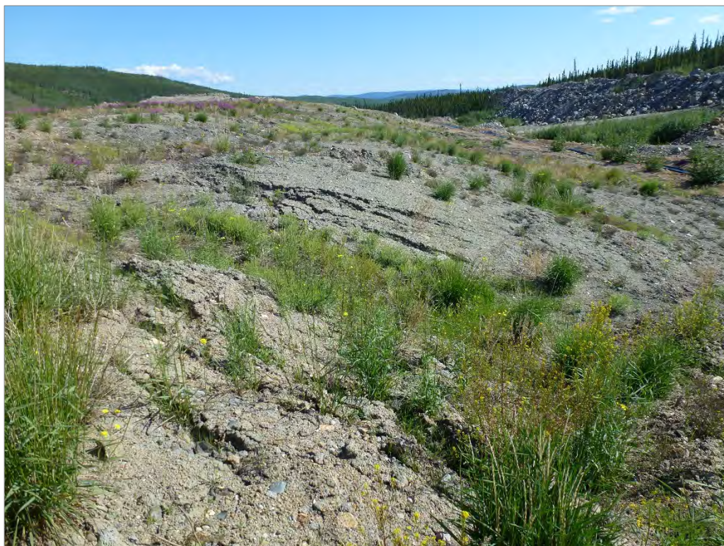
Photo 4: Observed slump and cracking at the crest (looking east)
