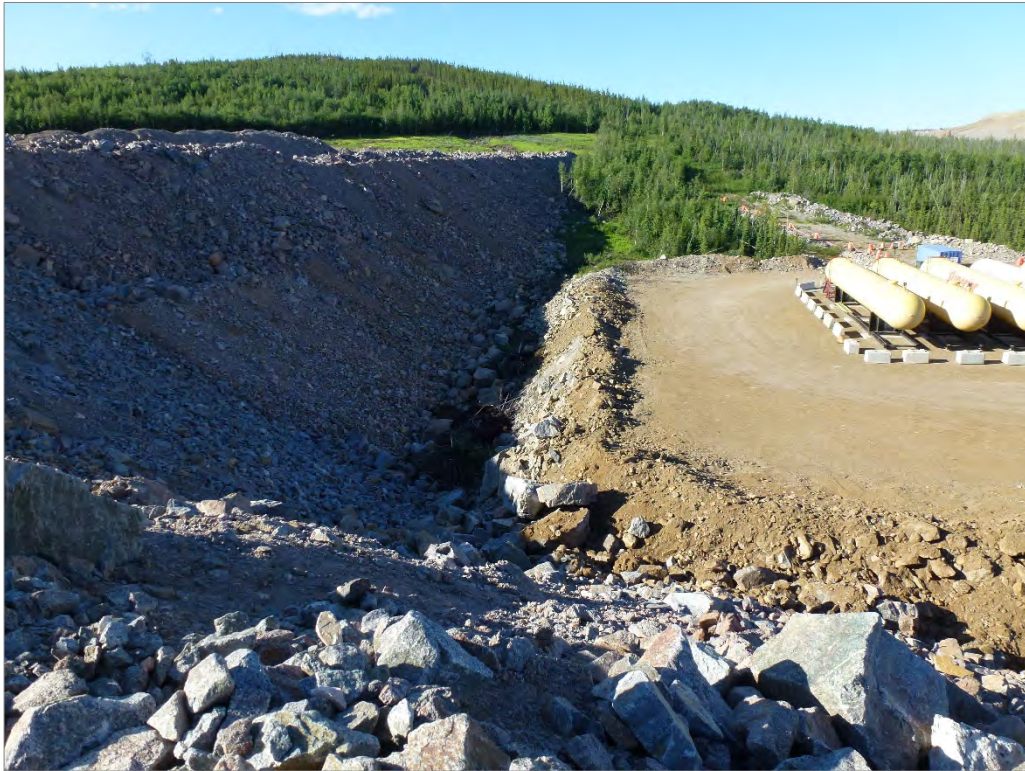
Photo 92: Expanded area of MPD (looking south)
