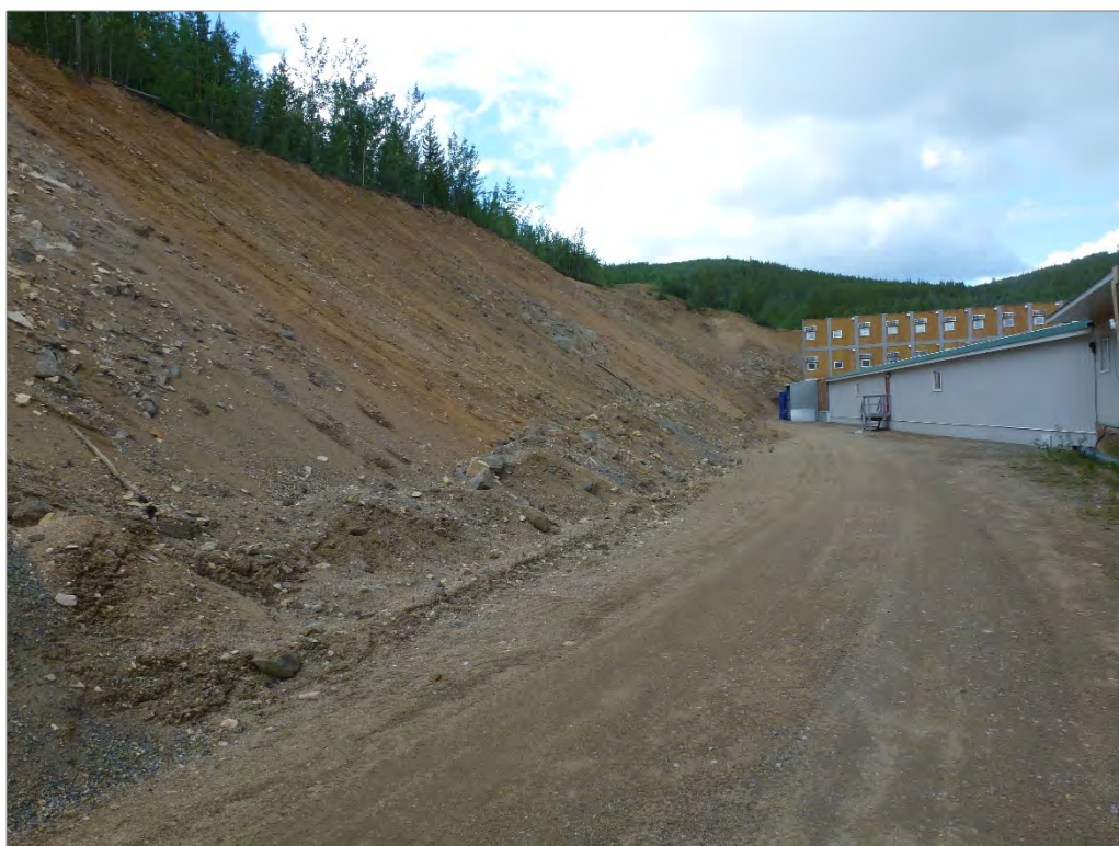
Photo 54: Highwall behind Camp Site (looking north)
