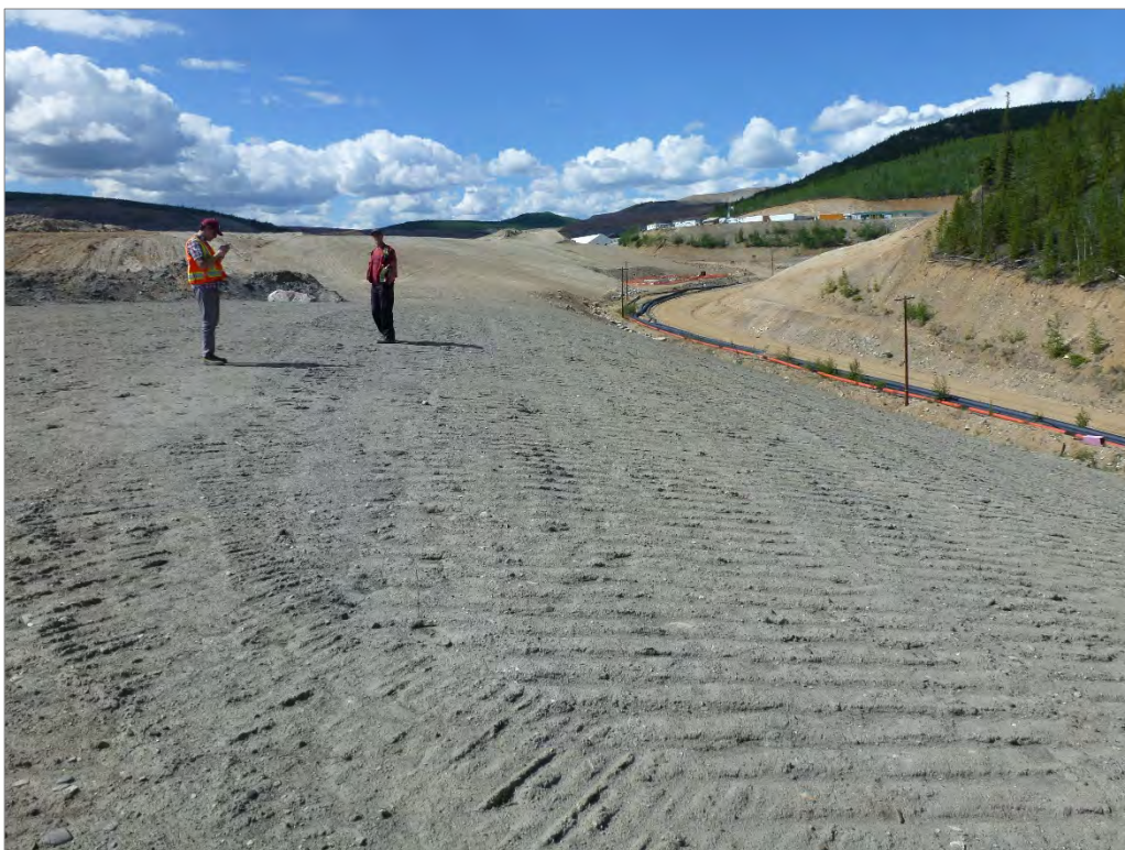
Photo 16: Looking across final surface of Tier C (looking west)
