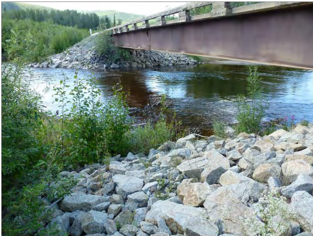
Photo 77: Side view of Big Creek Bridge (looking west)
