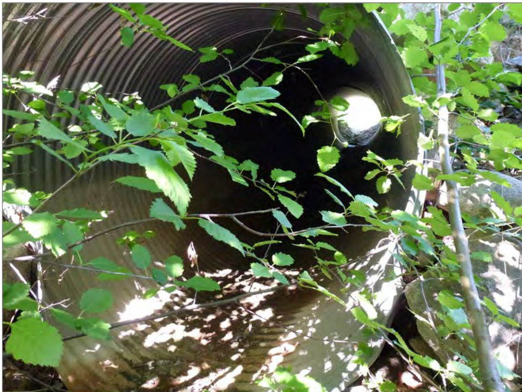
Photo 80: Single road culvert
