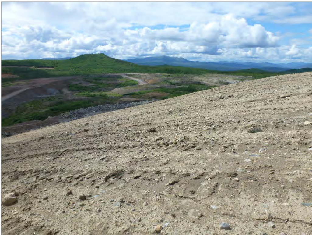
Photo 28: MWD regraded slope – looking south towards Reclamation Overburden Dump
