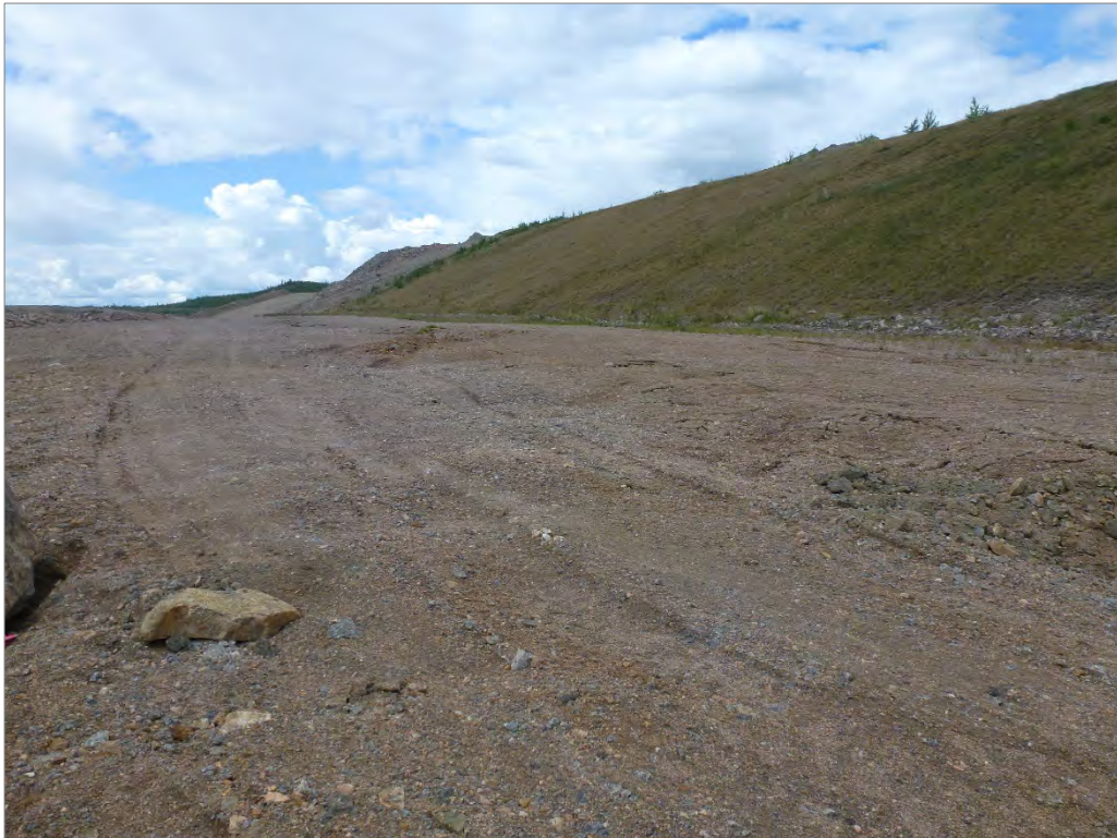
Photo 36: Additional areas of differential settlement and small sinkholes (looking west)
