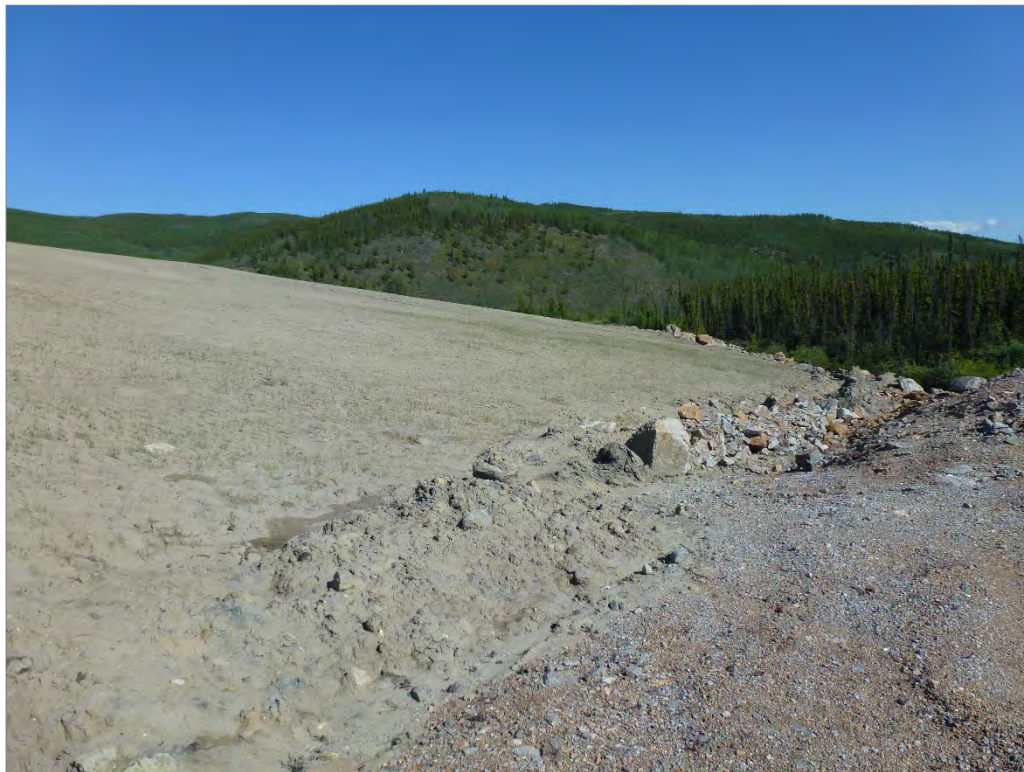
Photo 3: Covered and regraded slope of DSTSF at eastern corner
