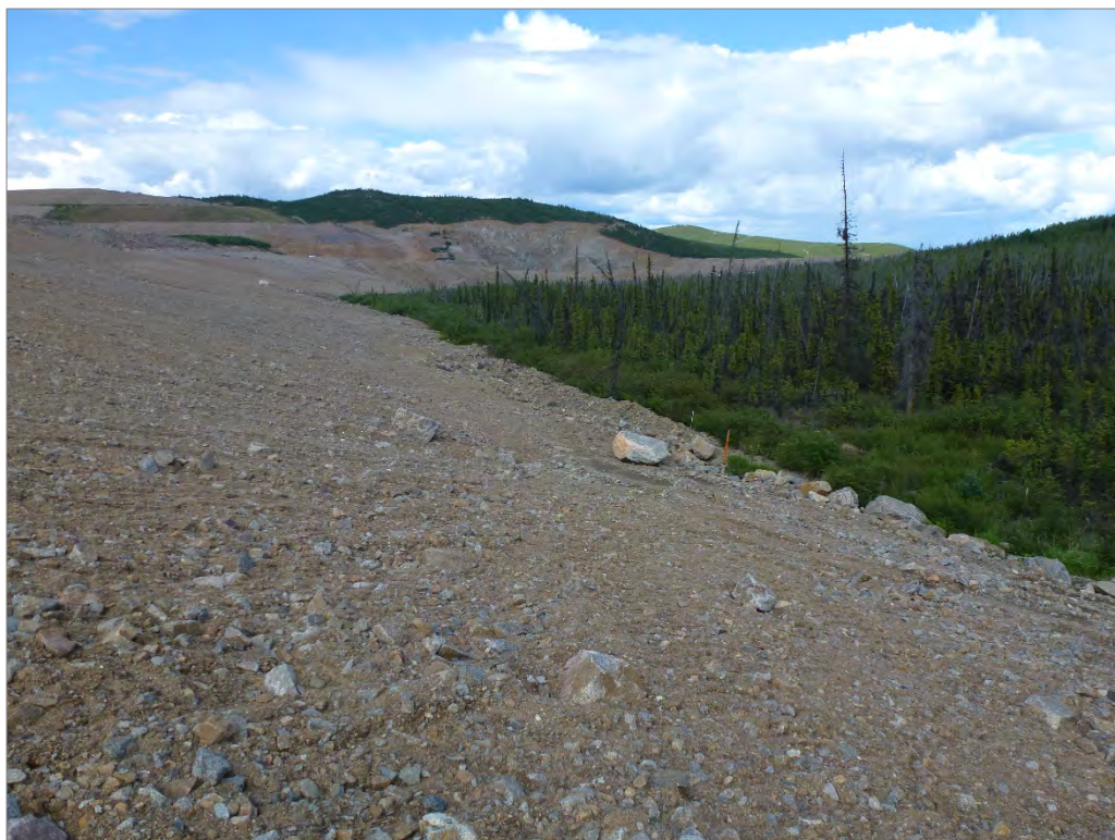
Photo 42: Regraded slopes of the SWD (looking north)
