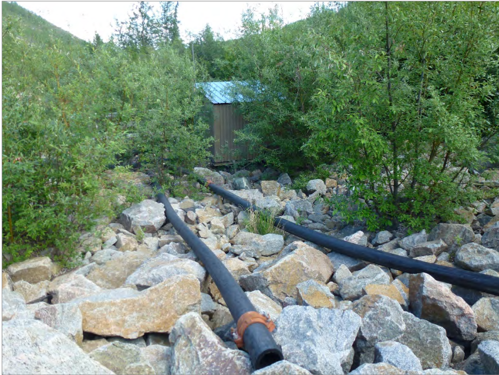
Photo 75: Looking downstream towards the seepage collection system
