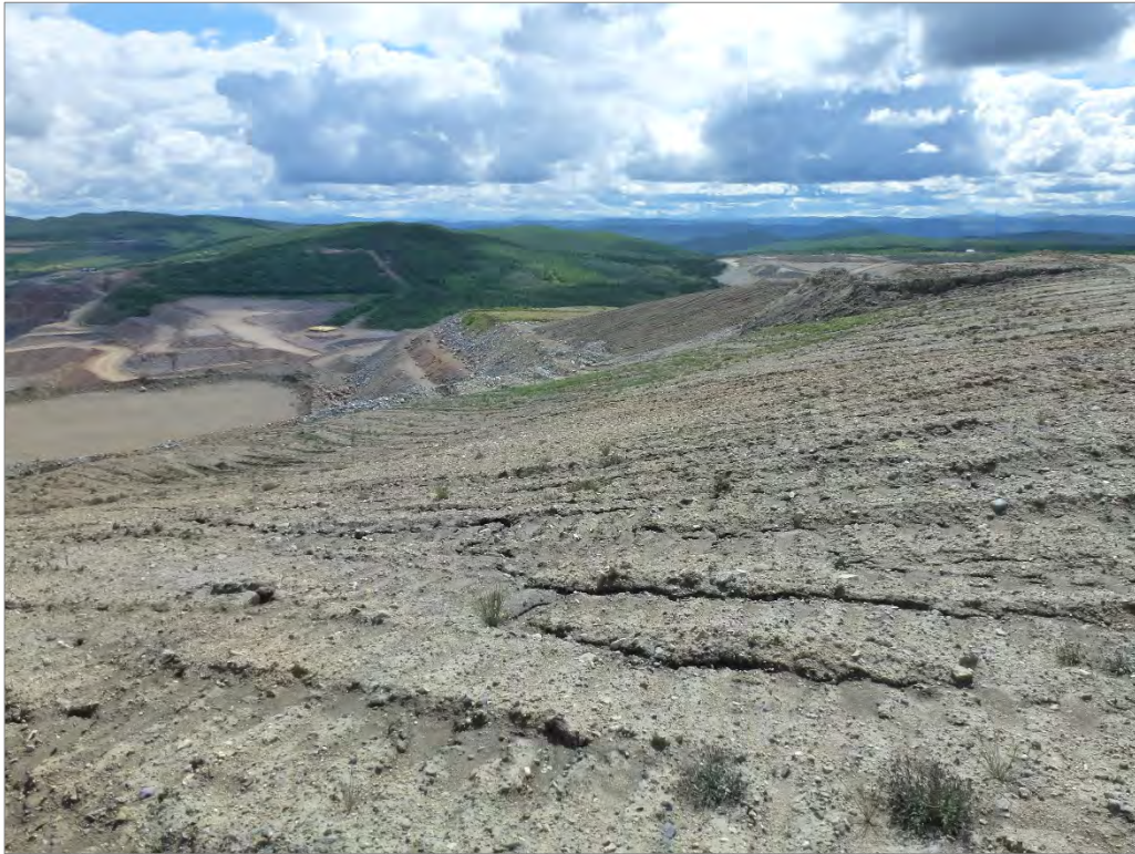
Photo 27: MWD regraded slope (looking southeast)
