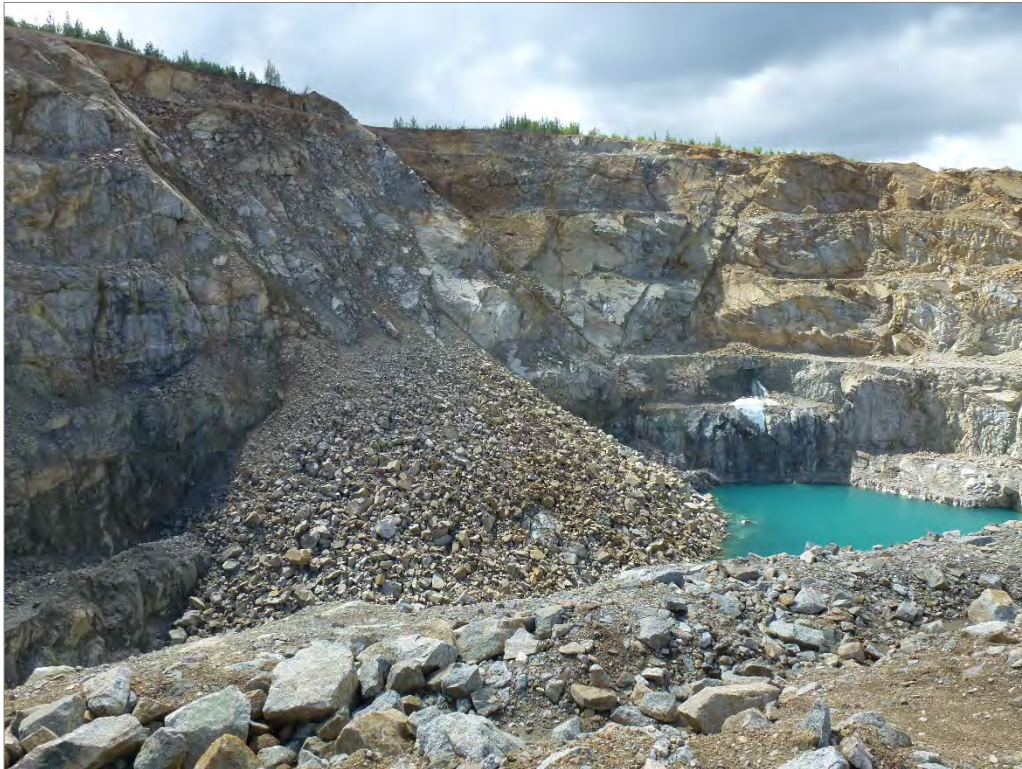
Photo 112: Previous pit wall failure in Minto North Pit (looking southwest)
