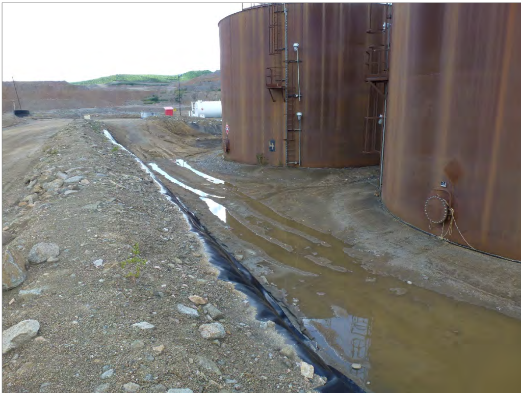
Photo 59: Fuel Containment Facility from berm crest (looking west)
