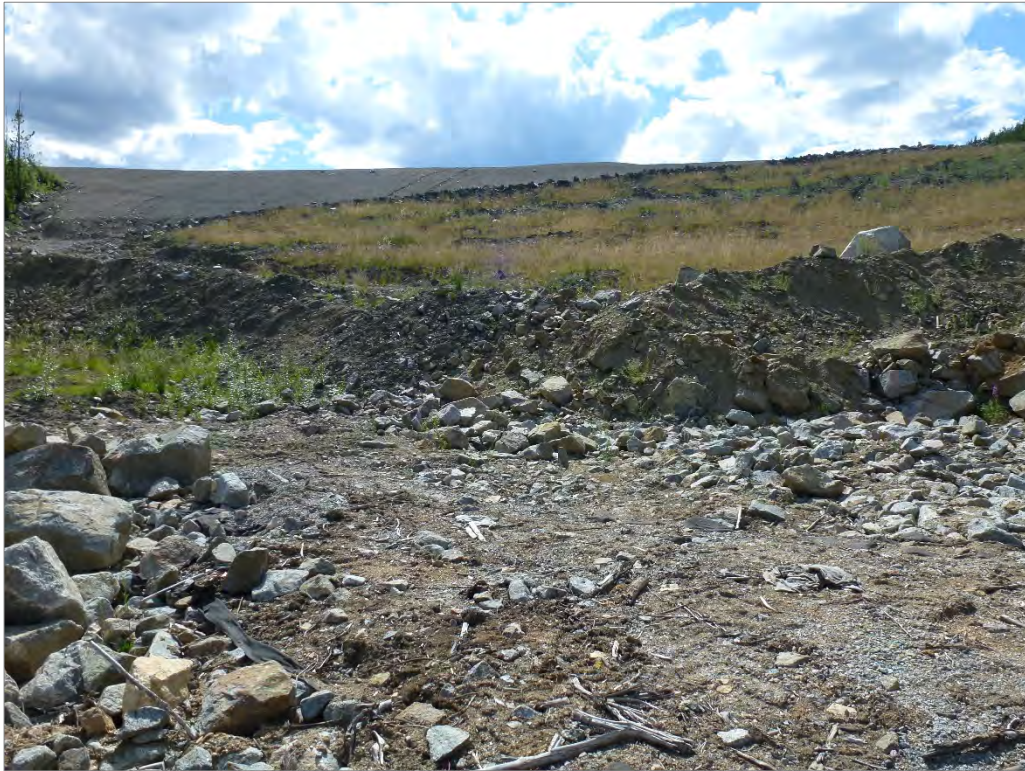
Photo 21: Downstream slope of the MVFE (looking west)
