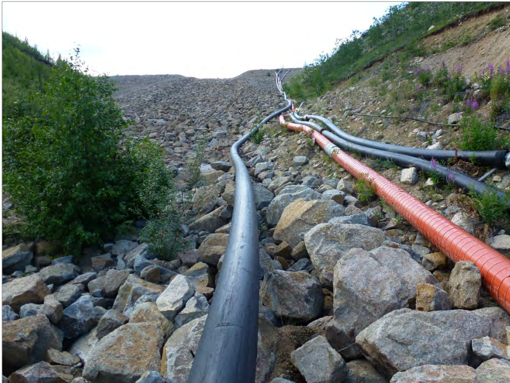
Photo 76: Looking back upslope towards the WSP Dam
