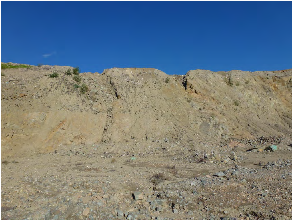
Photo 88: Highwall above In-Pit Dump with erosion gullies
