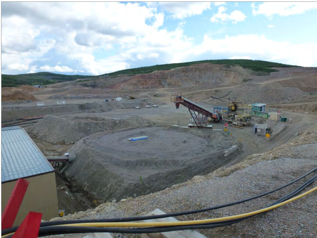
Photo 52: Mill feed stockpile pad (foreground) and ore stockpile (background) – looking south)
