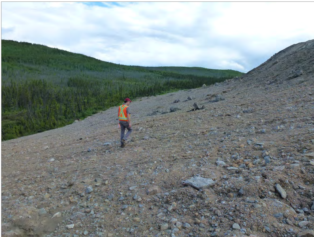
Photo 41: Regraded slopes of the SWD (looking south)
