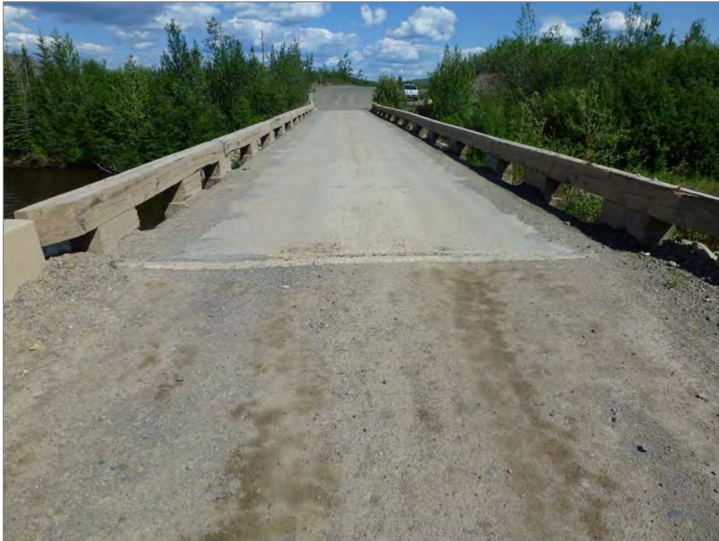
Photo 79: Top view of Big Creek Bridge (looking west)
