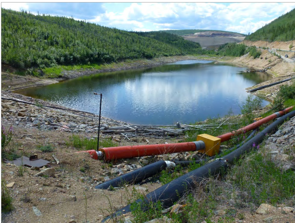
Photo 64: WSP from the upstream crest (looking southwest)
