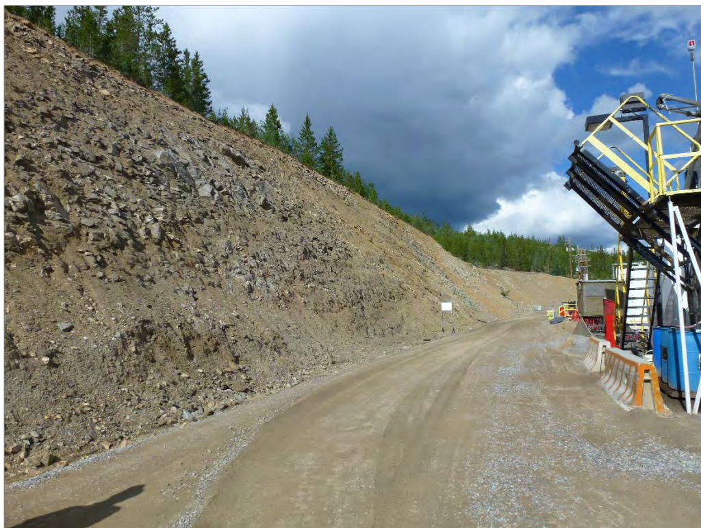
Photo 62: Highwall behind Fuel Containment Facility (looking east)
