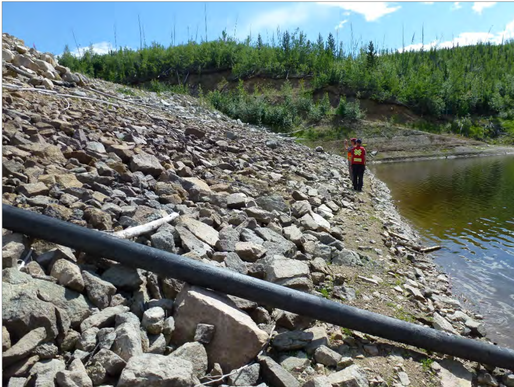
Photo 66: Upstream face of the WSP Dam (looking south)
