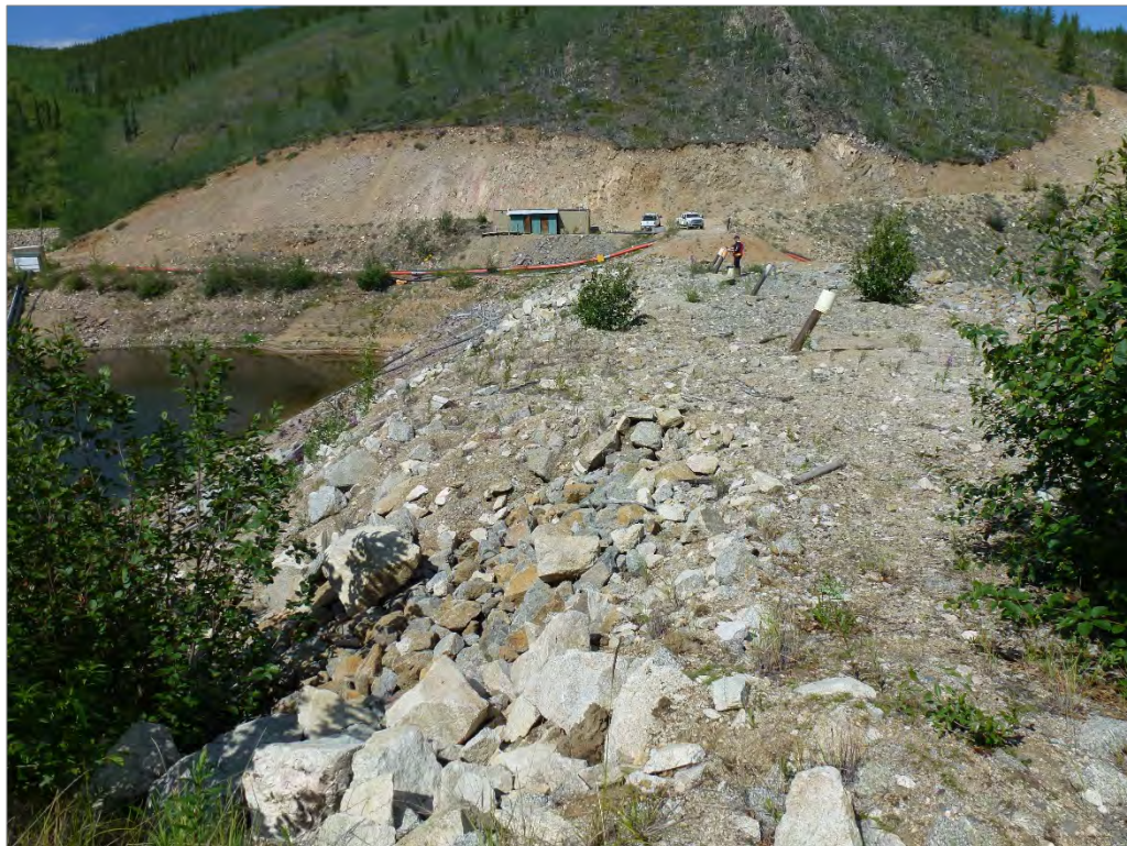
Photo 68: WSP Dam crest – looking north from the south abutment.
