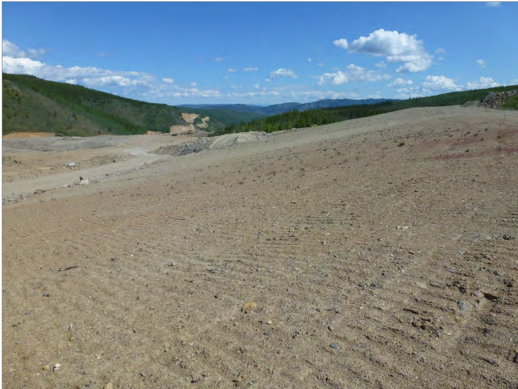
Photo 10: Covered and regraded slope of DSTSF (looking northeast)
