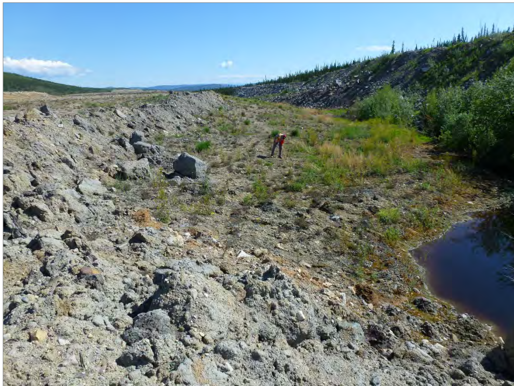
Photo 7: Portion of dry stack requiring regrading to 4H:1V closure slope (looking east)
