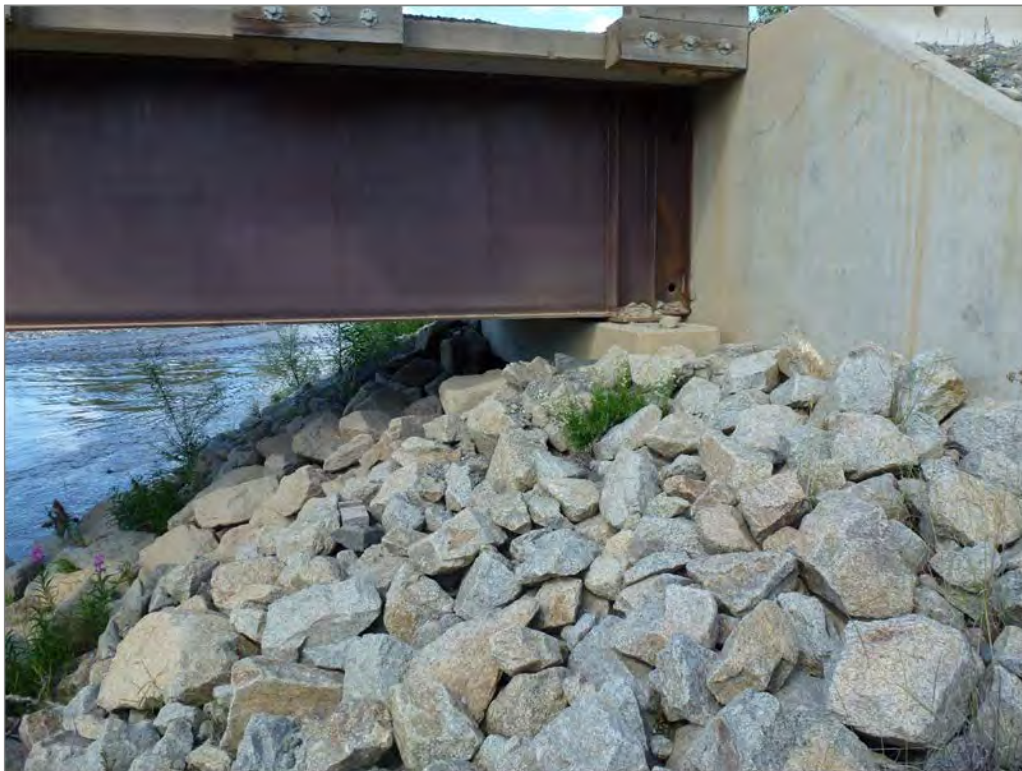
Photo 78: Big Creek Bridge eastern abutment
