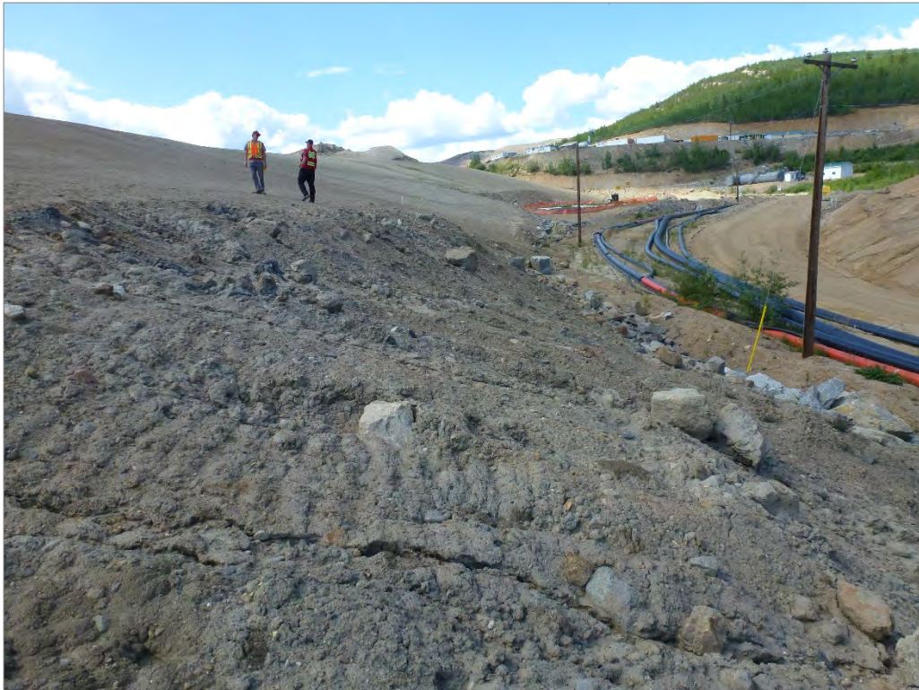
Photo 18: Area still to be regraded close to the toe (looking west)
