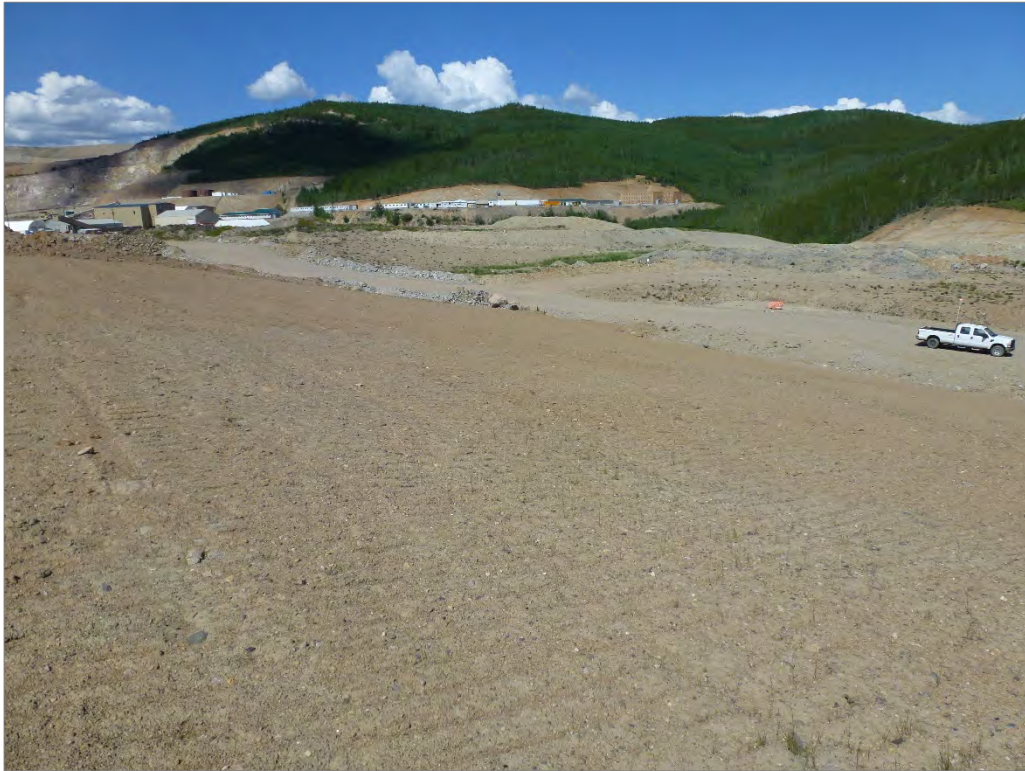
Photo 9: Covered and regraded slope of DSTSF (looking northwest)
