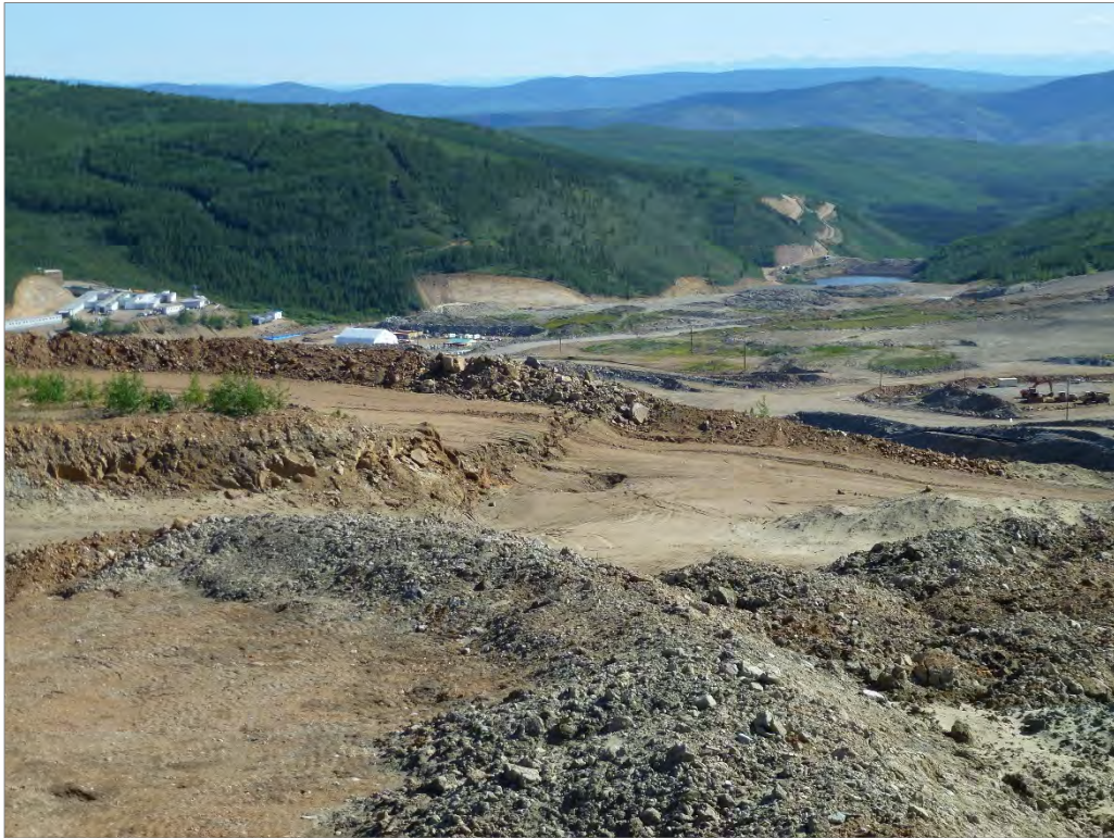
Photo 110: Slumping observed in Backfill Area
