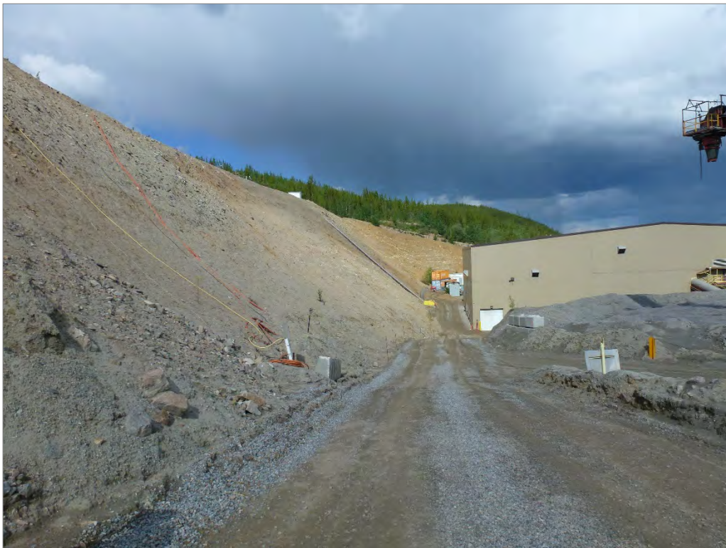
Photo 51: Highwall behind the Mill Site (looking east)
