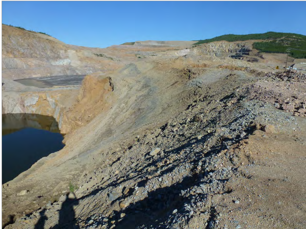
Photo 101: Slumping of the permafrost soils in the Area 2 Pit Stage 3 pit wall (looking west)
