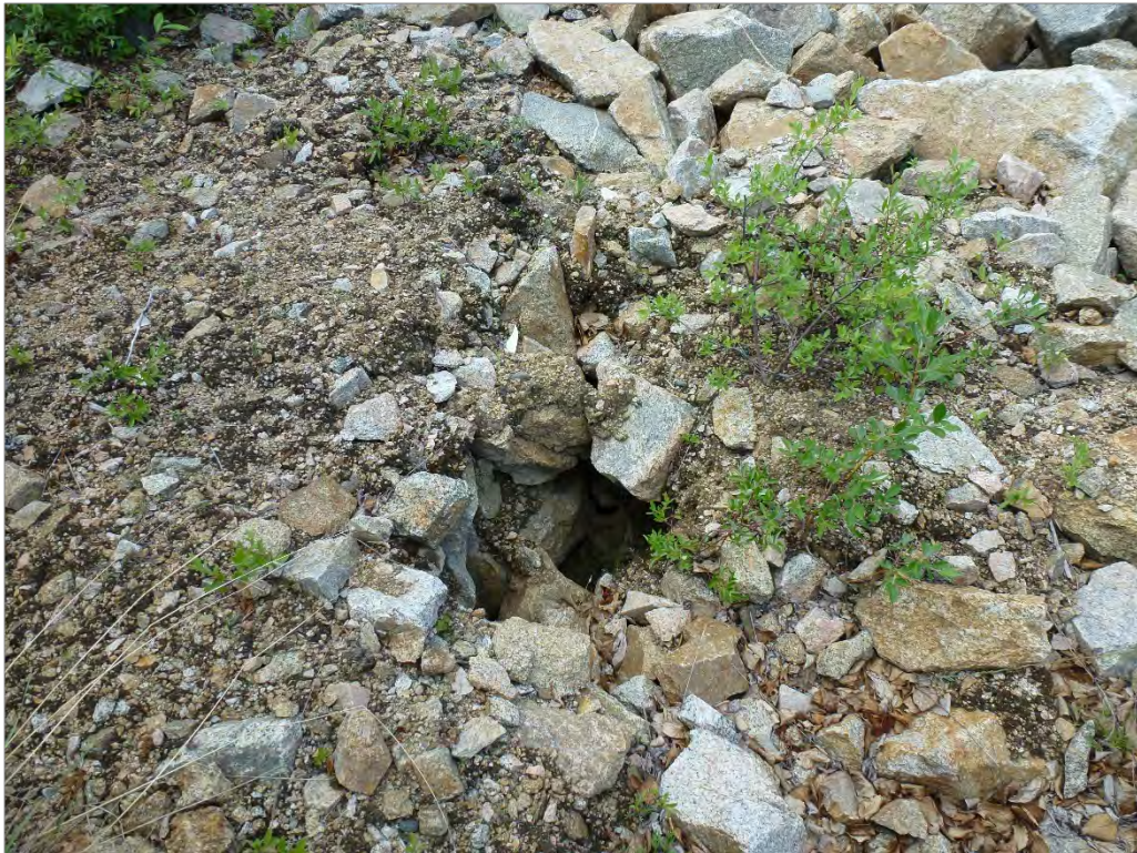
Photo 72: Potential minor sink hole
