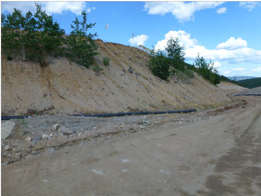
Photo 56: Erosion gullies on the slopes of the Camp Site pad (looking northeast)
