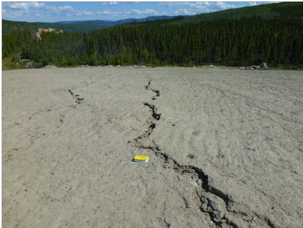
Photo 11: Erosion gully forming on closure cover (looking east)
