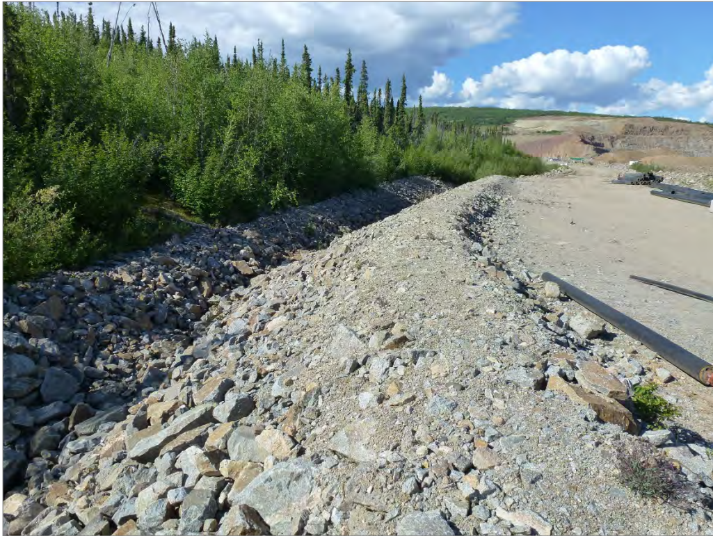
Photo 25: TDD vegetation free – looking upstream to the west
