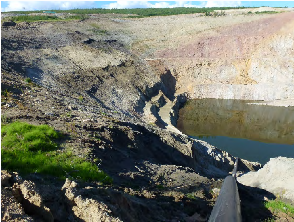
Photo 104: Erosion gully caused by surface water flow from upstream catchment
