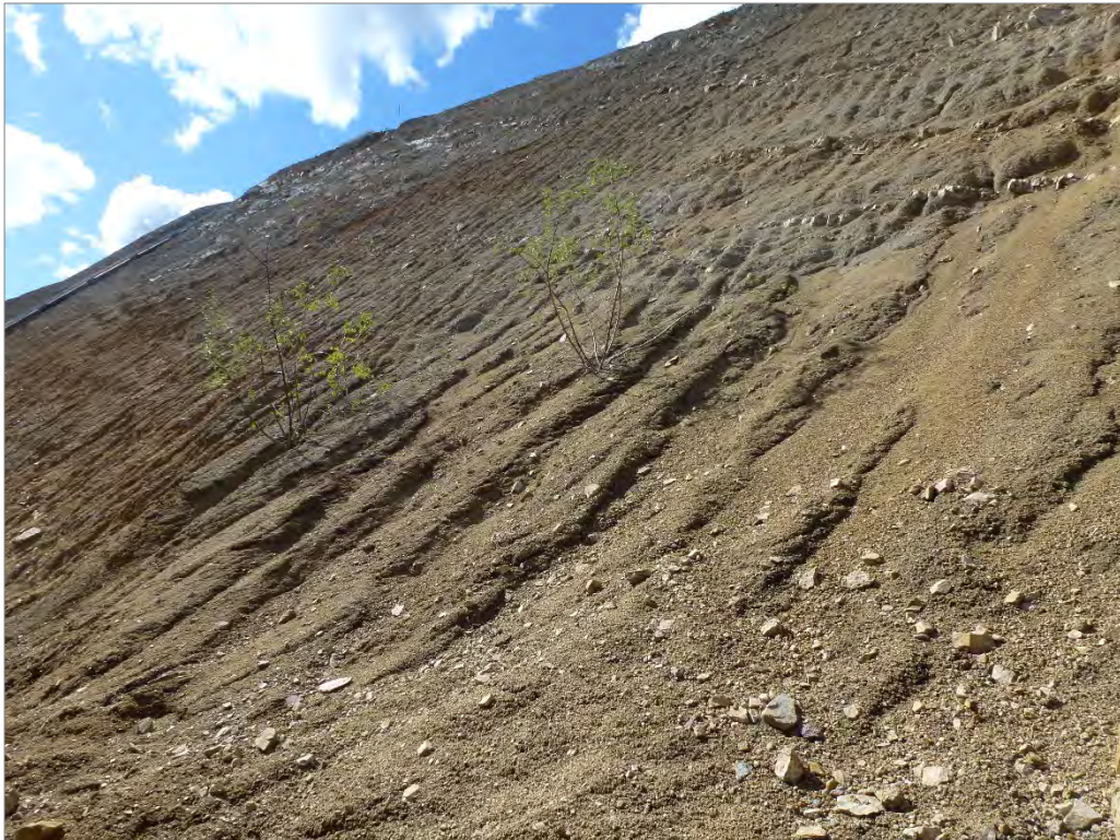
Photo 48: Minor slope erosion on the highwall
