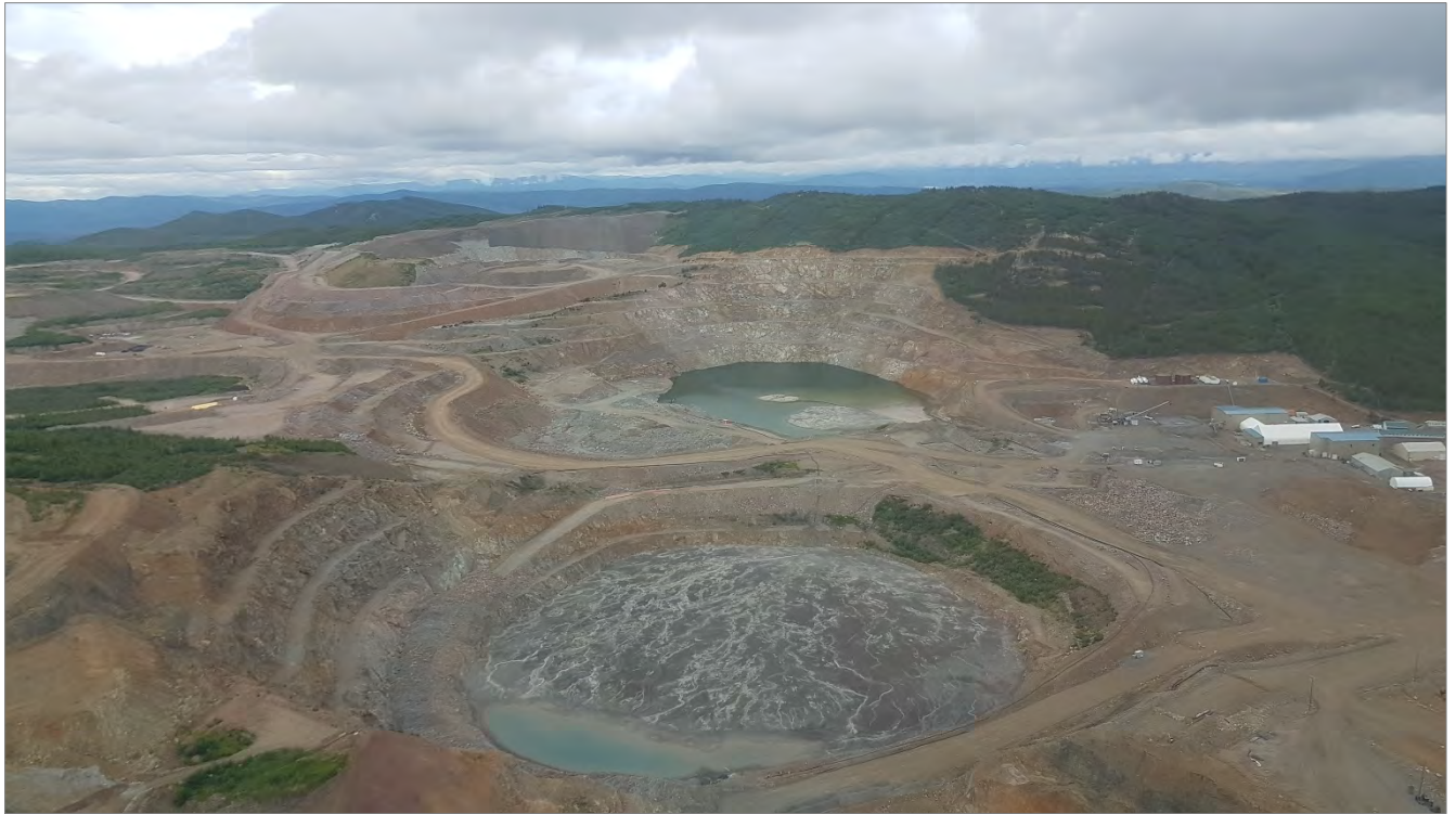
Photo 84: Aerial view of the Main Pit and Area 2 Pit Stage 2. Photo taken when flying into site. Photo location not shown on map.
