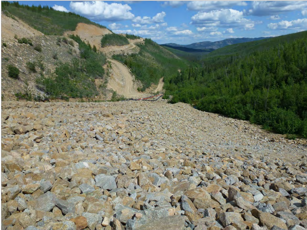
Photo 69: WSP Dam downstream slope (looking east)
