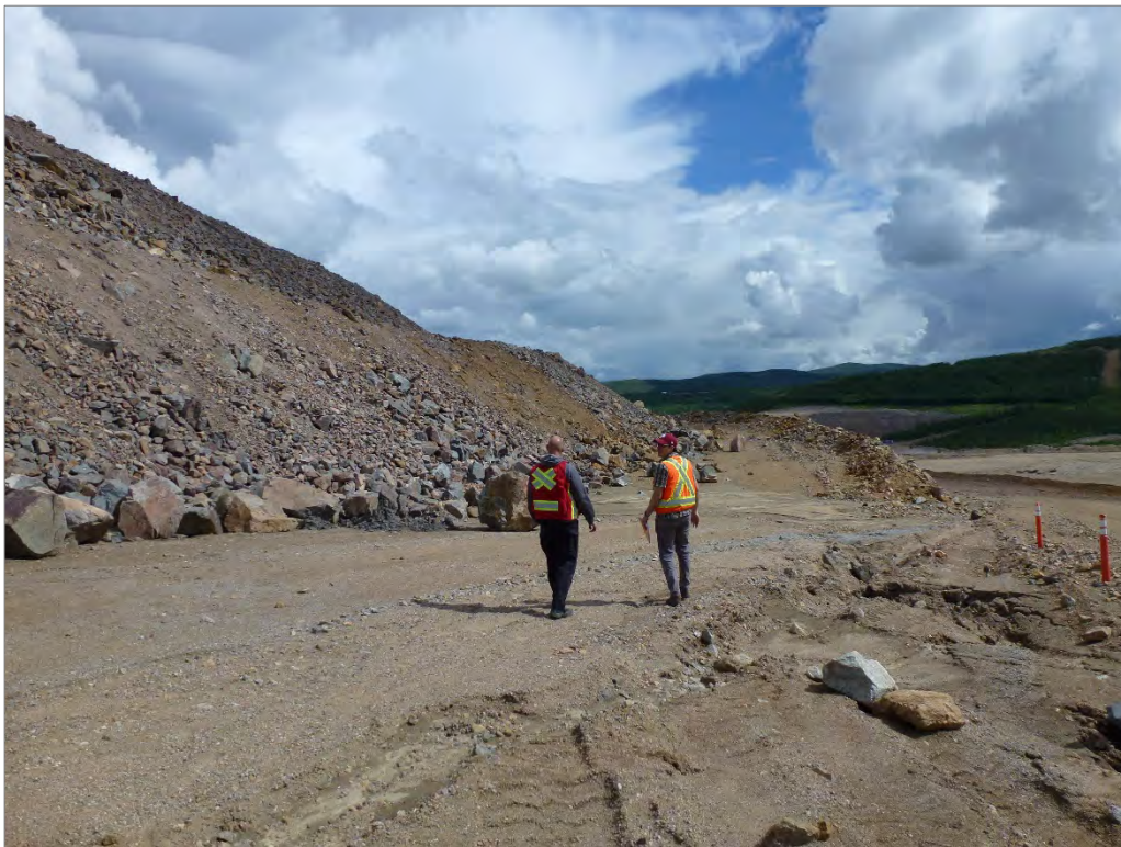
Photo 31: Toe of the MWD Wrap (looking east)
