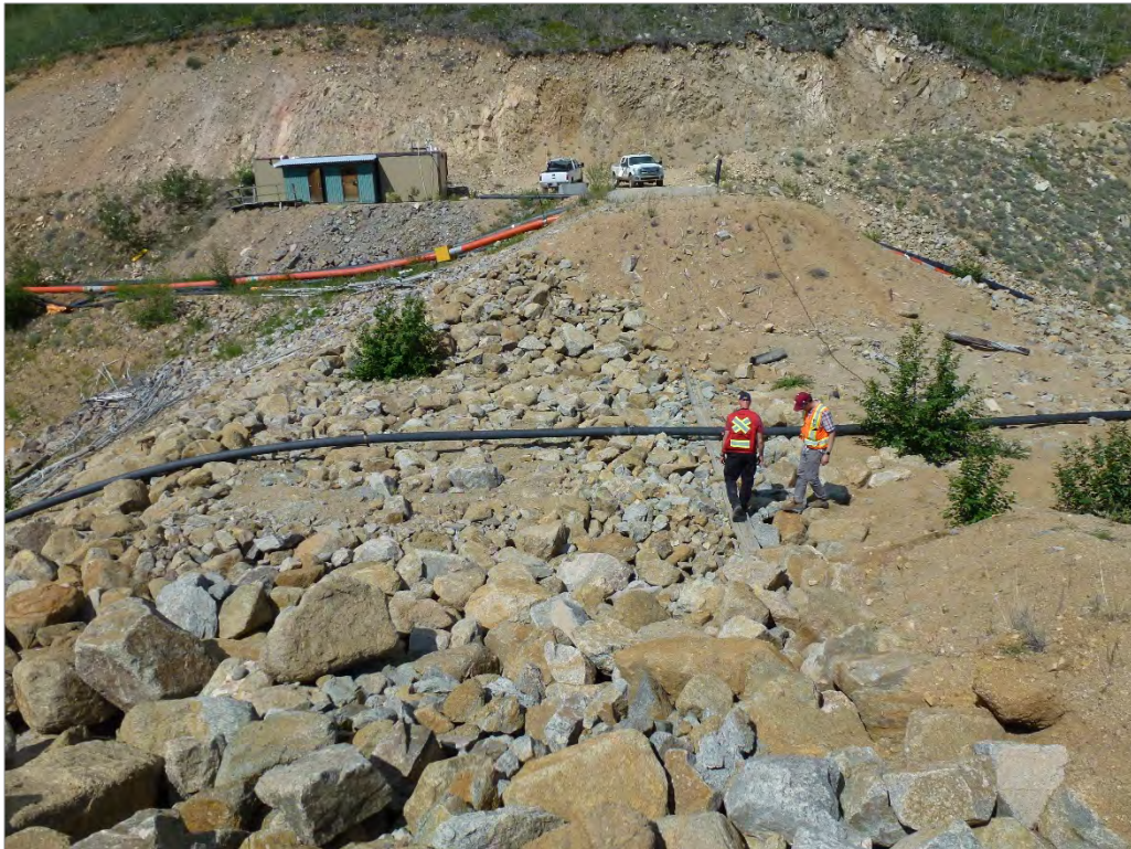
Photo 70: WSP Dam spillway (looking north)
