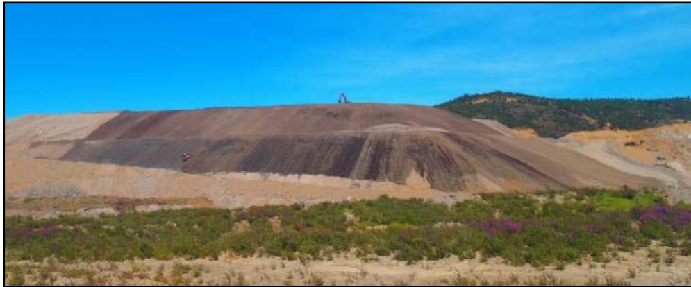
Figure 4-8 Main Waste Dump as it appeared in July 2012 with final placement of overburden into distinct plots
