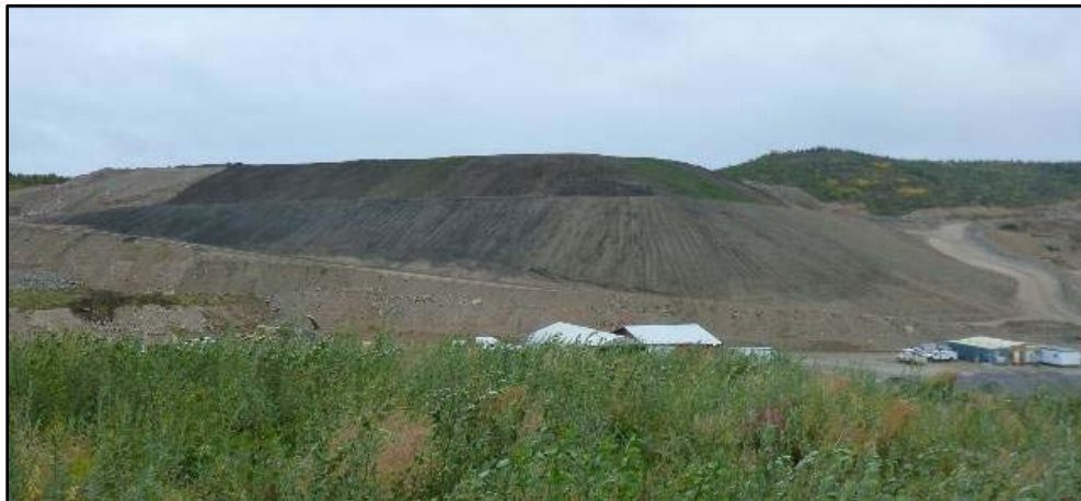
Figure 4-8 Main Waste Dump as it appeared in July 2012 with final placement of overburden into distinct plots
