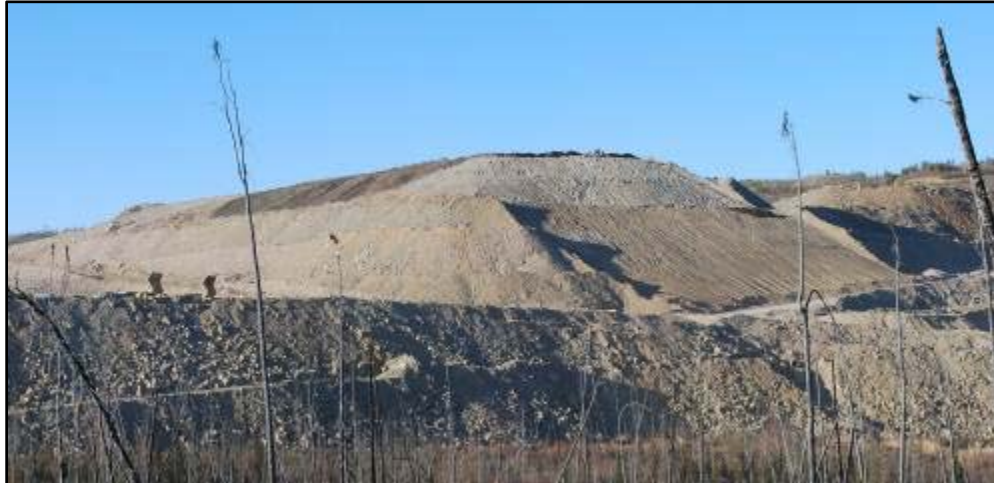
Figure 4-7 Main Waste Dump near the end of construction season 2011 (September)
