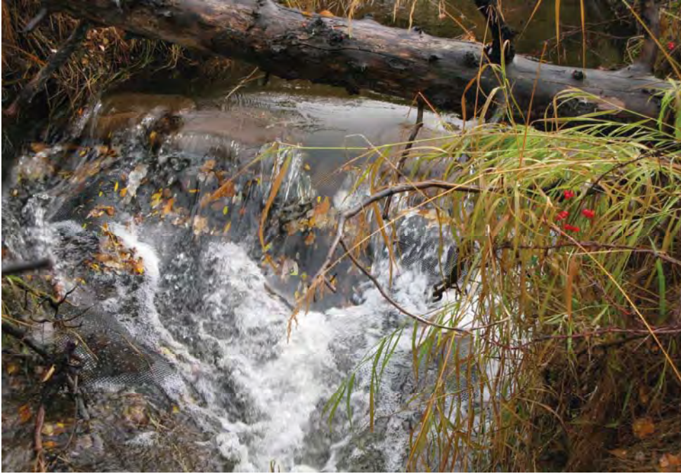
Plate 4. Different view of the same temporary fish barrier as in Plate 3.
