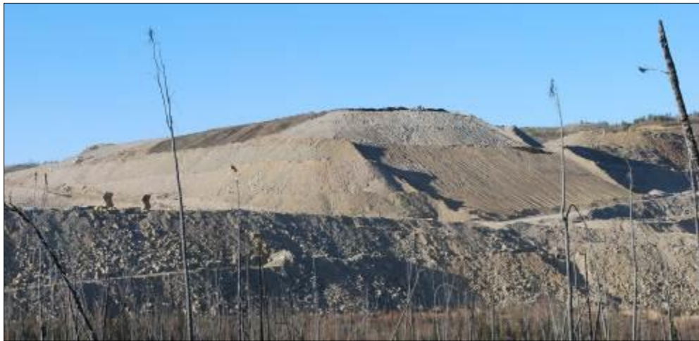
Figure 2-2: Main Waste Dump near the End of Construction Season 2011 (September)
