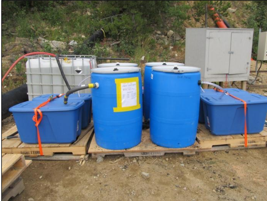
Figure 2-12: Pilot-Scale Bioreactors at Minto Mine (Picture taken in August 2014)
