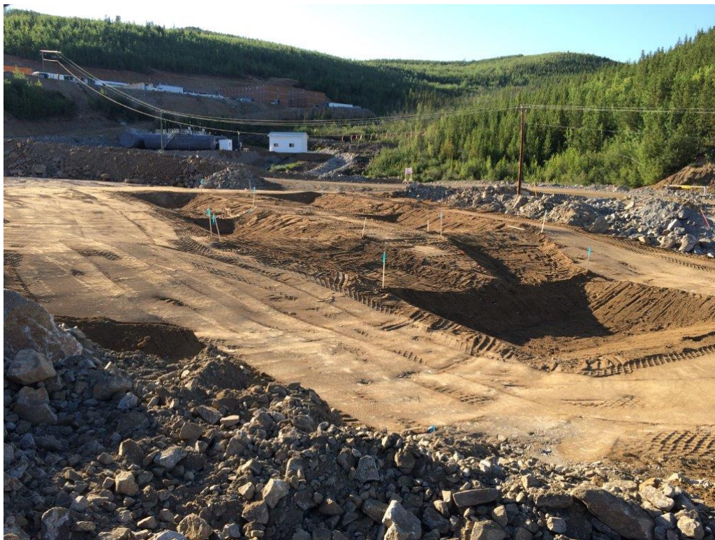
Figure 3. Demonstration-scale CWTS prior to liner installation.
