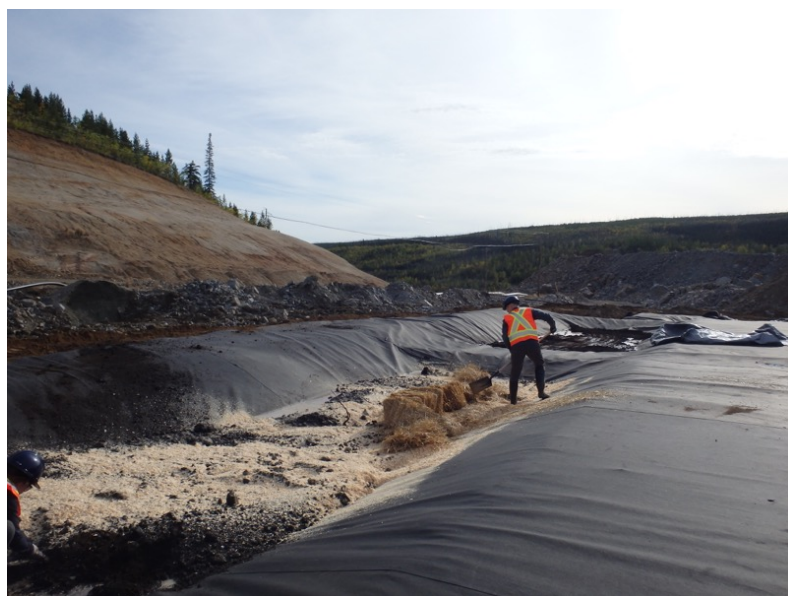
Figure 7. Mixing organic amendments into soil in demonstration-scale CWTS cell 2A.
