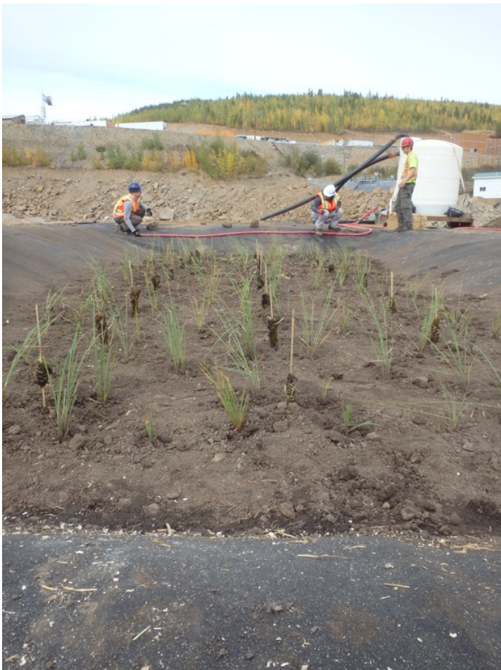
Figure 12. C. aquatilis planted within grid of moss stakes in demonstration-scale CWTS cell 2A, and influent perforated pipe being laid in place.
