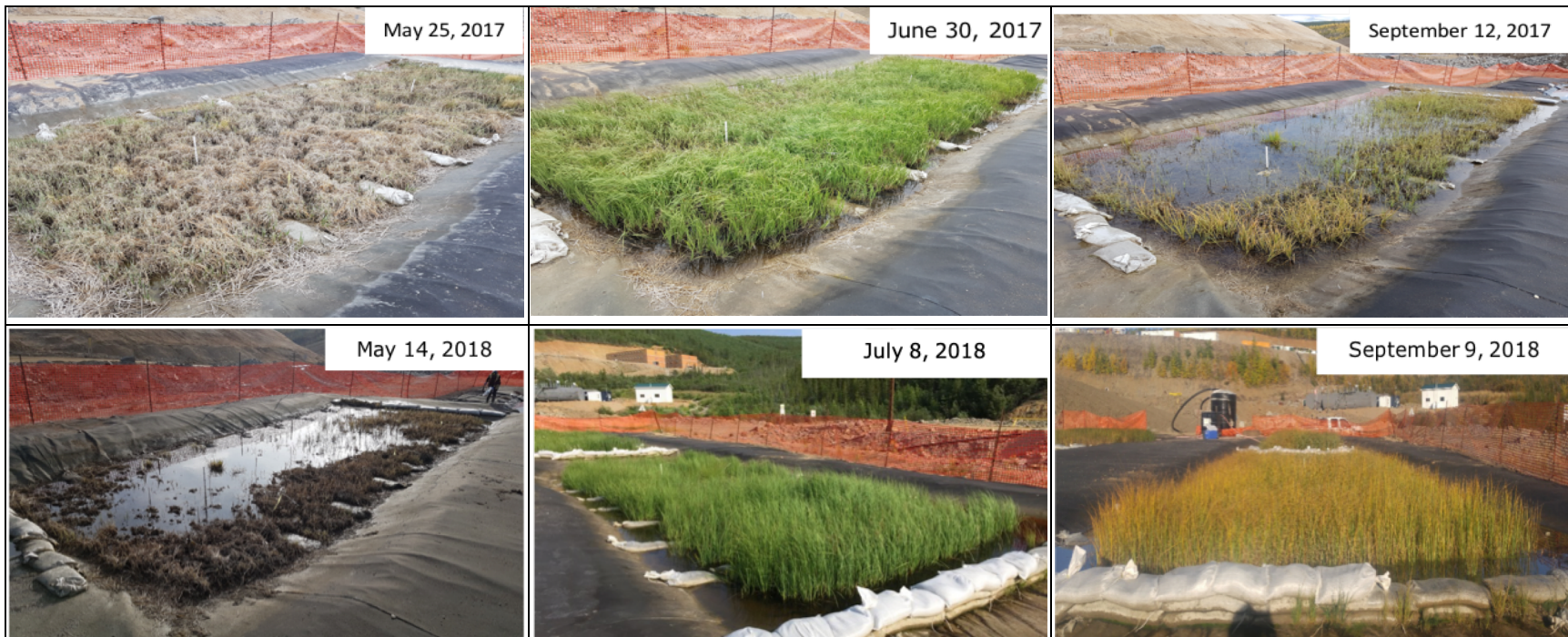
Figure 4 continued – Maturation of the CWTS from construction through operations. 2017 and 2018 pictures show cell 1B. September 12, 2017 shows increased yellowing and die off in cell 1B due to aphid infestation.
