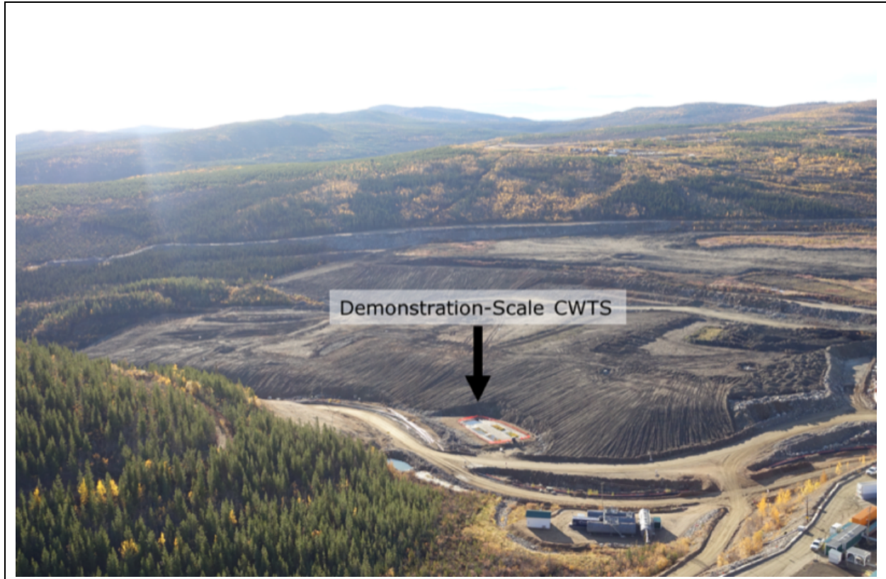
Figure 1 – Picture of demonstration-scale CWTS at Minto Mine.
