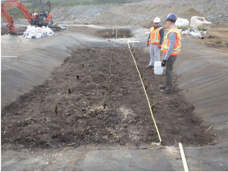
Figure 11. Moss stakes placed in demonstration-scale CWTS cell 2A, looking towards cell 2B.
