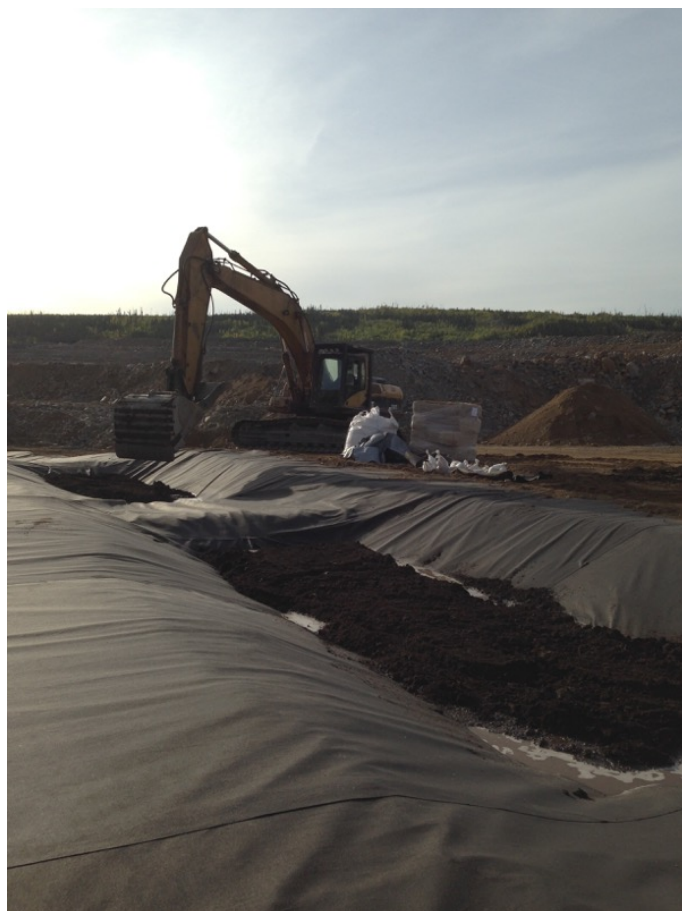
Figure 5. Soil being added to demonstration-scale CWTS cells.
