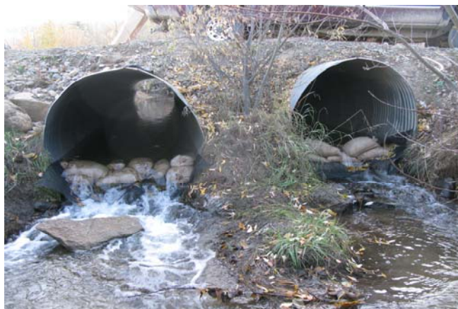
Plate 2. Temporary fish barriers placed at the outlets of Road crossing culverts – Km. 11, Minto Mine Road.
