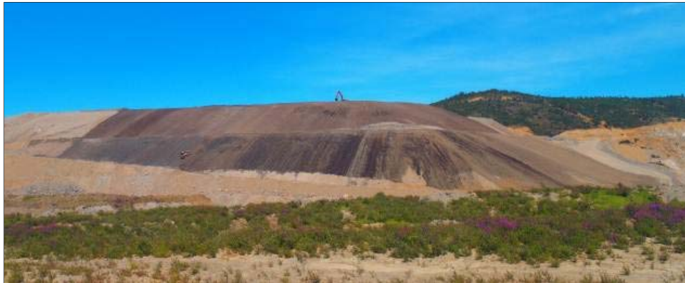
Figure 2-3 Main Waste Dump as it appeared in July 2012 with final placement of overburden into distinct plots
