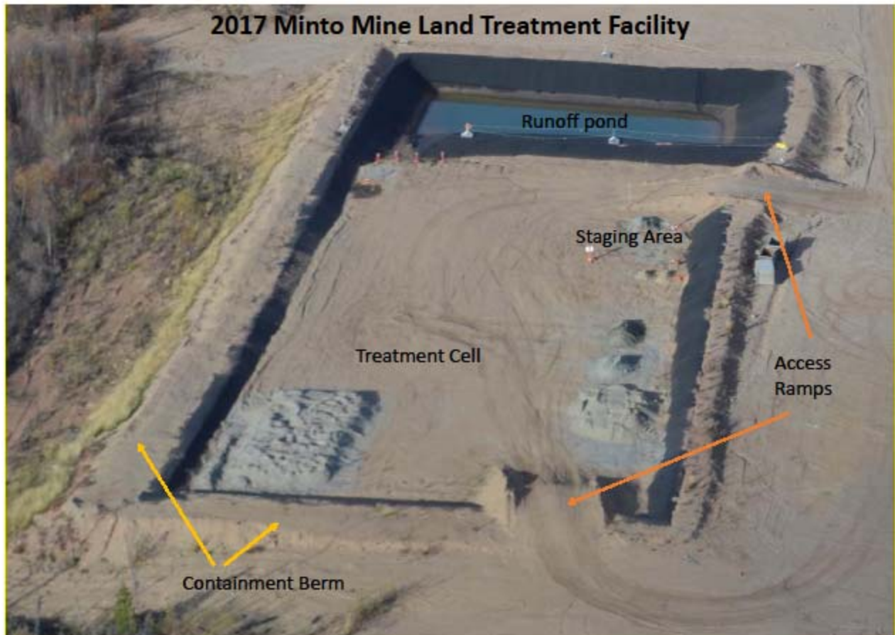
Figure 3-1: Land Treatment Facility
