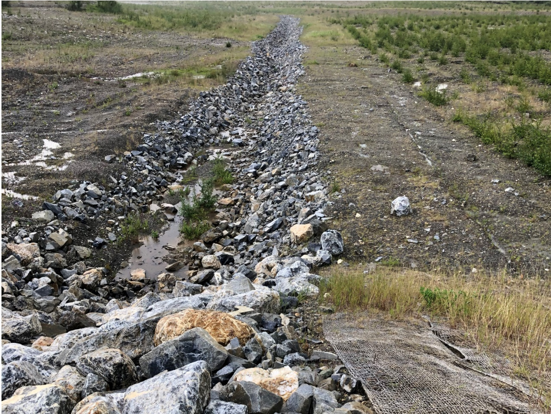
Photo 9 View south of the South Drainage Channel
