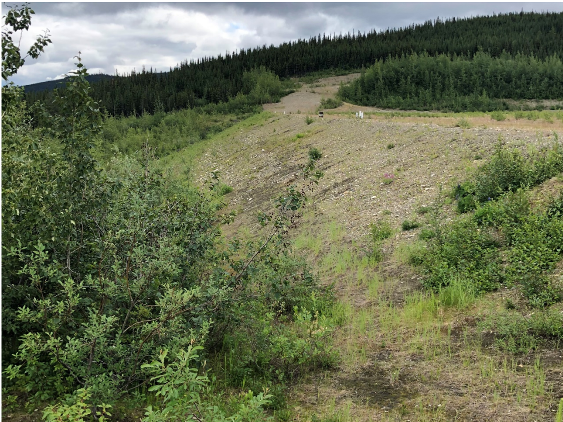
Photo 2 View east over the downstream face of the North Dam
