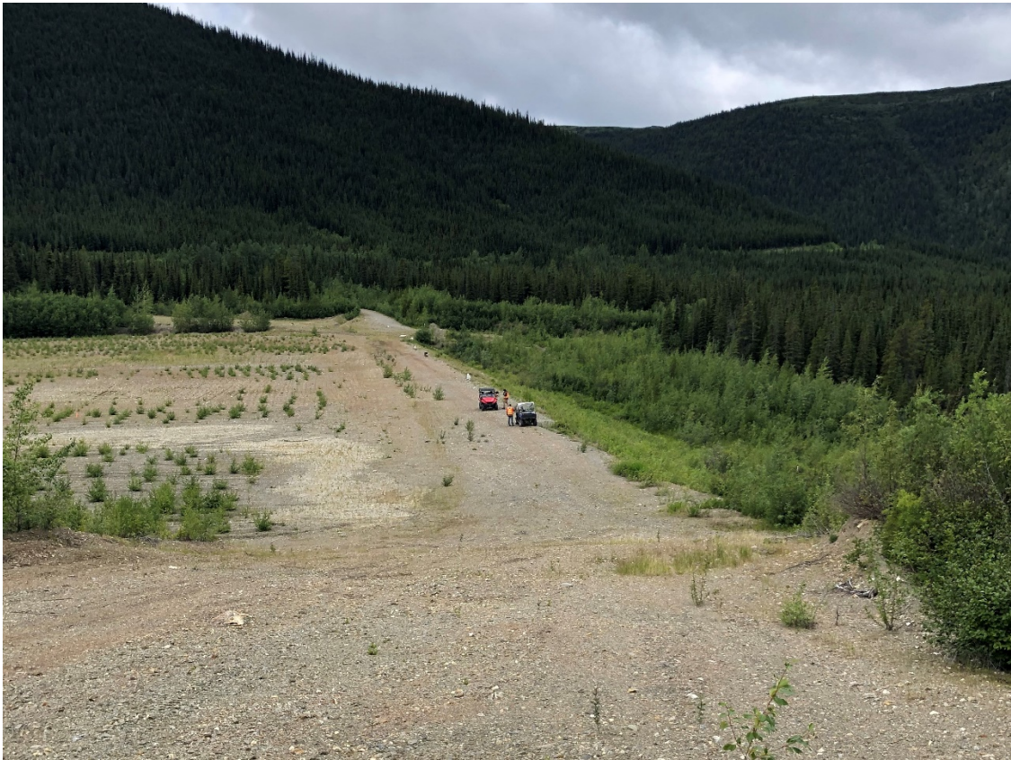
Photo 1 View West of the North Dam
