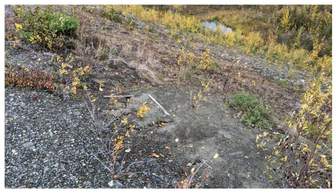
Photo ND-07: Wind-blown tailings on the downstream face of the dam immediately below the crest.
