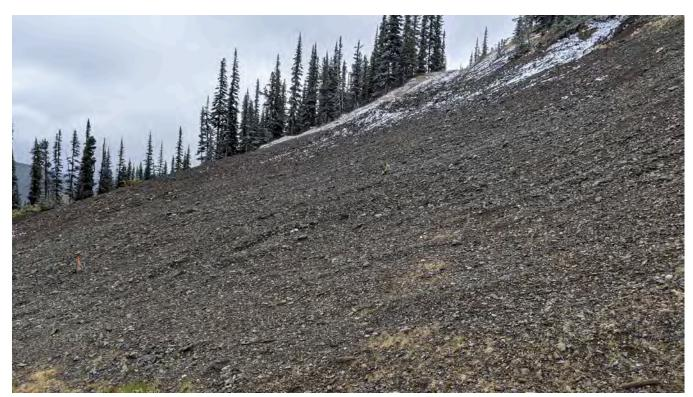
Photo WR-17: Regraded 1300 Portal Waste Rock Dump and 1300 Portal area.
