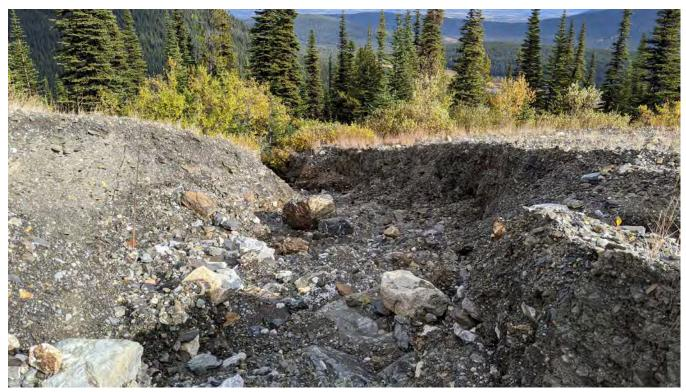
Photo WR-01: Erosion gulley at the base of Jewelbox Waste Rock Dump looking downslope. The gulley has eroded down to bedrock.
