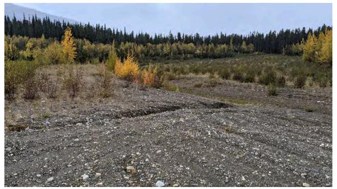
Photo L-02: Erosion gulley in the landfill area.
