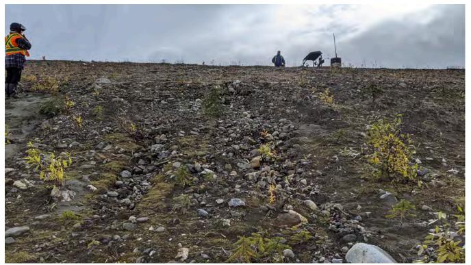
Photo ND-04: Sheet and rill erosion of wind-blown tailings and fine-grained soil on the downstream slope of the North Dam.
