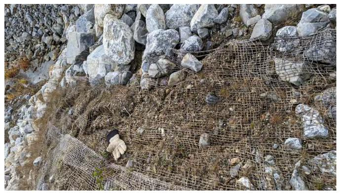
Photo SRS-05: Transverse cracking adjacent to the east spillway crest that is suspected to be due to froze heave.
