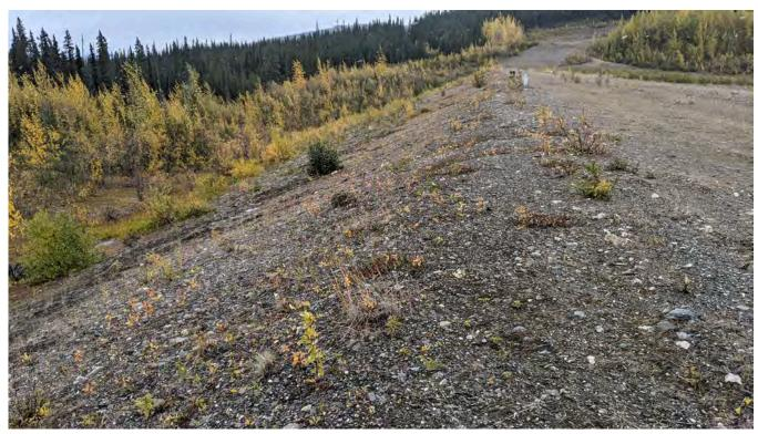
Photo ND-03: Downstream slope of the North Dam looking east from the near the west abutment. Minor sheet and rill erosion present
