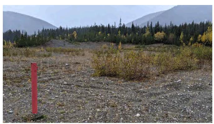
Photo L-01: Landfill area looking east. Frost heave has lifted the monitoring well casing in the photo foreground up approximately 15 cm.
