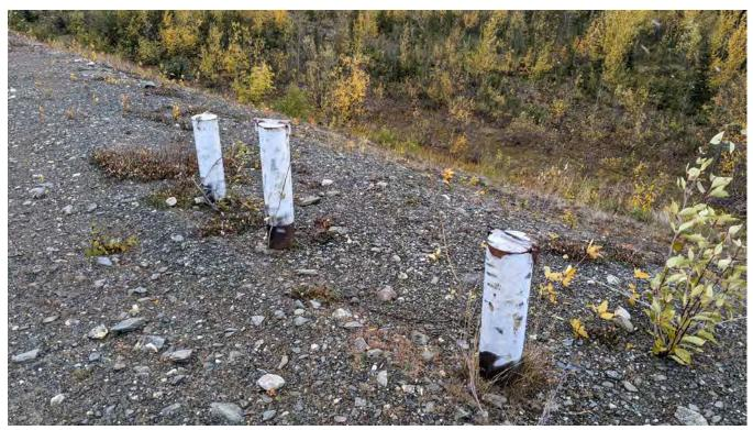
Photo ND-05: Piezometer protective casings on the North Dam crest.
