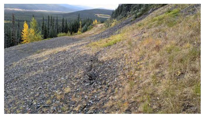
Photo WR-16: Regraded Burnick Waste Dump and 1200 Portal Area looking south. Minor settlement cracking is visible in the foreground. The scarp is approximately 5 cm in height.
