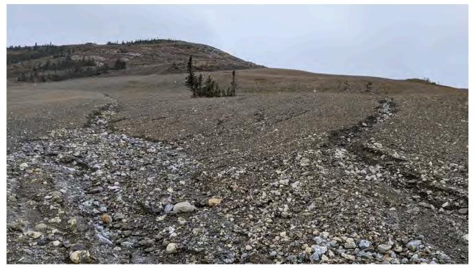
Photo WR-04: Jewelbox Waste Dump – confluence of erosion channel upstream of the gulley shown in Photos WR-01 to WR-03.
