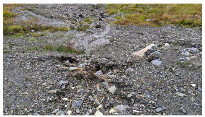
Photo DC-02: Area of the North Diversion berm repair area completed in 2020 looking west from the berm crest. Additional surface erosion over the berm has occured. Seepage emerging at the toe of the repair area is clear with no sign of sediment transport.
