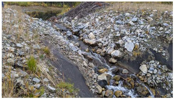
Photo NC-02: On-going channel erosion at the downstream end of the upper decommissioned access road crossing of North Creek to the landfill area.
