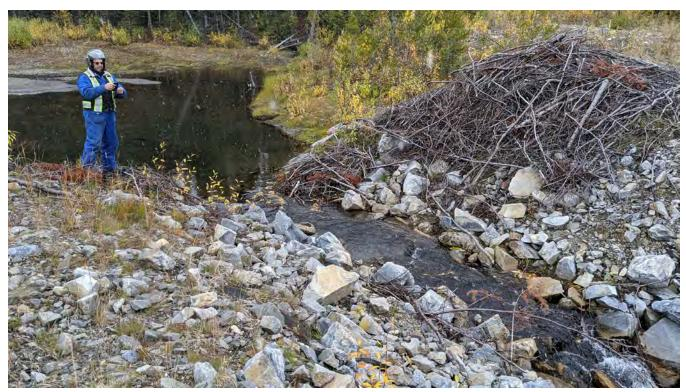
Photo NC-01: Beaver dam removed from the inlet of the upper decommissioned access road crossing of North Creek to the landfill area.
