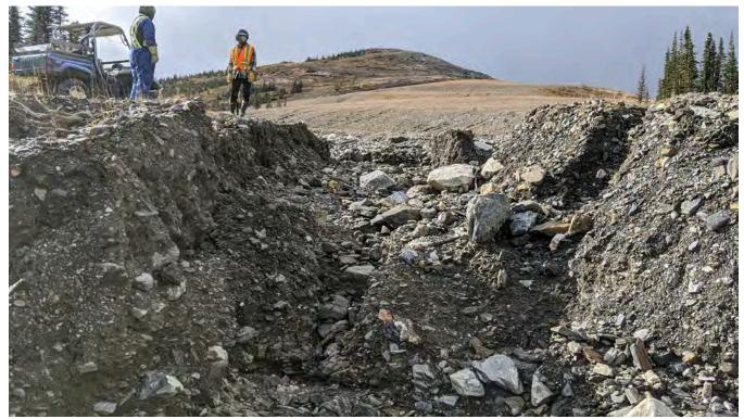
Photo WR-02: Erosion gulley at base of Jewelbox Waste Dump looking upslope.
