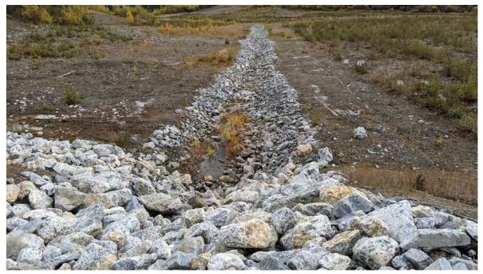
Photo SRS-04: Downstream slope of the SRS spillway and upstream end of the South Drainage Channel.
