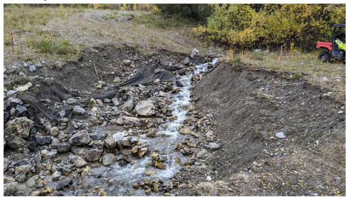
Photo NC-04: On-going channel and bank erosion at the downstream end of the lower decommissioned access road crossing of North Creek to the landfill area.
