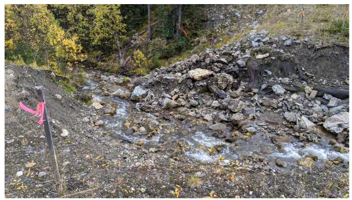
Photo NC-03: On-going channel and bank erosion at the downstream end of the lower decommissioned access road crossing of North Creek to the landfill area.
