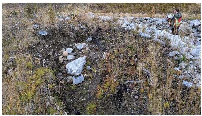
Photo DC-03: Erosion gulley at the downstream end of the North Diversion Channel Berm looking northeast.
