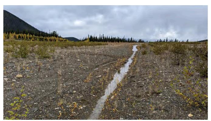
Photo TC-01: Drainage Swale that flows south through the middle of the tailings cover.
