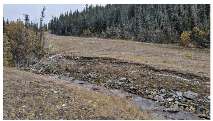
Photo WR-13: Subsidence of the south slope of North Creek across the decommissioned access road to the Burnick Zone.
