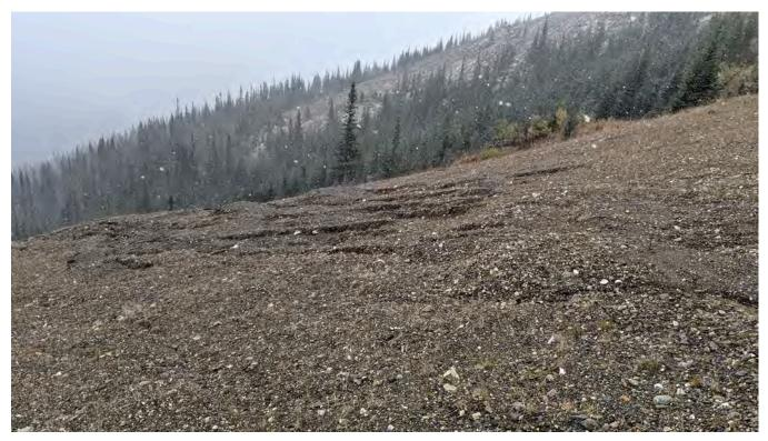
Photo WR-06: Surficial sloughing/deformation downslope of the 1408 Portal.
