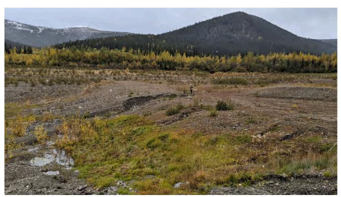
Photo TC-03: Erosion gully at the south end of the till cover and north of the SRS pond. No exposed tailings were observed.
