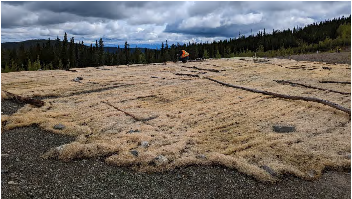
Photo NE-08: North embankment gully repair erosion protection mat.
