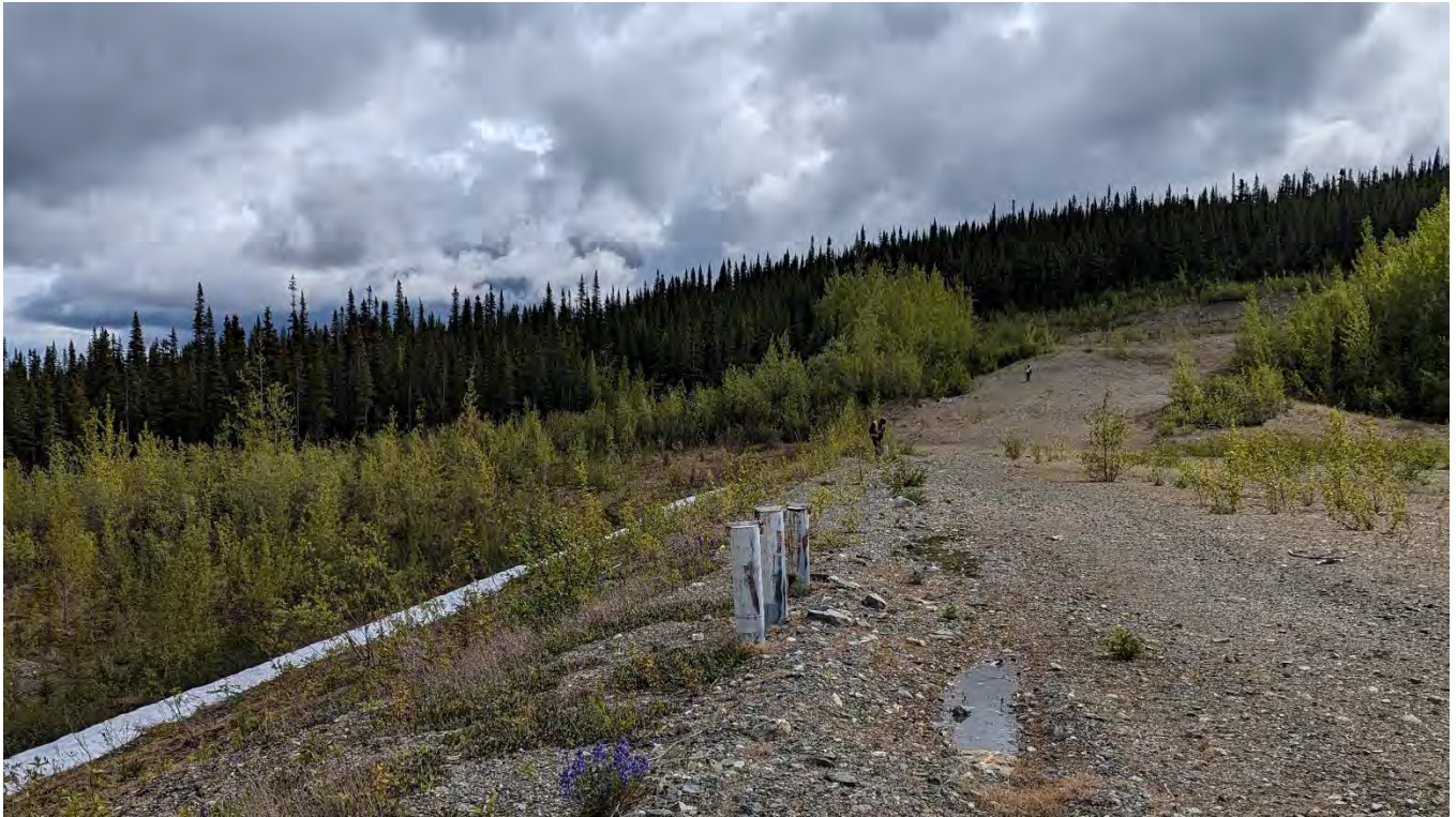
Photo NE-03: North embankment crest piezometers casings.
