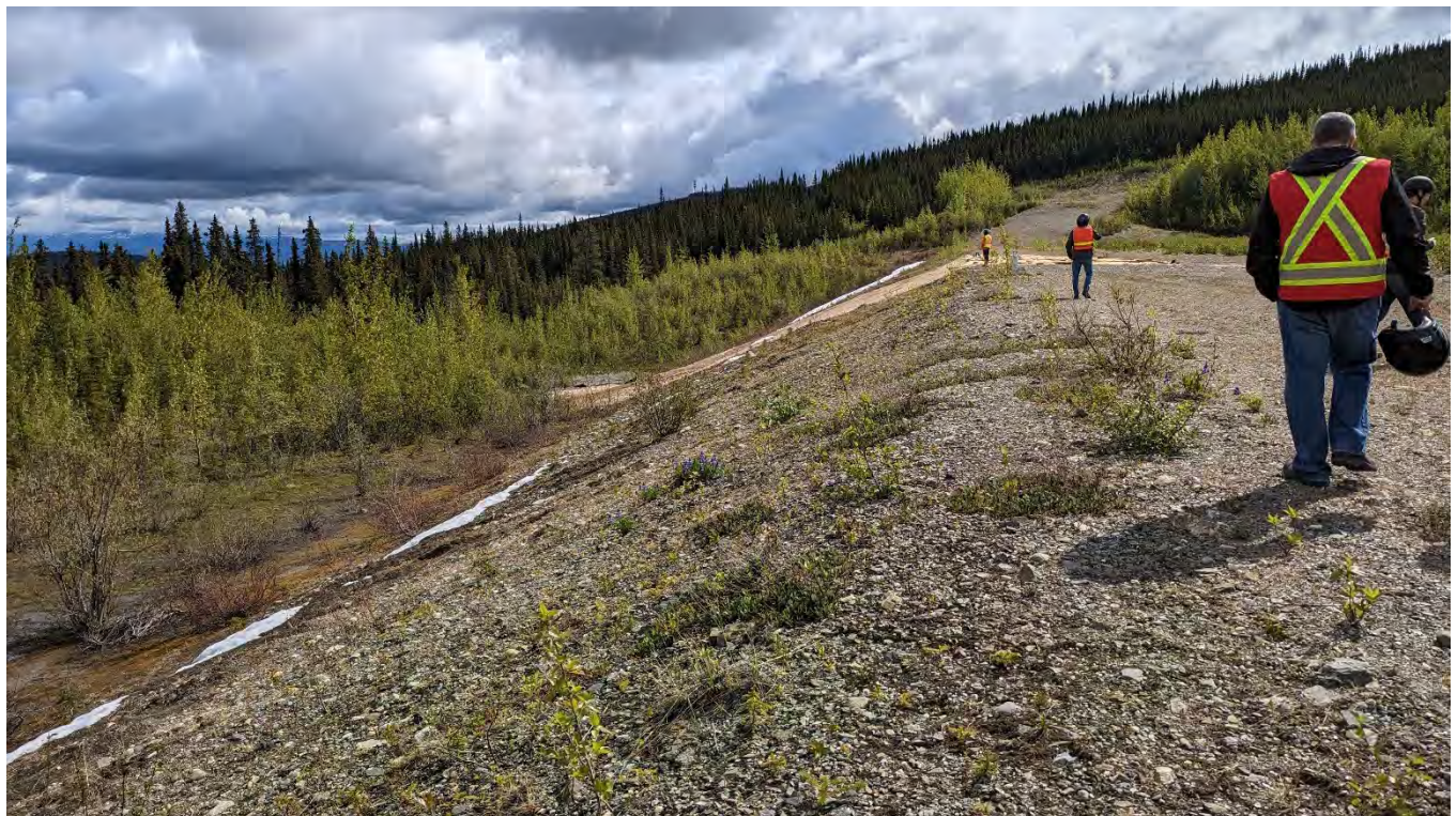
Photo NE-02: A closer look to the North embankment crest.
