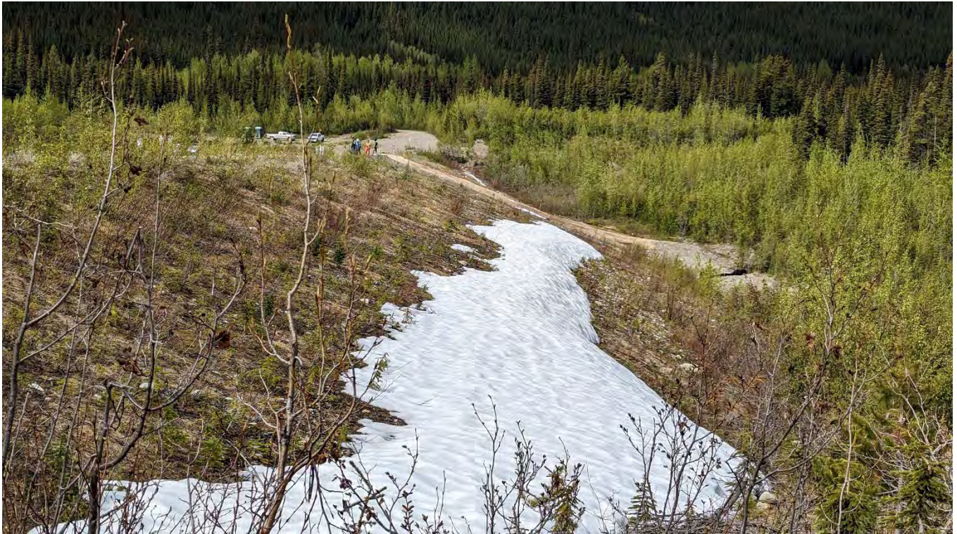
Photo NE-05: North embankment downstream slope vegetation seen from the east abutment.
