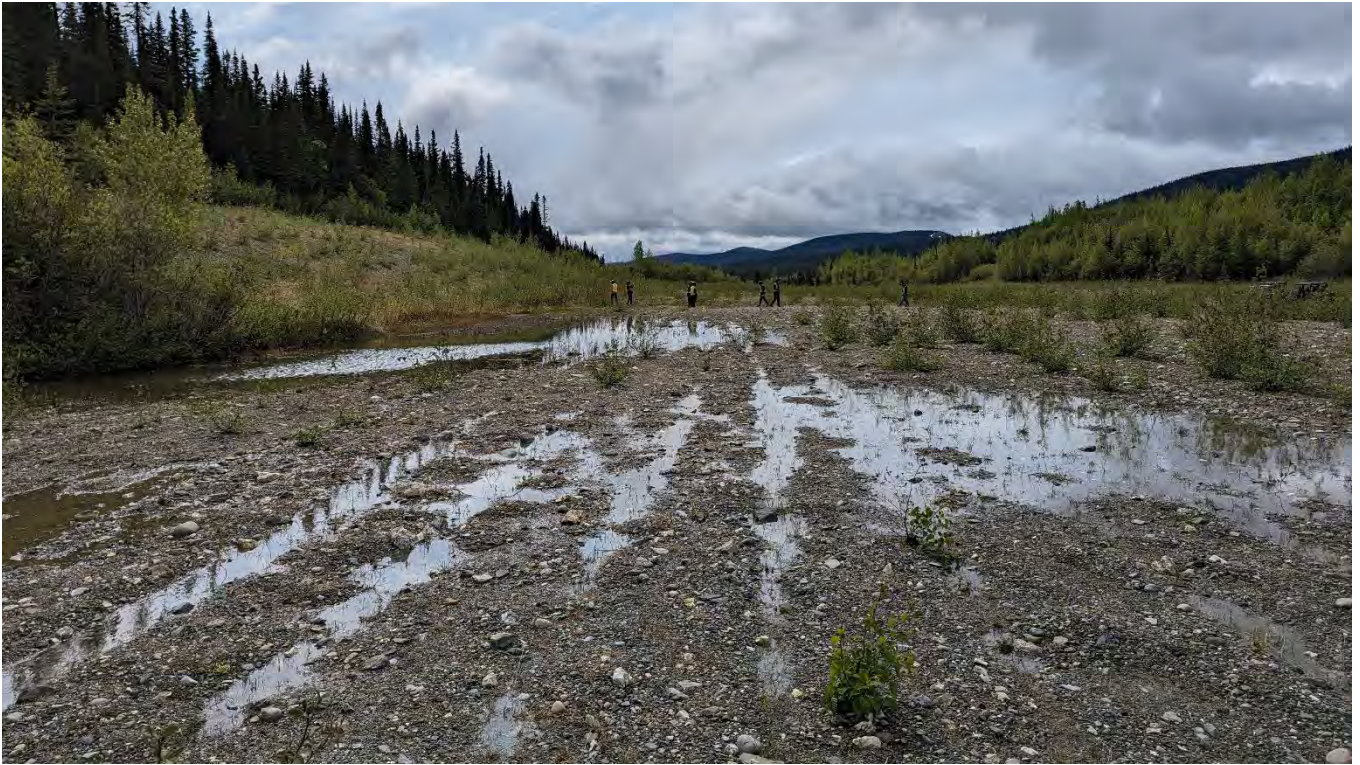
Photo TC-05: Scarification oriented parallel to the main drainage channel impeding drainage
