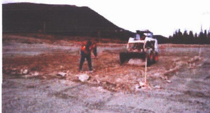
Plate 5 Machine and Manual Scarification of Site #5a
