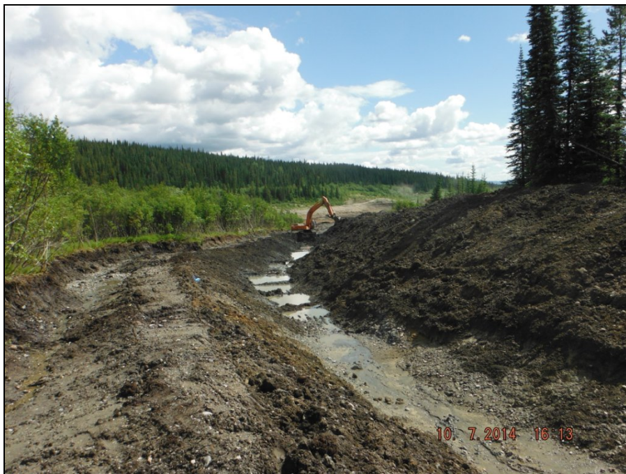
TMA Photograph 4: Excavation of Camp Creek Drainage Channel.
