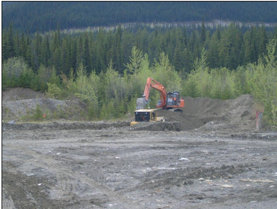
MISC Photograph 6: Construction of landfill cell.
