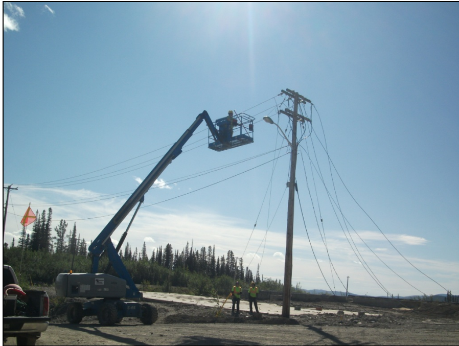
ELEC Photograph 5: CIPC disconnecting power cable from poles at mill site.
