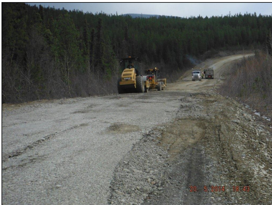
MISC Photograph 2: Road maintenance activities along SDH main access road.
