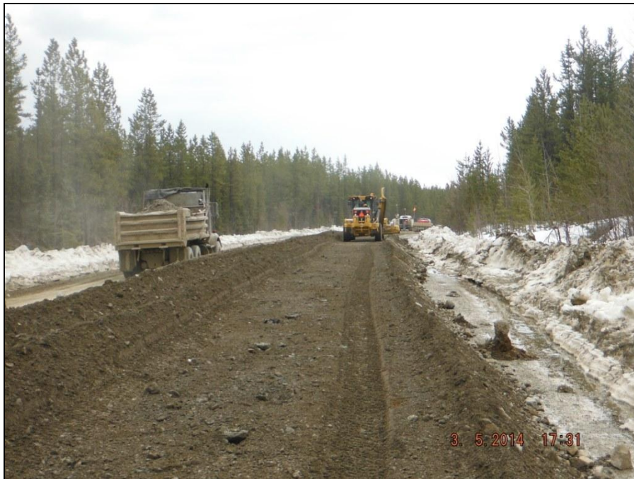
MISC Photograph 1: Road maintenance activities along SDH main access road.
