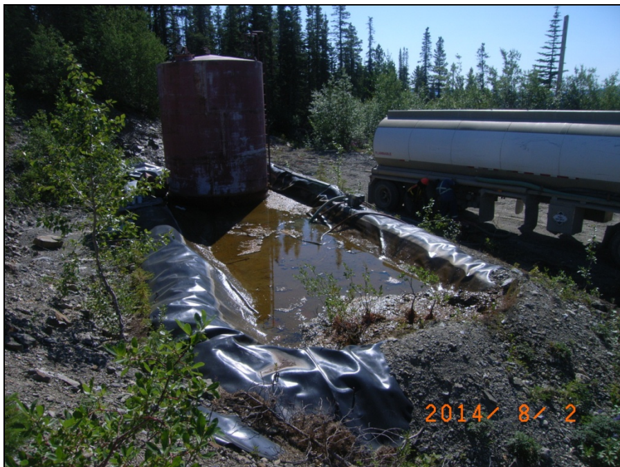
TANK Photograph 2: KPI pumping water from containment berm around tank near ball storage area into tanker for off-site disposal.
