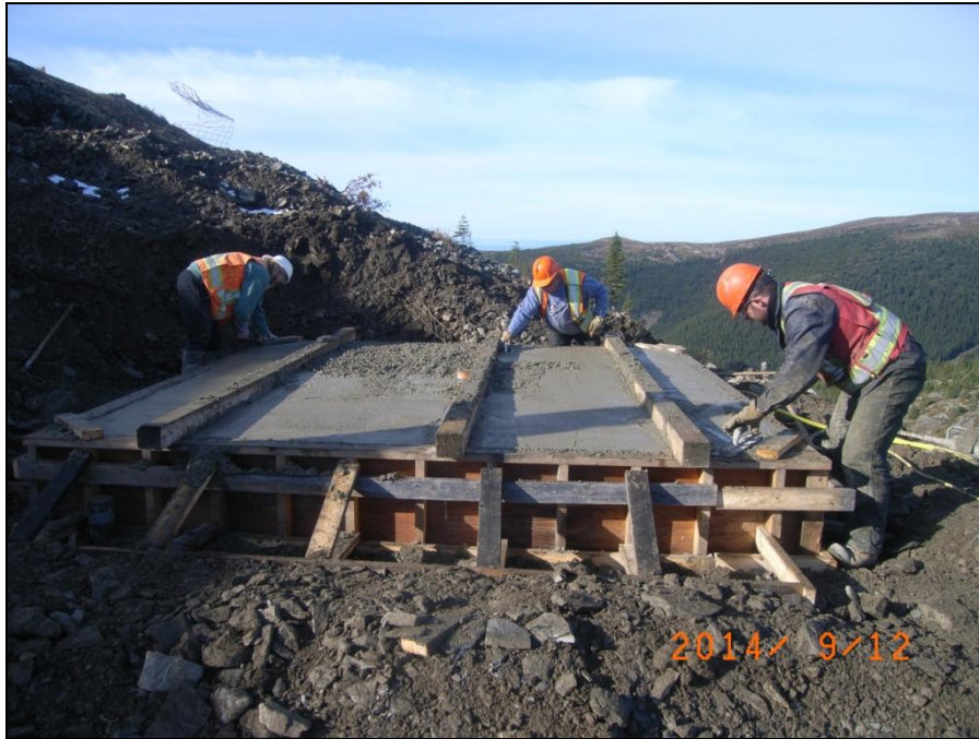
MTN Photograph 15: Concrete poured at Jewelbox Summit Ventilation Raise.
