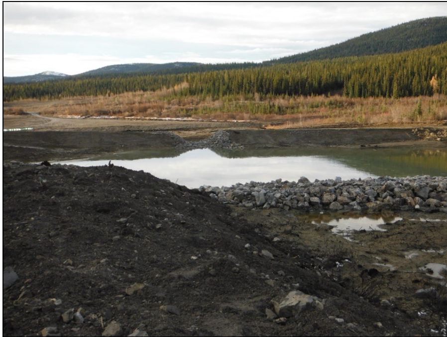
TMA Photograph 17: Looking south from east bank of former South Pond toward sediment retaining pond and sediment retaining structure with spillway construction completed.
