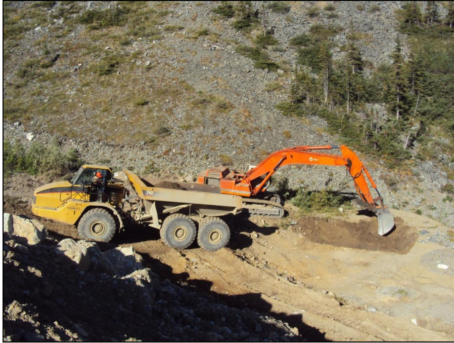
MTN Photograph 19: Excavation of Jewelbox 1380 gully sediment pond.
