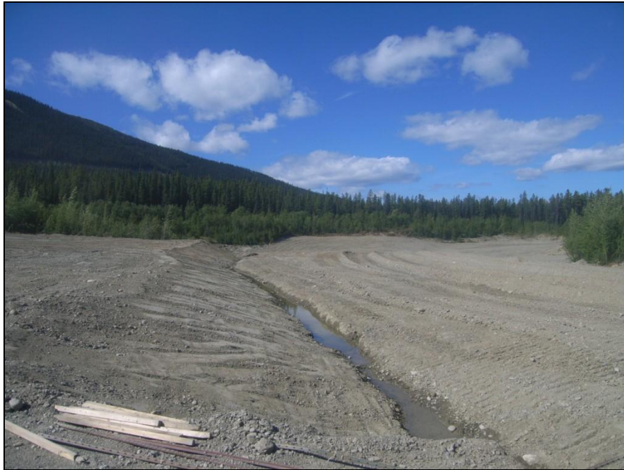
MISC Photograph 11: Surface water drainage channel constructed through landfill area.
