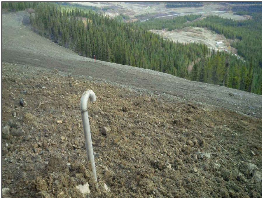
MTN Photograph 18: Jewelbox 1408 ventilation raise completed with stainless steel vent pipe protruding from slope.
