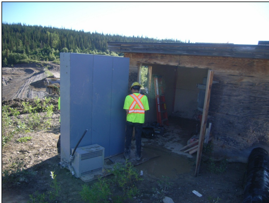
ELEC Photograph 2: CIPC removing electrical panel from Reclaim Dam pump shack.
