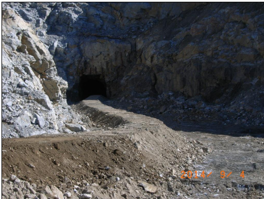
MTN Photograph 8: Jewelbox 1380 Portal plug (pipes contained within berm).
