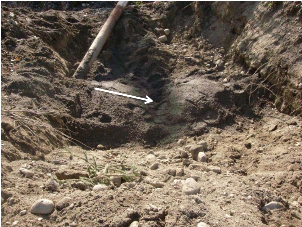
Photo 1: Monitoring Well TH15-91 exposed and cut down.
