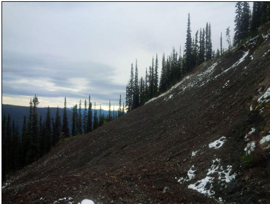
MTN Photograph 28: Reshaped waste rock dump slope at Burnick 1300 level.
