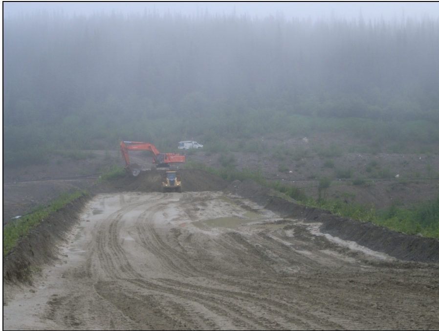
TMA Photograph 3: Excavation of Reclaim Dam.
