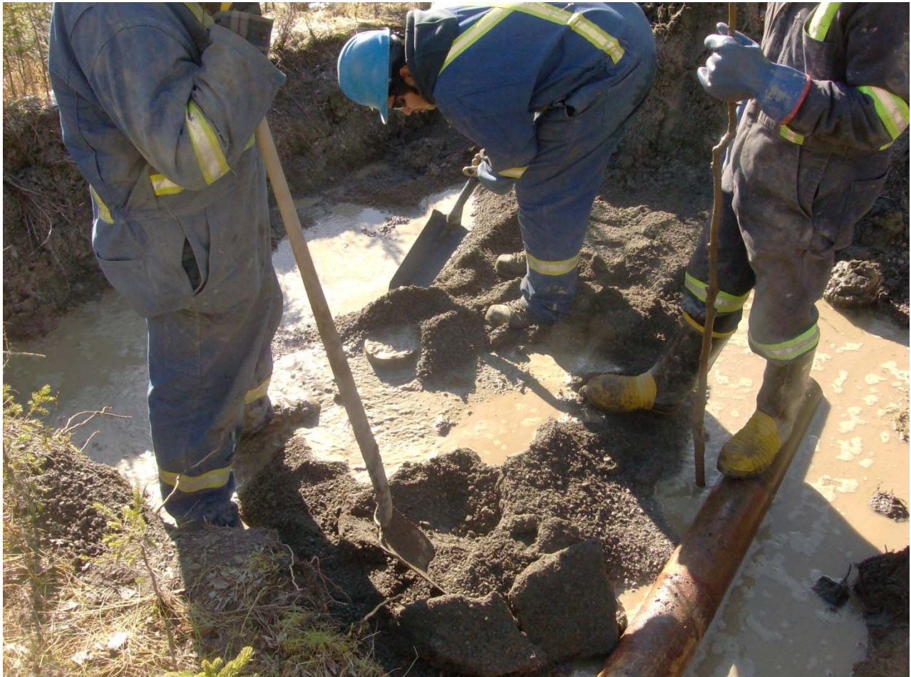
Photo 1: Monitoring Well TH20-91 being filled with sand after being exposed and cut down.
