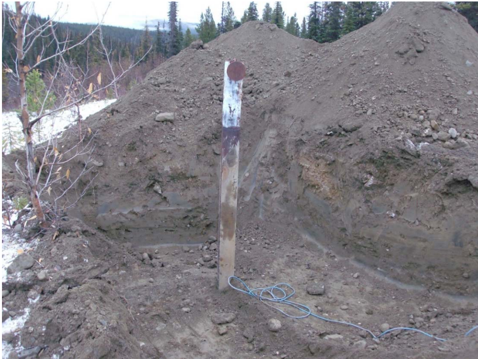
Photo 1: Monitoring Well TH18-91 exposed.
