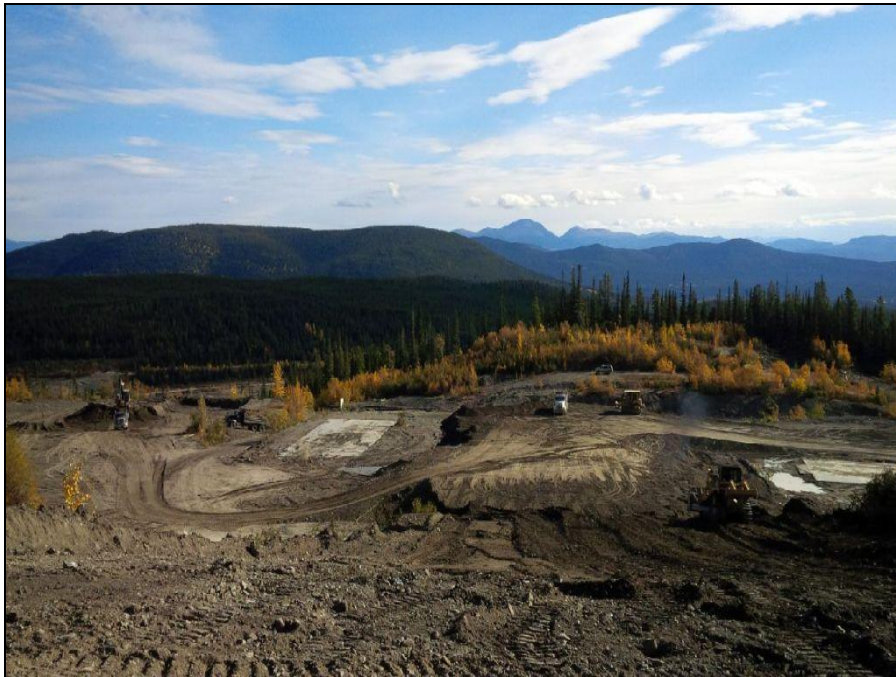
MISC Photograph 14: View of mill capping and shaping operations from former crusher pad.
