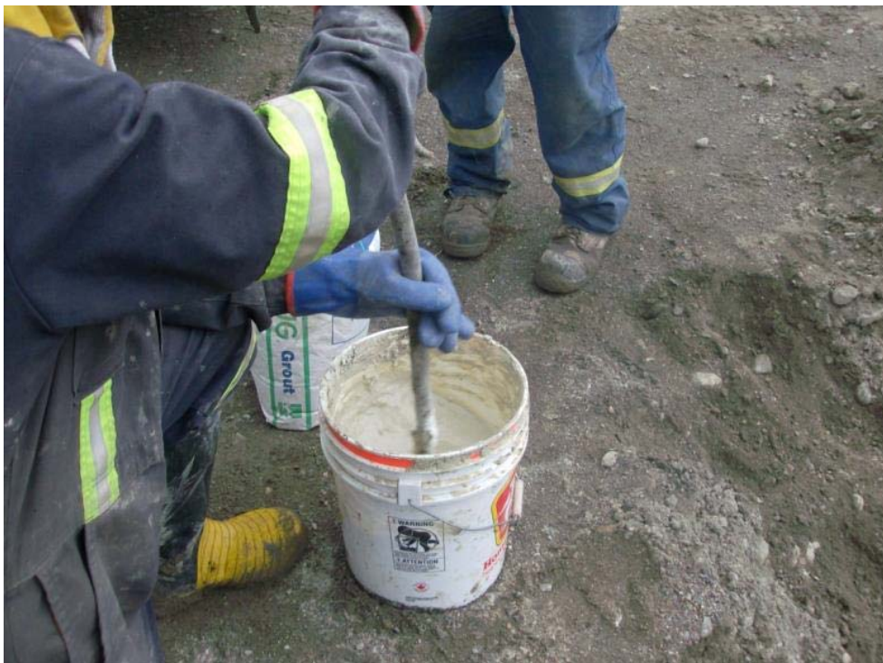
Photo 2: Mixing grout to cap TH01-91.
