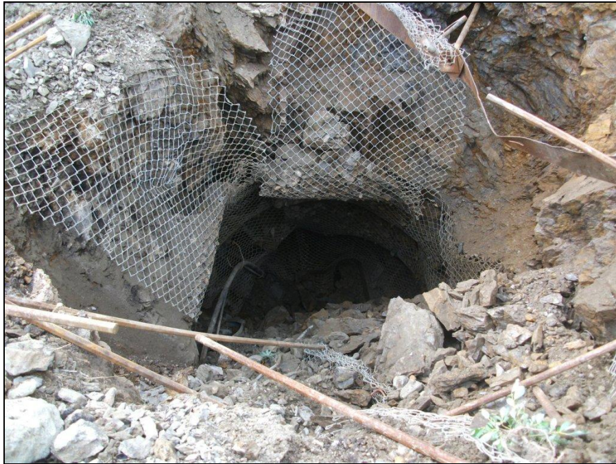
MTN Photograph 17: Jewelbox 1408 ventilation raise (before).
