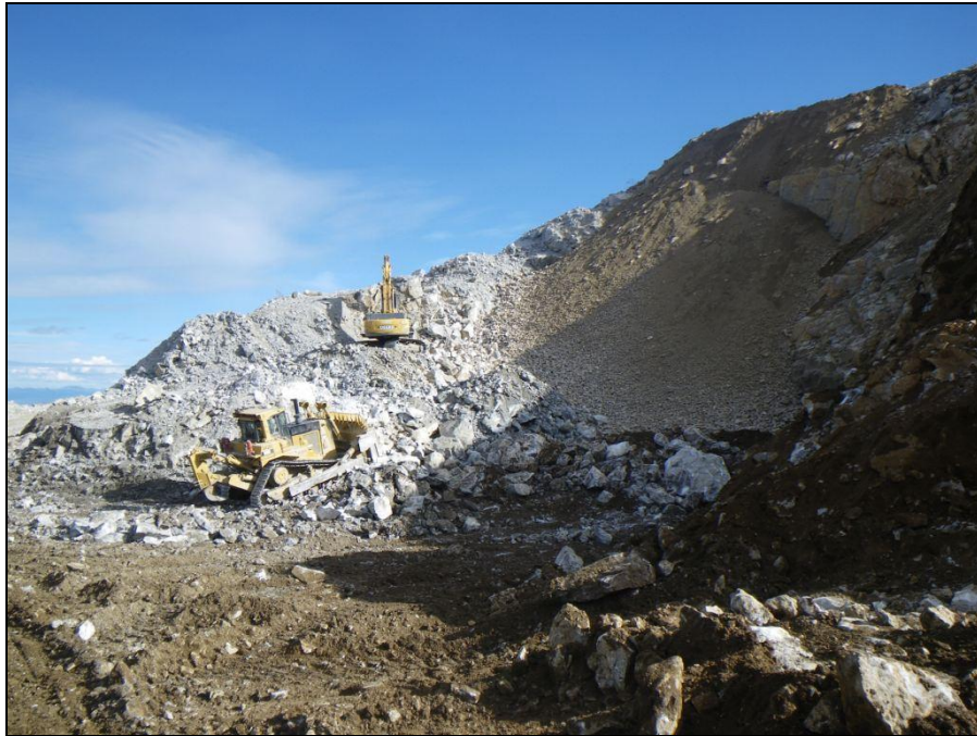
MTN Photograph 9: Main Zone Open Pit infilling operations nearing completion. Jewelbox 1380 Portal plug now buried beneath open pit infill material.
