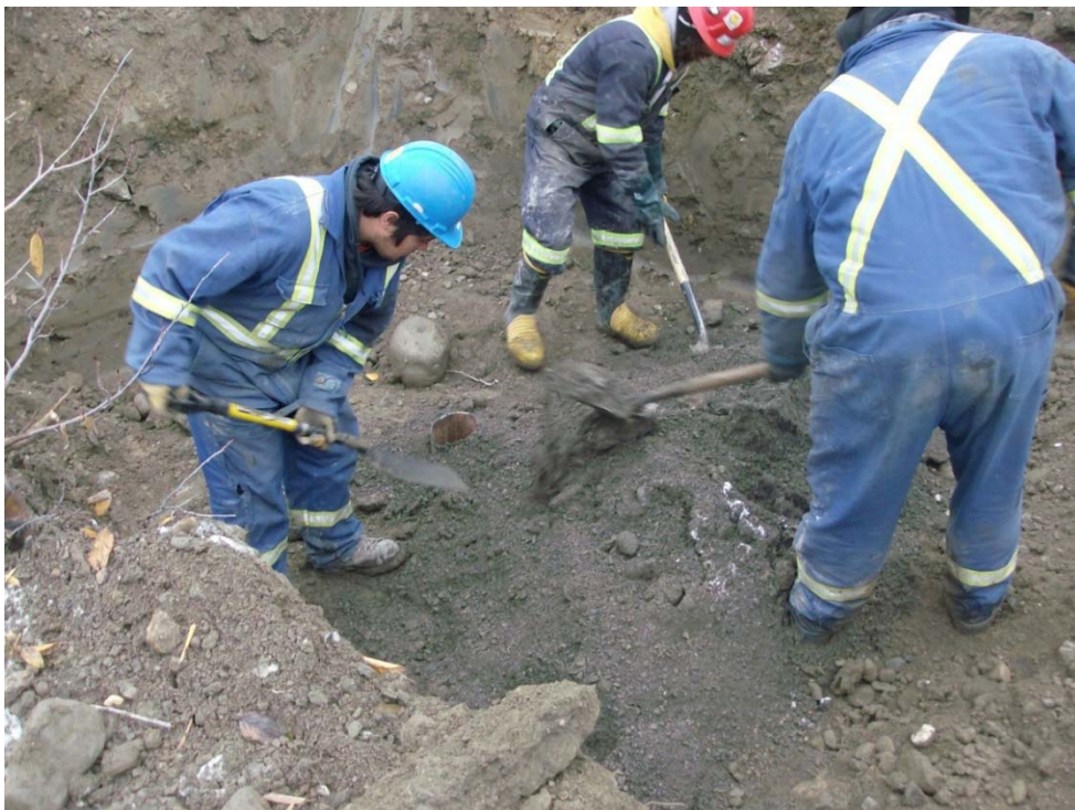
Photo 2: Sand being installed into TH18-91.
