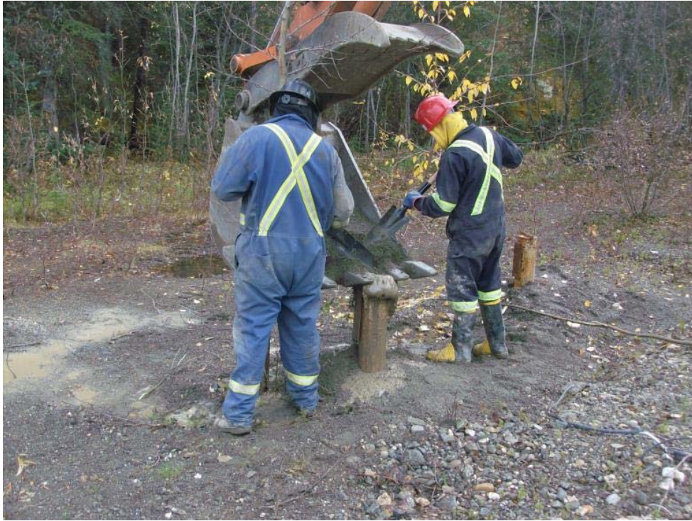
Photo 1: Adding sand to monitoring well TH07-91.
