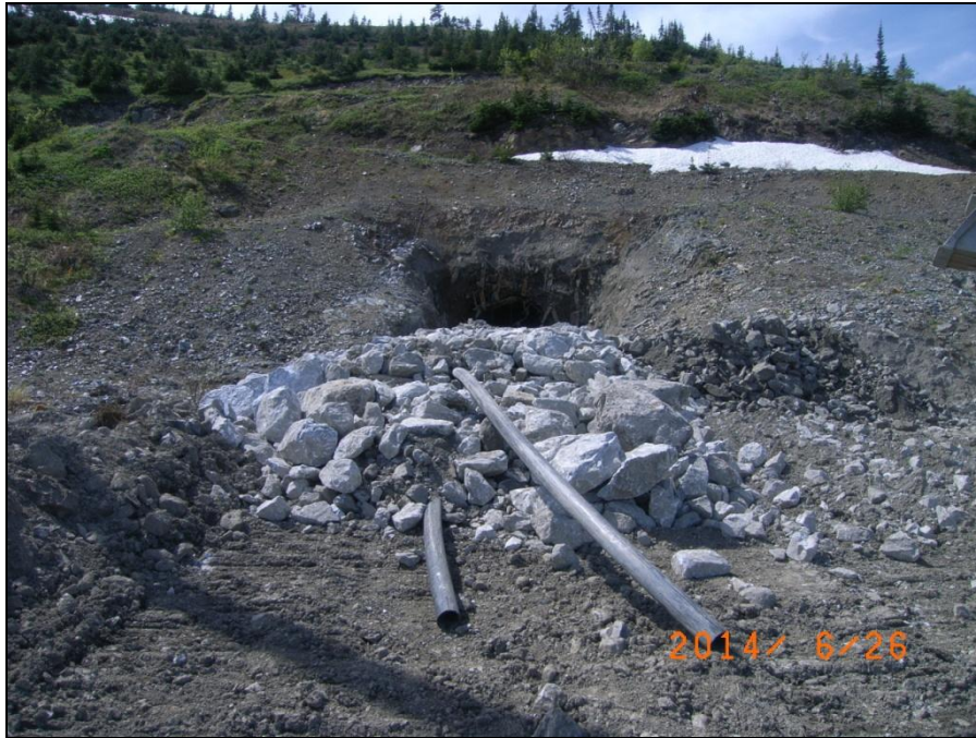
MTN Photograph 11: Jewelbox 1408 Portal plug construction in progress.
