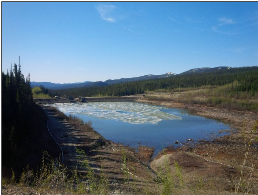
TMA Photograph 2: Reclaim Pond during dewatering operations.
