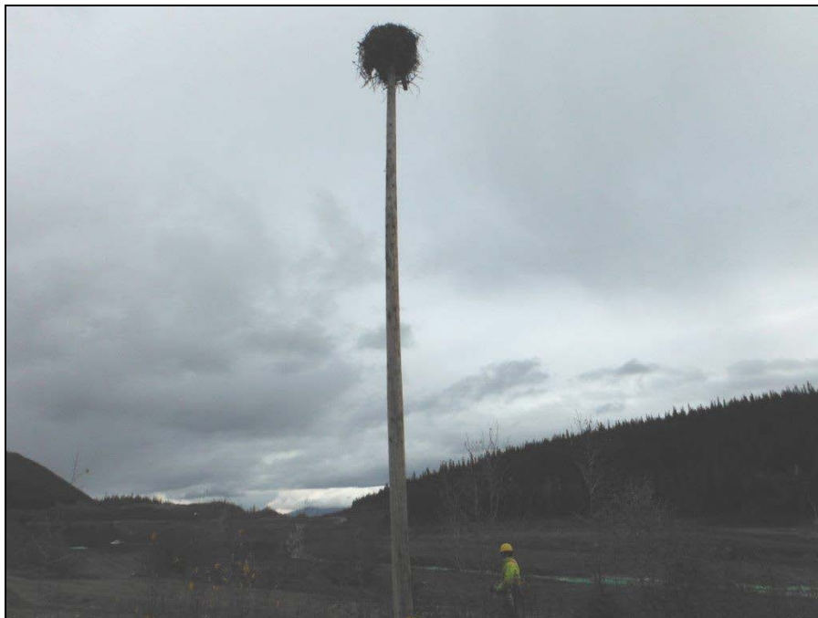
ELEC Photograph 10: One pole (with osprey nest) remains near former Reclaim Dam pump shack.
