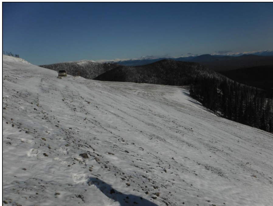
MTN Photograph 2: Jewelbox waste rock dump reshaping completed – angle 1.
