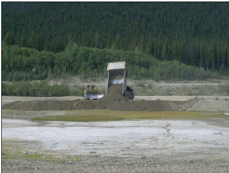
TMA Photograph 12: Capping of North Tailings Pond with excavated dam material.
