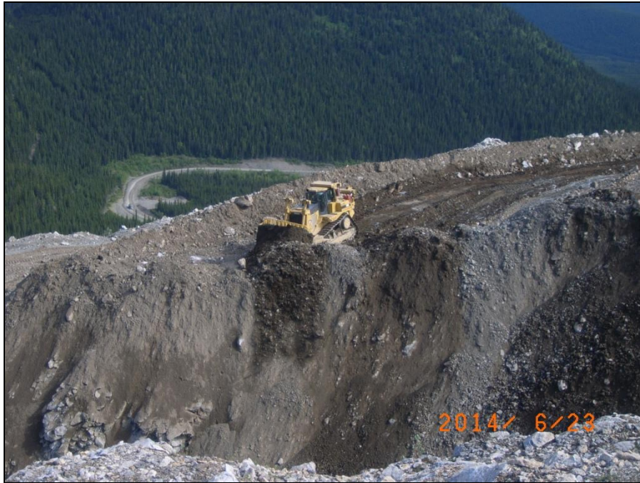
MTN Photograph 5: Jewelbox Open Pit infilling operations.
