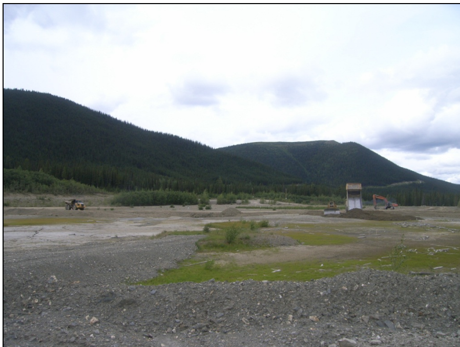
TMA Photograph 10: Capping of North Tailings Pond with excavated dam material.
