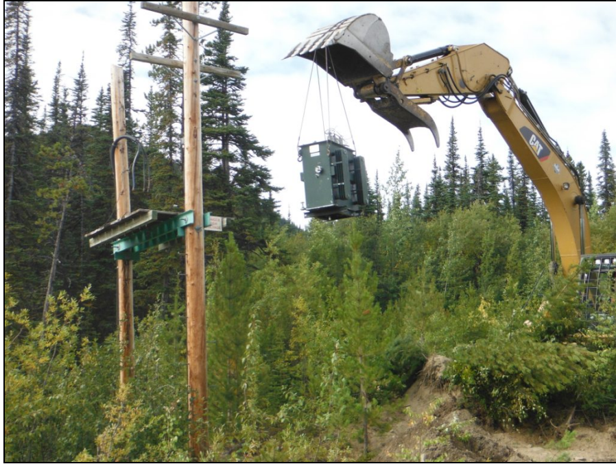
ELEC Photograph 7: Decommissioning of above-ground transformer near North Creek Dyke.
