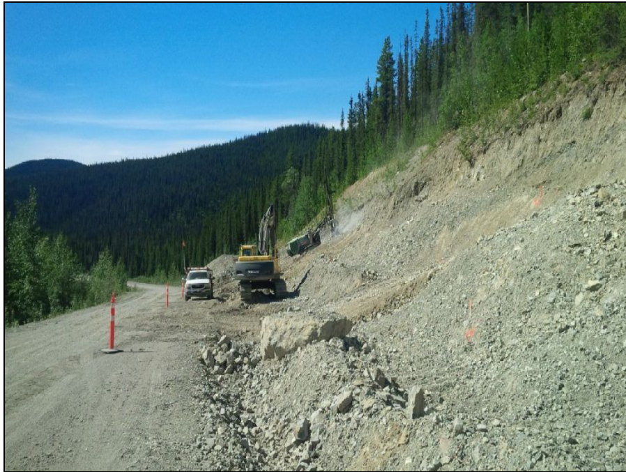
TMA Photograph 6: Drilling operations at km 17 quarry.
