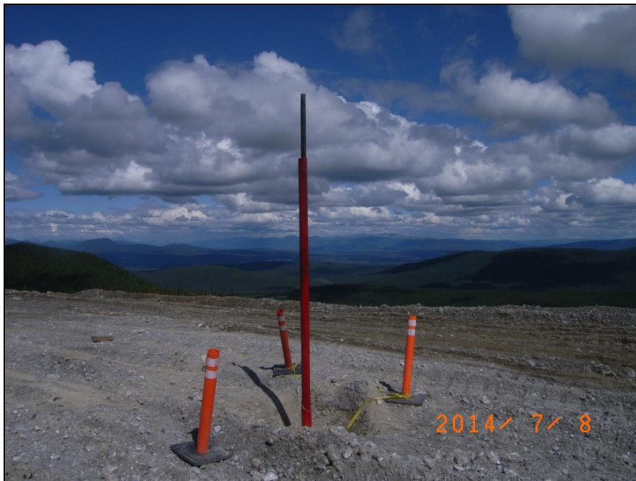
MTN Photograph 6: Extension of monitoring well MW13-03 which lies in footprint of reshaped Jewelbox Waste Rock Dump.
