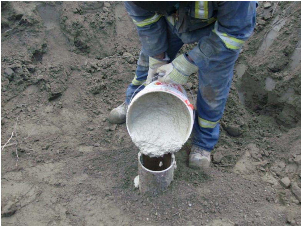
Photo 2: Adding grout to cap TH13-91.
