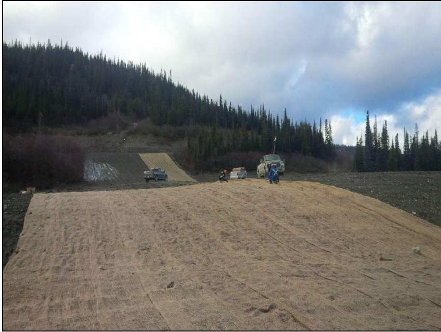
MISC Photograph 17: Rolled erosion control blanket installation at reshaped mill site.
