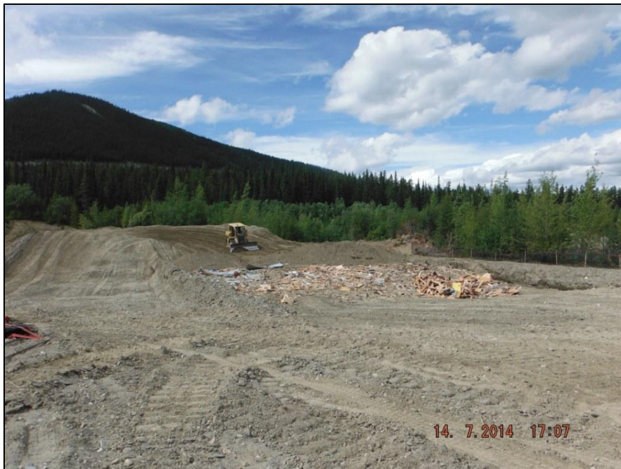
MISC Photograph 10: Crushing and capping activities at landfill.
