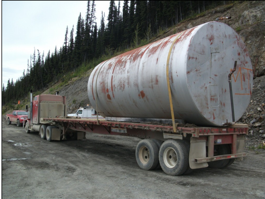
TANK Photograph 1: Diesel tank from Burnick 1200 level loaded onto truck for off-site disposal.
