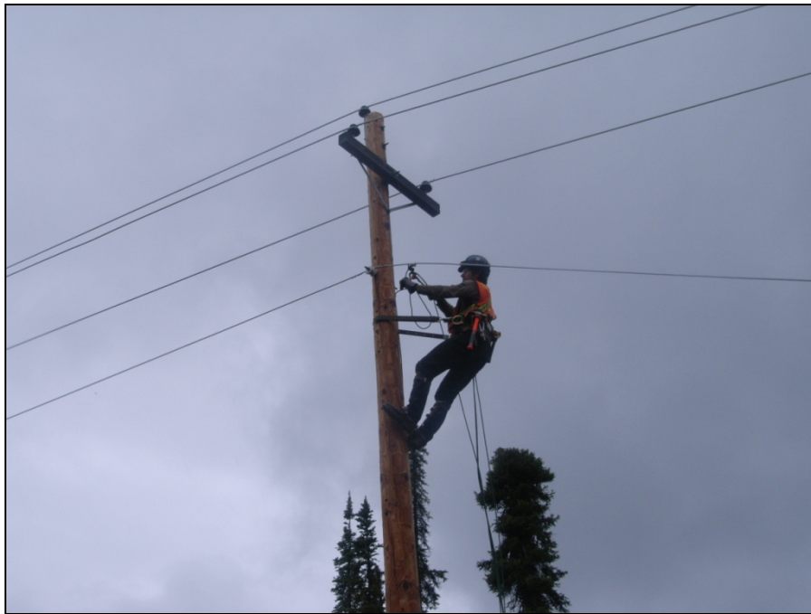
ELEC Photograph 1: CIPC technician disconnecting cable from power pole.
