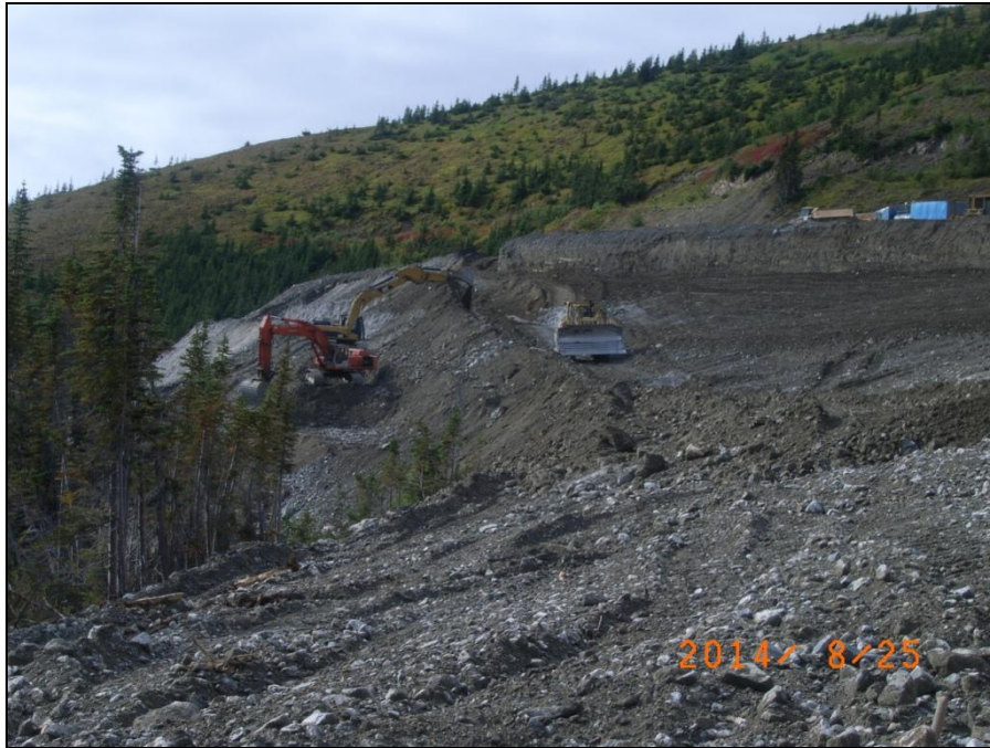
MTN Photograph 3: Jewelbox waste rock dump reshaping in progress – angle 2.
