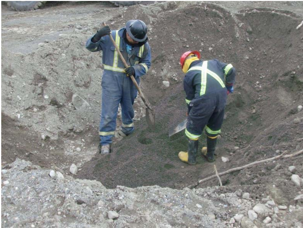
Photo 1: Monitoring Well TH01-91 being filled with sand after being exposed and cut down.
