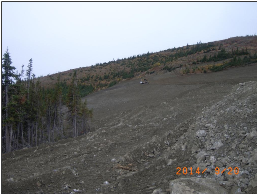
MTN Photograph 4: Jewelbox waste rock dump reshaping nearing completion – angle 2.
