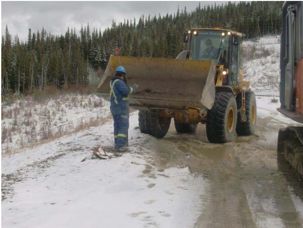
Photo 1: Loading sand into monitoring well TH14-91.
