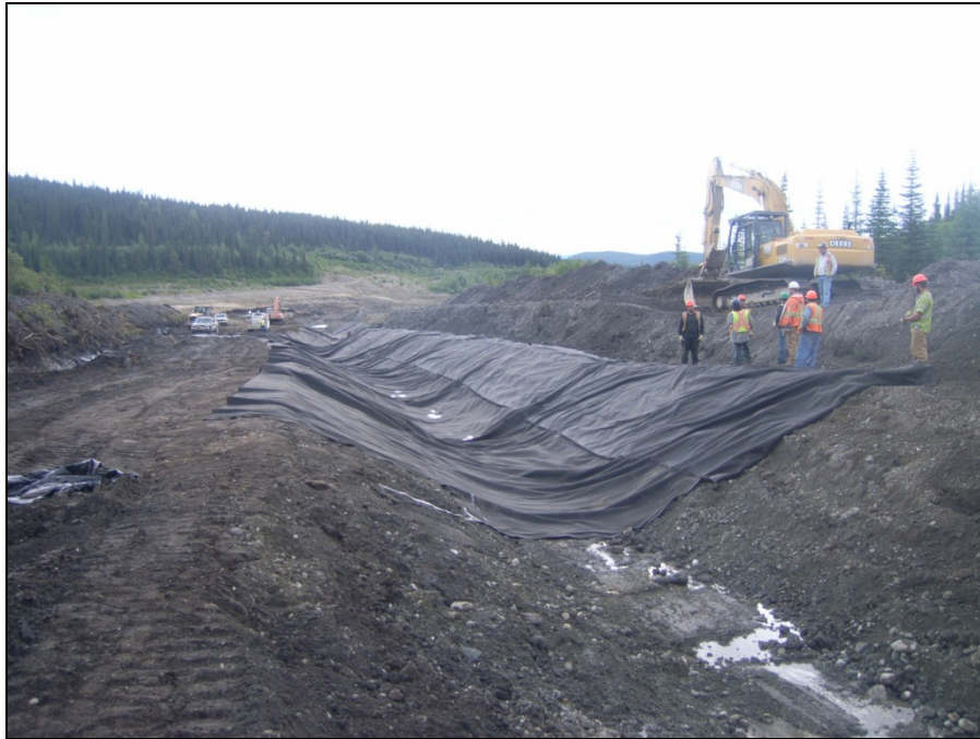
TMA Photograph 11: Installing geotextile in Camp Creek Drainage Channel.
