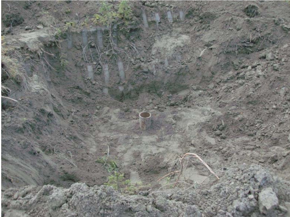
Photo 1: Monitoring Well TH13-91 exposed and cut down.
