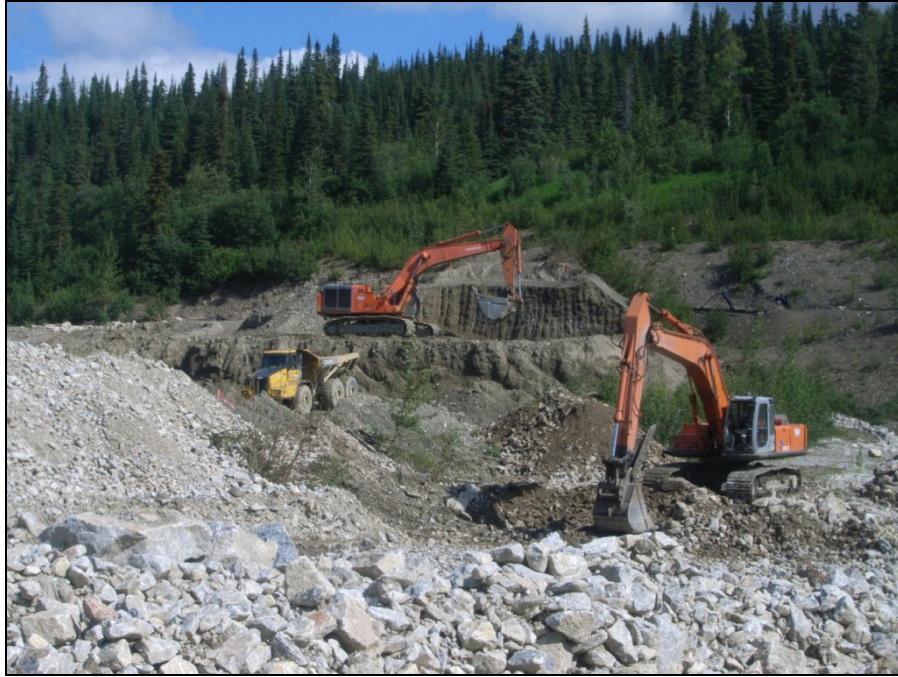
TMA Photograph 5: Reclaim Dam excavation and salvage of toe buttress riprap.
